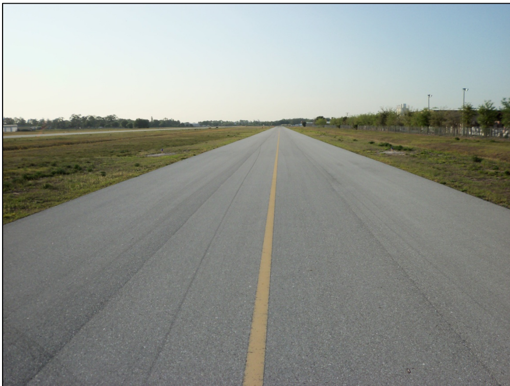
Taxiway Alpha, Section 105, Sample Unit 109 – Low severity (52) Weathering and Raveling
