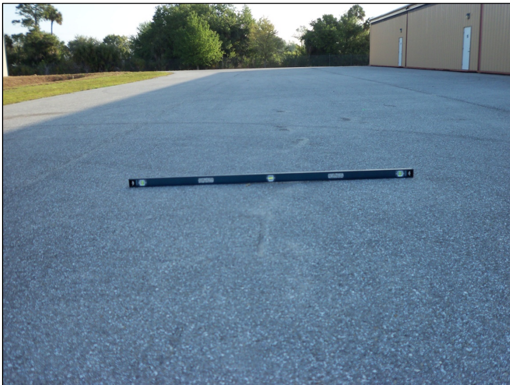
Hangars, Section 4305, Sample Unit 202 – Low severity (45) Depression, low severity (48) Longitudinal and Transverse Cracking, low and medium severity (52) Weathering and Raveling
