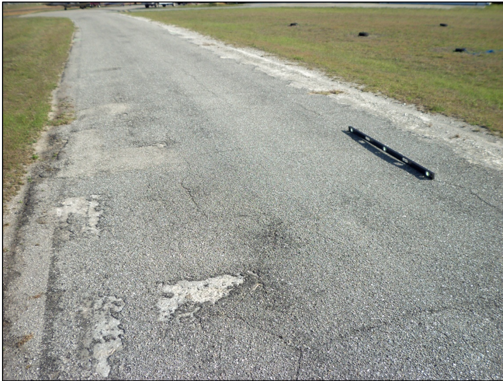
Taxiway NW Apron, Section 605, Sample Unit 101 – Low severity (43) Block Cracking, low severity (48) Longitudinal and Transverse Cracking, medium and high severity (52) Weathering and Raveling, low severity (56) Swell
