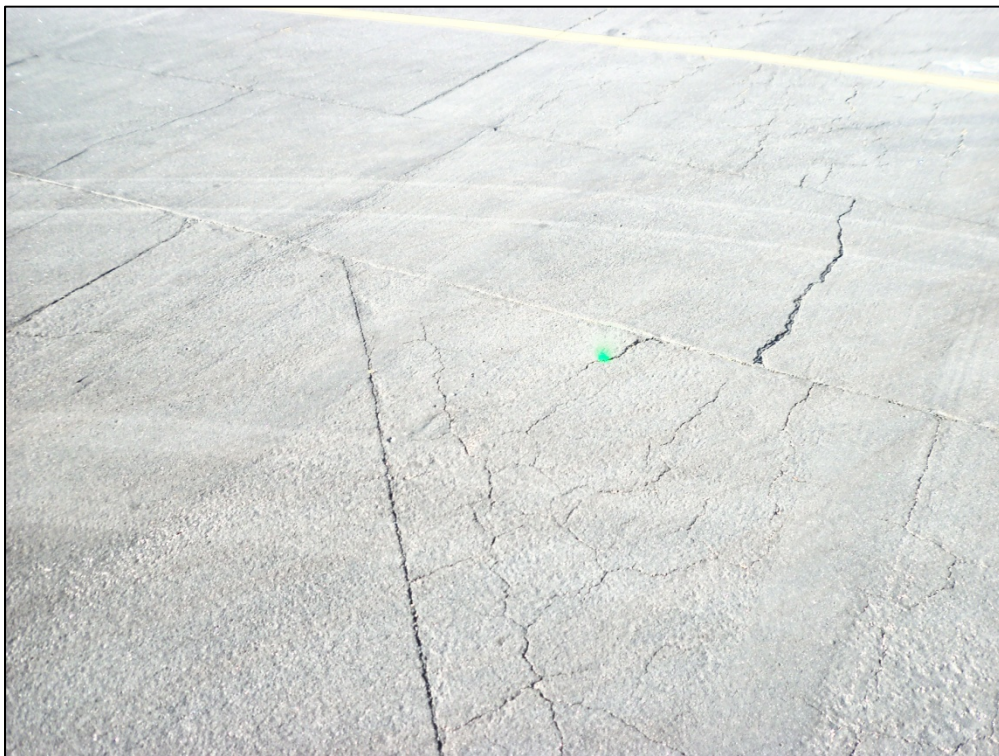
Apron, Section 4110, Sample Unit 505 – Low and medium severity (48) Longitudinal and Transverse Cracking, low and medium severity (52) Weathering and Raveling
