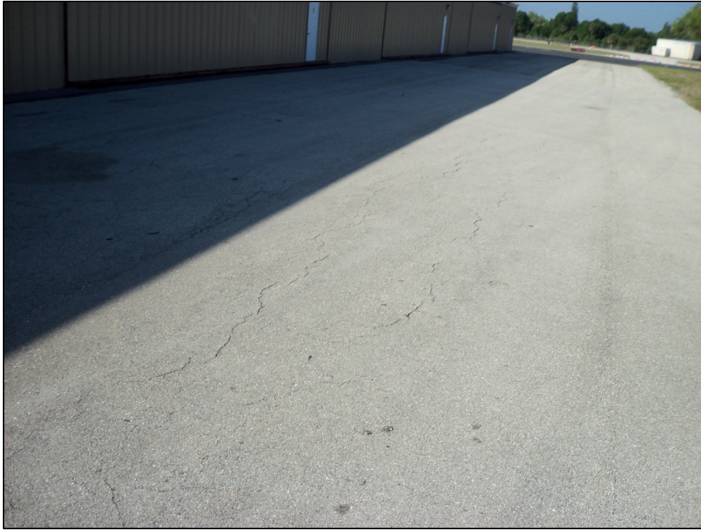
Hangars, Section 4135, Sample Unit 601 – Low severity (43) Block Cracking, low severity (48) Longitudinal and Transverse Cracking, low and medium severity (52) Weathering and Raveling
