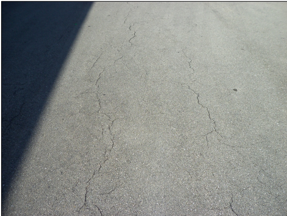
Hangars, Section 4135, Sample Unit 601 – Low severity (43) Block Cracking, low severity (48) Longitudinal and Transverse Cracking, (49) Oil Spillage, low and medium severity (52) Weathering and Raveling
