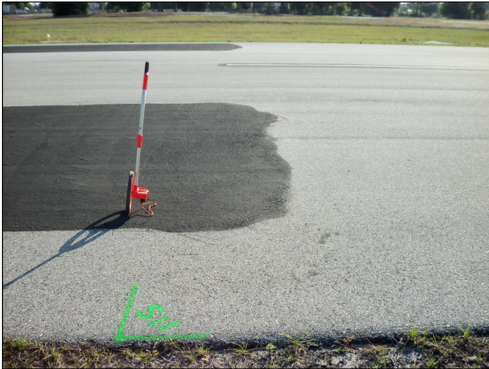
Runway 14-32, Section 6105, Sample Unit 115 – Low severity (48) Longitudinal and Transverse Cracking, low and medium severity (52) Weathering and Raveling
