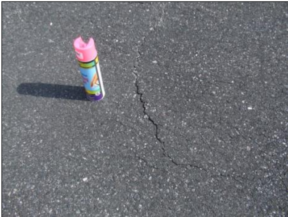
Run Up Apron to Runway 10-28, Section 5125, Sample Unit 105 – Low and medium severity (48) Longitudinal and Transverse Cracking, low severity (52) Weathering and Raveling, low and medium severity (56) Swelling.
