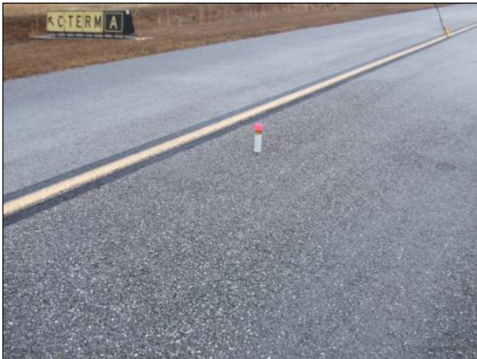
Taxiway Alpha 1, Section 105, Sample Unit 118 – Low severity (48) Longitudinal and Transverse Cracking, low severity (50) Patching, low and medium severity (52) Weathering and Raveling.
