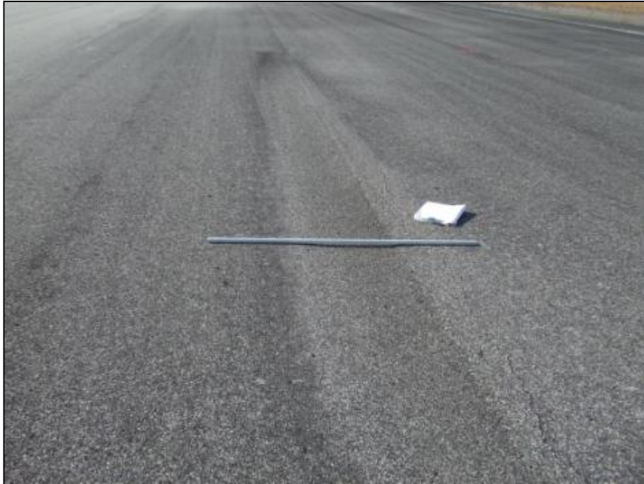
Runway 10-28, Section 6105, Sample Unit 391 – Medium severity (45) Depression, low severity (48) Longitudinal and Transverse Cracking, low severity (50) Patching, low severity (52) Weathering and Raveling, low severity (56) Swelling.
