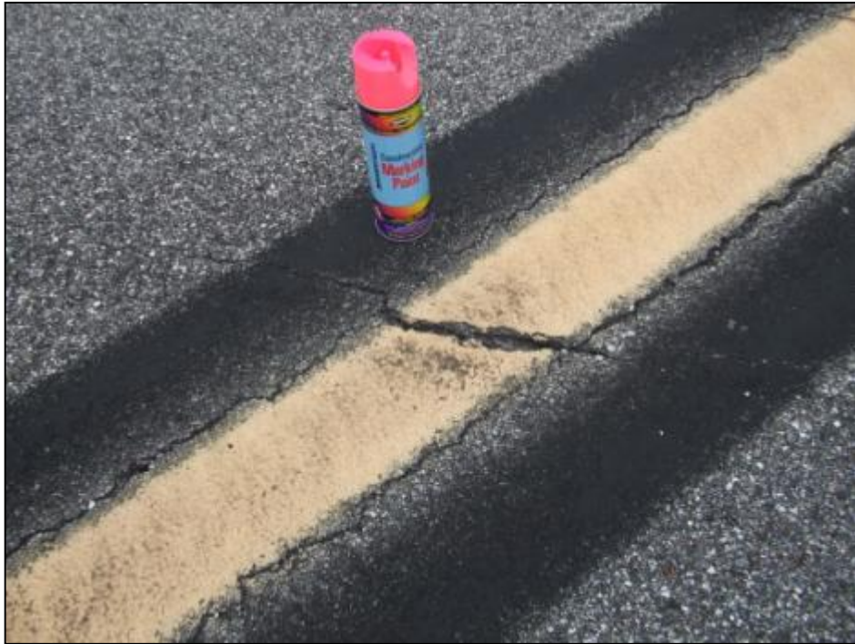
Runway 10-28, Section 6110, Sample Unit 136 – Low and medium severity (48) Longitudinal and Transverse Cracking, medium severity (50) Patching, low severity (52) Weathering and Raveling, low severity (56) Swelling.
