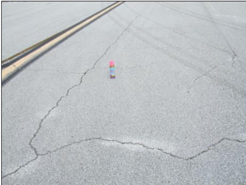
Taxiway Charlie, Section 304, Sample Unit 100 – Low severity (43) Block Cracking, low and medium severity (48) Longitudinal and Transverse Cracking, low severity (50) Patching, low severity (52) Weathering and Raveling.
