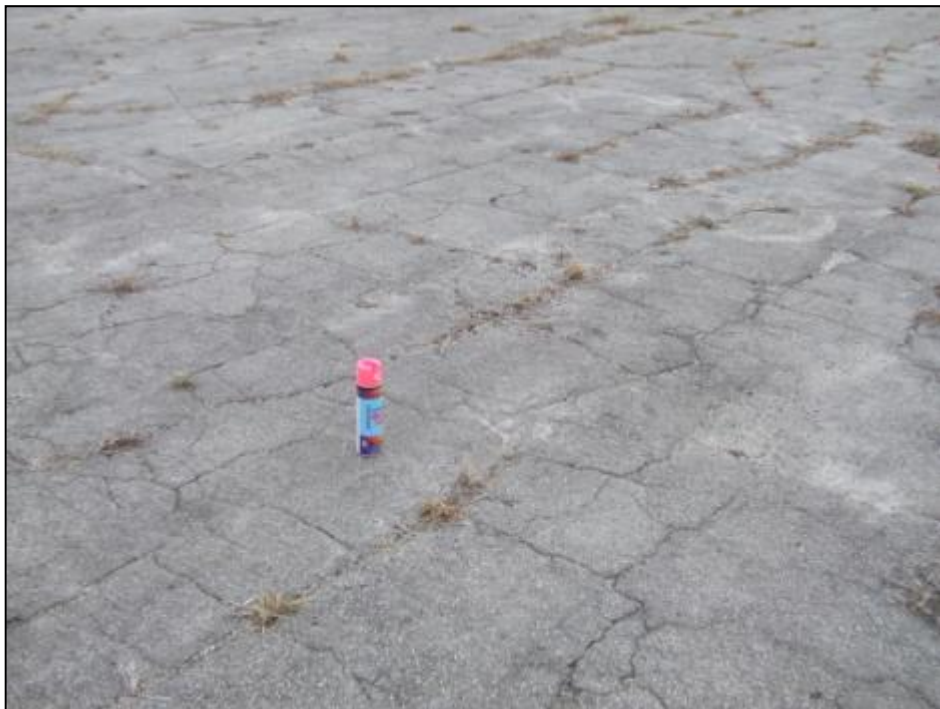
Apron East, Section 4242, Sample Unit 110 – Medium severity (43) Block Cracking, medium severity (50) Patching, medium severity (52) Weathering and Raveling.
