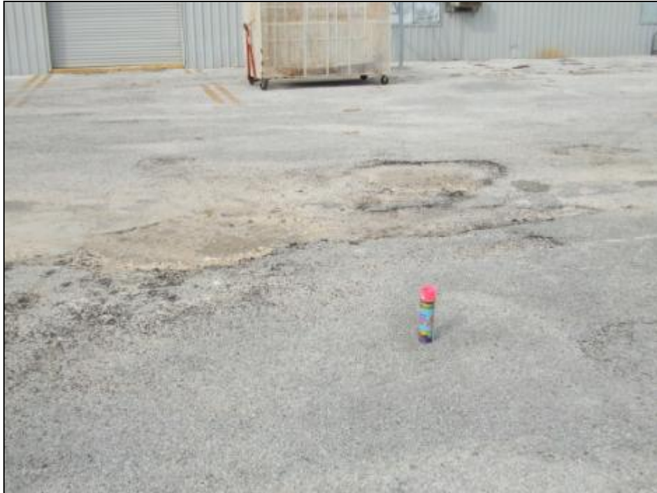
East Apron, Section 4228, Sample Unit 101 – Low and medium severity (45) Depression, low severity (48) Longitudinal and Transverse Cracking, low and medium (50) Patching, medium and high severity (52) Weathering and Raveling.
