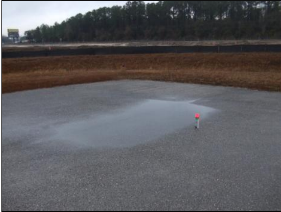
Run Up and Turnaround Apron RW 10-28, Section 5105, Sample Unit 100 – Low severity (45) Depression, low severity (48) Longitudinal and Transverse Cracking, low severity (50) Patching, low severity (52) Weathering and Raveling.
