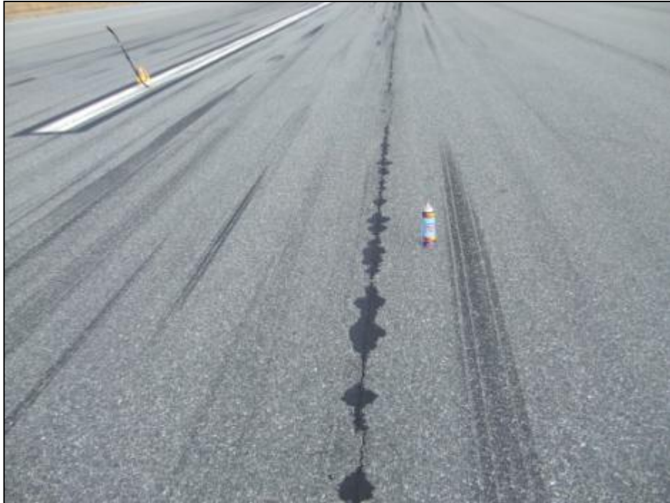
Runway 10-28, Section 6114, Sample Unit 423 – Low severity (42) Bleeding, low and medium severity (48) Longitudinal and Transverse Cracking, low severity (52) Weathering and Raveling.
