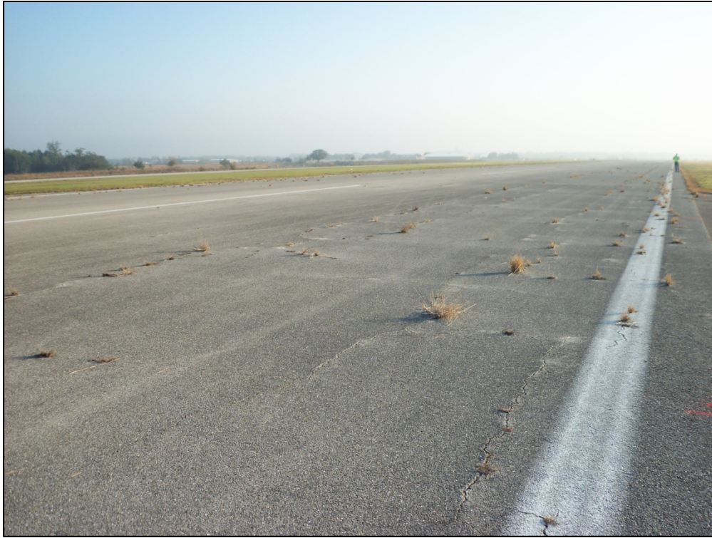
Runway 6-24, Section 6105, Sample Unit 103 – Low and medium severity (43) Block Cracking, low and medium severity (48) Longitudinal and Transverse Cracking, low severity (52) Weathering and Raveling
