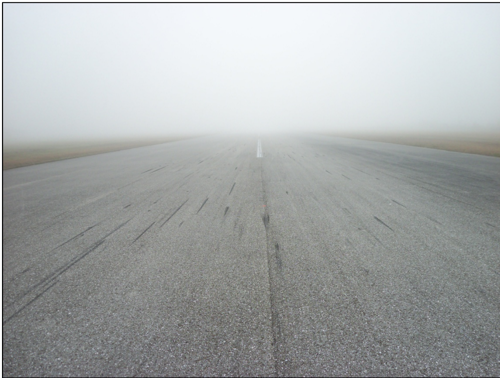
Runway 17-35, Section 6205, Sample Unit 166 – Low severity (48) Longitudinal and Transverse Cracking, low severity (52) Weathering and Raveling
