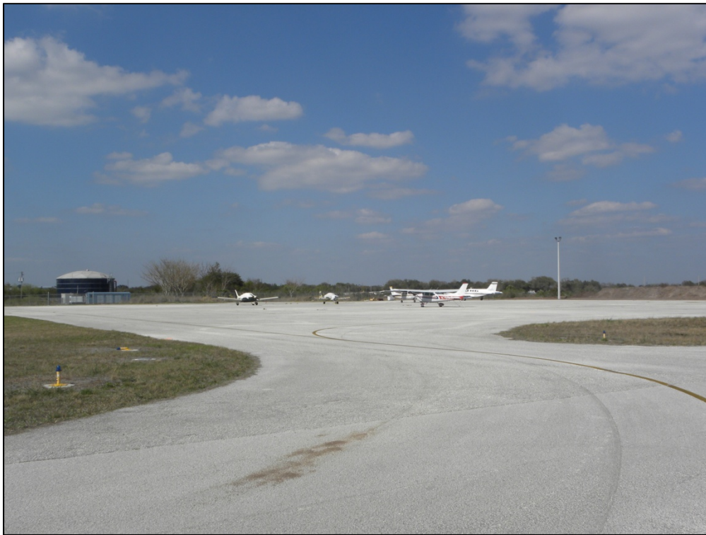
Apron, Section 110, Sample Unit 100 – Low severity (48) Longitudinal and Transverse Cracking, medium severity (52) Weathering and Raveling
