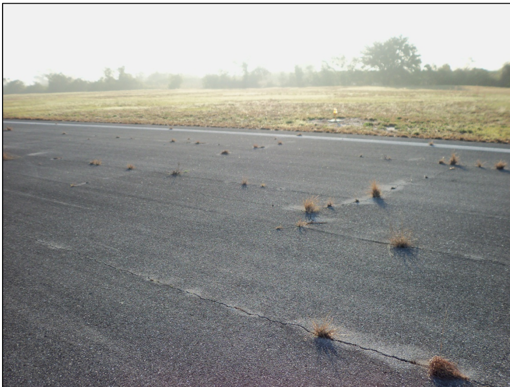
Runway 6-24, Section 6105, Sample Unit 107 – Low severity (43) Block Cracking, low severity (48) Longitudinal and Transverse Cracking, low severity (52) Weathering and Raveling
