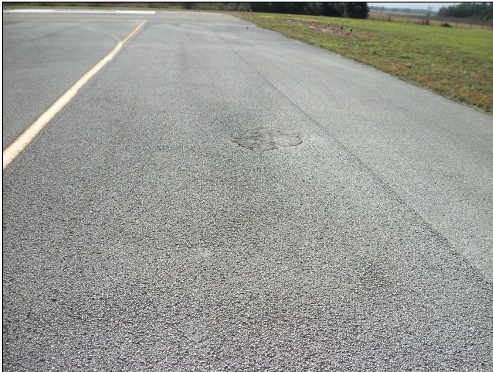
Taxiway Delta, Section 410, Sample Unit 100 – Low severity (43) Block Cracking, low severity (48) Longitudinal and Transverse Cracking, low severity (50) Patch, low severity (52) Weathering and Raveling
