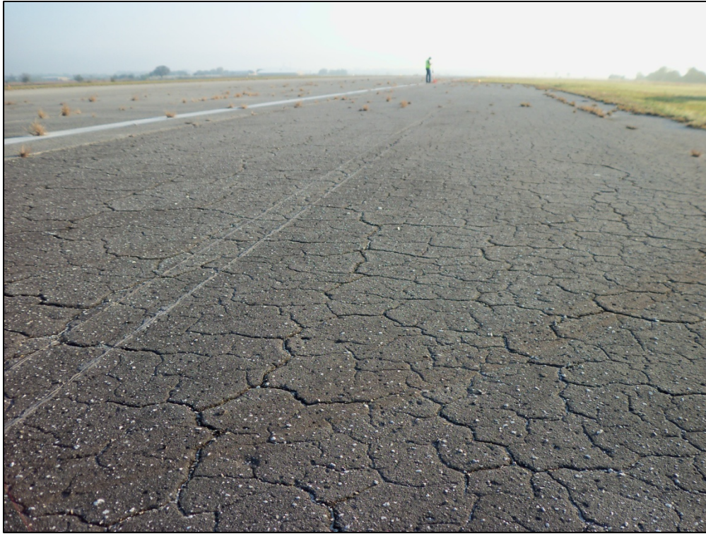
Runway 6-24 Shoulder, Section 5102, Sample Unit 181 – Medium severity (43) Block Cracking, medium severity (52) Weathering and Raveling
