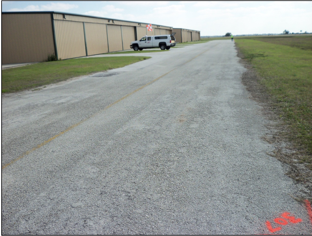
Hangars, Section 4110, Sample Unit 307 – Low and medium severity (52) Weathering and Raveling
