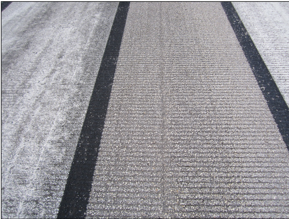
Runway 9-27, Section 6105, Sample Unit 302 – Medium severity (52) Weathering and Raveling
