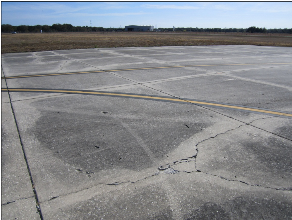
Taxiway Lima, Section 520, Sample Unit 125 – Low severity (70) Scaling, Crazeing, and Map Cracking, low severity (74) Joint Spalling, medium severity (72) Shattered Slab, low severity (63) Linear Cracking
