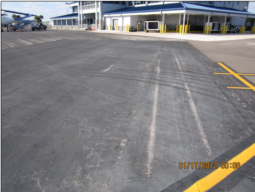
Northeast Apron, Section 4140, Sample Unit 203 – Low severity (52) Weathering and Raveling, low severity (43) Block Cracking
