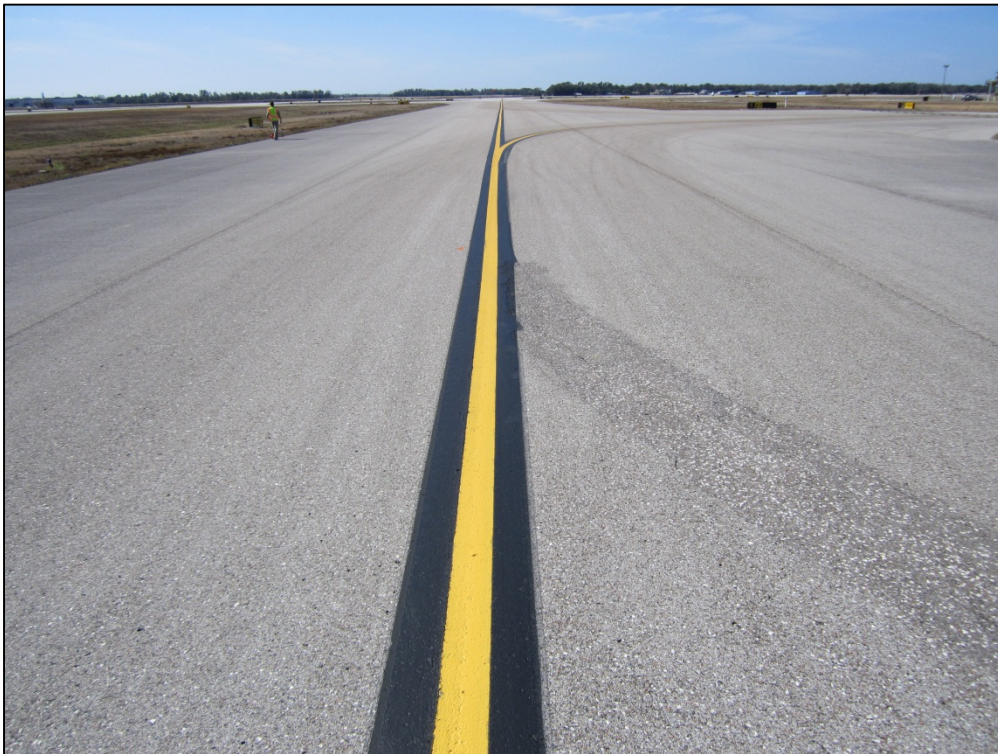
Taxiway Bravo, Section 210, Sample Unit 217 – Low severity (52) Weathering and Raveling
