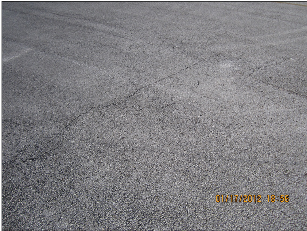
Taxiway Sierra, Section 905, Sample Unit 915 – Low severity (48) Longitudinal and Transverse Cracking, low severity (52) Weathering and Raveling
