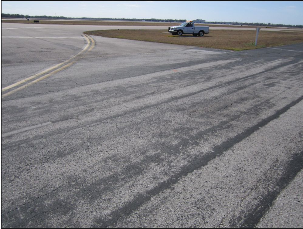
Northeast Apron, Section 4215, Sample Unit 200 – Low severity (52) Weathering and Raveling, low severity (53) Rutting, low severity (43) Block Cracking, low severity (48) Longitudinal and Transverse Cracking
