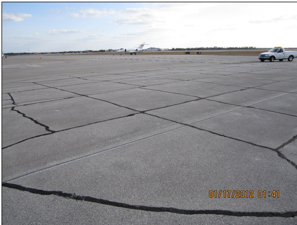
North Apron, Section 4110, Sample Unit 700 – Medium severity (47) Joint Reflection Cracking, medium severity (48) Longitudinal and Transverse Cracking, low severity (52) Weathering and Raveling
