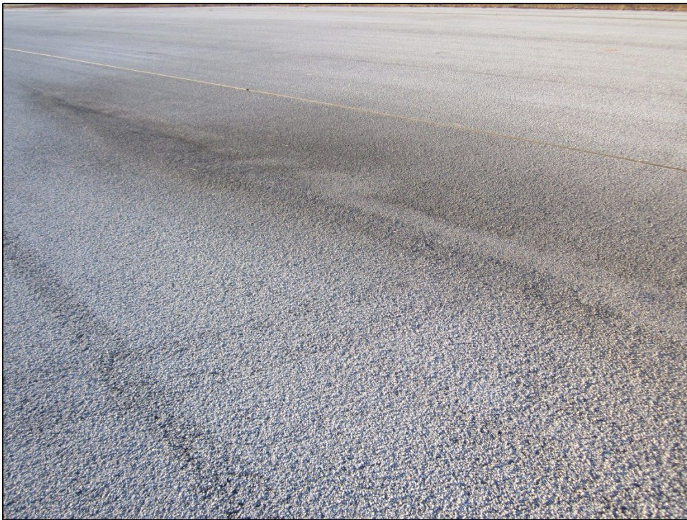
South Apron, Section 4505, Sample Unit 305 – Medium severity (52) Weathering and Raveling, low severity (48) Longitudinal and Transverse Cracking, low severity (45) Depression
