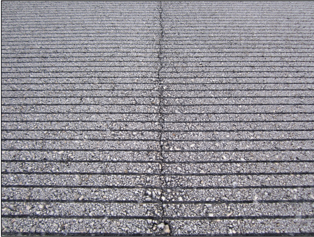
Runway 9-27, Section 6150, Sample Unit 443 – Low severity (48) Longitudinal and Transverse Cracking
