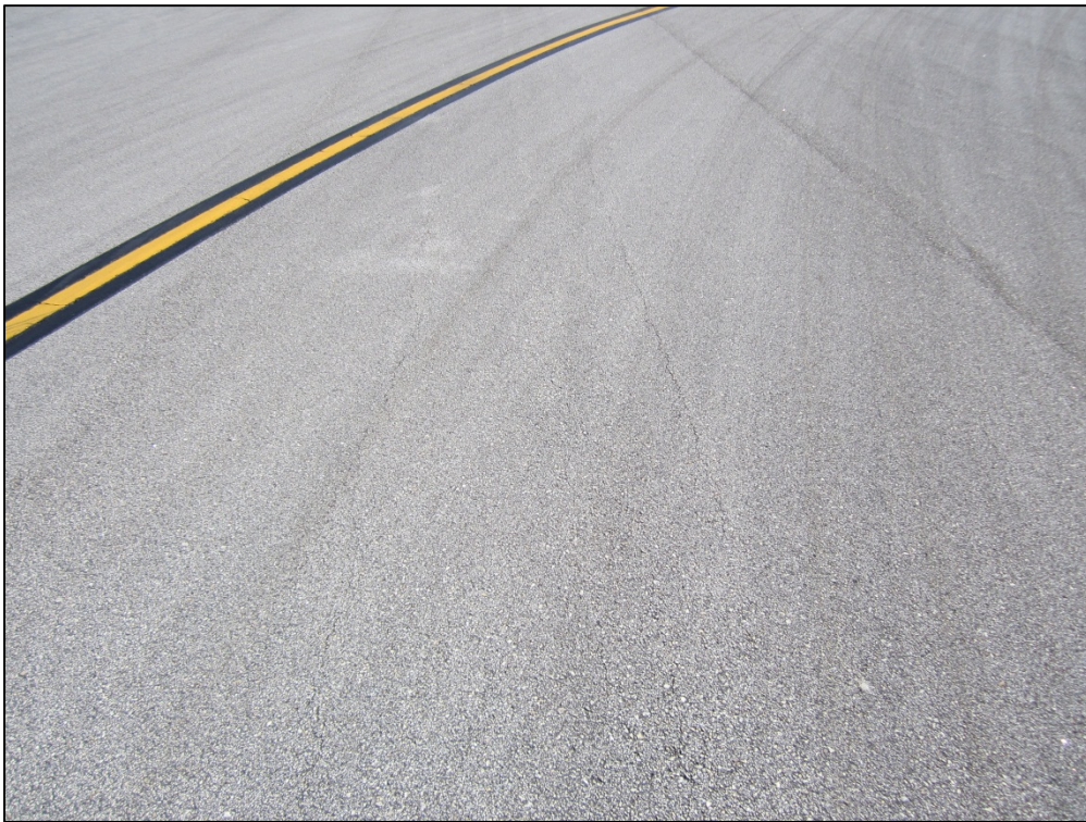
Taxiway Alpha, Section 150, Sample Unit 227 – Low severity (48) Longitudinal and Transverse Cracking, low severity (52) Weathering and Raveling
