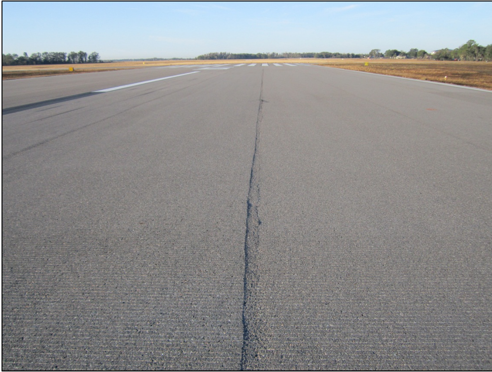
Runway 5-23, Section 6215, Sample Unit 310 – Low severity (48) Longitudinal and Transverse Cracking, low severity (52) Weathering and Raveling
