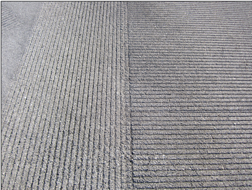
Runway 5-23, Section 6260, Sample Unit 560 – Low severity (52) Weathering and Raveling
