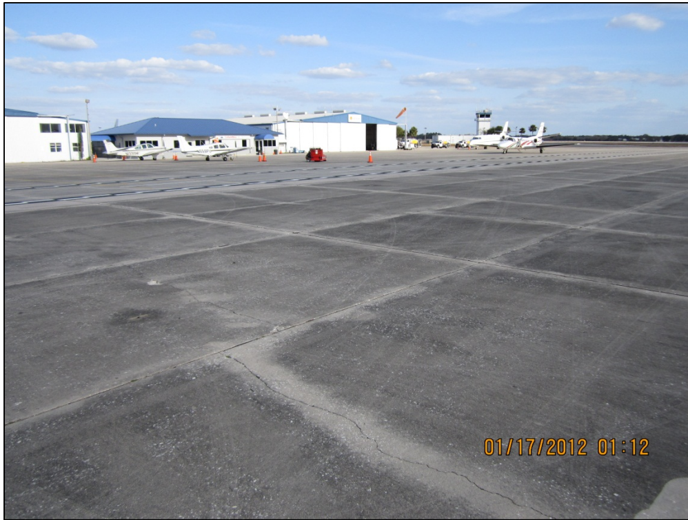
North Apron, Section 4120, Sample Unit 500 – Low severity (63) Longitudinal, Transverse, and Diagonal Cracking, low severity (70) Scaling, Craziing, and Map Cracking
