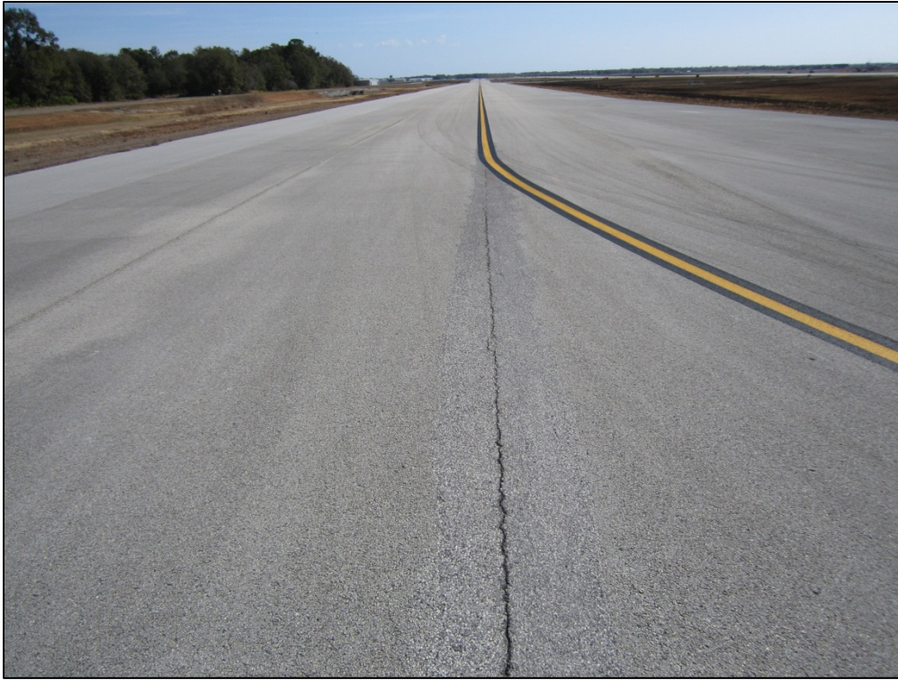
Taxiway Alpha, Section 105, Sample Unit 102 – Low severity (48) Longitudinal and Transverse Cracking, low severity (52) Weathering and Raveling
