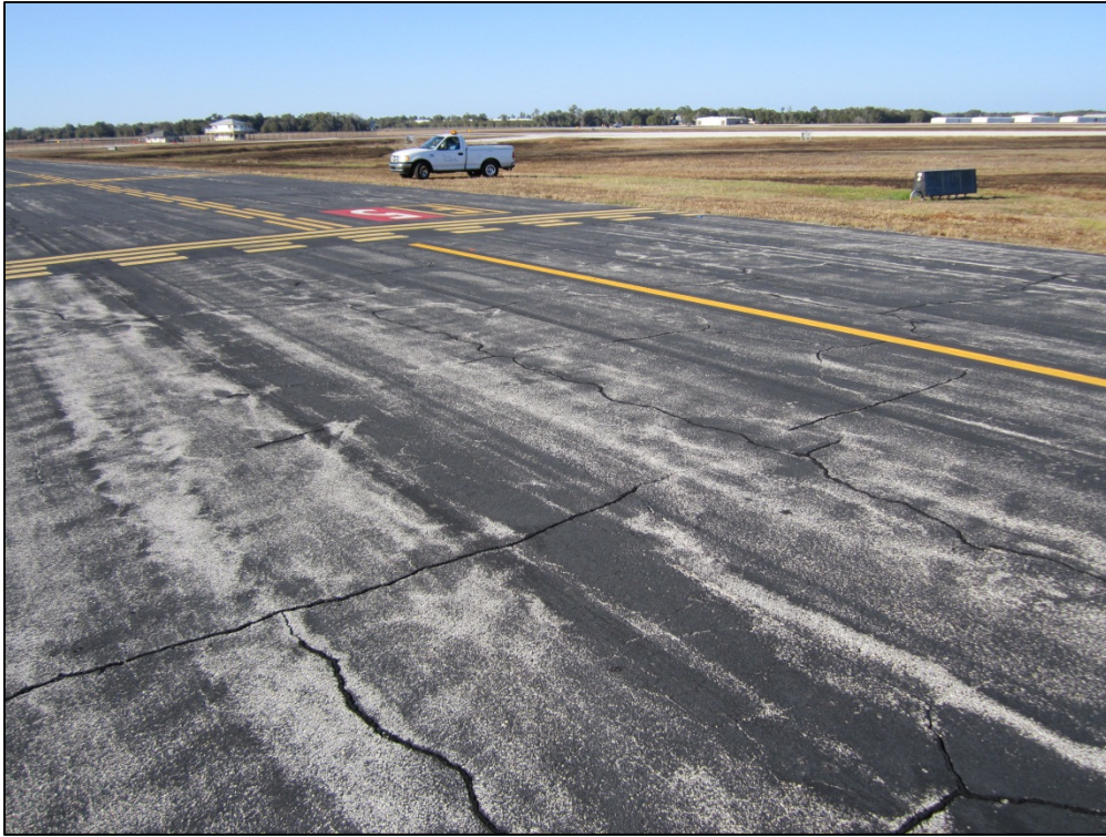
Taxiway Foxtrot, Section 615, Sample Unit 602 – Low severity (43) Block Cracking
