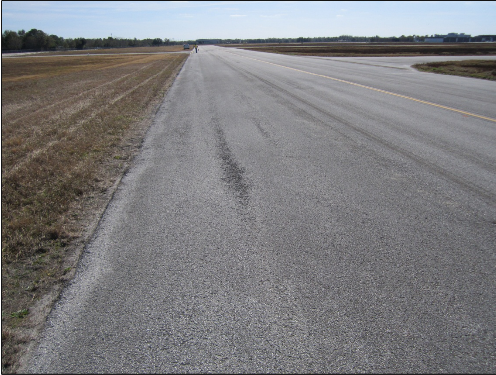
Taxiway Echo, Section 525, Sample Unit 403 – Low severity (48) Longitudinal and Transverse Cracking, low and medium severity (52) Weathering and Raveling
