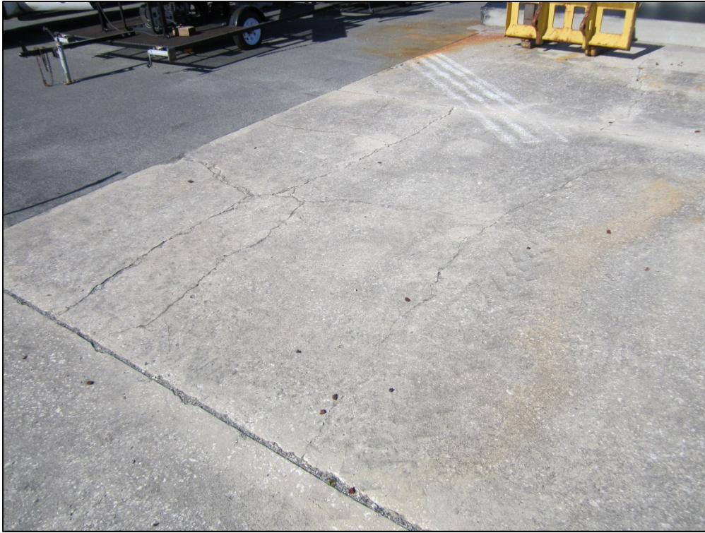
Taxiway Charlie, Section 322, Sample Unit 203 – Medium severity (72) Shattered Slab
