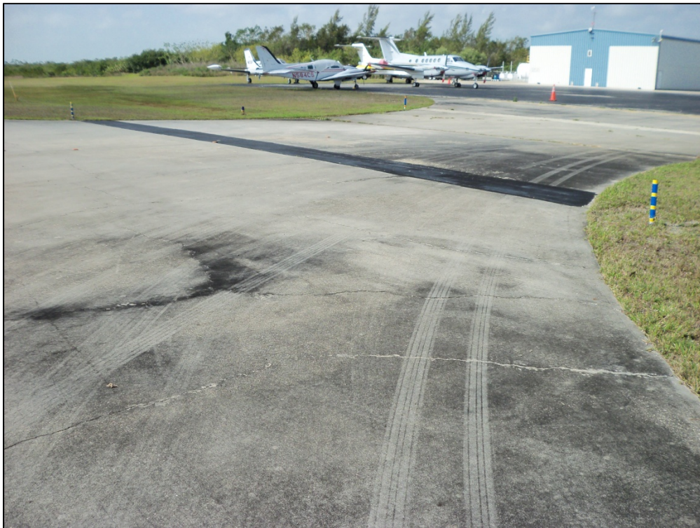
Taxiway Connector, Section 105, Sample Unit 100 – Low severity (63) LTD Cracking, medium severity (66) Patch, low severity (70) Scaling/Map Cracking, medium severity (72) Shattered Slabs, (73) Shrinkage Cracks, low severity (74) Joint Spalling
