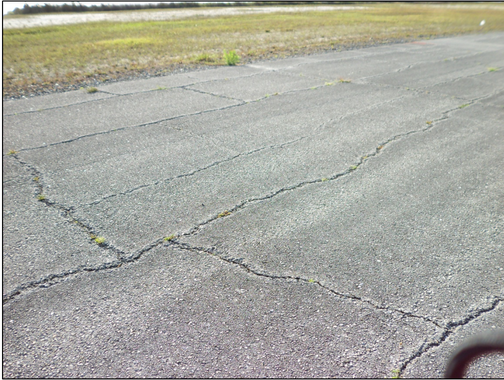
Runway 17-35, Section 6110, Sample Unit 145 – Medium severity (43) Block Cracking, medium severity (52) Weathering and Raveling
