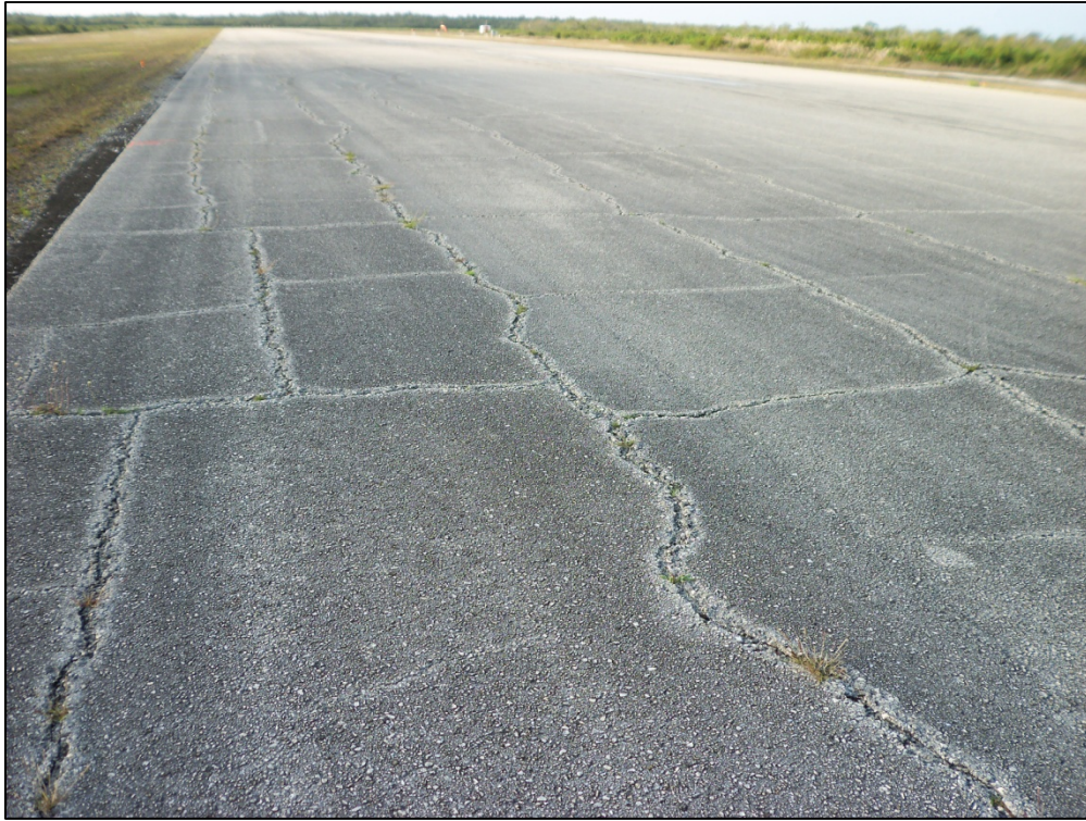
Runway 17-35, Section 6110, Sample Unit 130 – Medium severity (43) Block Cracking, medium severity (52) Weathering and Raveling
