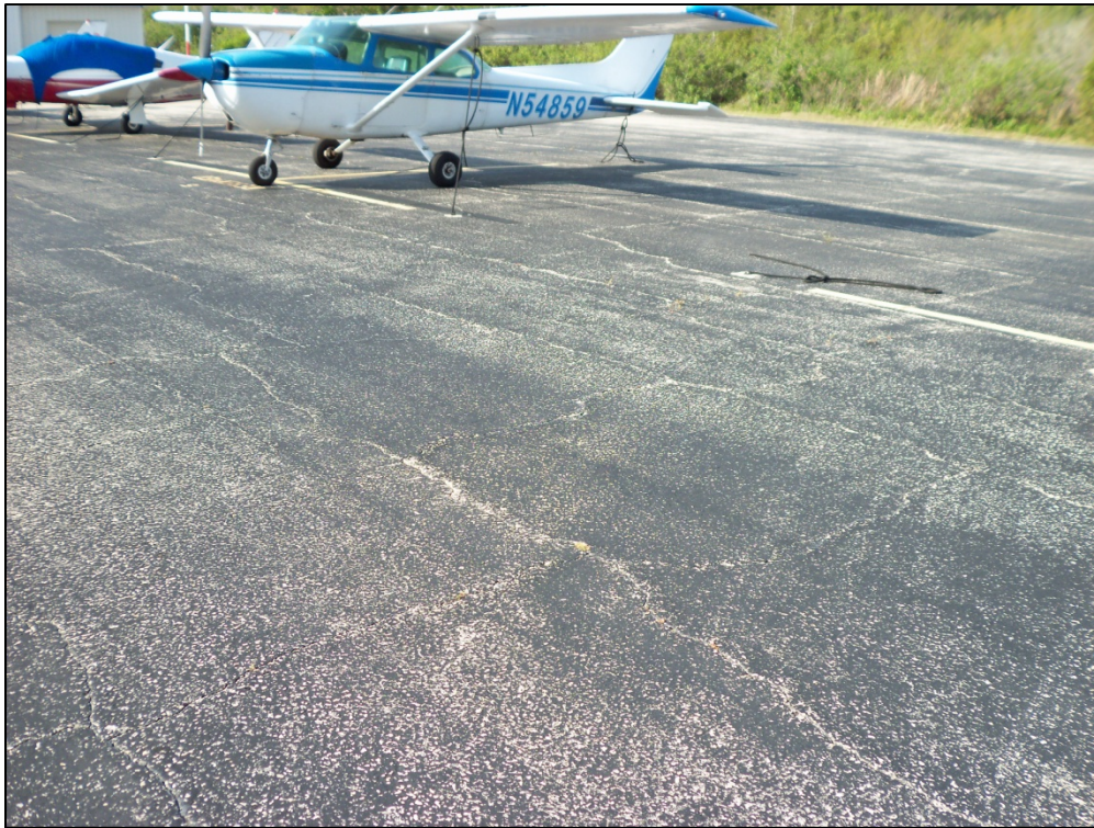
Apron, Section 4205, Sample Unit 455 – Low and medium severity (43) Block Cracking, low severity (52) Weathering and Raveling
