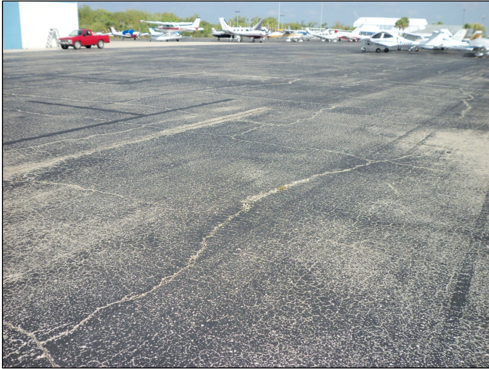
Apron, Section 4205, Sample Unit 257 – Low and medium severity (43) Block Cracking, low severity (52) Weathering and Raveling
