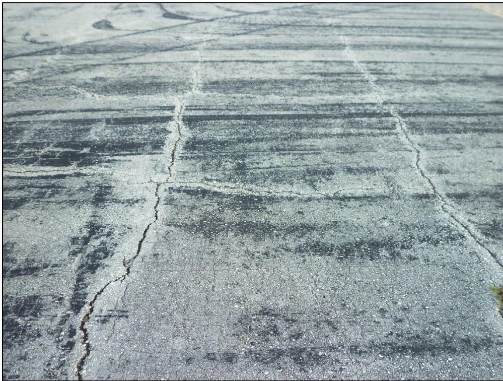
AP TA RW 35, Section 5105, Sample Unit 300 – Low and medium severity (43) Block Cracking, low severity (52) Weathering and Raveling
