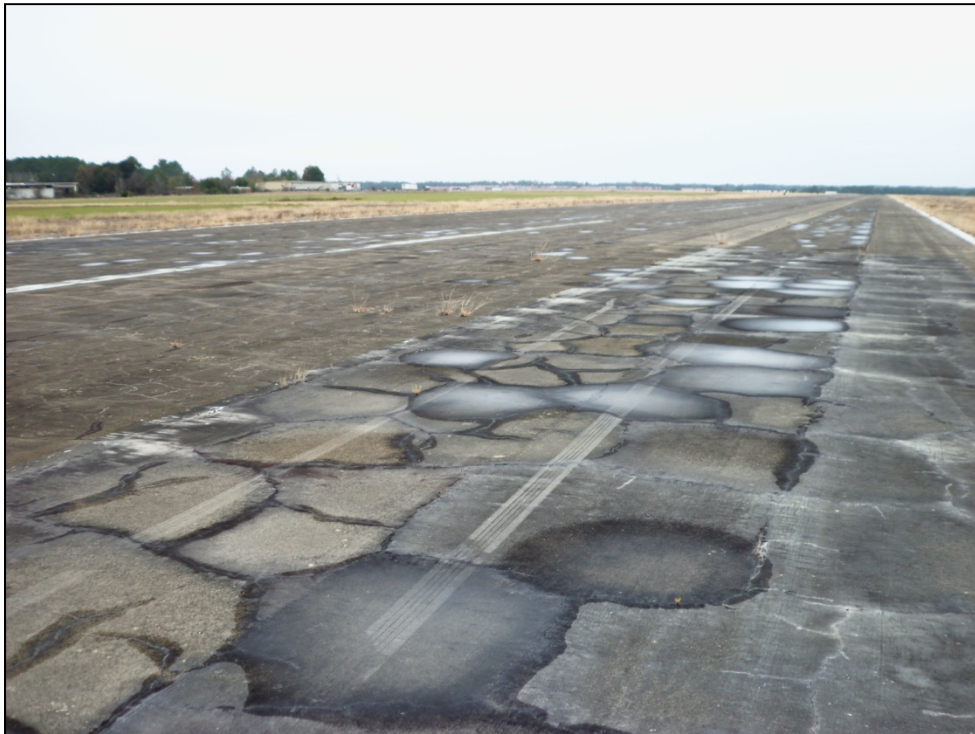
Runway 8-26, Section 6105, Sample Unit 300 – Medium severity (52) Weathering and Raveling; low severity (43) Block Cracking
