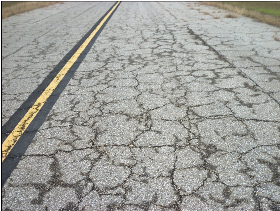
Taxiway Golf, Section 105, Sample Unit 107 – Medium severity (43) Block Cracking, medium severity (52) Weathering and Raveling.
