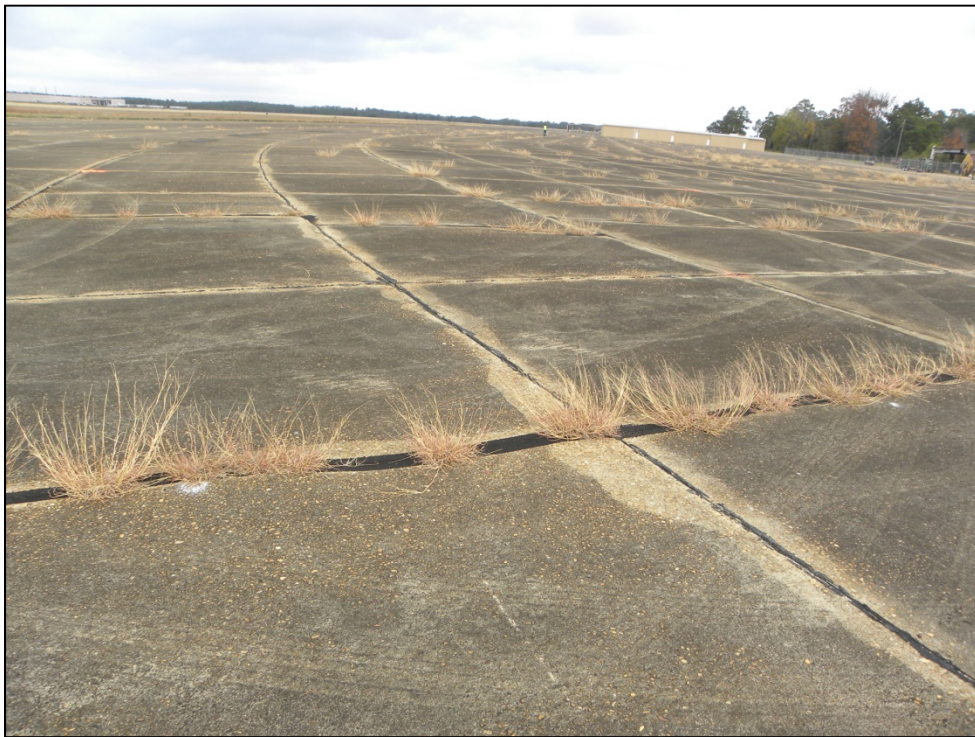
Apron, Section 4105, Sample Unit 242 – Low, medium, and high severity (63) Longitudinal/Transverse/Diagonal Cracking, medium severity (65) Joint Seal Damage, low severity (75) Corner Spalling, and low severity (74) Joint Spalling
