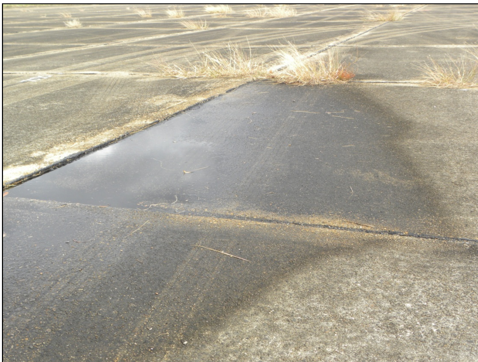
Apron, Section 4105, Sample Unit 204 – Medium, and high severity (63) Longitudinal/Transverse/Diagonal Cracking, medium severity (65) Joint Seal Damage, and low and medium (71) Faulting of Slabs
