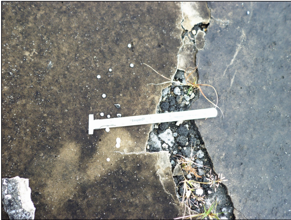
Runway 8-26, Section 6105, Sample Unit 300 – Medium severity (52) Weathering and Raveling; low severity (43) Block Cracking. Image depicts a close up of raveling “E-Crete” overlay material as well as raveled underlying asphalt material.
