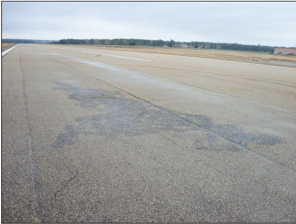
Runway 18-36, Section 6205, Sample Unit 165 – Low severity (52) Weathering and Raveling; low, medium, and high severity (48) Longitudinal and Transverse Cracking; N/A severity
