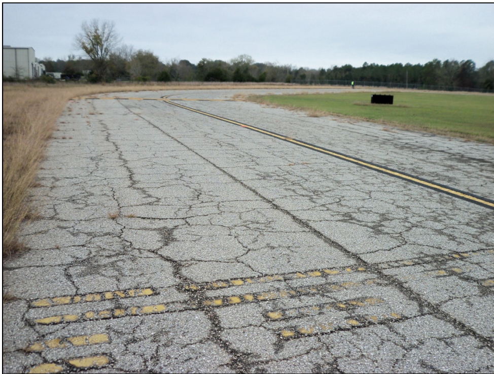
Taxiway Golf, Section 105, Sample Unit 101 – Medium severity (43) Block Cracking, medium severity (52) Weathering and Raveling.
