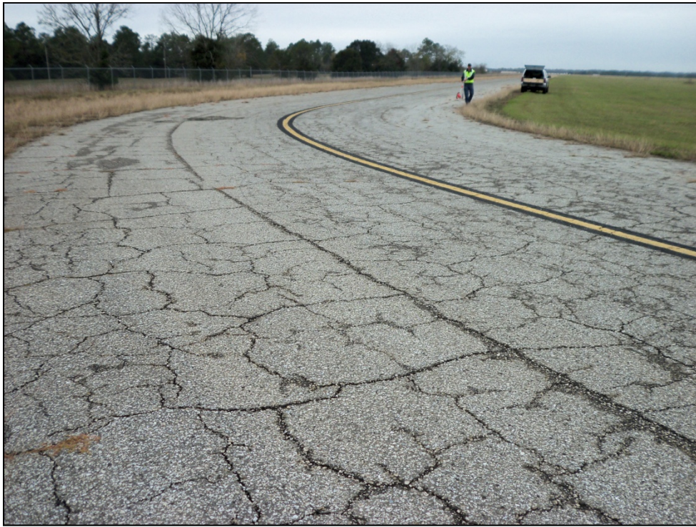
Taxiway Golf, Section 105, Sample Unit 105 – Medium severity (43) Block Cracking, medium severity (52) Weathering and Raveling.
