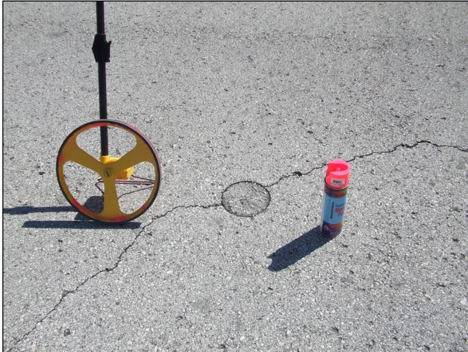
Apron, Section 4105, Sample Unit 101 - Low severity (48) Longitudinal and Transverse Cracking, low severity (49) Oil Spillage, low severity (50) Patch, low severity (52) Weathering and Raveling.
