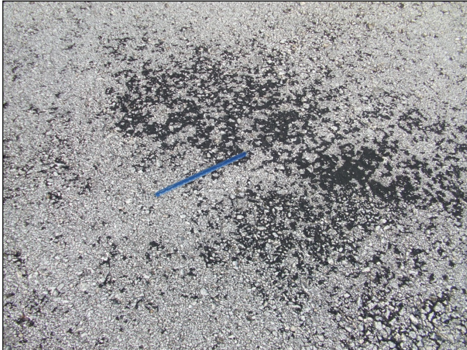
Runway 5-23, Section 6210, Sample Unit 162 - (42) Bleeding, low severity (48) Longitudinal and Transverse Cracking, low severity (52) Weathering and Raveling, low severity (56) Swelling.
