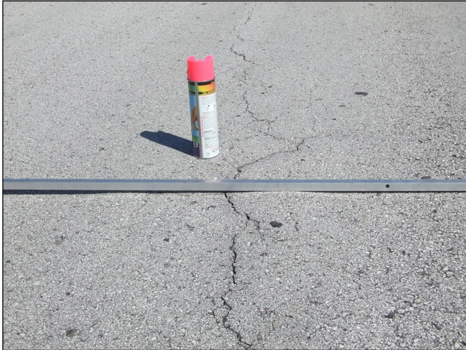
Taxiway Echo, Section 110, Sample Unit 105 – Low severity (43) Block Cracking, low and medium severity (52) Weathering and Raveling, low severity (56) Swelling.
