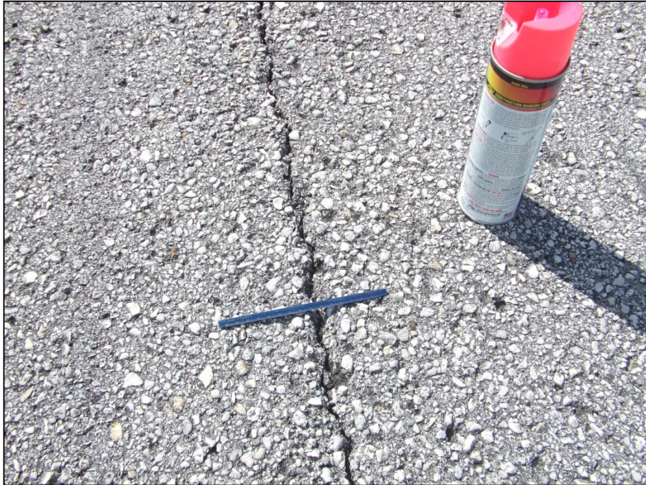
Runway 9-27, Section 6105, Sample Unit 108 – Low and medium severity (48) Longitudinal and Transverse Cracking, low and medium severity (52) Weathering and Raveling.
