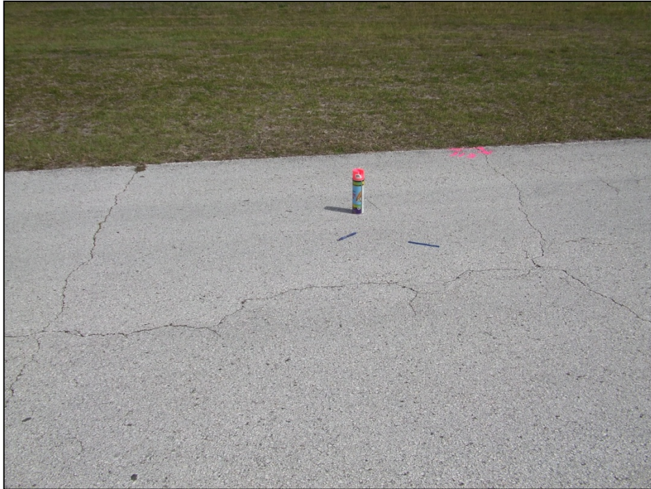
Taxiway Echo, Section 110, Sample Unit 113 - Low severity (43) Block Cracking, low and medium severity (48) Longitudinal and Transverse Cracking, low severity (52) Weathering and Raveling, low severity (56) Swelling.
