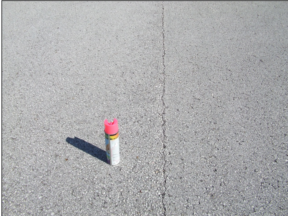
Taxiway Echo, Section 105, Sample Unit 100 - Low severity (48) Longitudinal and Transverse Cracking, low severity (50) Patch, low and medium severity (52) Weathering and Raveling.
