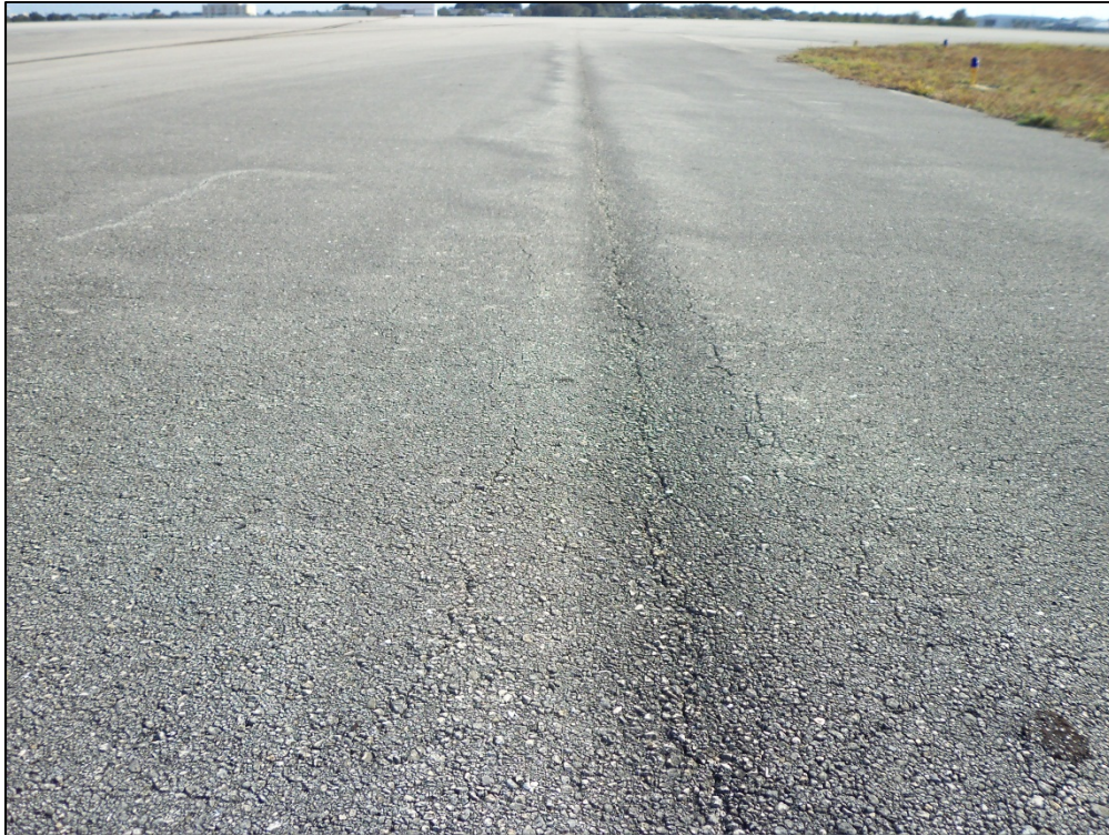
Taxiway Charlie, Section 333, Sample Unit 112 – Low severity (48) Longitudinal and Transverse Cracking, low severity (56) Swelling
