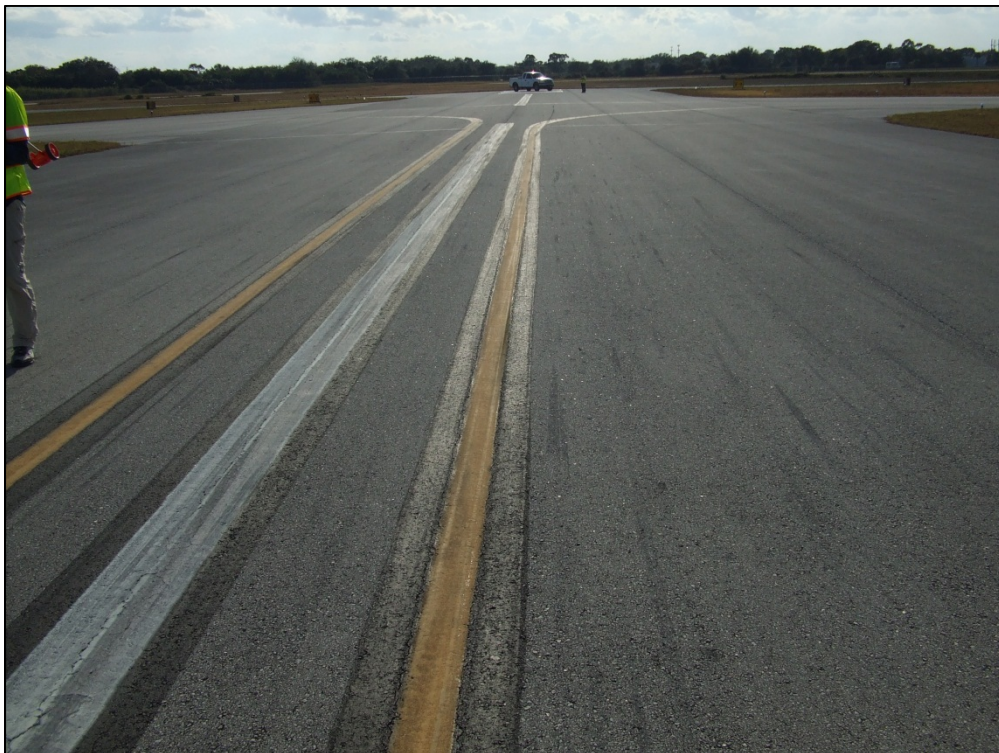
Runway 5-23, Section 6305, Section 108 – Low severity (48) Longitudinal and Transverse Cracking
