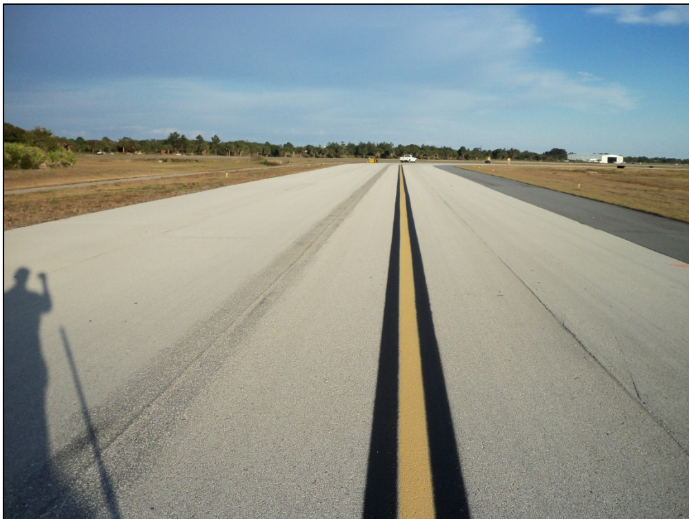
Taxiway Kilo, Section 1130, Sample Unit 171 – Low severity (48) Longitudinal and Transverse Cracking
