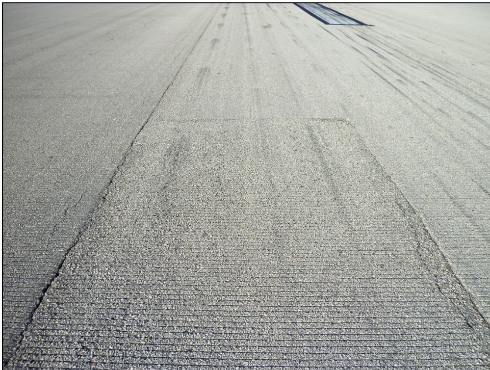
Runway 9R-27L, Section 6105, Sample Unit 375 – Low and medium severity (48) Longitudinal and Transverse Cracking, low severity (52) Weathering and Raveling
