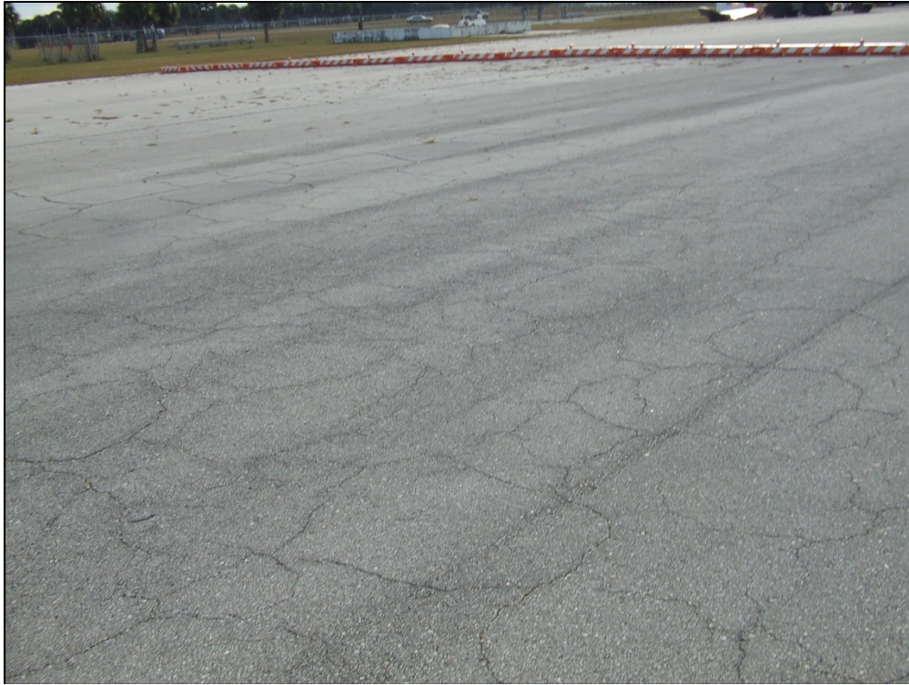
East Apron, Section 4406, Sample Unit 200 – Low severity (43) Block Cracking, low severity (52) Weathering and Raveling
