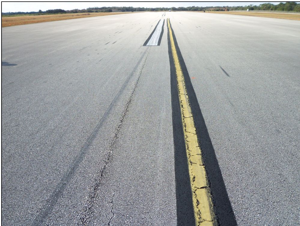
Runway 9R-27L, Section 6205, Sample Unit 342 – Low severity (48) Longitudinal and Transverse Cracking, low severity (52) Weathering and Raveling
