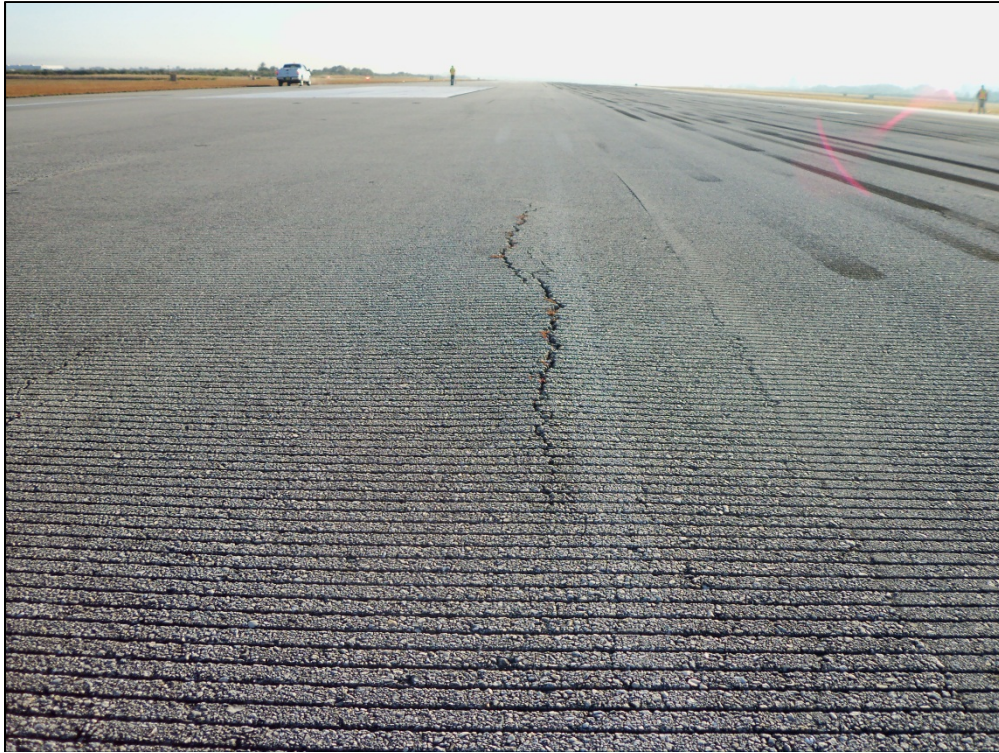
Runway 9R-27L, Section 6105, Sample Unit 318 – Low and medium severity (48) Longitudinal and Transverse Cracking, low severity (52) Weathering and Raveling
