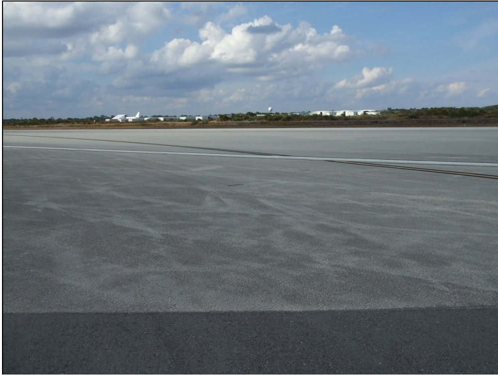
Taxiway Papa, Section 1602, Sample Unit 399 – Low severity (52) Weathering and Raveling
