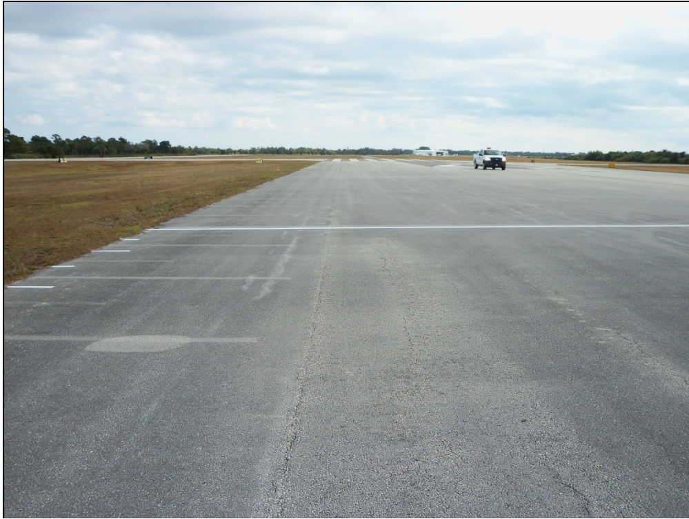
Runway 9R-27L, Section 6205, Sample Unit 208 – Low severity (48) Longitudinal and Transverse Cracking, low severity (52) Weathering and Raveling
