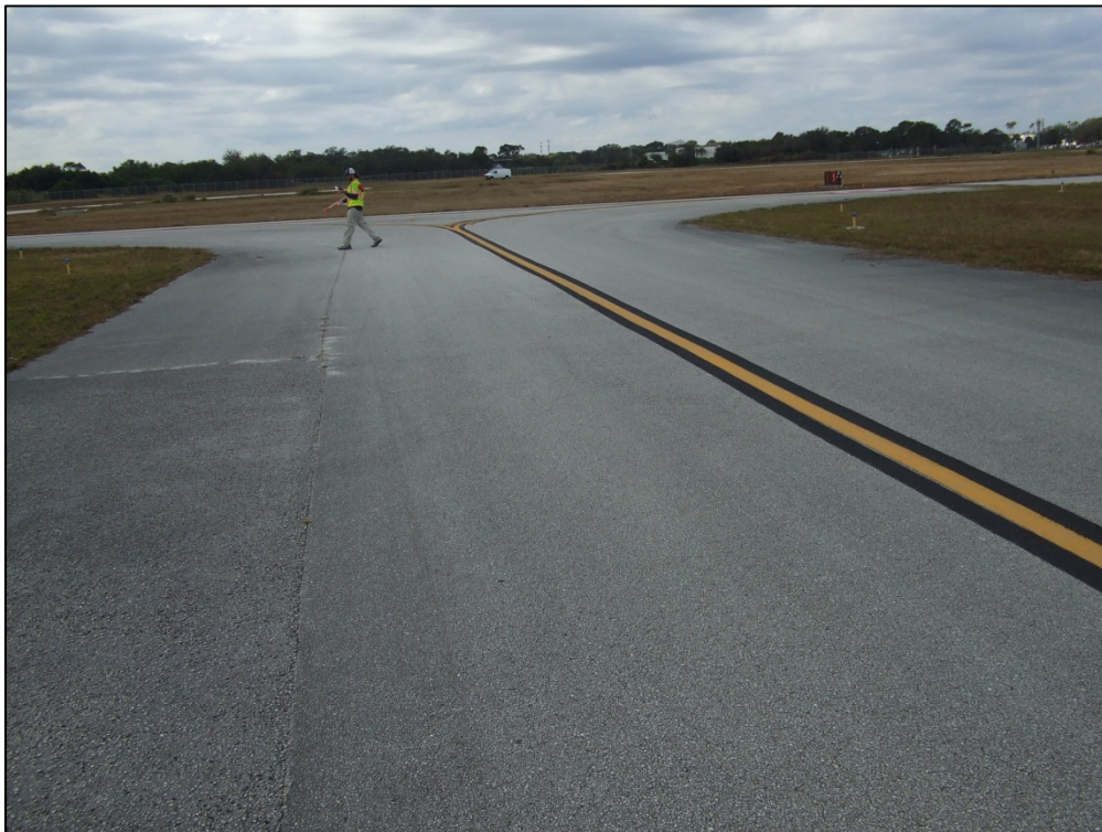
Taxiway Delta, Section 410, Sample Unit 102 – Low severity (48) Longitudinal and Transverse Cracking, medium severity (50) Patching, low severity (52) Weathering and Raveling
