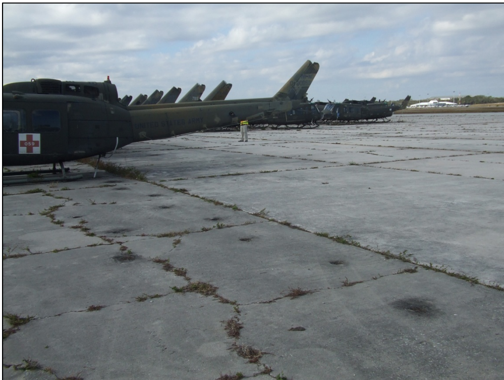
West Apron, Section 4330, Sample Unit 404 – High severity (72) Shattered Slab
