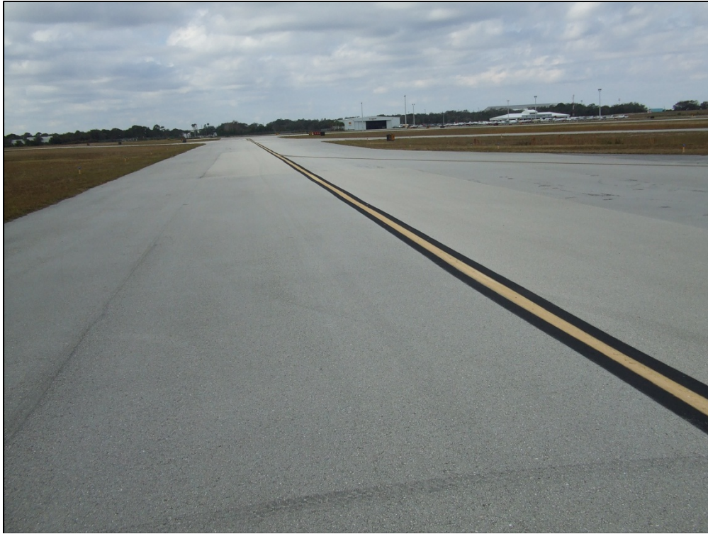
Taxiway Charlie, Section 305, Sample Unit 307 – Low severity (48) Longitudinal and Transverse Cracking, low severity (52) Weathering and Raveling
