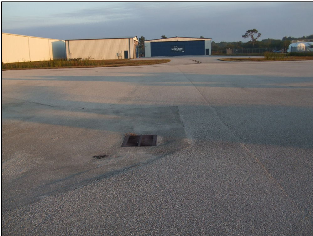
GA Apron, Section 4105, Sample Unit 107 – Medium severity (50) Patching, low severity (48) Longitudinal and Transverse Cracking, low severity (52) Weathering and Raveling
