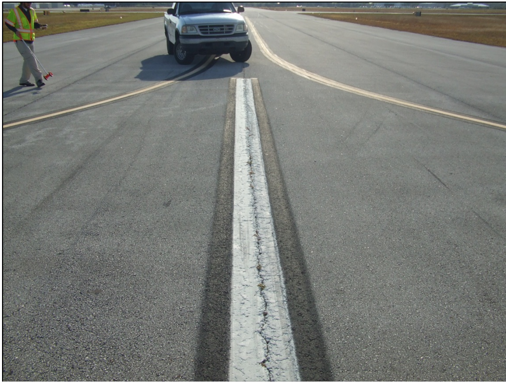
Runway 5-23, Section 6315, Sample Unit 147 – Low severity (48) Longitudinal and Transverse Cracking, low severity (52) Weathering and Raveling
