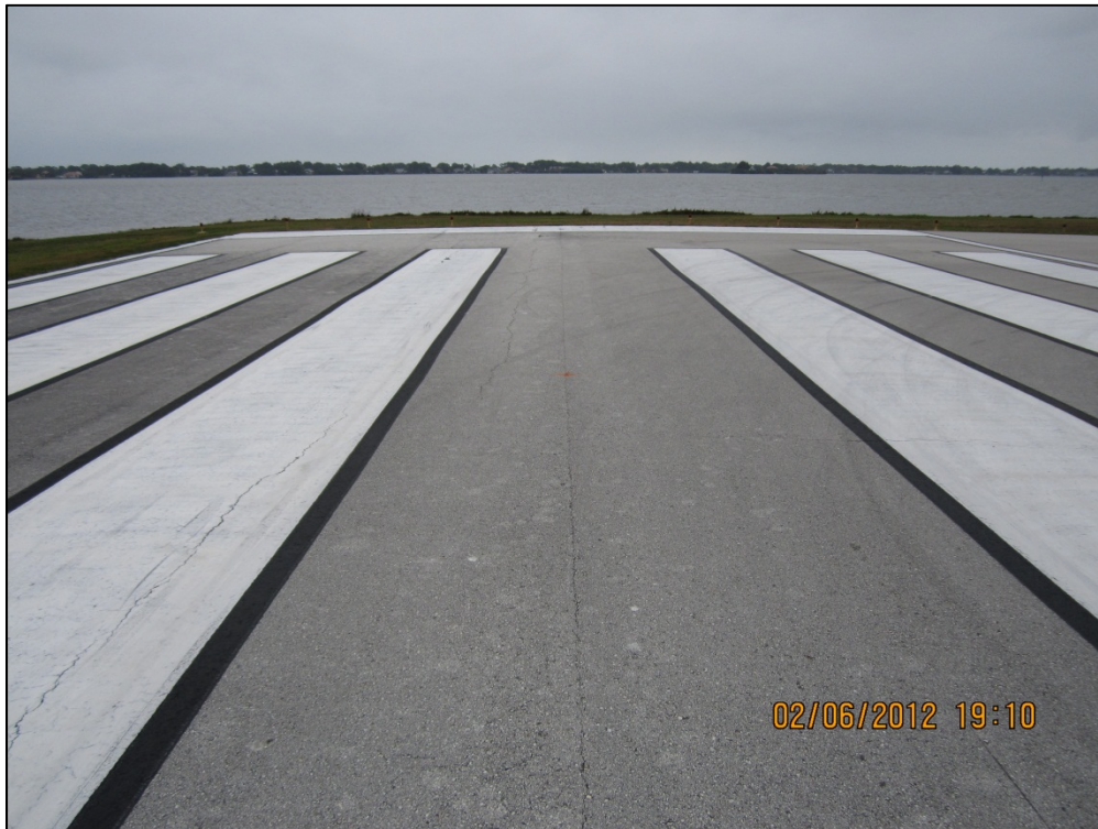
Runway 11-29, Section 6105, Sample Unit 170 – Low severity (48) Longitudinal and Transverse Cracking, low severity (52) Weathering and Raveling
