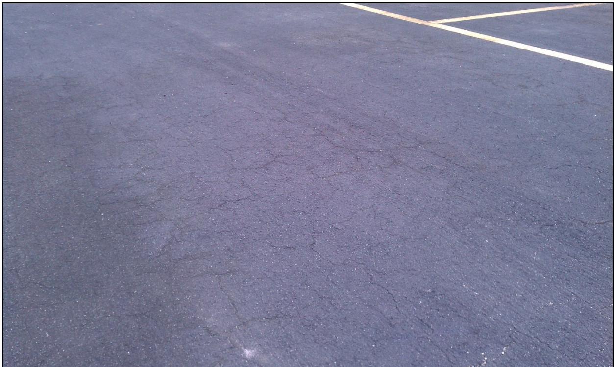
South Apron, Section 4106, Sample Unit 199 – Medium severity (52) Weathering and Raveling
