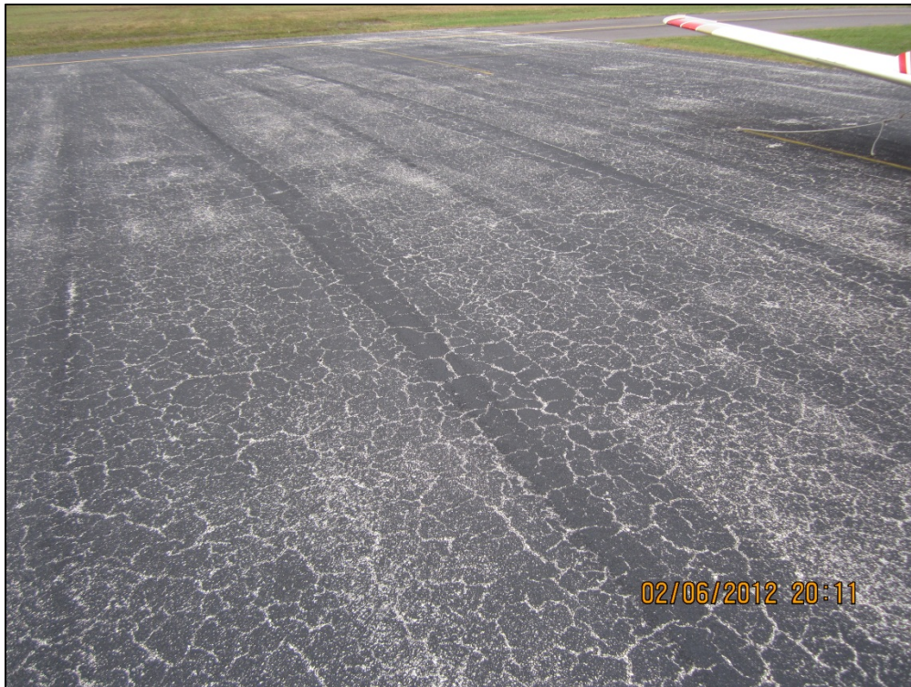
North Apron, Section 4205, Sample Unit 197 – Low severity (43) Block Cracking, medium severity (52) Weathering and Raveling
