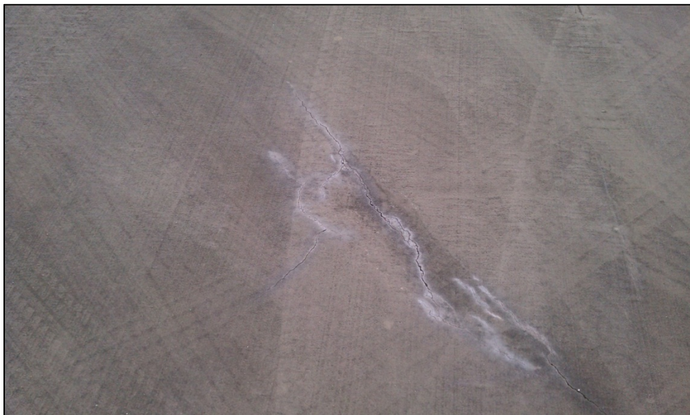
Southwest Apron, Section 4305, Sample Unit 200 – Low severity (48) Longitudinal and Transverse Cracking
