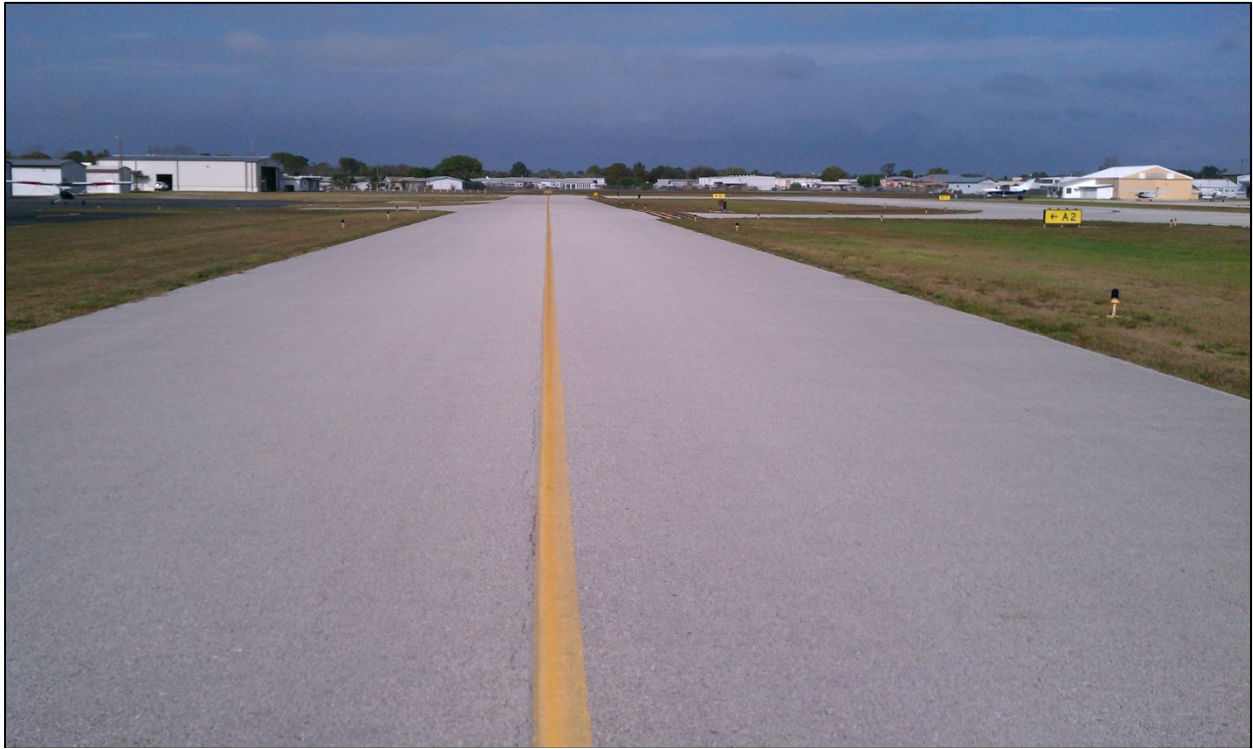
Taxiway Alpha, Section 105, Sample Unit 107 – Low severity (48) Longitudinal and Transverse Cracking
