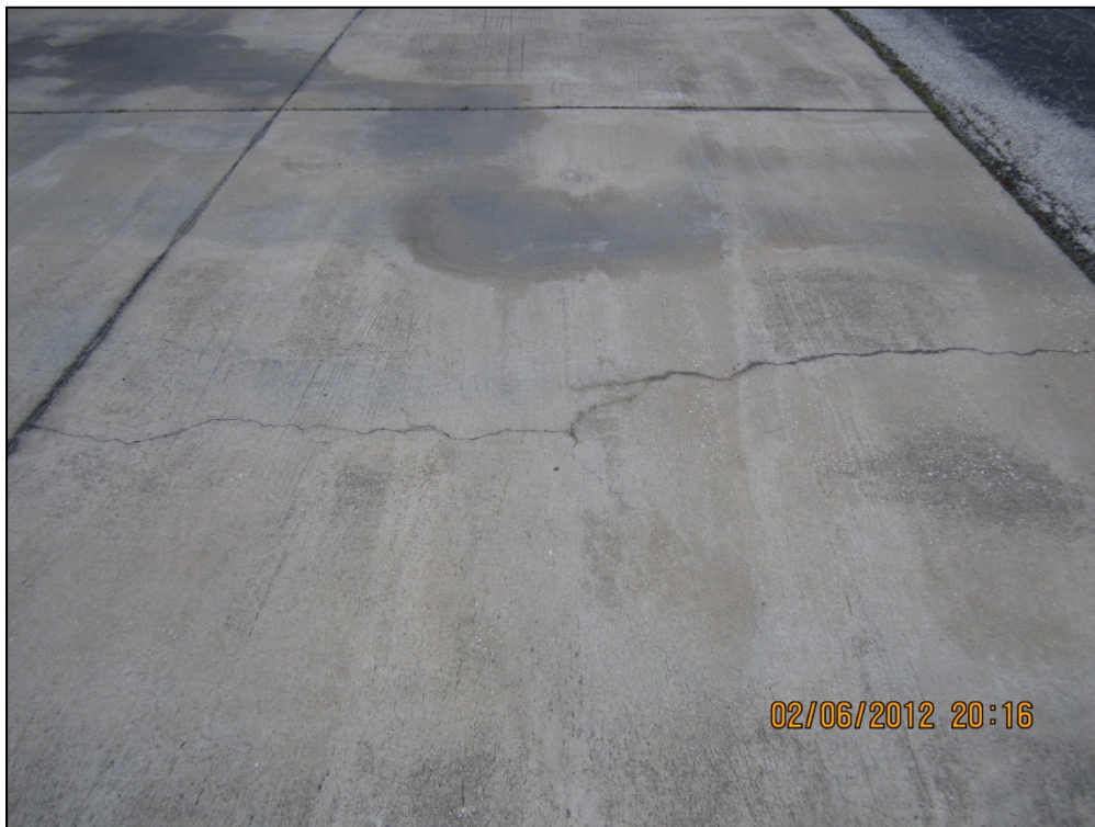
North Apron, Section 4203, Sample Unit 100 – Low severity (70) Scaling, Crazing and Map Cracking; low severity (63) Longitudinal, Transverse, and Diagonal Cracking; low severity (65) Joint Seal Damage
