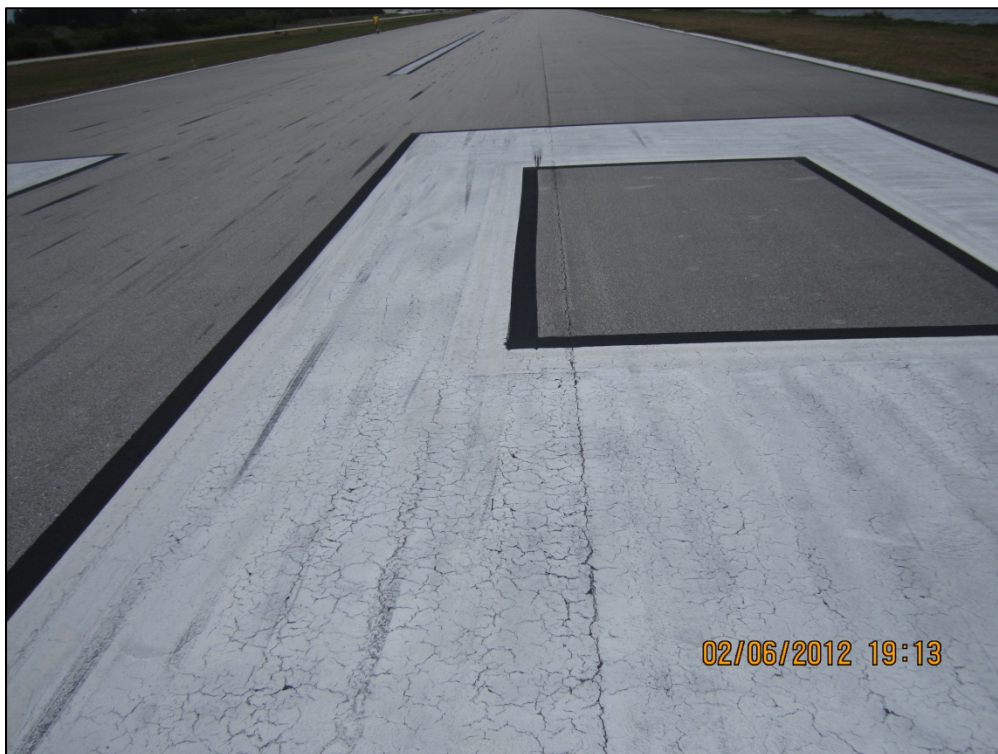
Runway 11-29, Section 6105, Sample Unit 167 – Low severity (48) Longitudinal and Transverse Cracking, low severity (52) Weathering and Raveling
