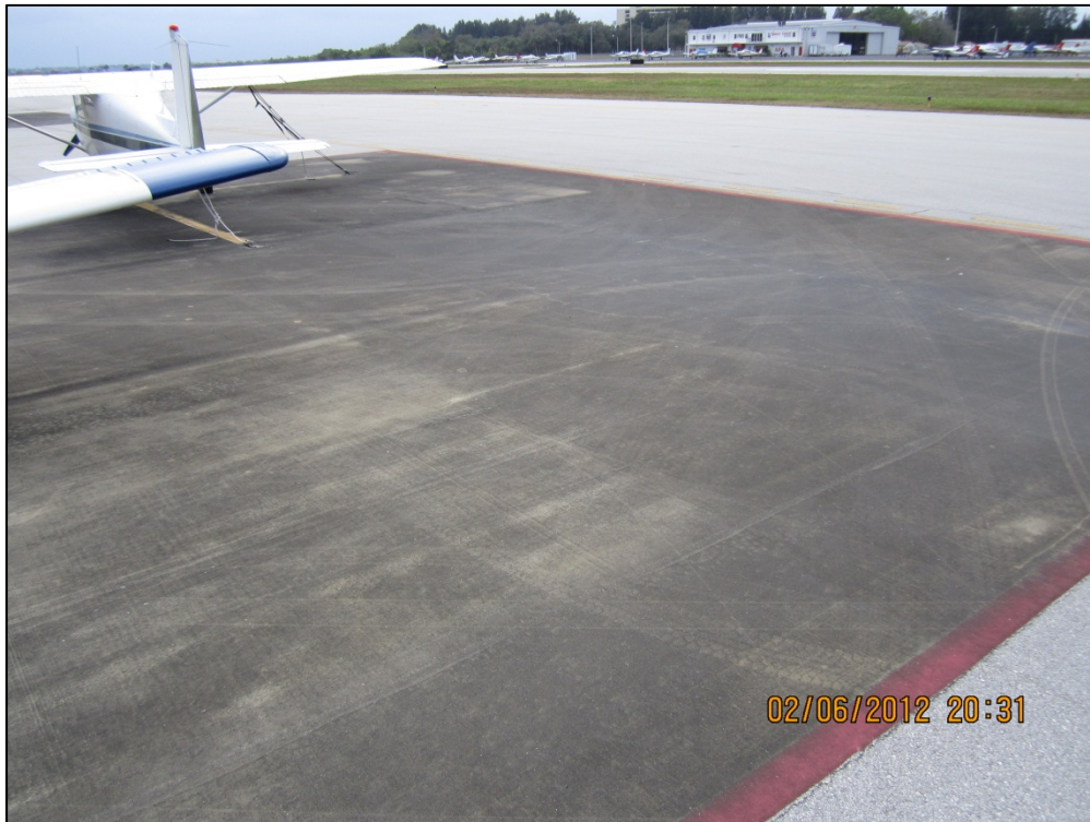
North Apron, Section 4218, Sample Unit 820 – Low severity (50) Patching
