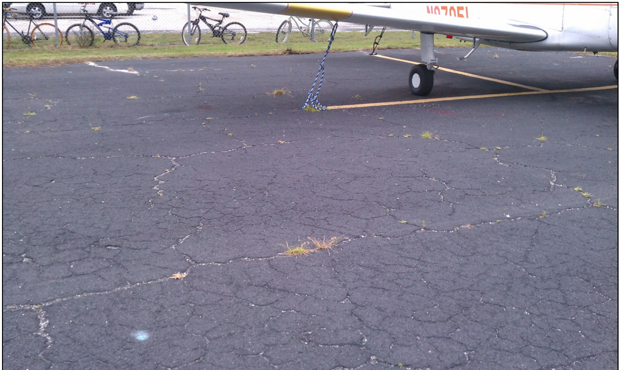
South Apron, Section 4115, Sample Unit 177 – Medium Severity (43) Block Cracking, medium severity (52) Weathering and Raveling
