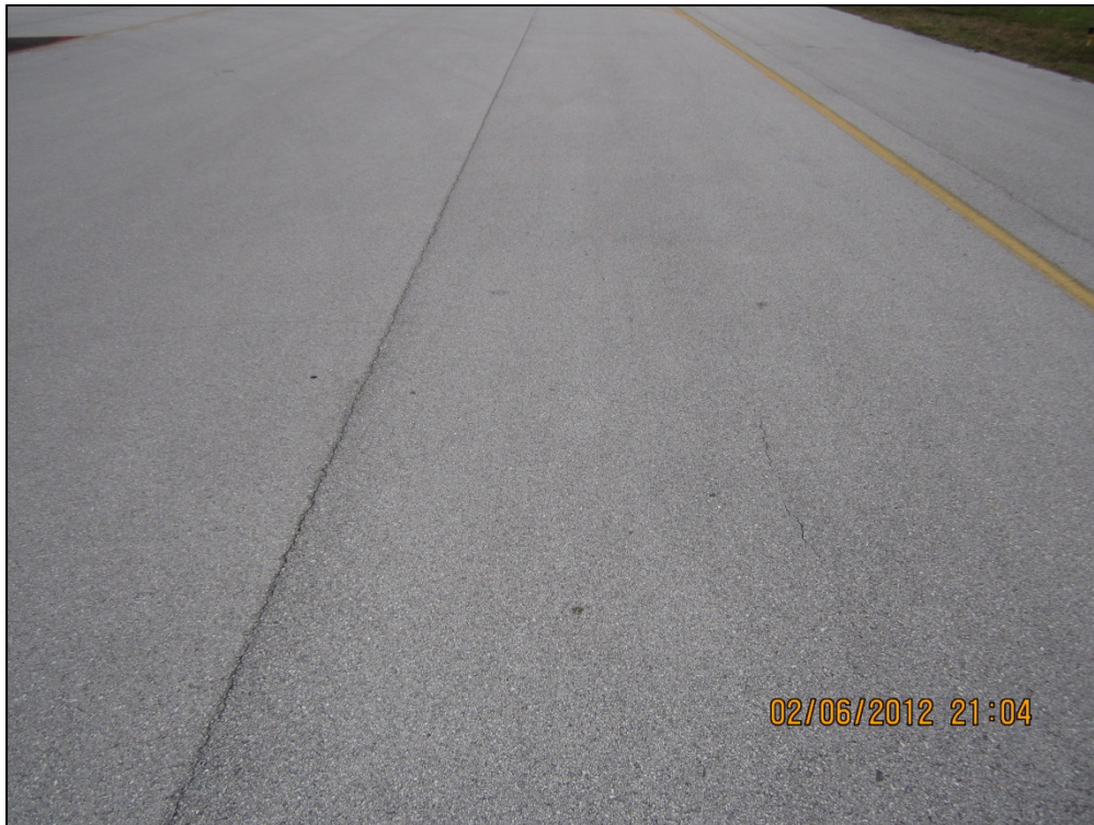
Taxiway Bravo, Section 205, Sample Unit 102 – Low severity (48) Longitudinal and Transverse Cracking
