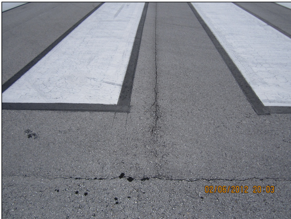
Runway 11-29, Section 6105, Sample Unit 100 – Low severity (48) Longitudinal and Transverse Cracking, low severity (52) Weathering and Raveling
