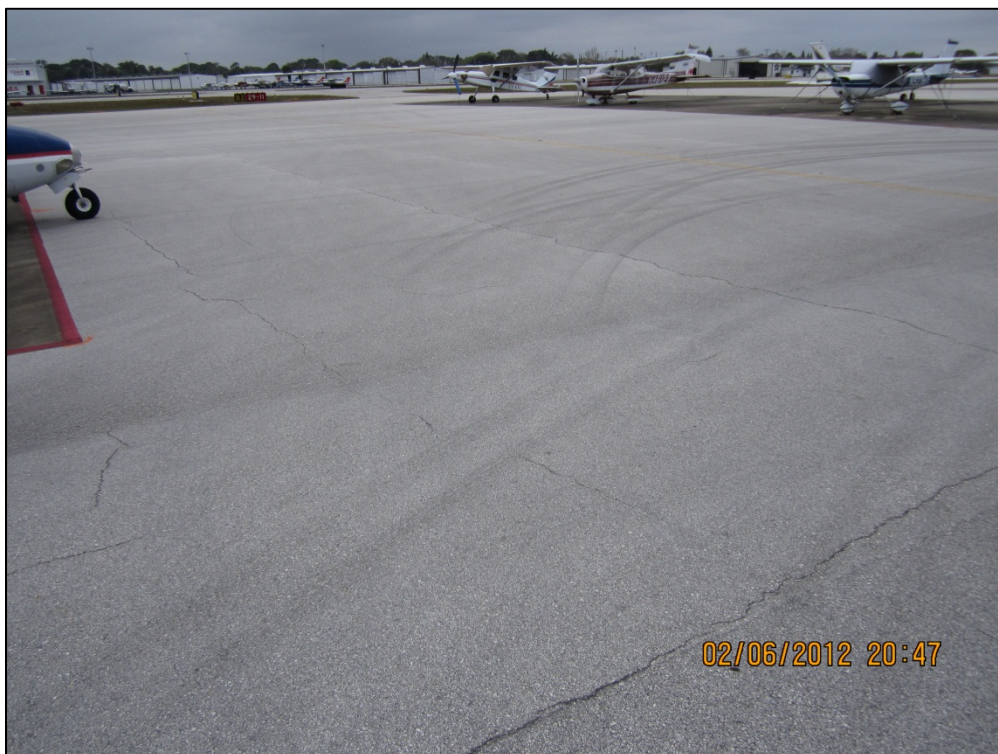
North Apron, Section 4215, Sample Unit 355 – Low severity (48) Longitudinal and Transverse Cracking, low severity (52) Weathering and Raveling
