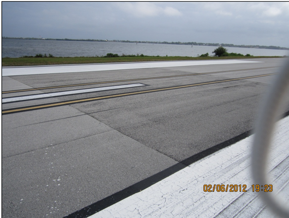
Runway 11-29, Section 6105, Sample Unit 149 – Low severity (48) Longitudinal and Transverse Cracking, medium severity (50) Patching
