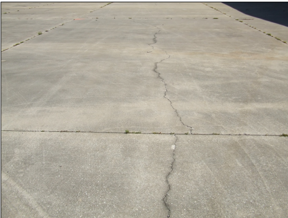
South Apron, Section 4215, Sample Unit 401 – Medium severity (63) Linear Cracking, high severity (65) Joint Seal Damage, and low severity Map Cracking / Scaling / Crazeing.
