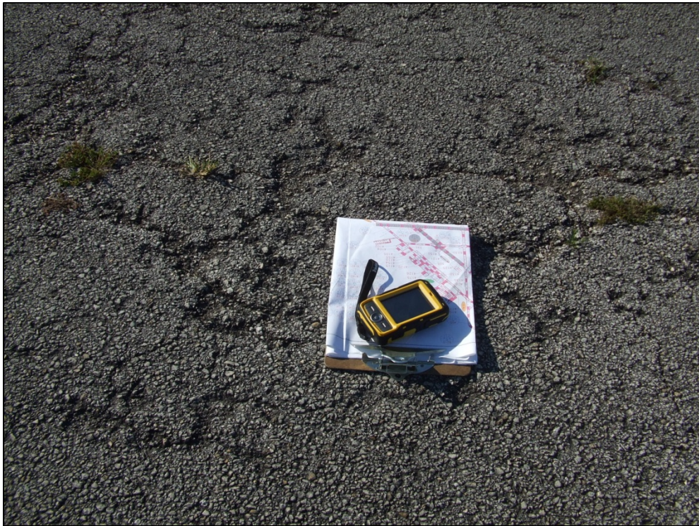
Apron, Section 4170, Sample Unit 217 – Medium severity (48) Longitudinal and Transverse Cracking and medium severity (52) Weathering and Raveling.
