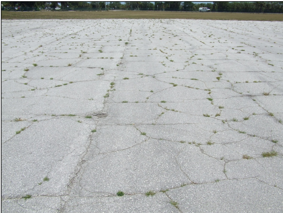
Runway 2-20, Section 6445, Sample Unit 196 – Medium severity (43) Block Cracking and low severity (52) Weathering and Raveling.
