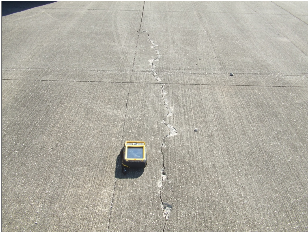
Apron, Section 4150, Sample Unit 106 (Whitetopping) – High severity (3) Linear Cracking.
