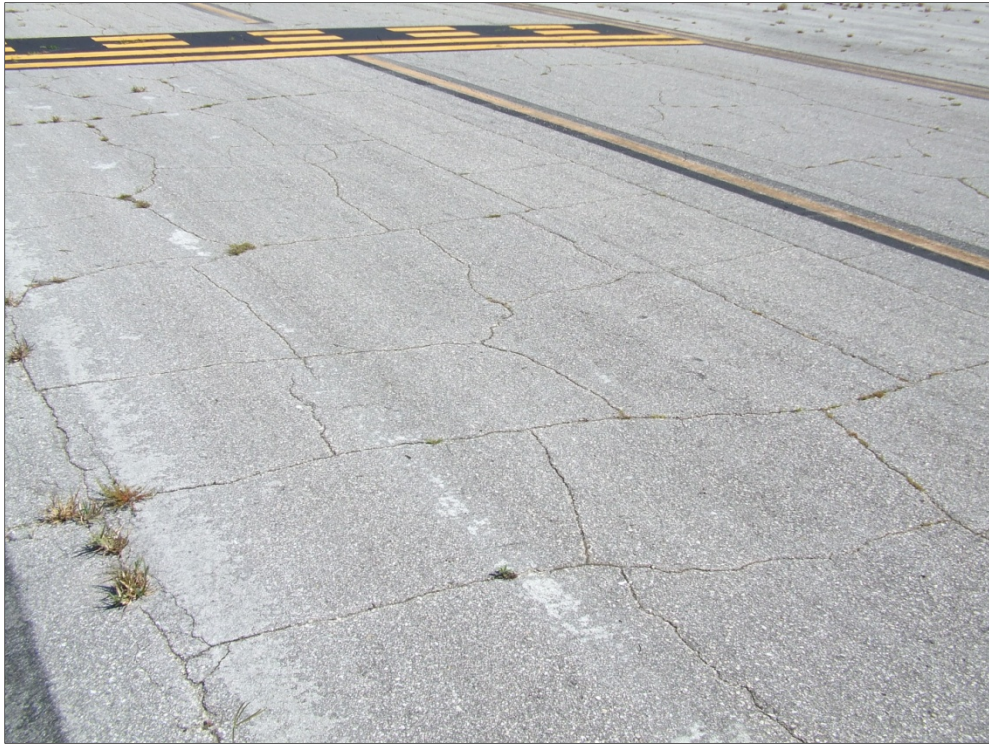
Taxiway Echo, Section 505, Sample Unit 102 – Medium severity (43) Block Cracking and low severity (52) Weathering and Raveling.
