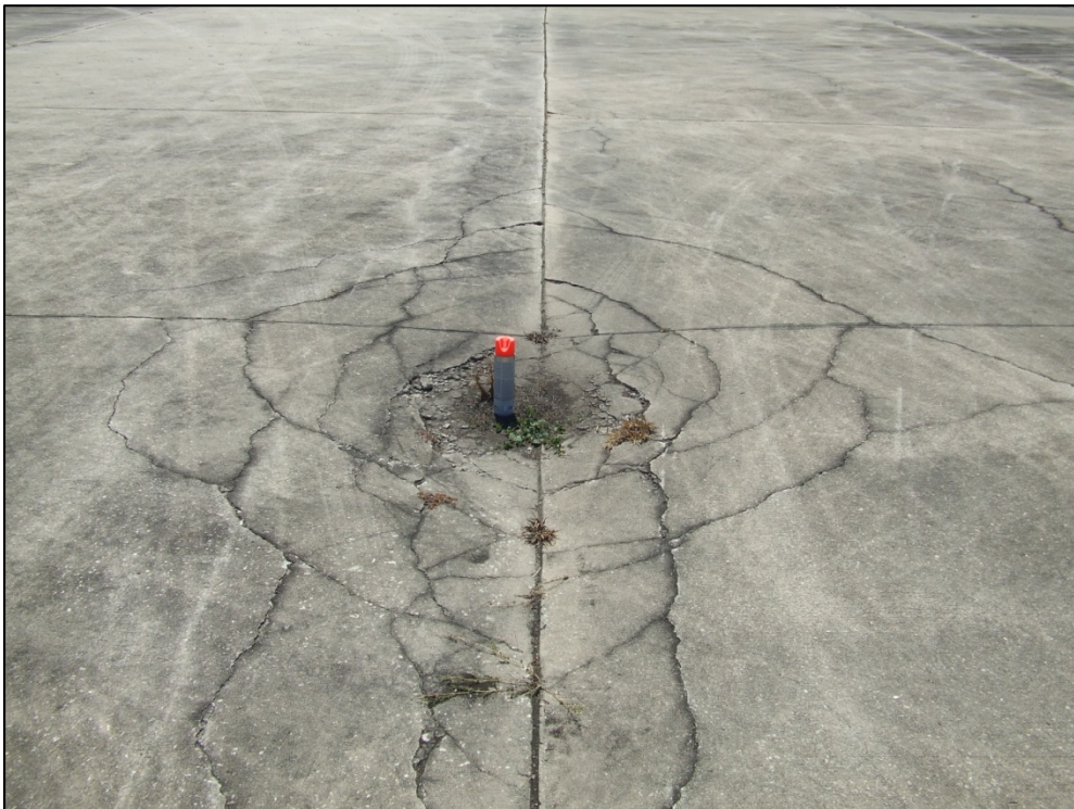
Apron, Section 4102, Sample Unit 101 – High severity (62) Corner Break, low severity (70) Map Cracking / Scaling / Cracking, high severity (74) Joint Spalling.
