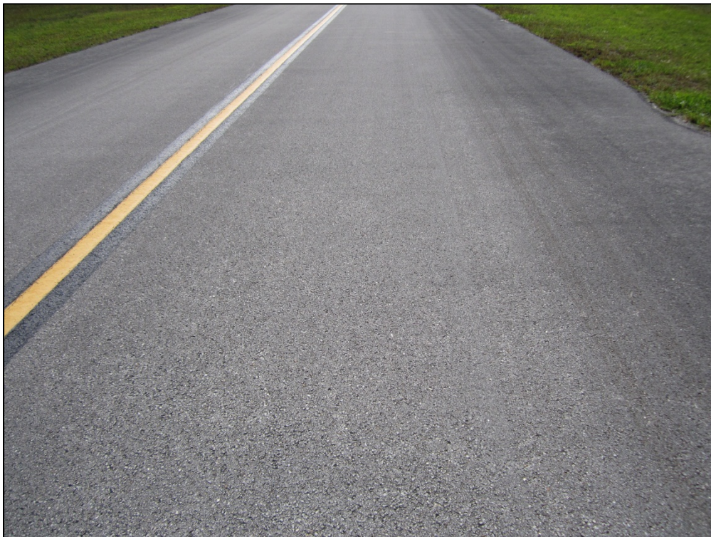
Taxiway Kilo, Section 1105, Sample Unit 110 – Low severity (52) Weathering and Raveling
