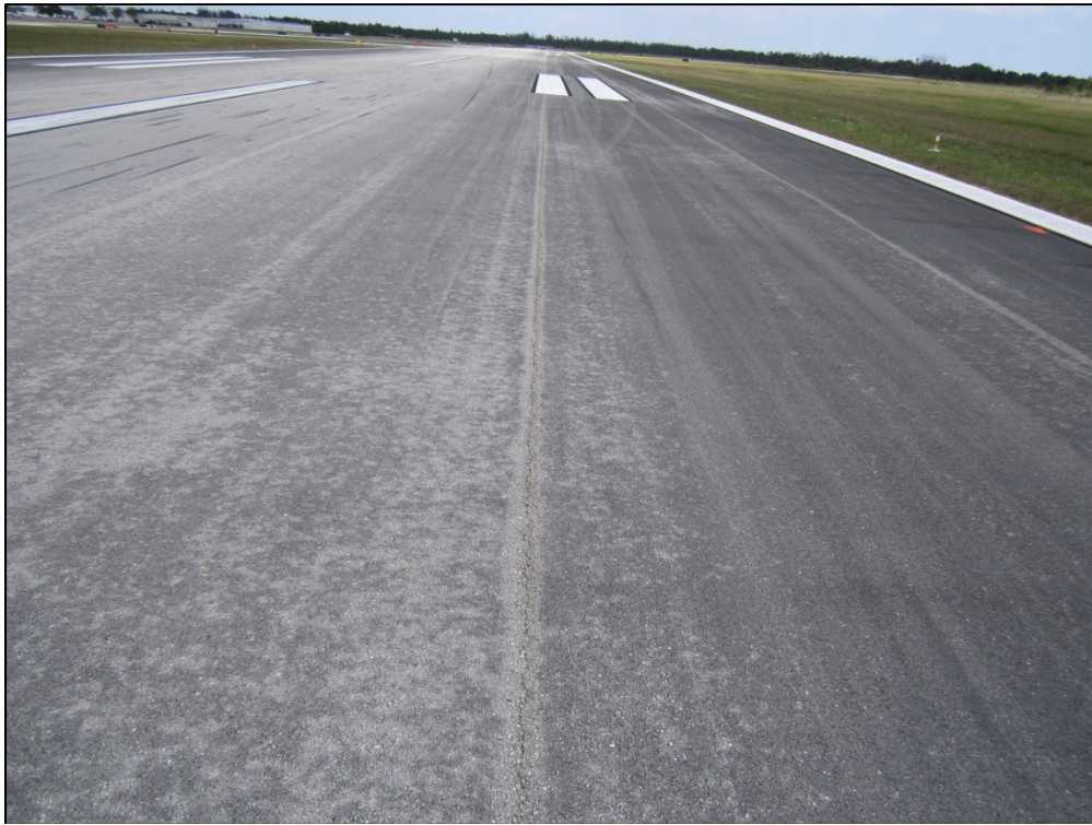
Runway 8R-26L, Section 6105, Sample Unit 128 – Low severity (48) Longitudinal and Transverse Cracking, low severity (52) Weathering and Raveling
