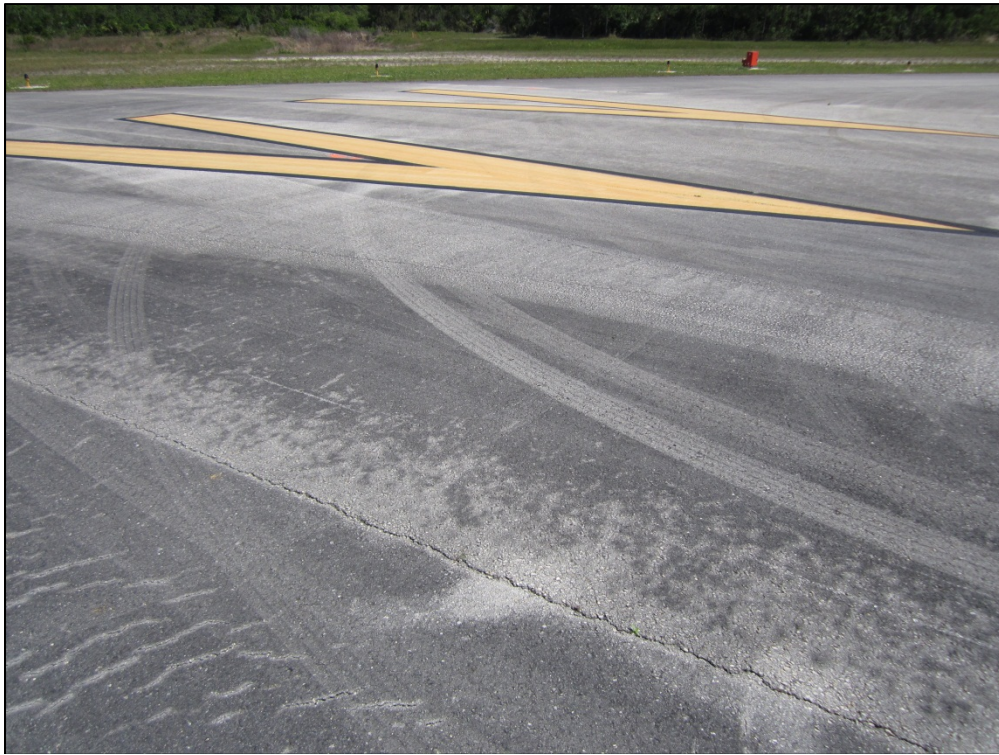
Runway 13-31, Section 6205, Sample Unit 186 – Low severity (48) Longitudinal and Transverse Cracking, low severity (52) Weathering and Raveling
