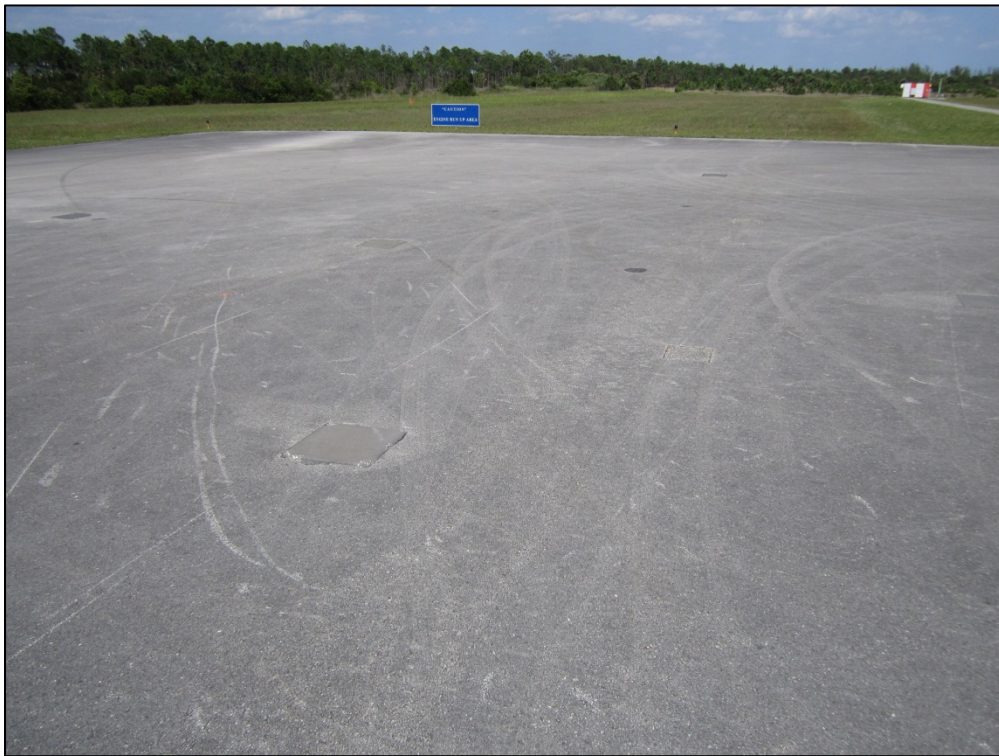
Apron Run-Up, Section 5110, Sample Unit 101– Low severity (48) Longitudinal and Transverse Cracking, low severity (52) Weathering and Raveling, low severity (50) Patching
