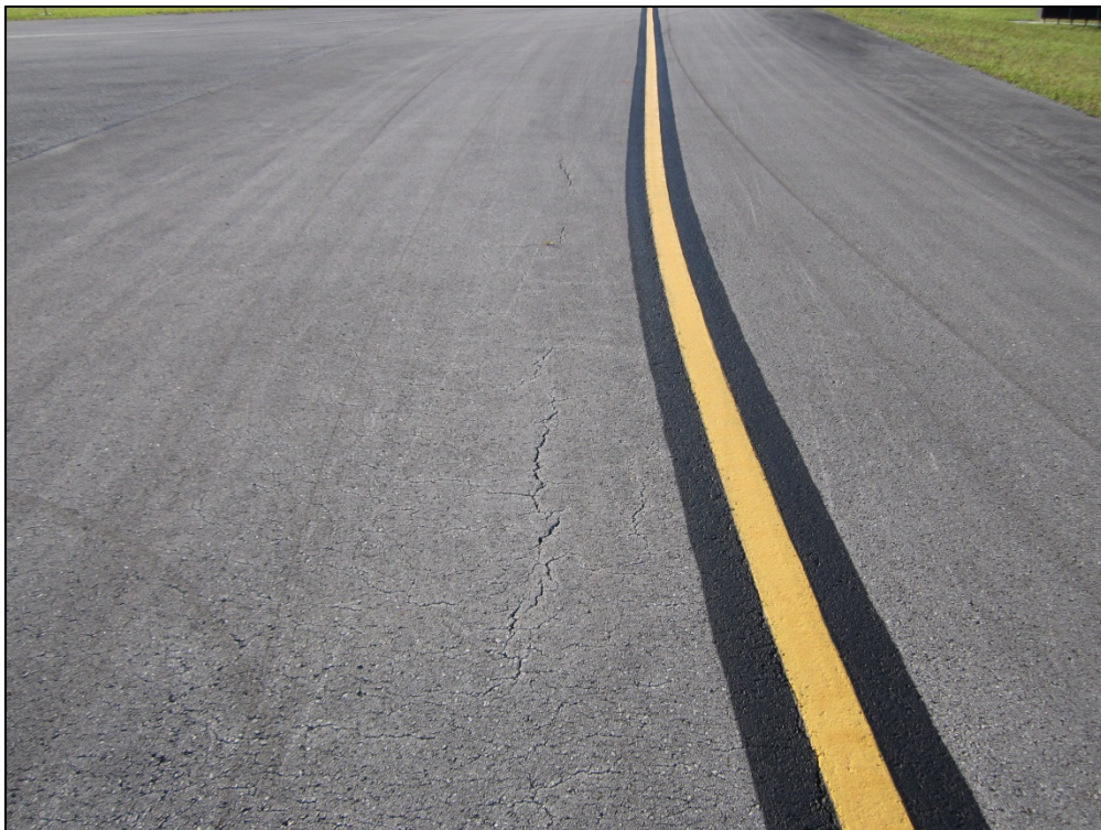
Taxiway Foxtrot, Section 605, Sample Unit 142 – Low severity (48) Longitudinal and Transverse Cracking, low severity (52) Weathering and Raveling
