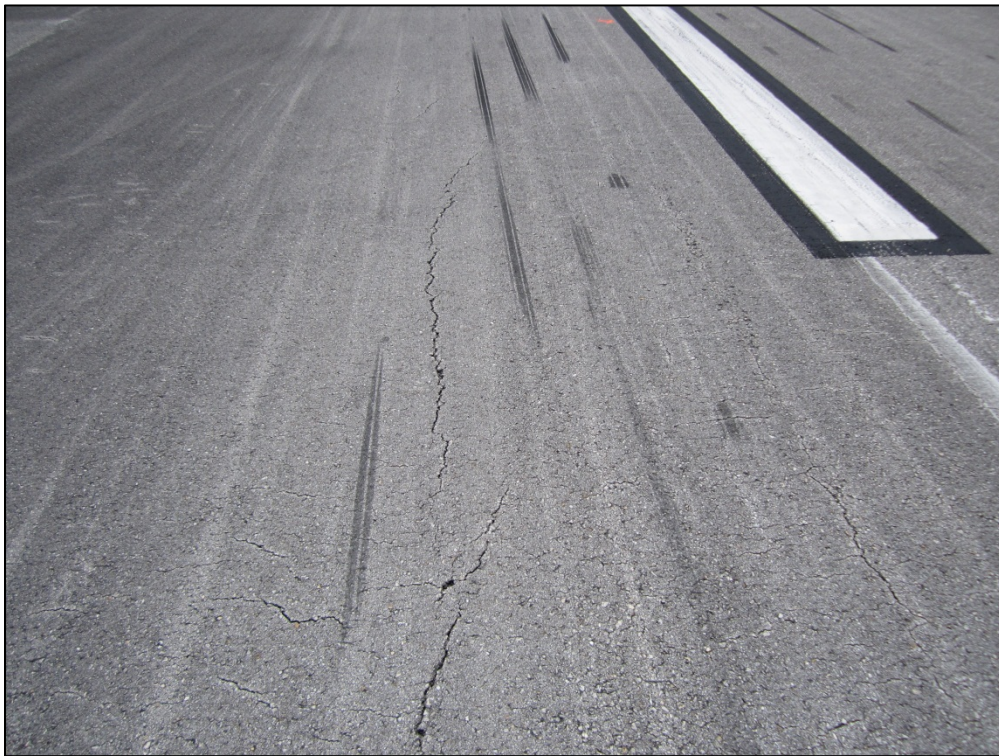
Runway 13-31, Section 6205, Sample Unit 120 – Low severity (48) Longitudinal and Transverse Cracking, low severity (52) Weathering and Raveling
