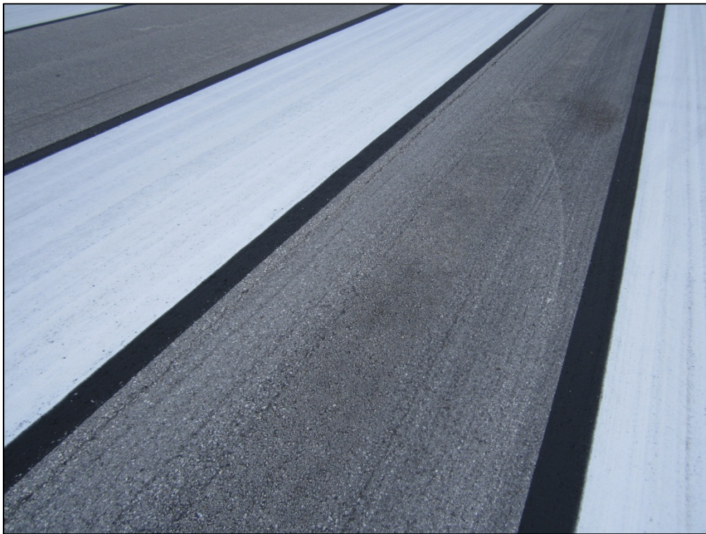
Runway 8R-26L, Section 6105, Sample Unit 101 – Low severity (48) Longitudinal and Transverse Cracking, low and medium severity (52) Weathering and Raveling
