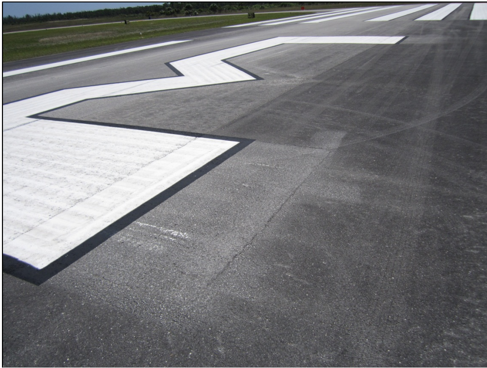
Runway 13-31, Section 6205, Sample Unit 105– Low severity (48) Longitudinal and Transverse Cracking, low severity (52) Weathering and Raveling
