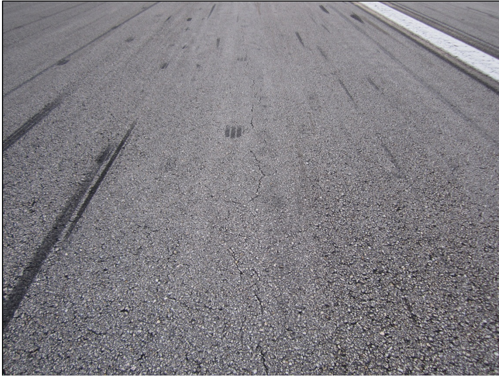
Runway 10R-28L, Section 6405, Sample Unit 112 – Low severity (48) Longitudinal and Transverse Cracking, low severity (52) Weathering and Raveling
