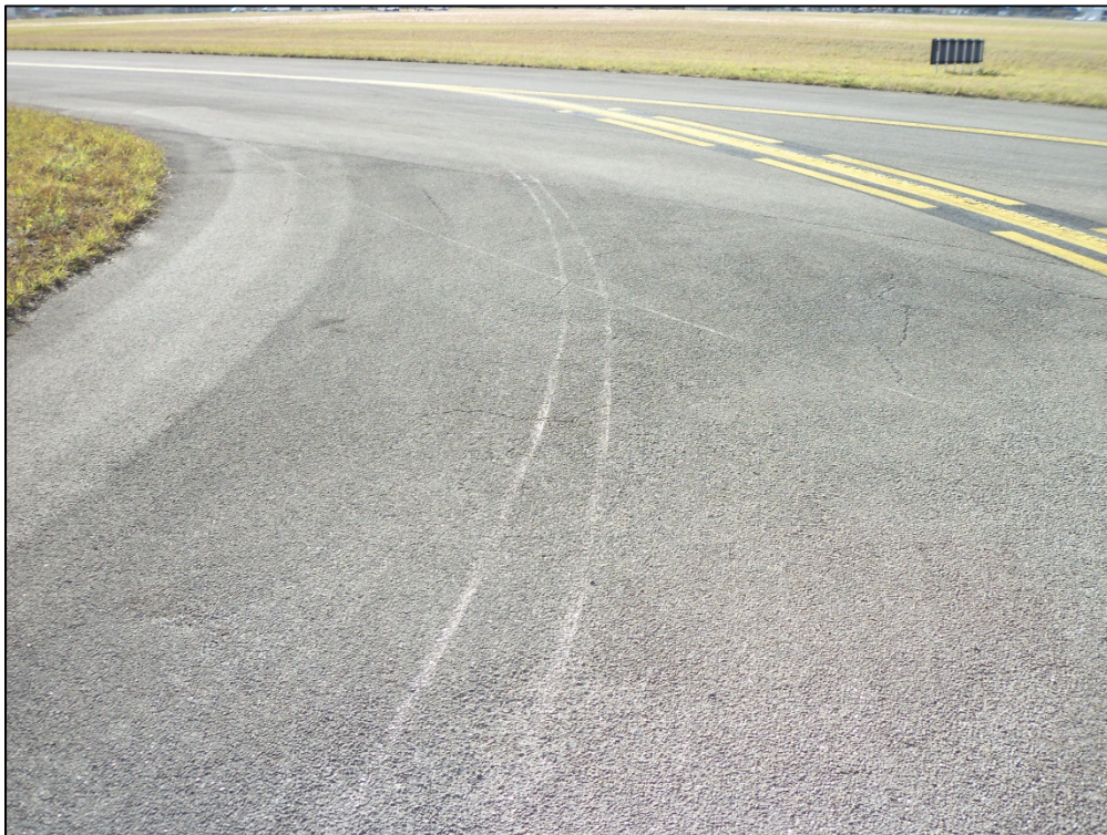
Taxiway N-2, Section 710, Sample Unit 101 – Low and medium severity (52) Weathering and Raveling, low severity (48) Longitudinal and Transverse Cracking
