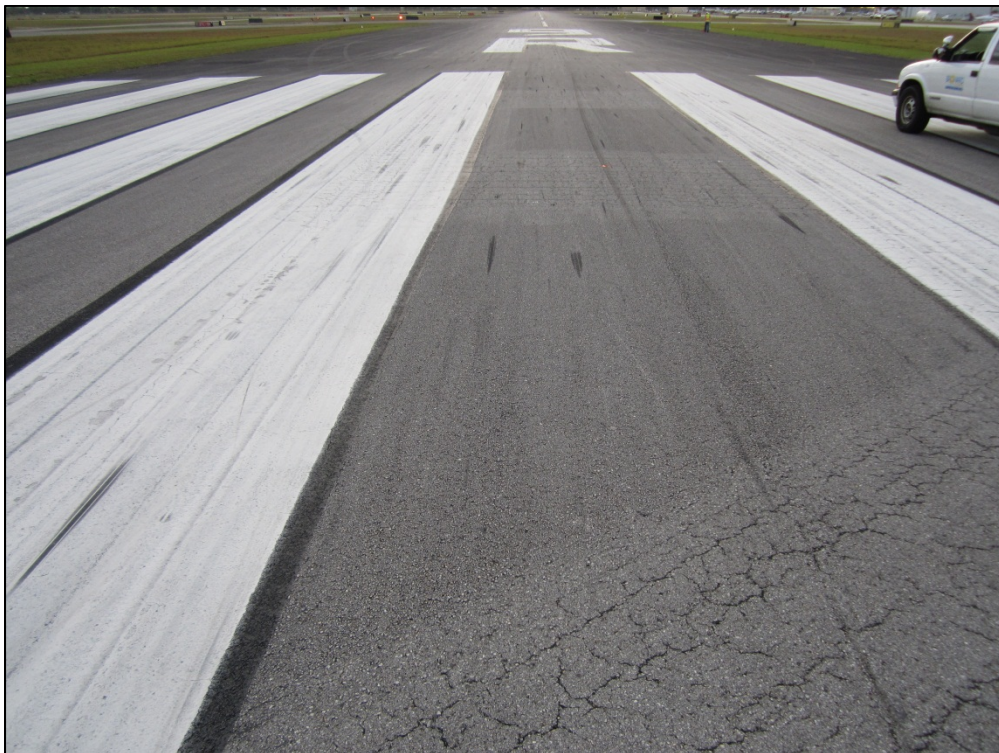
Runway 10R-28L, Section 6405, Sample Unit 102 – Low severity (48) Longitudinal and Transverse Cracking, low severity (52) Weathering and Raveling
