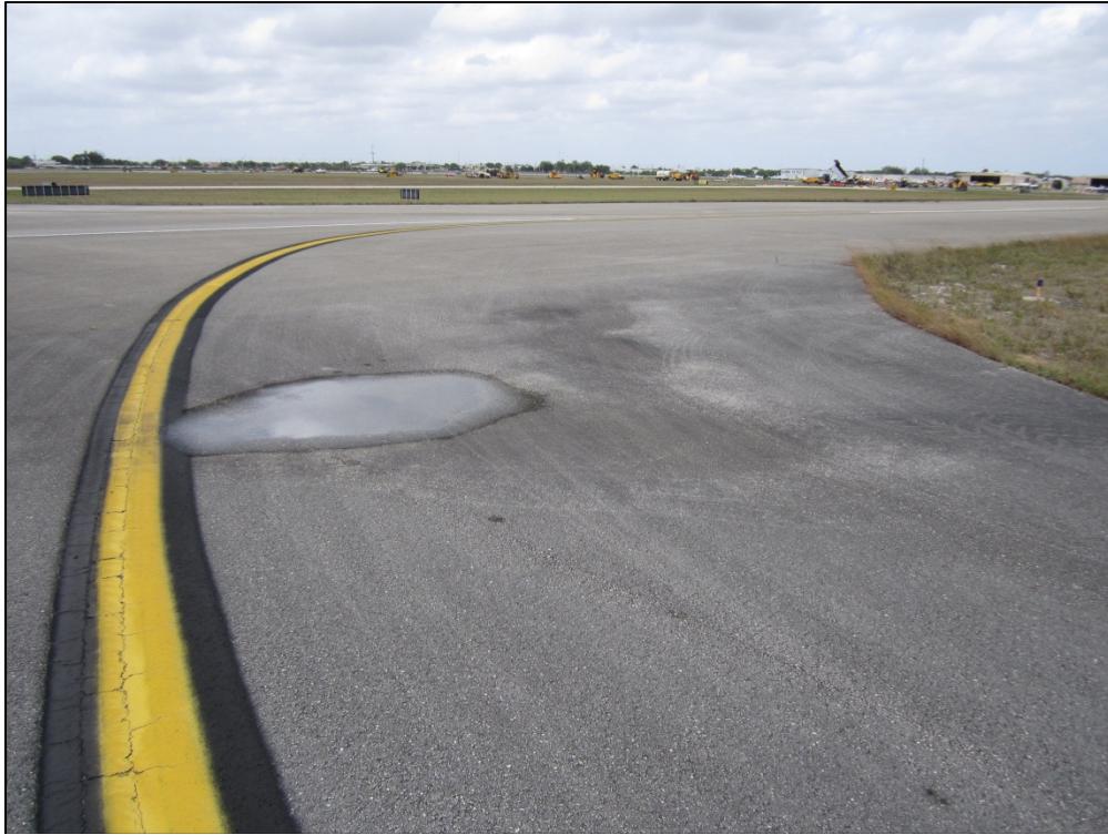
Taxiway D-1, Section 1315, Sample Unit 101 – Low severity (48) Longitudinal and Transverse Cracking, low severity (45) Depression
