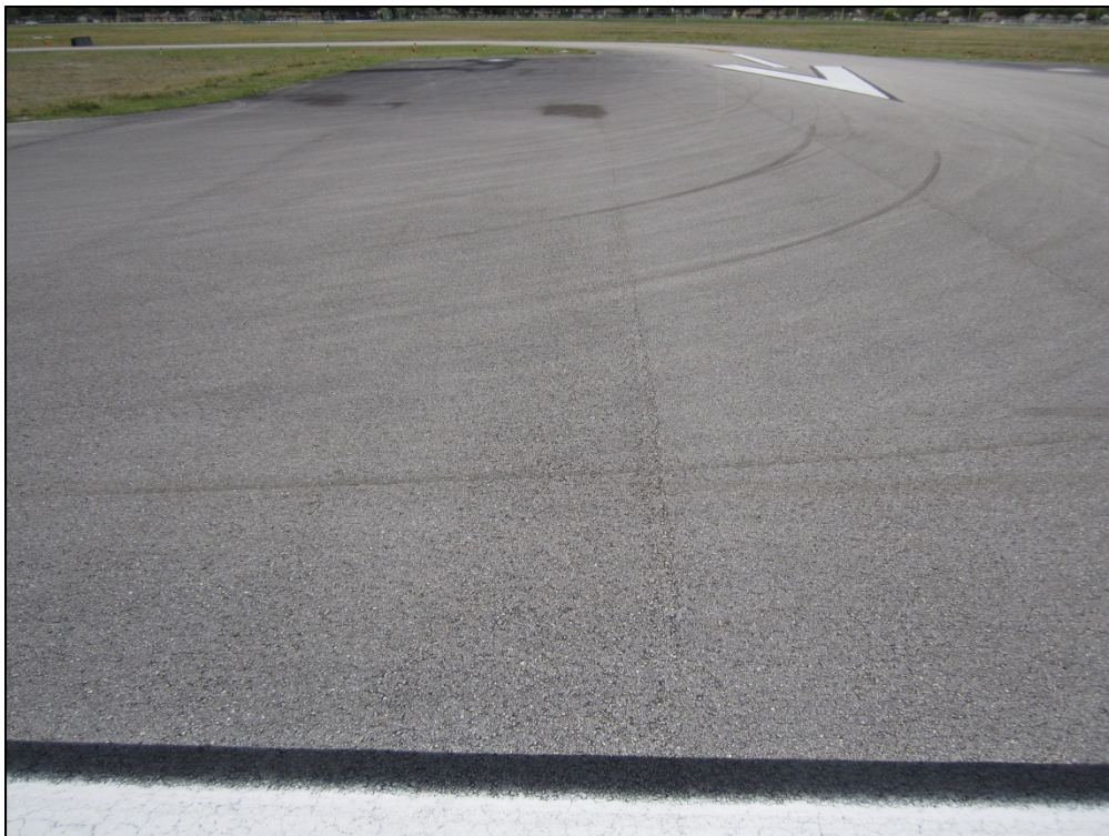
Runway 19R-01L, Section 6120, Sample Unit 95 – Low severity (52) Weathering and Raveling
