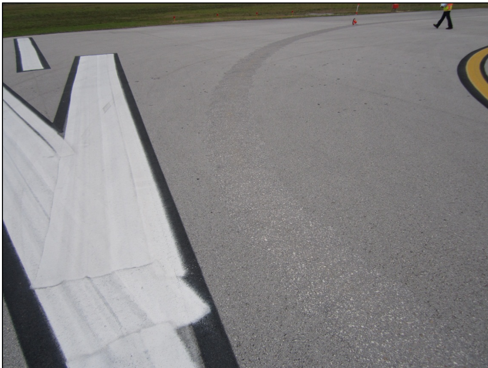
Runway 19R-01L, Section 6105, Sample Unit 158 – Low severity (52) Weathering and Raveling
