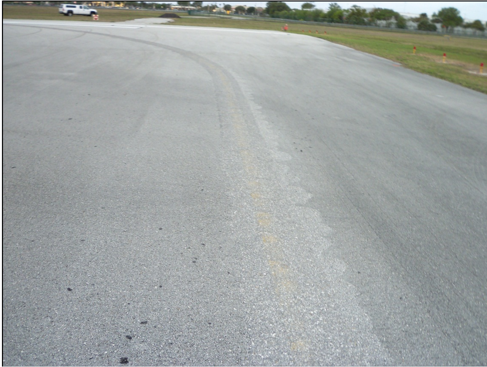
Taxiway Bravo, Section 215, Sample Unit 400 – Low severity (52) Weathering and Raveling
