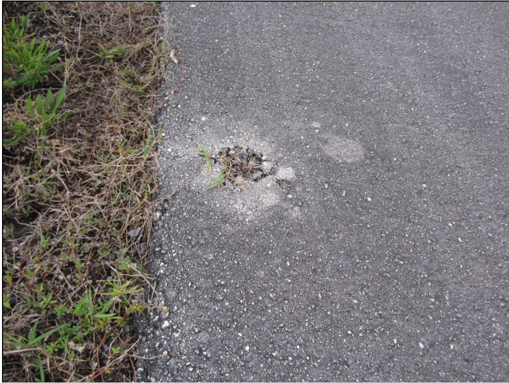
Runway 19R-01L, Section 6105, Sample Unit 117 – High severity (52) Weathering and Raveling
