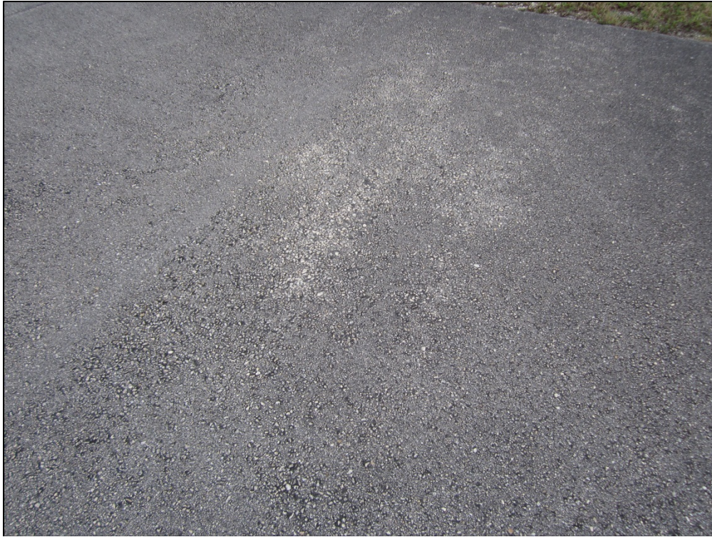
Taxiway Papa, Section 2105, Sample Unit 100 – Low severity (52) Weathering and Raveling
