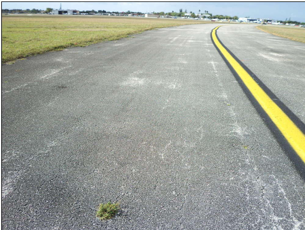
Taxiway Juliet, Section 1110, Sample Unit 111 – Medium severity (52) Weathering and Raveling, low severity (48) Longitudinal and Transverse Cracking, low severity (41) Alligator Cracking, low severity (43) Block Cracking
