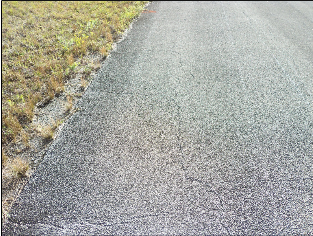
Taxiway November, Section 1405, Sample Unit 118 – Low severity (52) Weathering and Raveling, low severity (48) Longitudinal and Transverse Cracking
