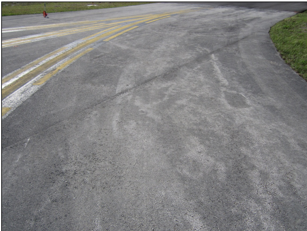
Taxiway P-2, Section 1625, Sample Unit 101 – Low severity (52) Weathering and Raveling, low severity (48) Longitudinal and Transverse Cracking
