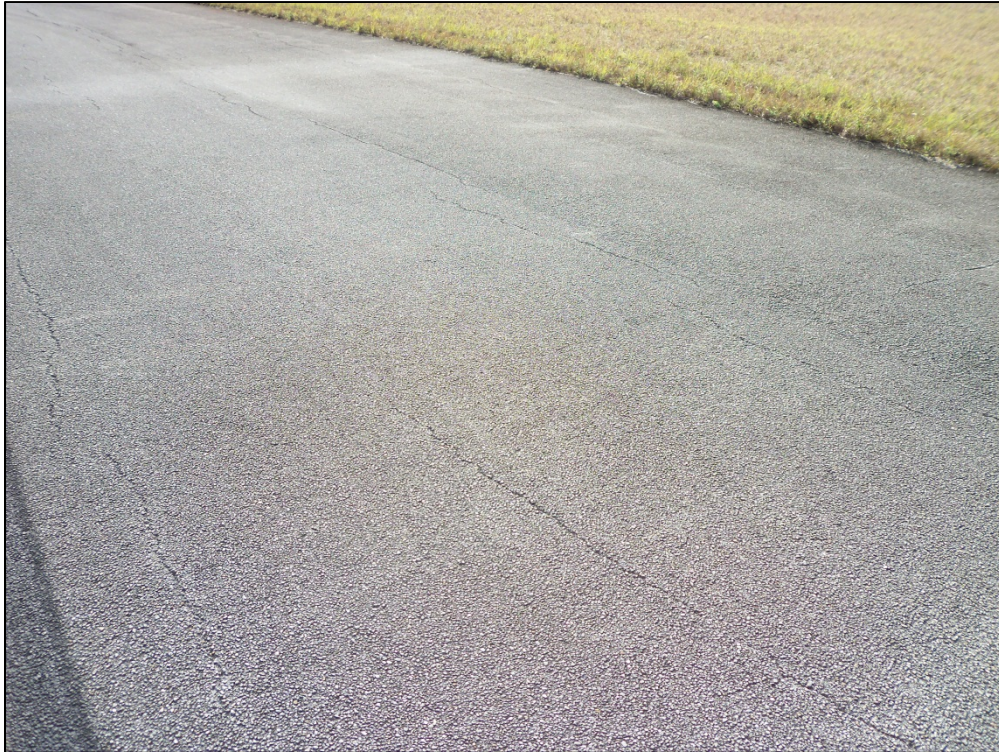
Taxiway November, Section 1405, Sample Unit 127 – Low severity (52) Weathering and Raveling, low severity (48) Longitudinal and Transverse Cracking
