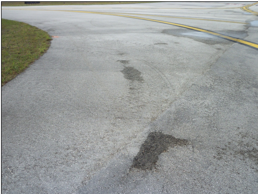
Taxiway Bravo, Section 205, Sample Unit 102 – Low and medium severity (52) Weathering and Raveling, low severity (48) Longitudinal and Transverse Cracking
