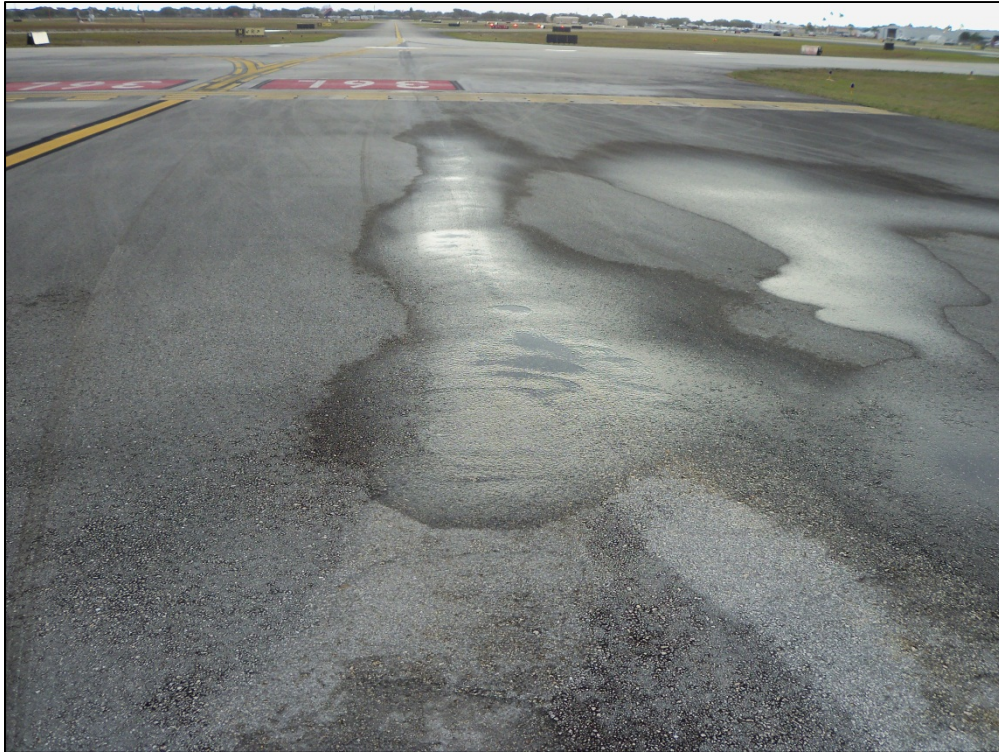
Taxiway Mike, Section 2005, Sample Unit 100 – Low severity (52) Weathering and Raveling, low severity (45) Depression
