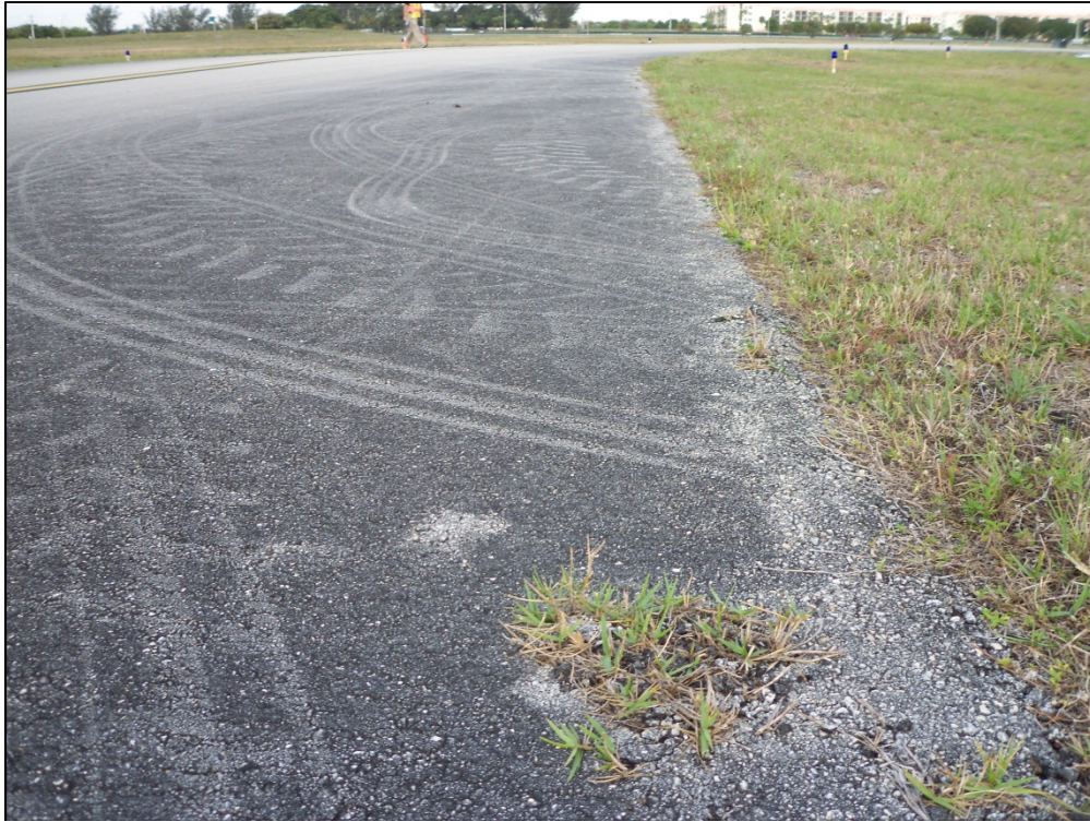
Taxiway Lima, Section 1225, Sample Unit 201 – Low and high severity (52) Weathering and Raveling
