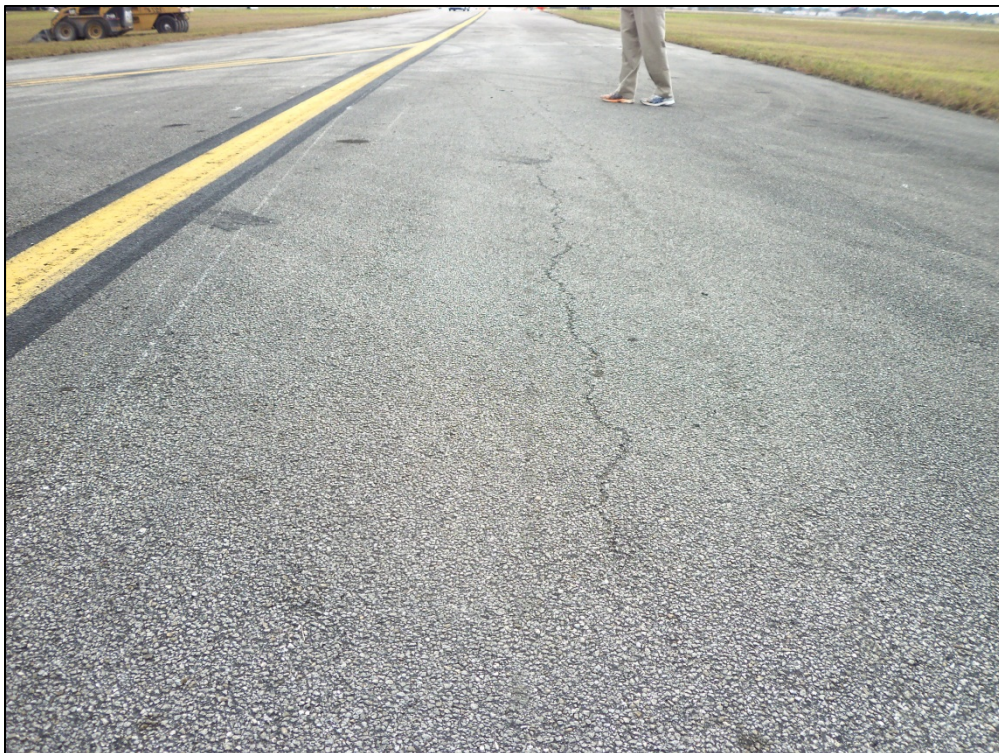
Taxiway November, Section 1405, Sample Unit 107 – Low severity (52) Weathering and Raveling, low severity (48) Longitudinal and Transverse Cracking
