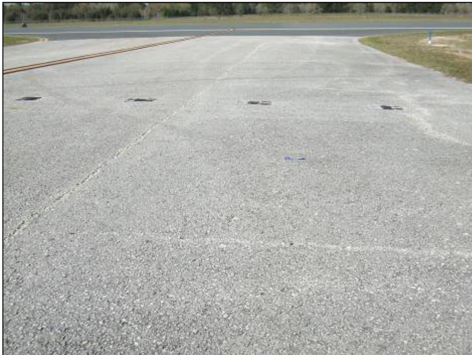
Taxiway Echo 6, Section 530, Sample Unit 601 – Low severity (43) Block Cracking, low severity (48) Longitudinal and Transverse Cracking, low and medium severity (52) Weathering and Raveling.
