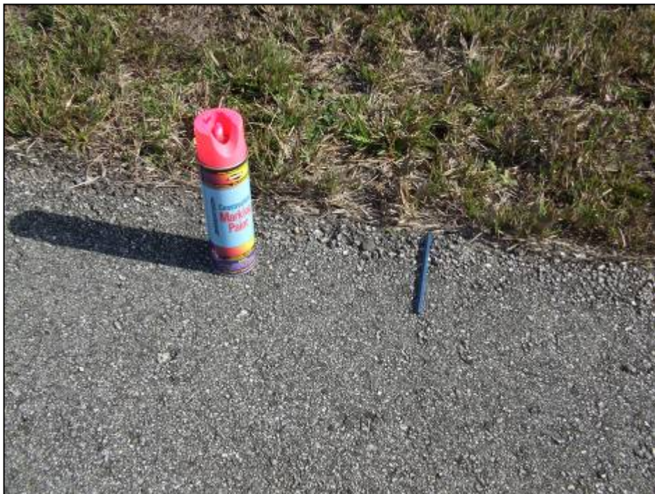
Parallel Taxiway to RW 8-26, Section 106, Sample Unit 200 – Low and medium severity (48) Longitudinal and Transverse Cracking; low, medium and high severity (52) Weathering and Raveling.
