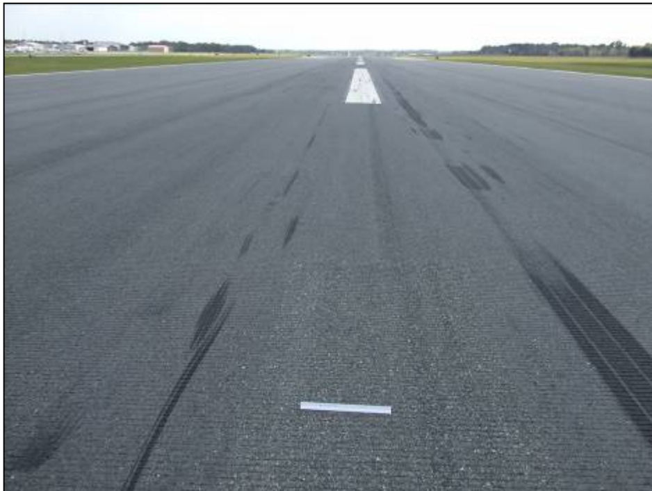
Runway 18-36, Section 6180, Sample Unit 390 – Low severity (50) Patch, low severity (52) Weathering and Raveling.
