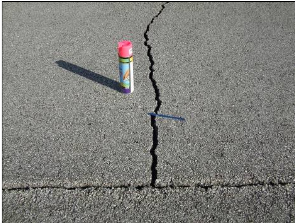
Runway 8-26, Section 6205, Sample Unit 128 – Low, medium and high severity (48) Longitudinal and Transverse Cracking; low and medium severity (52) Weathering and Raveling.
