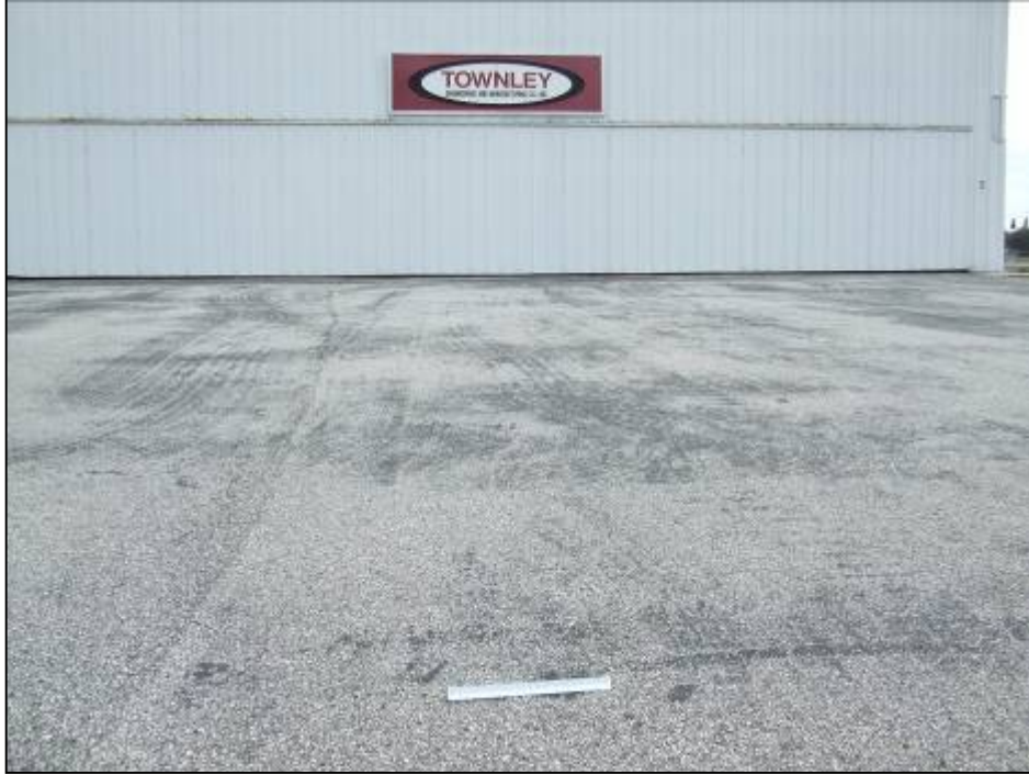
South Apron, Section 4305, Sample Unit 100 – Low severity (45) Depression, low severity (48) Longitudinal and Transverse Cracking, low and medium severity (52) Weathering and Raveling, low severity (56) Swelling
