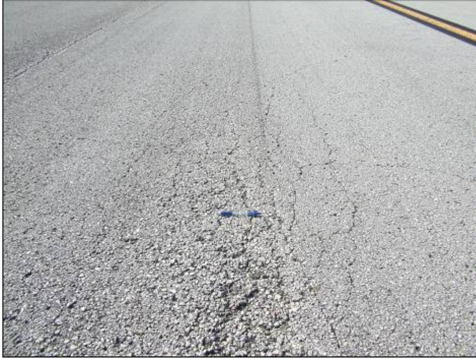
Taxiway Echo, Section 540, Sample Unit 112 – Low severity (41) Alligator Crack, low severity (42) Bleeding, low and medium severity (48) Longitudinal and Transverse Cracking, low severity (50) Patching, low and medium severity (52) Weathering and Raveling.
