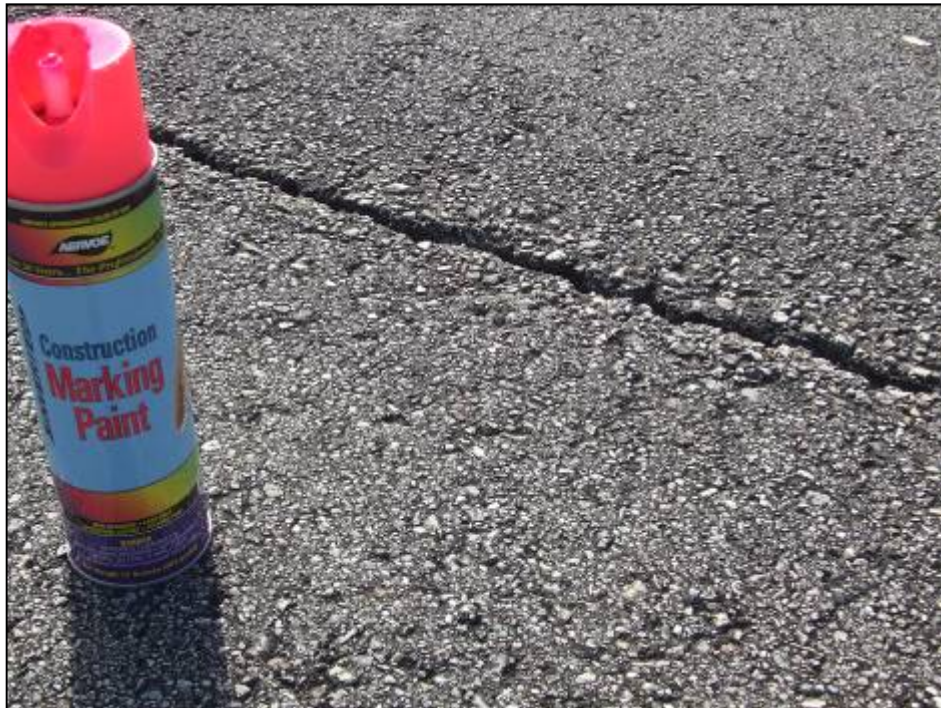
Runway 8-26, Section 6205, Sample Unit 112 – Low, medium and high severity (48) Longitudinal and Transverse Cracking; low and medium severity (52) Weathering and Raveling.
