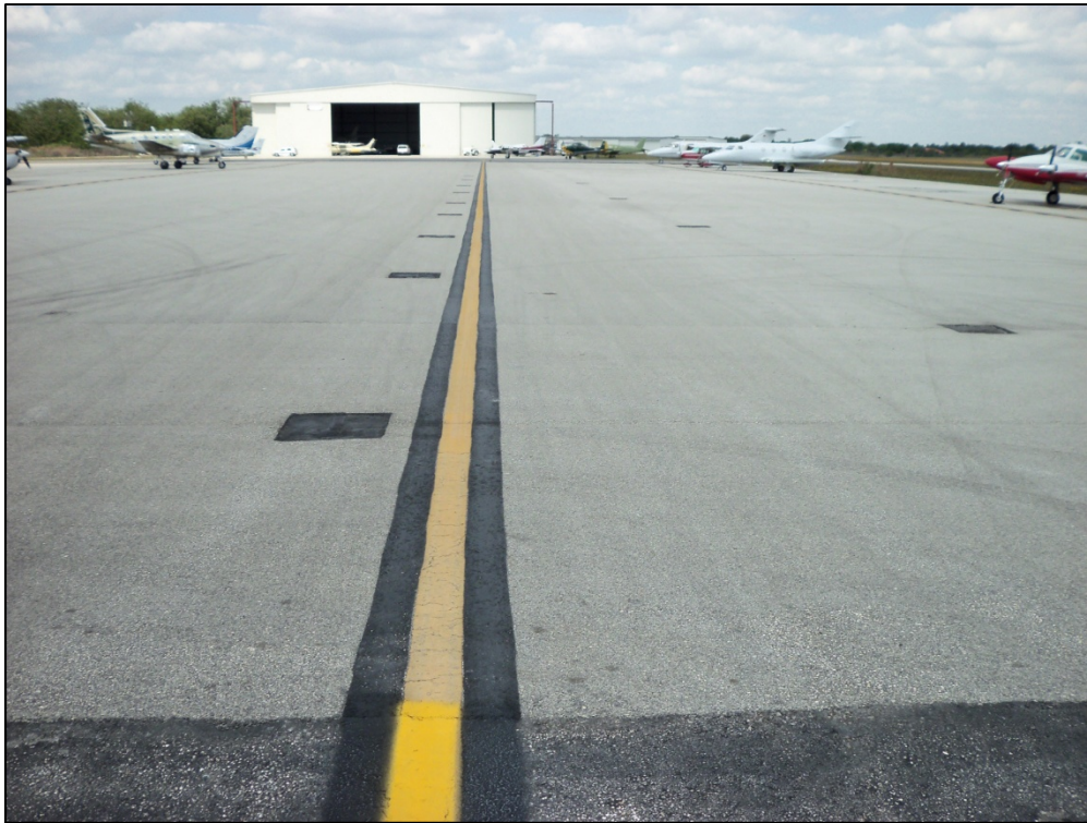
Apron, Section 4105, Sample Unit 460 – Low severity (50) Patching
