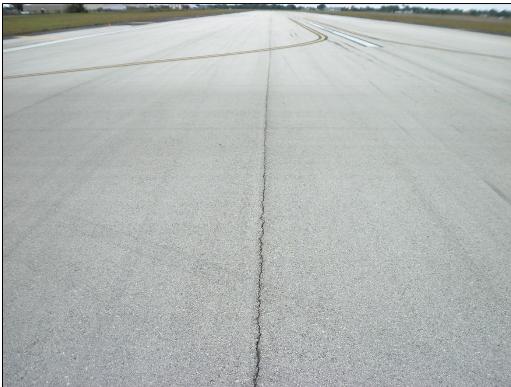
Runway 5-23, Section 6105, Sample Unit 129 – Low severity (48) Longitudinal Cracking and low severity (52) Weathering and Raveling
