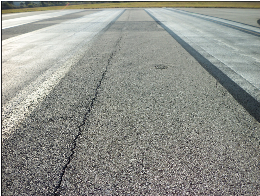
Runway 14-32, Section 6205, Sample Unit 301 – Low severity (48) Longitudinal Cracking, low severity (52) Weathering and Raveling, low severity (56) Swell
