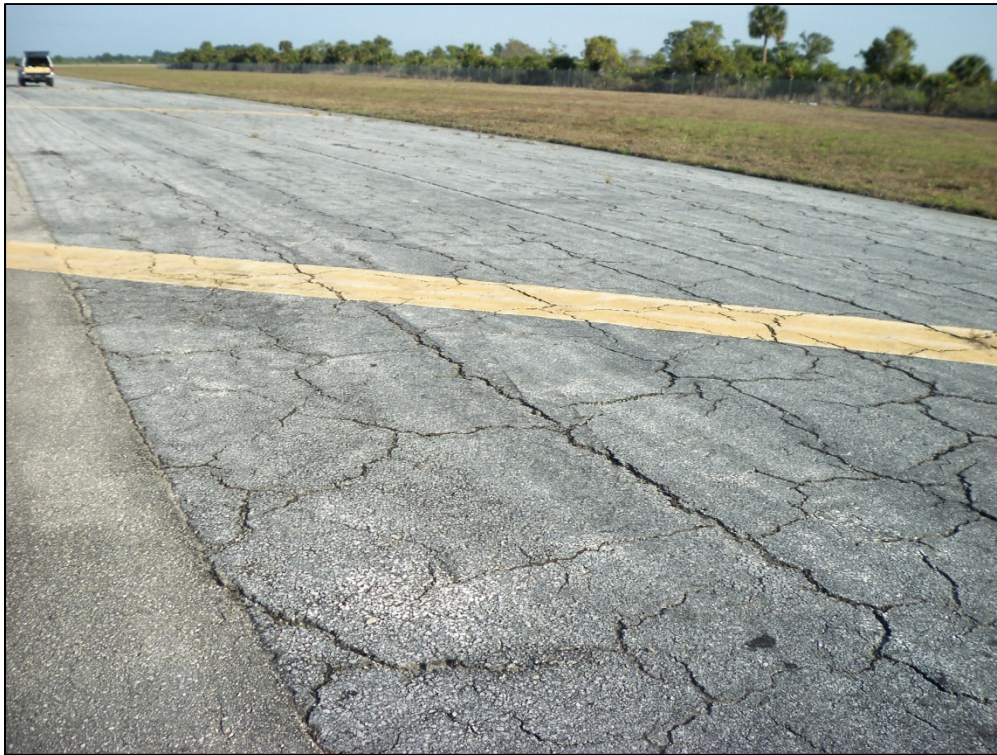
Runway 14-32 Shoulder, Section 6210, Sample Unit 500 – Medium and high severity (43) Block Cracking, medium severity (52) Weathering and Raveling
