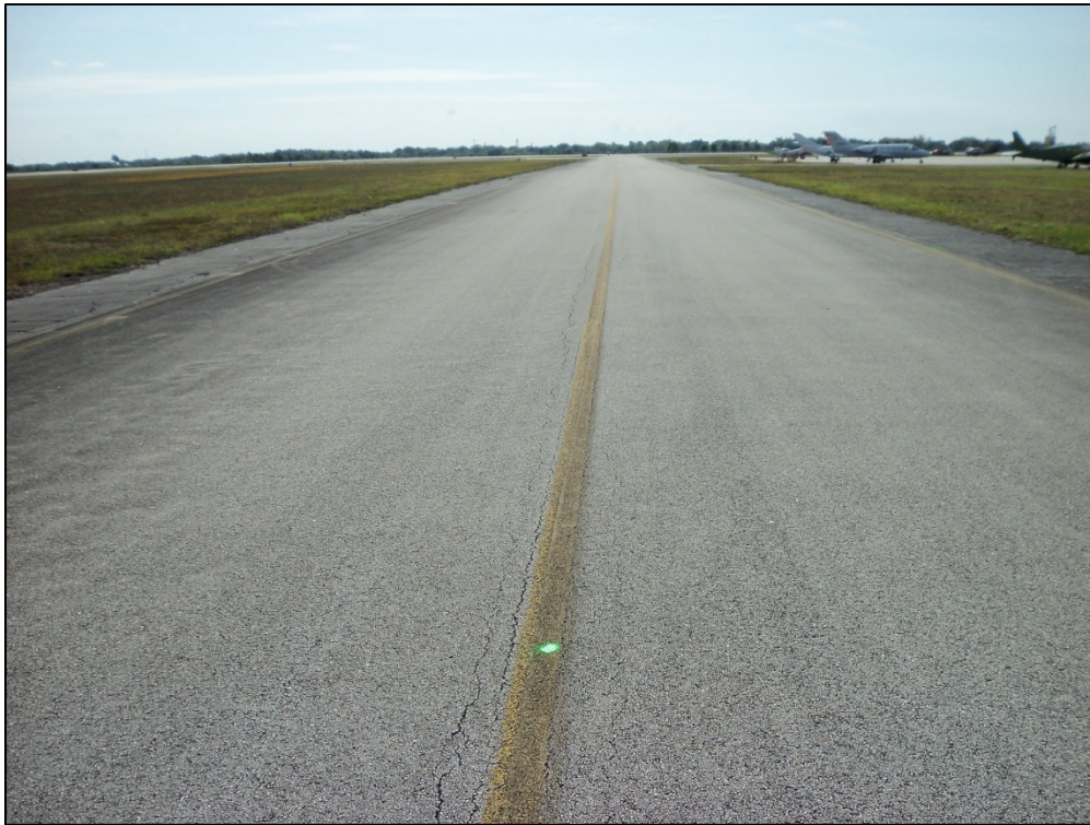
Taxiway Bravo, Section 205, Sample Unit 137 – Low severity (48) Longitudinal Cracking, low severity (52) Weathering and Raveling
