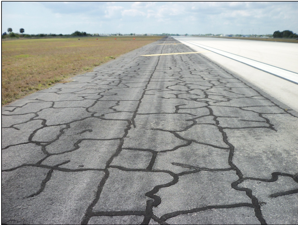
Runway 5-23 Shoulder, Section 6110 – Medium and high severity (43) Block Cracking, medium severity (52) Weathering and Raveling
