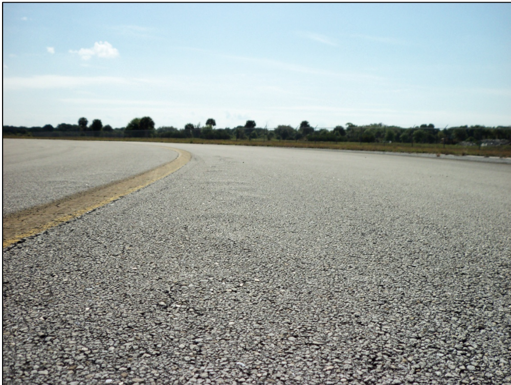
Taxiway Bravo, Section 205, Sample Unit 105 – Low severity (48) Longitudinal and Transverse Cracking, low severity (52) Weathering and Raveling, low severity (56) Swell
