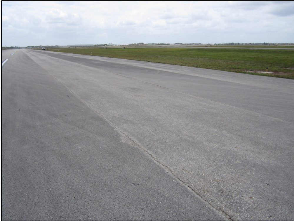
Runway 9R-27L, Section 6410, Sample Unit 182 – Low severity (48) Longitudinal and Transverse Cracking, low severity (52) Weathering and Raveling
