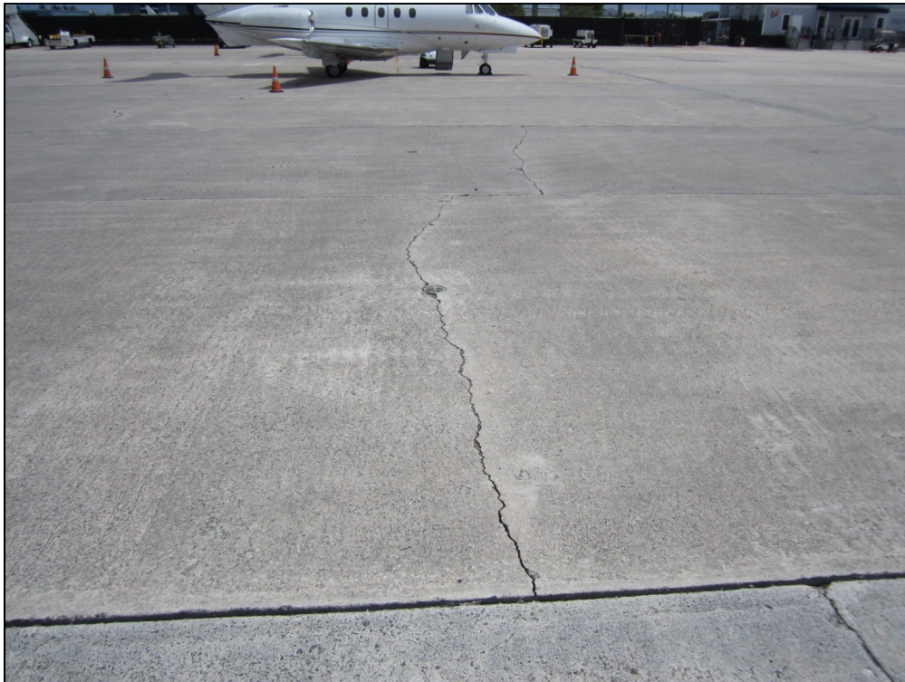
Center Apron, Section 4110, Sample Unit 403 – Low severity (63) Longitudinal, Transverse, and Diagonal Cracking; low severity (65) Joint Seal Damage
