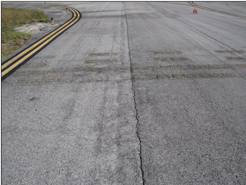
Taxiway Charlie, Section 310, Sample Unit 602 – Low severity (48) Longitudinal and Transverse Cracking, low severity (56) Swelling, low severity (52) Weathering and Raveling
