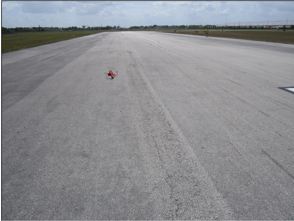
Runway 9R-27L, Section 6405, Sample Unit 112 – Low and medium severity (52) Weathering and Raveling, low severity (48) Longitudinal and Transverse Cracking
