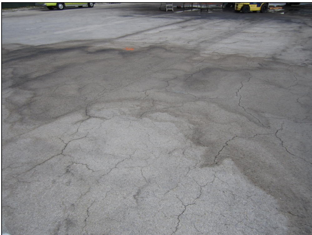
Northeast Apron, Section 4305, Sample Unit 428 – Low severity (43) Block Cracking, low severity (52) Weathering and Raveling, (49) Oil Spillage
