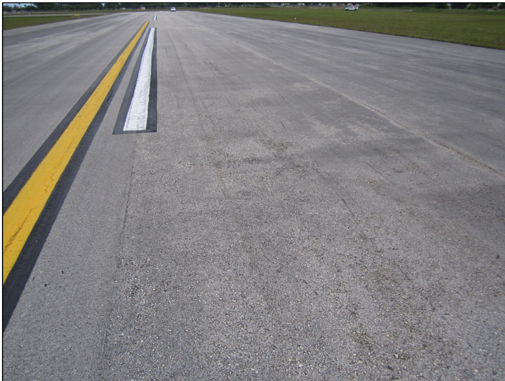
Runway 9R-27L, Section 6410, Sample Unit 171 – Low severity (48) Longitudinal and Transverse Cracking, low and medium severity (52) Weathering and Raveling
