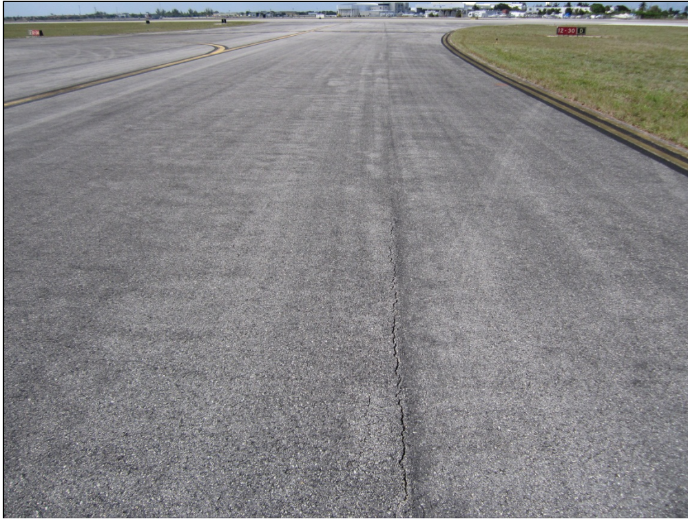
Taxiway Delta, Section 410, Sample Unit 312 – Low severity (48) Longitudinal and Transverse Cracking, low severity (52) Weathering and Raveling, low severity (56) Swelling
