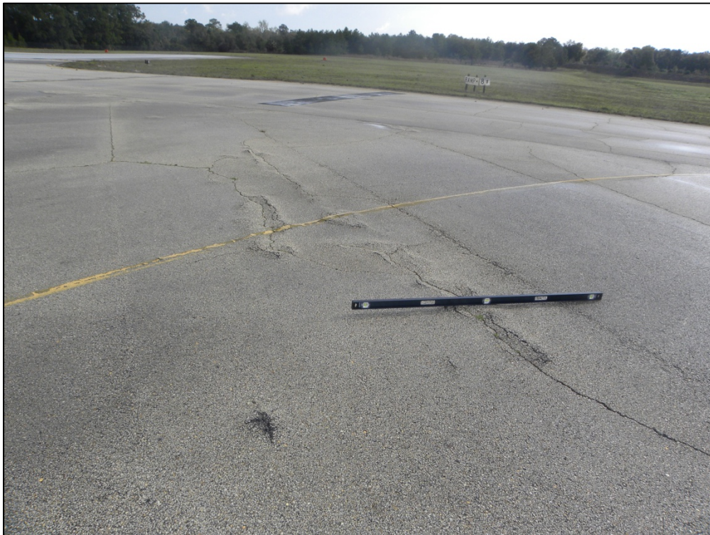
Taxiway Charlie, Section 805, Sample Unit 100 – Low and medium severity (43) Block Cracking, medium severity (48) Longitudinal and Transverse Cracking, medium severity (52) Weathering and Raveling, medium severity (56) Swell
