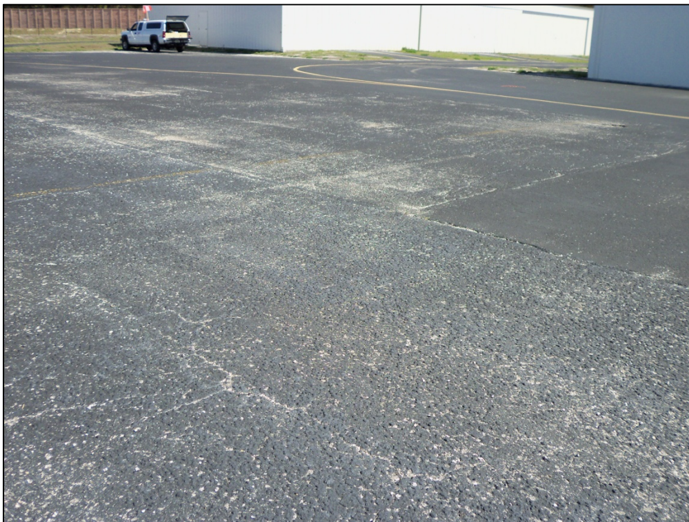
Apron, Section 4205, Sample Unit 111 – Low severity (48) Longitudinal and Transverse Cracking, low severity (43) Block Cracking, medium severity (52) Weathering and Raveling
