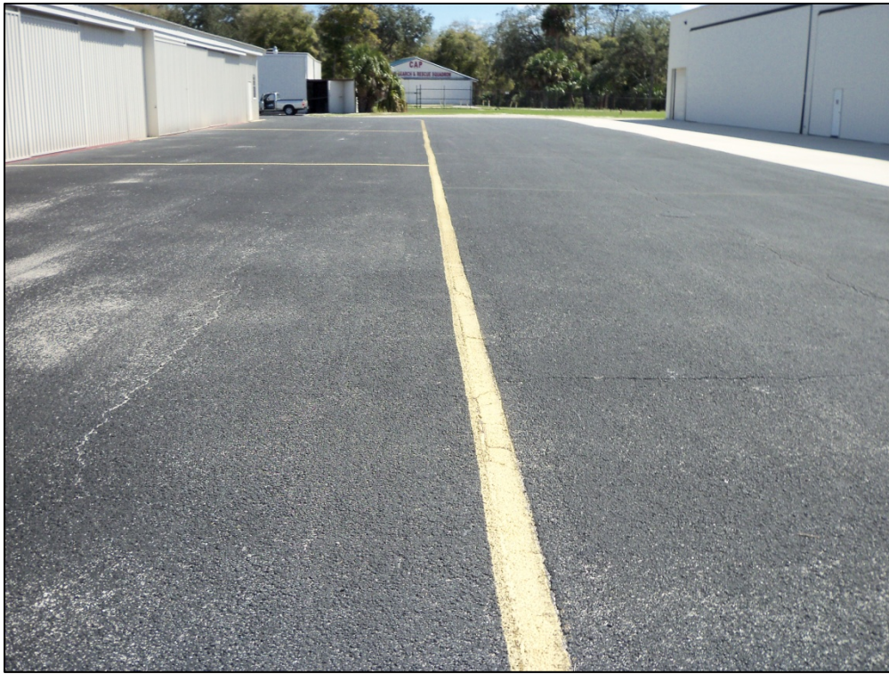
Apron, Section 4305, Sample Unit 104 – Low severity (48) Longitudinal and Transverse Cracking, low severity (43) Block Cracking, medium severity (52) Weathering and Raveling
