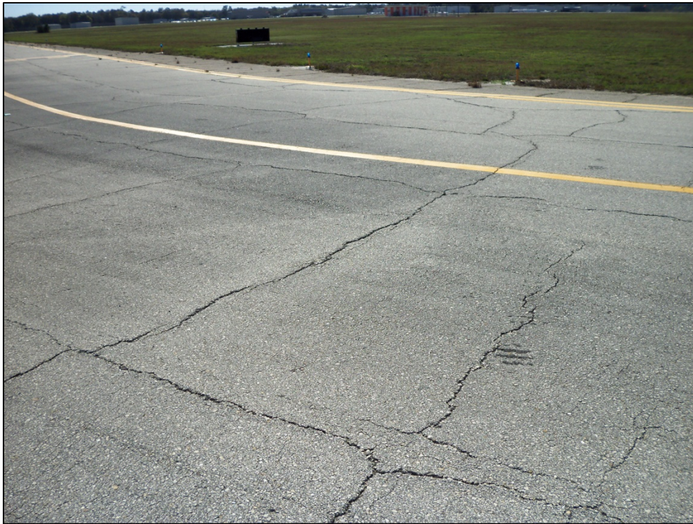
Taxiway Echo, Section 505, Sample Unit 101 – Low and medium severity (43) Block Cracking, low severity (52) Weathering and Raveling
