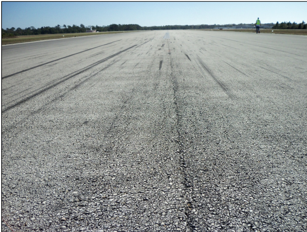
Runway 8-26, Section 6105, Sample Unit 117 – Medium severity (48) Longitudinal and Transverse Cracking, low and medium severity (52) Weathering and Raveling
