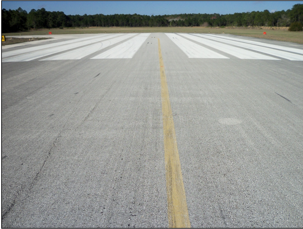
Runway 8-26, Section 6105, Sample Unit 103 – Low severity (48) Longitudinal and Transverse Cracking, low and medium severity (52) Weathering and Raveling
