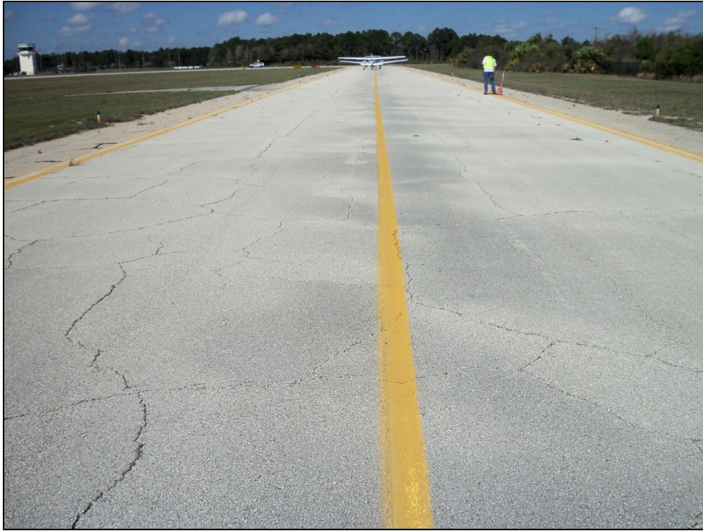
Taxiway Echo, Section 505, Sample Unit 107 – Low and medium severity (43) Block Cracking, low severity (52) Weathering and Raveling
