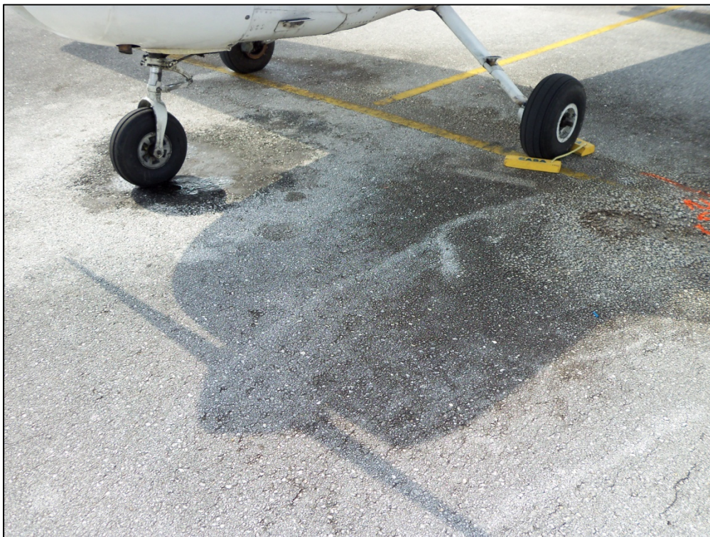
Apron, Section 4105, Sample Unit 205 – Low and medium severity (48) Longitudinal and Transverse Cracking, (49) Oil Spillage, low severity (52) Weathering and Raveling
