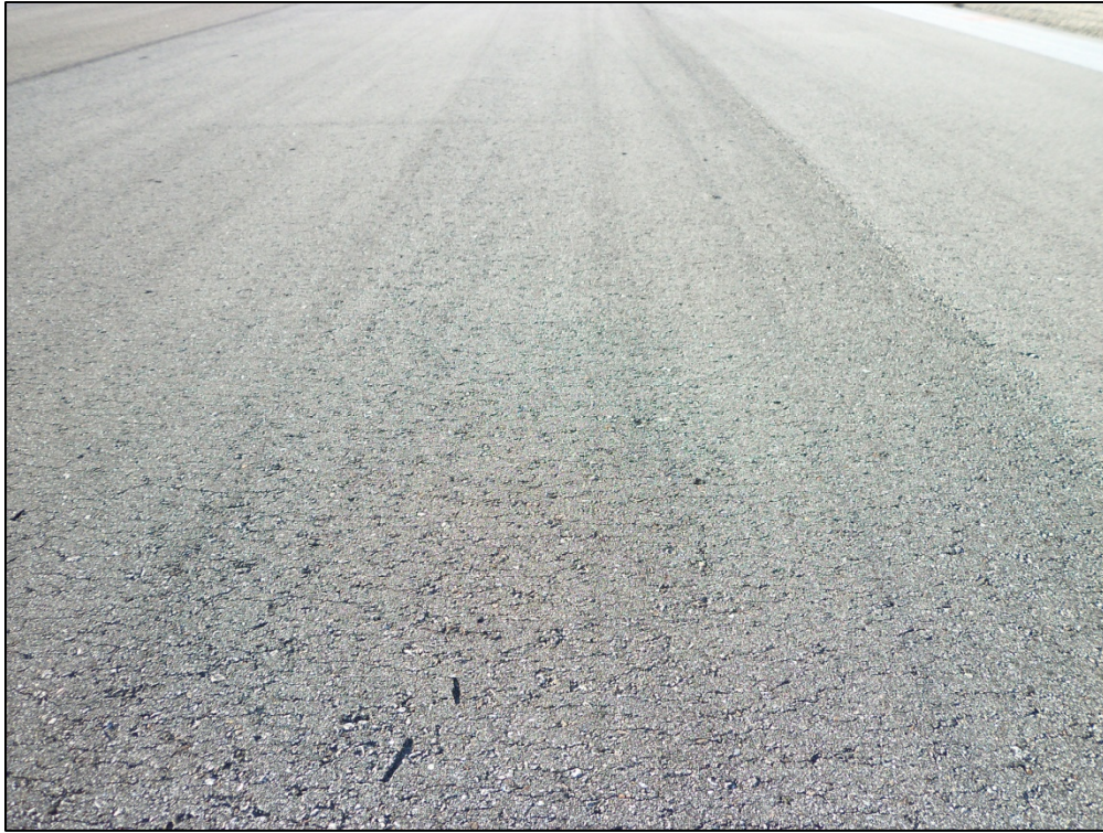
Runway 17-35, Section 6205, Sample Unit 164 – Low severity (52) Weathering and Raveling
