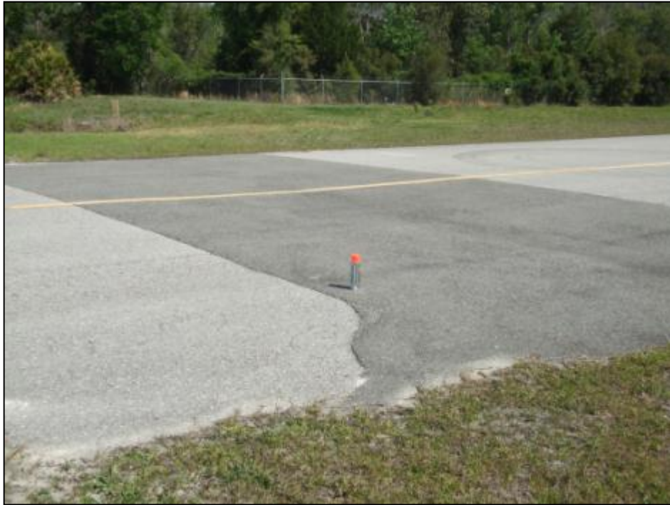
Taxiway Charlie, Section 310, Sample Unit 115 – Low severity (48) Longitudinal and Transverse Cracking, low severity (50) Patching, low and medium severity (52) Weathering and Raveling.
