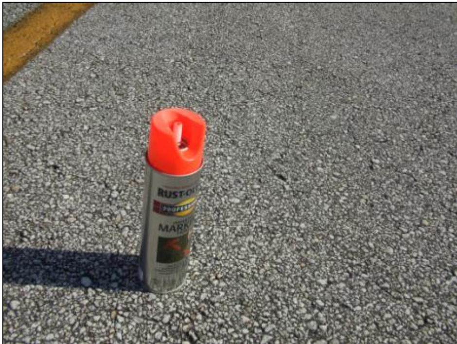
Taxiway Charlie, Section 305, Sample Unit 106 – Low severity (48) Longitudinal and Transverse Cracking, low severity (50) Patching, low and medium severity (52) Weathering and Raveling, low severity (56) Swelling.
