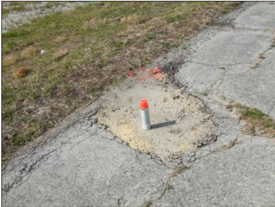
Taxiway Bravo, Section 705, Sample Unit 105 – Medium severity (41) Alligator Cracking, low and medium severity (43) Block Cracking, low and medium severity (50) Patching, medium and high severity (52) Weathering and Raveling, low severity (56) Swelling.
