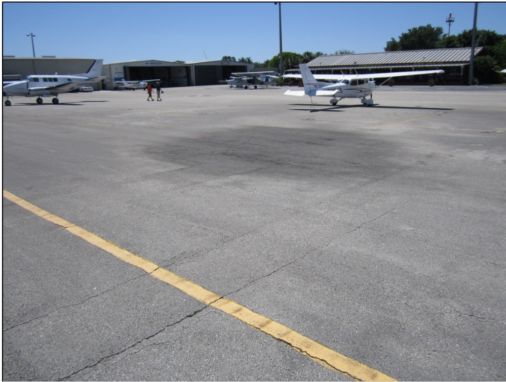
GA Apron, Section 4115, Sample Unit 614 – Low and medium severity (48) Longitudinal and Transverse Cracking, low and high severity (52) Weathering and Raveling, low severity (56) Swelling
