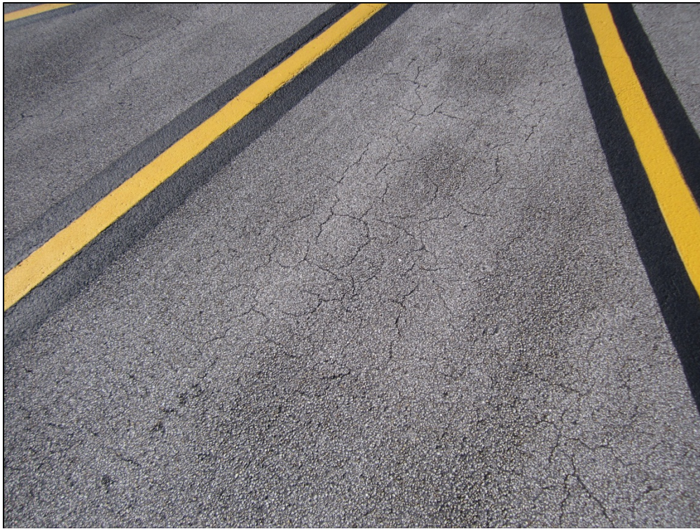
Taxiway A-1, Section 120, Sample Unit 302 – Low severity (52) Weathering and Raveling, low severity (43) Block Cracking
