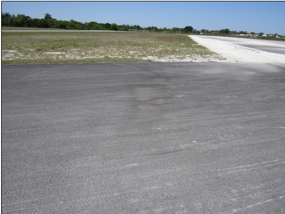
Runway 3-21, Section 6305, Sample Unit 156 – Low severity (52) Weathering and Raveling, low severity (45) Depression
