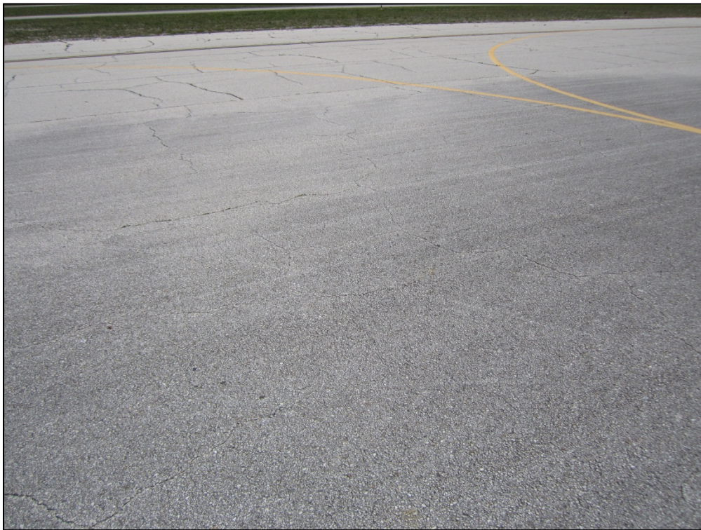
GA Apron, Section 4115, Sample Unit 720 – Low severity (48) Longitudinal and Transverse Cracking, low severity (43) Block Cracking, low severity (52) Weathering and Raveling
