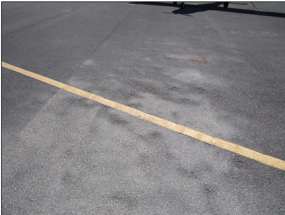
GA Apron, Section 4105, Sample Unit 302 – Low severity (48) Longitudinal and Transverse Cracking, low severity (52) Weathering and Raveling, low severity (56) Swelling
