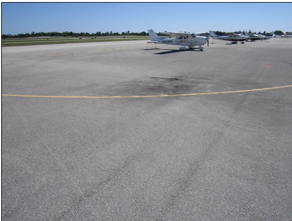
GA Apron, Section 4115, Sample Unit 661 – Low severity (48) Longitudinal and Transverse Cracking, low and medium (52) Weathering and Raveling, low severity (45) Depression
