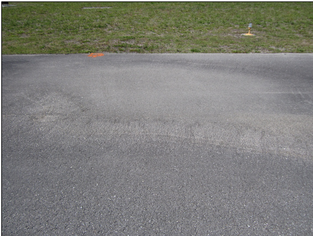
Runway 9-27, Section 6105, Sample Unit 319 – Low severity (52) Weathering and Raveling, low severity (45) Depression
