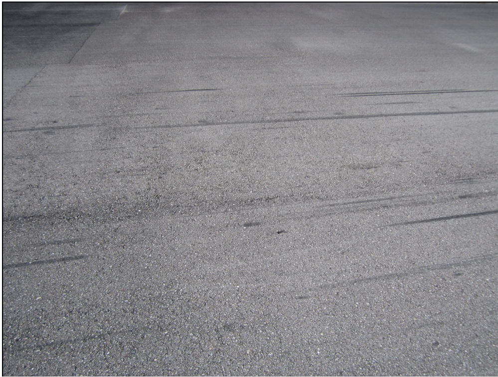
Runway 9-27, Section 6105, Sample Unit 6105, Sample Unit 313 – Low severity (48) Longitudinal and Transverse Cracking, low severity (52) Weathering and Raveling
