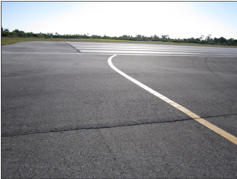
Taxiway Bravo, Section 215, Sample Unit 100 – Low severity (48) Longitudinal and Transverse Cracking, low severity (56) Swelling
