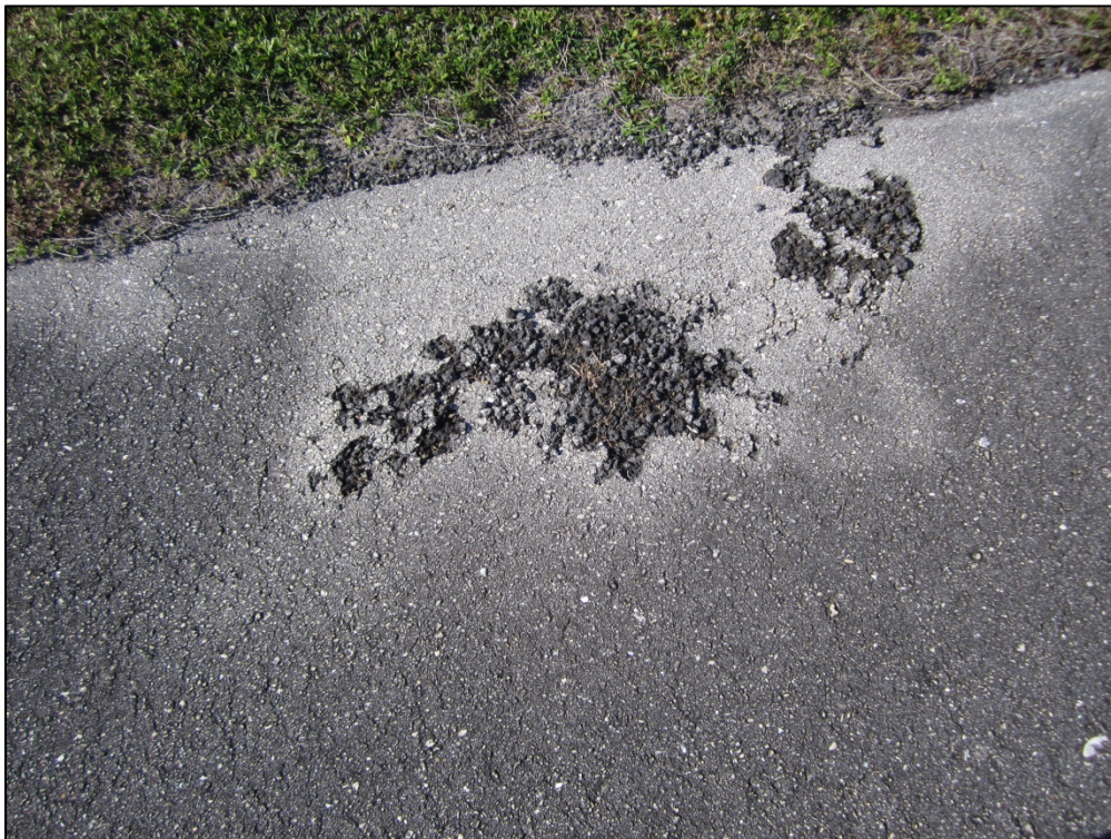
Taxiway Alpha, Section 310, Sample Unit 322 – High severity (52) Weathering and Raveling
