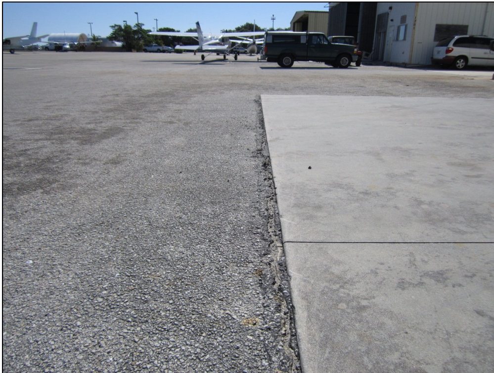
GA Apron, Section 4105, Sample Unit 258 – Low severity (52) Weathering and Raveling, low severity (54) Shoving, (49) Oil Spillage
