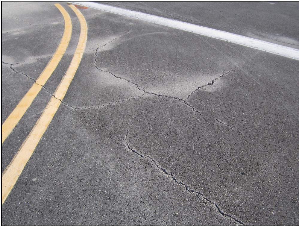
Taxiway B-1, Section 220, Sample Unit 100 – Low and medium severity (48) Longitudinal and Transverse Cracking, low severity (52) Weathering and Raveling
