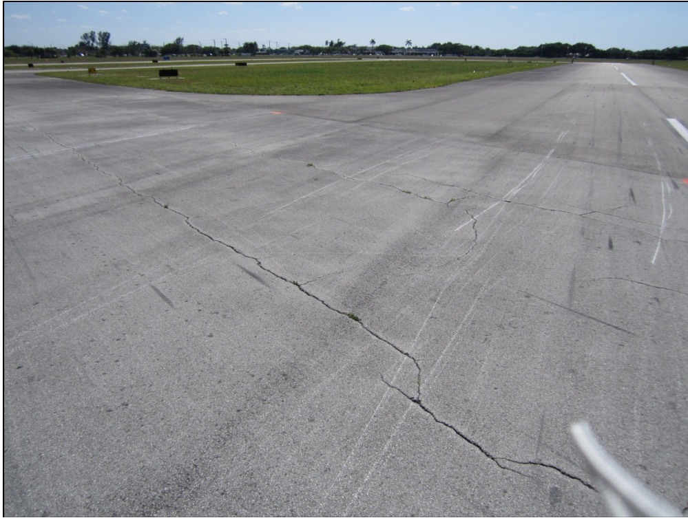
Runway 3-21, Section 6310, Sample Unit 109 – Low, medium, and high severity (48) Longitudinal and Transverse Cracking; low severity (52) Weathering and Raveling
