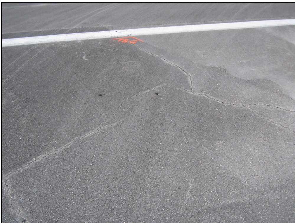
Runway 3-21, Section 6305, Sample Unit 156 – Low severity (52) Weathering and Raveling, low and medium severity (48) Longitudinal and Transverse Cracking
