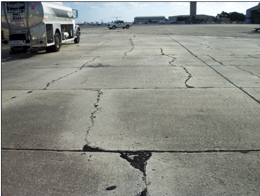
Southwest GA Apron, Section 4307, Sample Unit 549 – Medium severity (72) Shattered Slab, low severity (74) Joint Spalling, medium severity (65) Joint Seal Damage
