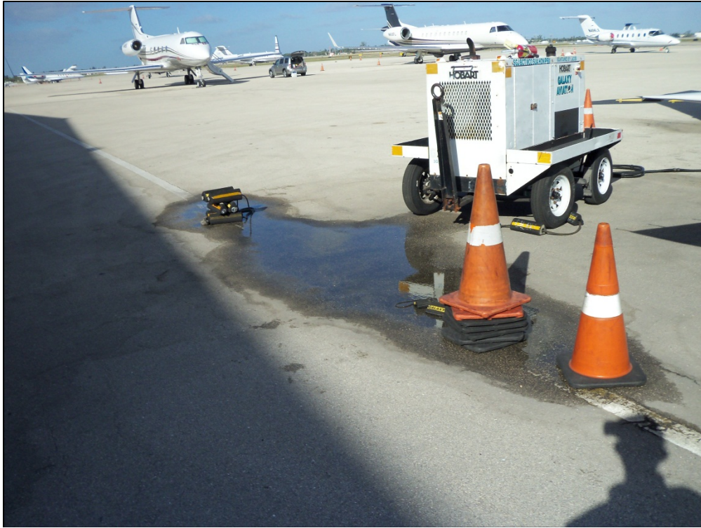
Southwest GA Apron, Section 4305, Sample Unit 370 – Low severity (45) Depression, medium severity (52) Weathering and Raveling, low severity (48) Longitudinal and Transverse Cracking
