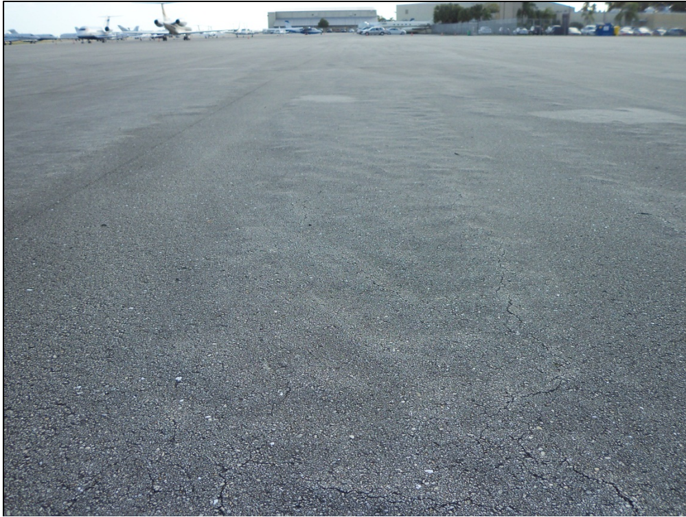
Southwest GA Apron, Section 4305, Sample Unit 552 – Low Severity (56) Swelling, Low severity (48) Longitudinal and Transverse Cracking
