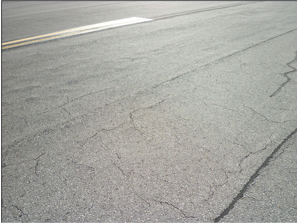
Taxiway R, Section 1810, Sample Unit 249 – Low severity (48) Longitudinal and Transverse Cracking, low severity (56) Swelling, medium severity (52) Weathering and Raveling
