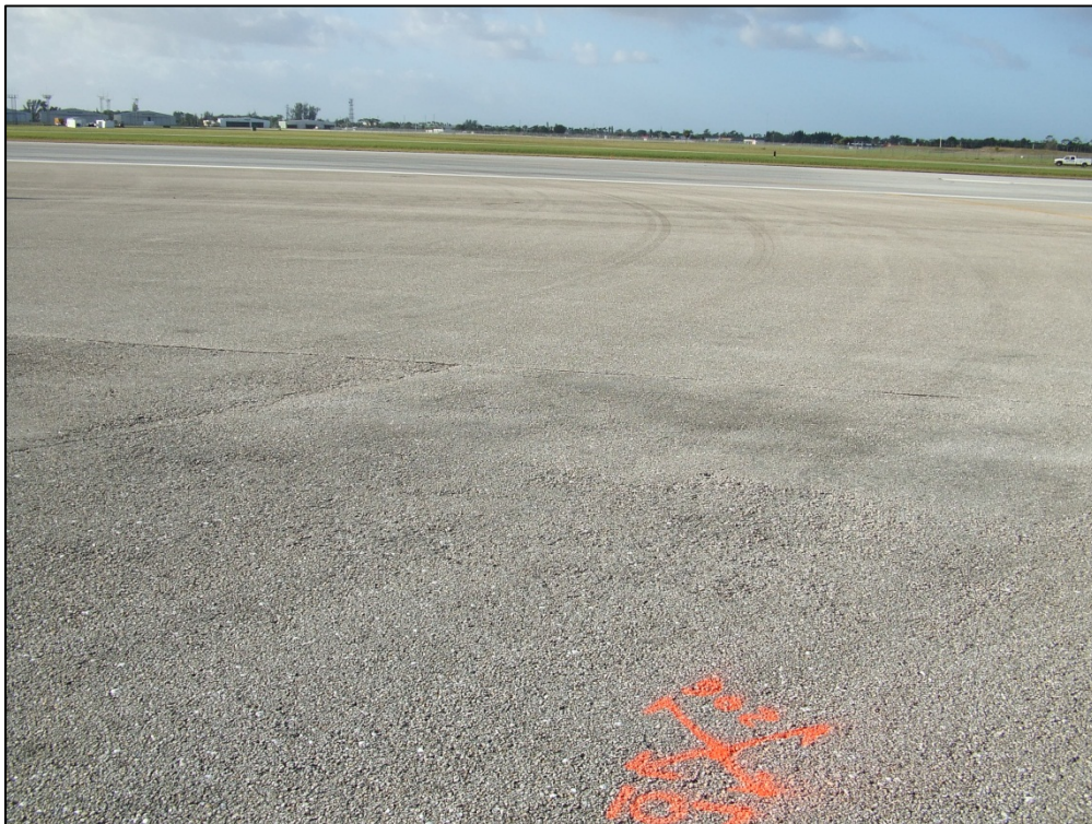
Taxiway B, Section 205, Sample Unit 206 – Low severity (48) Longitudinal and Transverse Cracking, low severity (52) Weathering and Raveling
