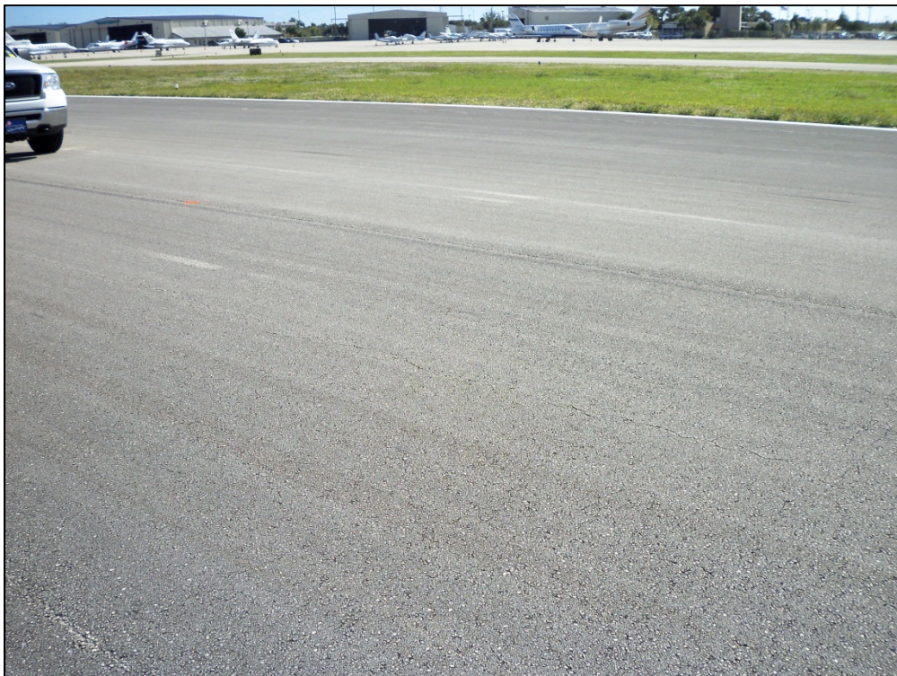
Runway 10R-28L, Section 6210, Sample Unit 139 – Low severity (52) Longitudinal and Transverse Cracking, low severity (48) Weathering and Raveling
