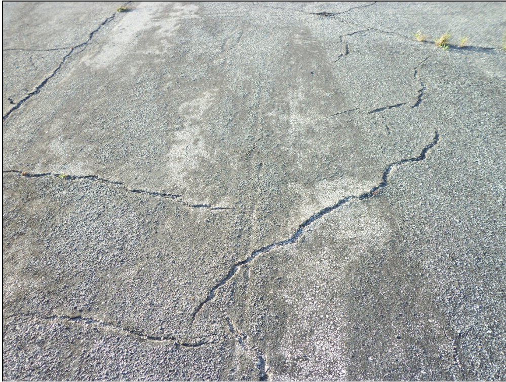
Taxiway E, Section 505, Sample Unit 163 – Medium severity (43) Block Cracking, medium severity (52) Weathering and Raveling
