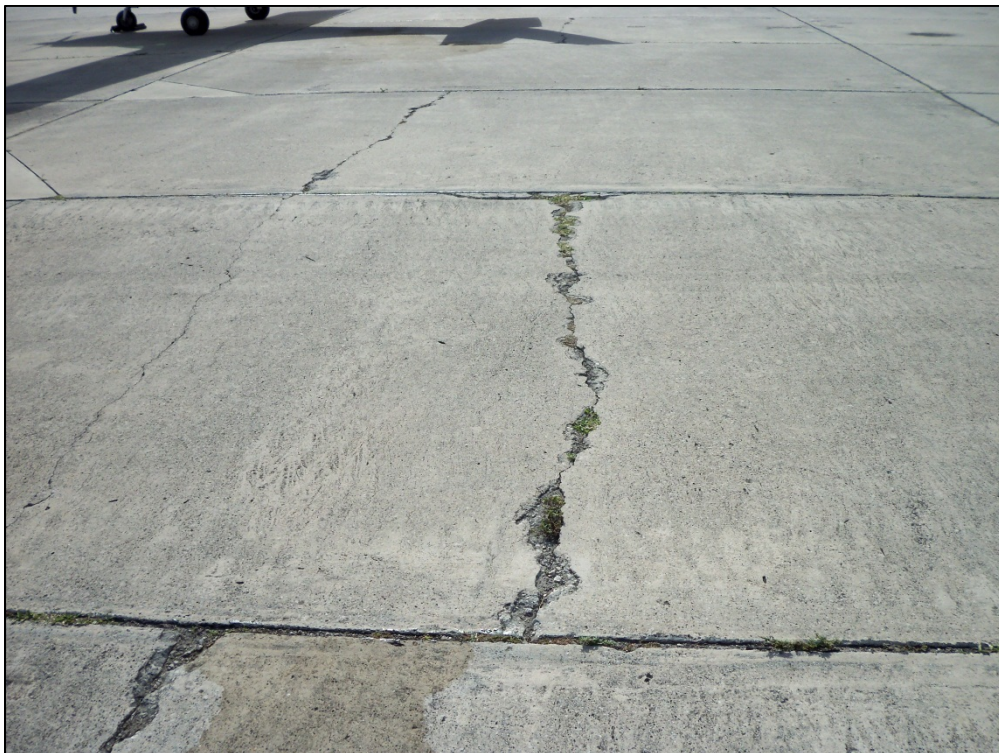
Southeast GA Apron, Section 4510, Sample Unit 414 – Low Severity (74) Joint Spalling, low and medium severity (63) Longitudinal, Transverse, and Diagonal Cracking
