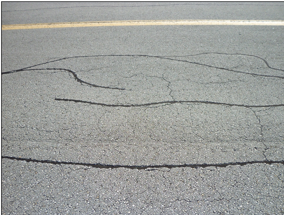
Taxiway R, Section 1805, Sample Unit 215 – Low severity (48) Longitudinal and Transverse Cracking, low severity (43) Block Cracking, low severity (52) Weathering and Raveling
