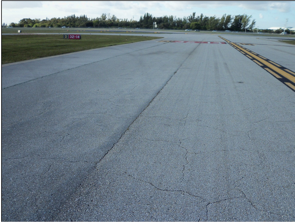
Taxiway D, Section 405, Sample Unit 308 – Low severity (48) Longitudinal and Transverse Cracking, low severity (56) Swelling
