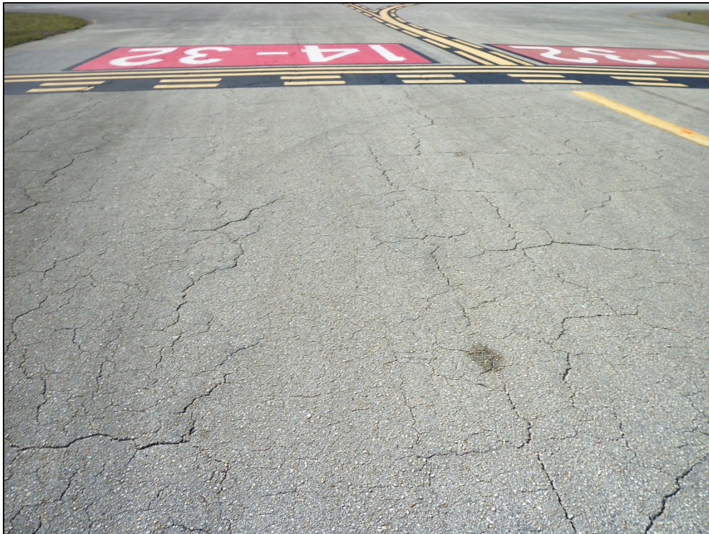
Taxiway F, Section 630, Sample Unit 104 – Low severity (52) Weathering and Raveling, low severity (43) Block Cracking
