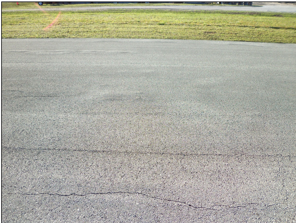
Taxiway E, Section 502, Sample Unit 107 – low severity (48) Longitudinal and Transverse Cracking, low severity (56) Swelling, low severity (52) Weathering and Raveling
