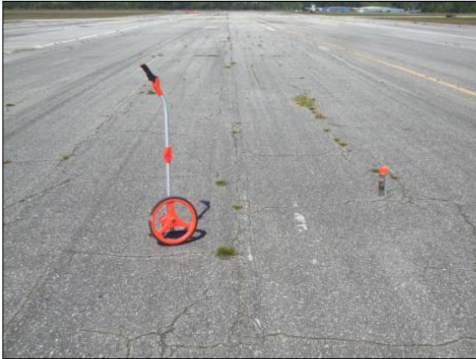
Runway 12-30, Section 6315, Sample Unit 143 – Low severity (41) Alligator Cracking, low and medium severity (43) Block Cracking, low severity (50) Patching, low and medium severity (52) Weathering and Raveling.
