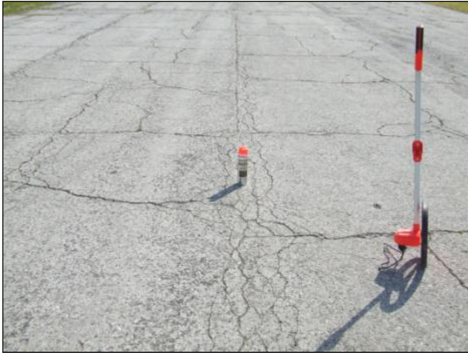
Taxiway Bravo, Section 705, Sample Unit 101 – Medium severity (41) Alligator Cracking; medium severity (43) Block Cracking; low severity (45) Depression; low, medium and high severity (52) Weathering and Raveling.
