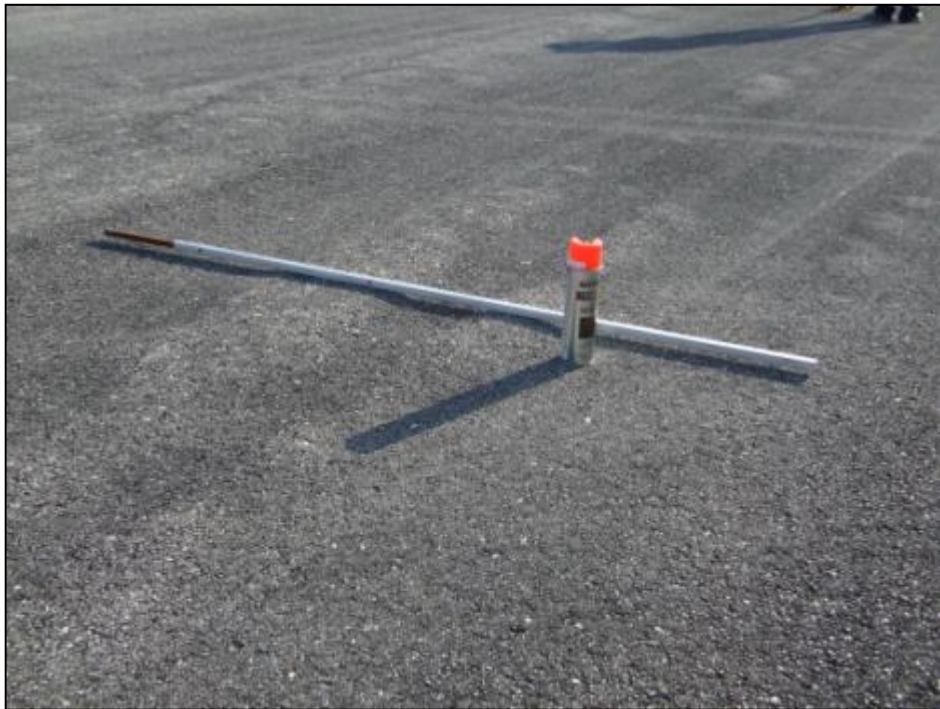
Runway 9-27, Section 6105, Sample Unit 105 – Low severity (48) Longitudinal and Transverse Cracking, low severity (52) Weathering and Raveling, low severity (56) Swelling.
