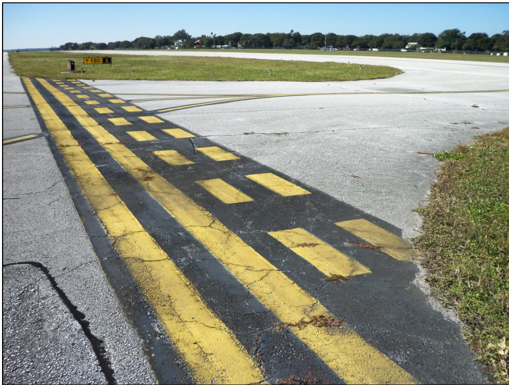
Taxiway D, Section 425, Sample Unit 300 – Low severity (48) Longitudinal and Transverse Cracking, Low and medium severity (52) Weathering and Raveling, Low severity (43) Block Cracking
