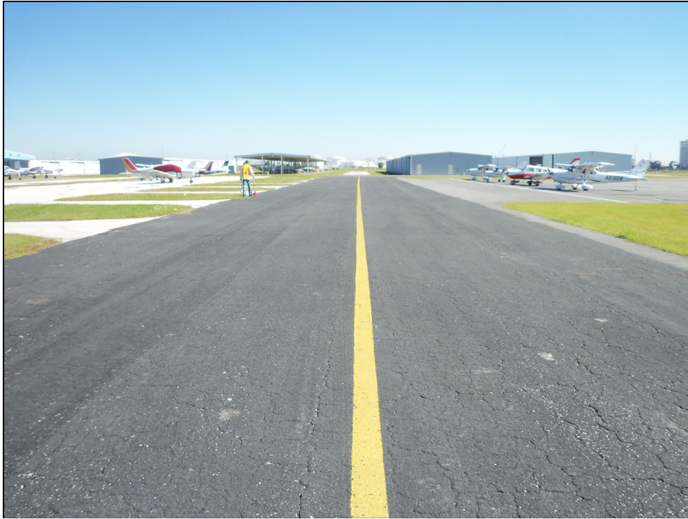
Taxiway B, Section 310, Sample Unit 101 – Low severity (43) Block Cracking, Low severity (52) Weathering and Raveling
