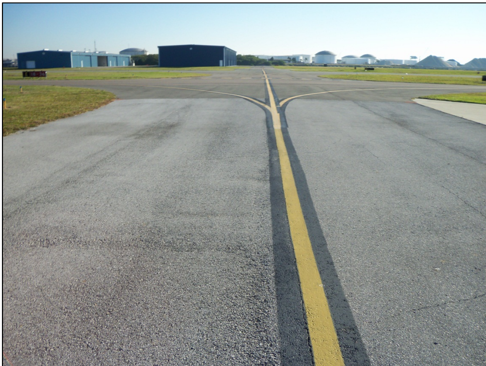
Taxiway E, Section 510, Sample Unit 100 – Low severity (48) Longitudinal and Transverse Cracking, Low severity (52) Weathering and Raveling
