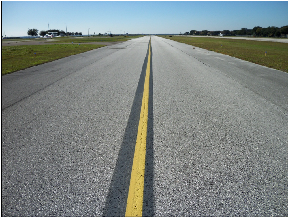
Taxiway A, Section 105, Sample Unit 116 – Low severity (48) Longitudinal and Transverse Cracking, Low and medium severity (52) Weathering and Raveling
