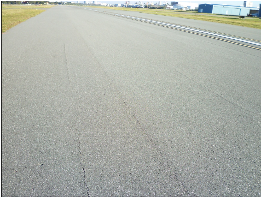
Runway 18-36, Section 6205, Sample Unit 114 – Low severity (48) Longitudinal and Transverse Cracking
