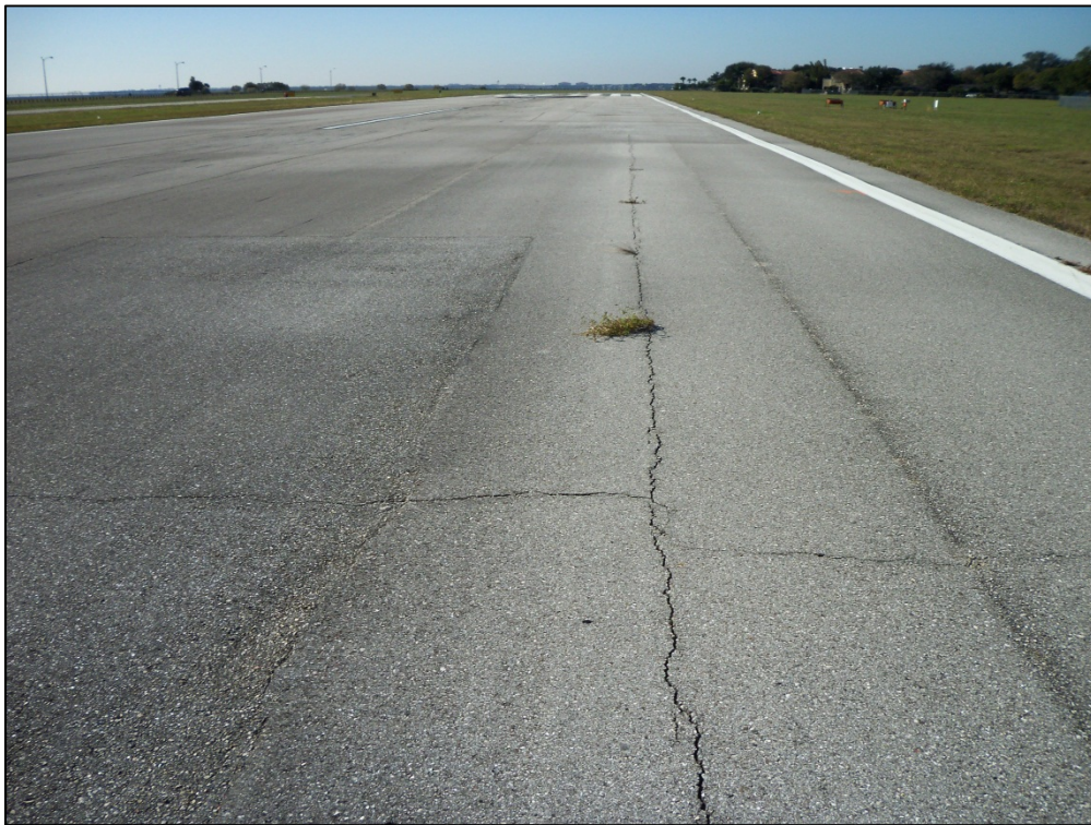
Runway 4-22, Section 6105, Sample Unit 114 – Low and medium severity (48) Longitudinal and Transverse Cracking, Medium severity (50) Patching, Low severity (52) Weathering and Raveling
