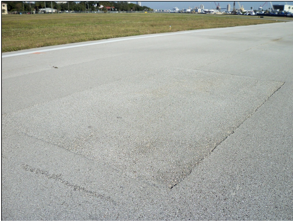
Runway 4-22, Section 6105, Sample Unit 153 – Low severity (48) Longitudinal and Transverse Cracking, Low severity (50) Patching, Low and medium severity (52) Weathering and Raveling
