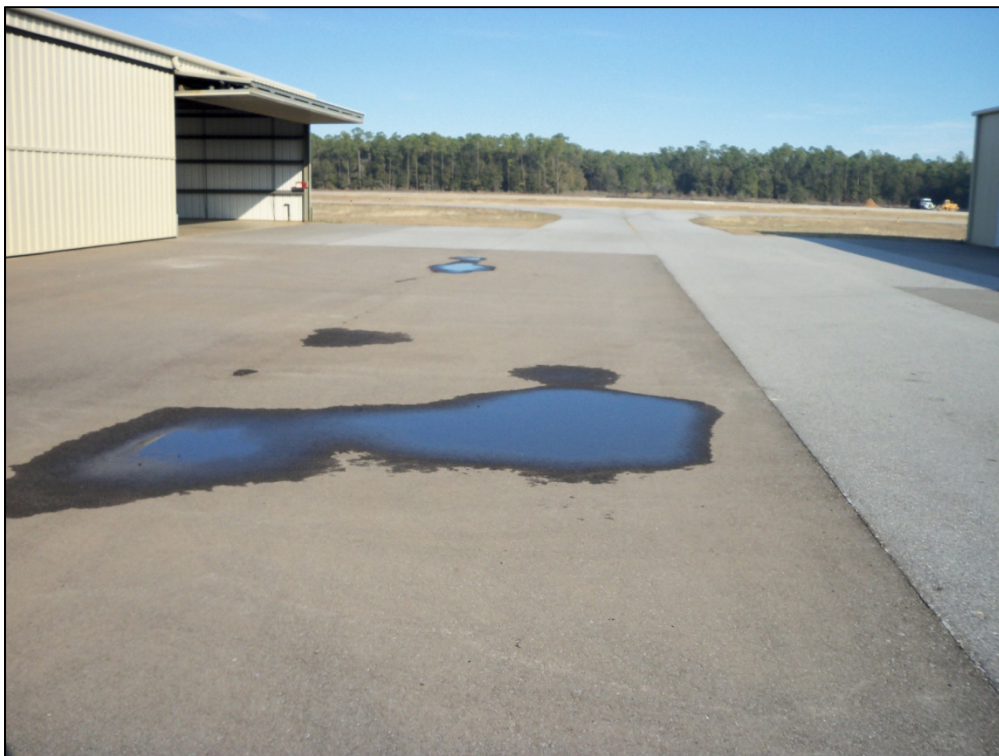
Hangars, Section 4130, Sample Unit 116 – Low severity (48) Longitudinal and Transverse Cracking, low severity (52) Weathering and Raveling
