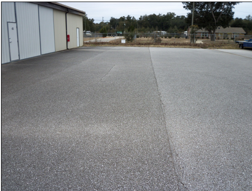
Hangars, Section 4125, Sample Unit 500 – Low severity (48) Longitudinal and Transverse Cracking, low severity (52) Weathering and Raveling
