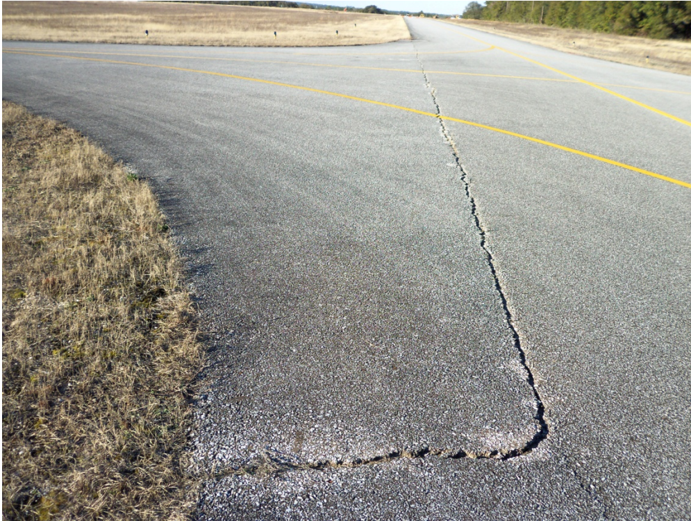
Taxiway B-3, Section 210, Sample Unit 200 – Medium and high severity (48) Longitudinal and Transverse Cracking, low severity (52) Weathering and Raveling
