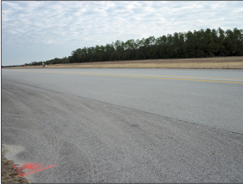
Runway 18-36, Section 6105, Sample Unit 135 – Low severity (48) Longitudinal and Transverse Cracking, low severity (52) Weathering and Raveling
