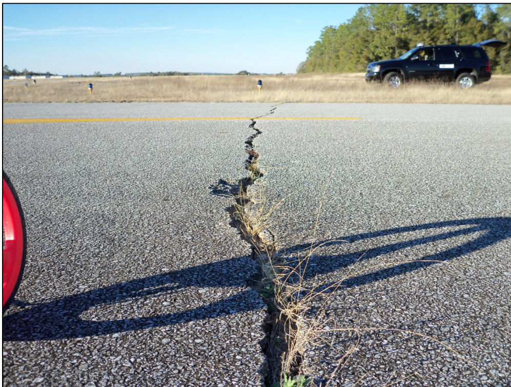
Taxiway Connector, Section 250, Sample Unit 200 – Low, medium and high severity (48) Longitudinal and Transverse Cracking, low severity (52) Weathering and Raveling
