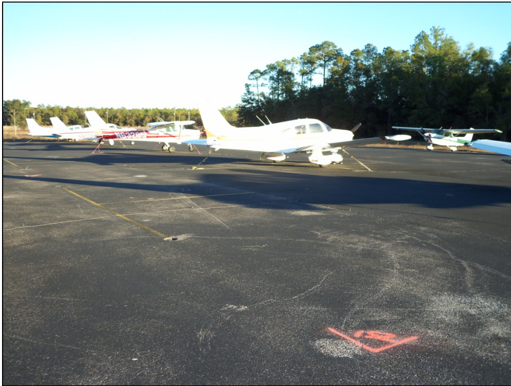
Apron, Section 4205, Sample Unit 251 – Medium severity (43) Block Cracking, high severity (48) Longitudinal and Transverse Cracking, low severity (52) Weathering and Raveling
