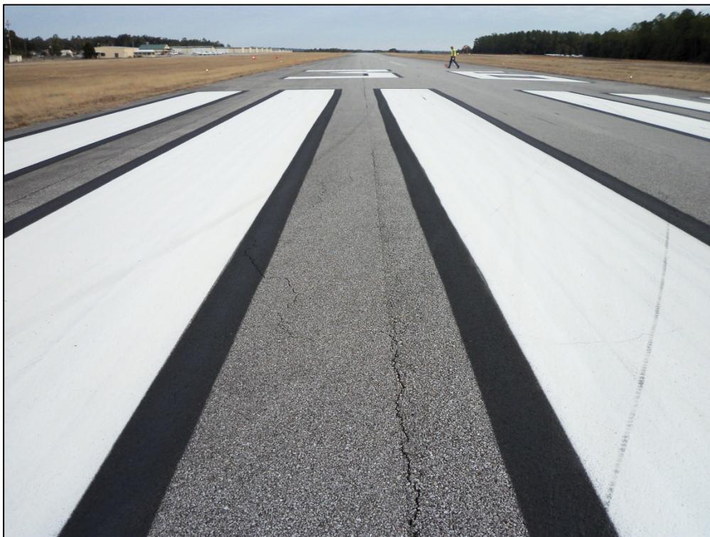
Runway 18-36, Section 6105, Sample Unit 171 – Low and medium severity (48) Longitudinal and Transverse Cracking, low severity (52) Weathering and Raveling
