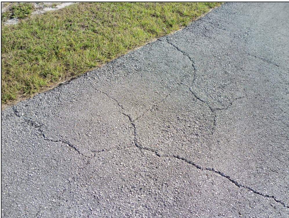
Taxiway Connector Alpha, Section 170, Sample Unit 400 – Low severity (48) Longitudinal and Transverse Cracking, (52) Raveling and Weathering
