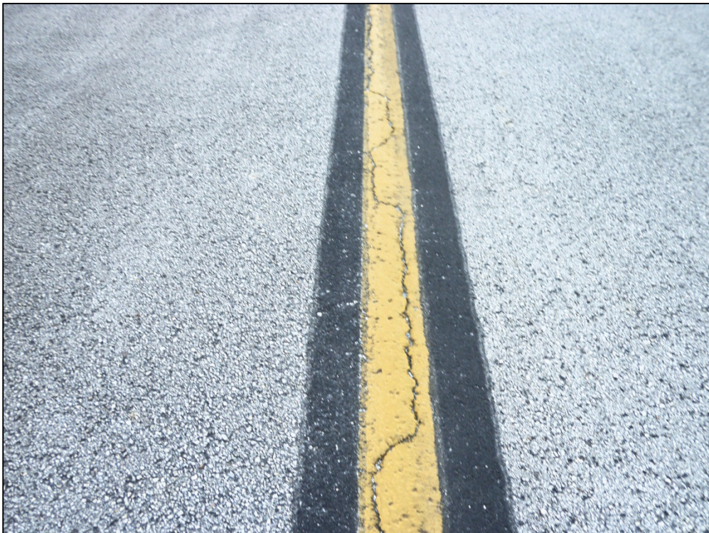
Taxiway T-Hangar, Section 710, Sample Unit 200 – Low severity (48) Longitudinal and Transverse Cracking, (52) Raveling and Weathering
