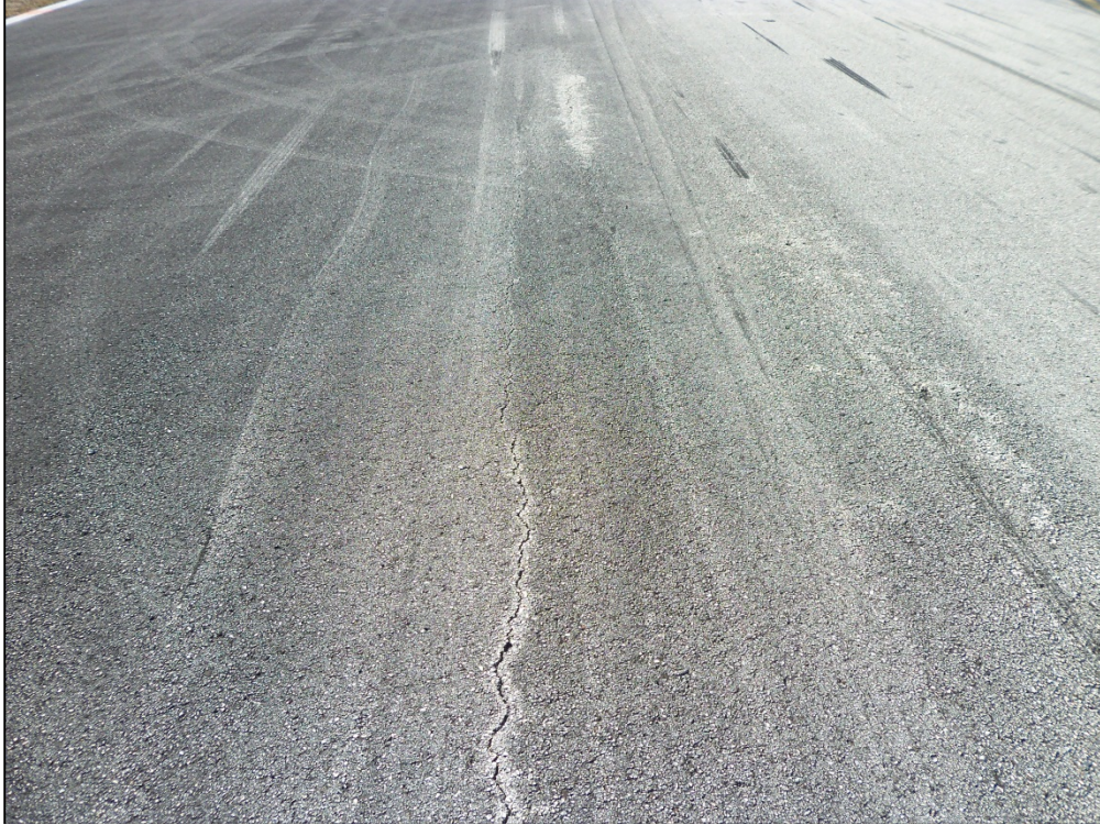
Runway 10-28, Section 6120, Sample Unit 362 – Low severity (48) Longitudinal and Transverse Cracking, (52) Raveling and Weathering
