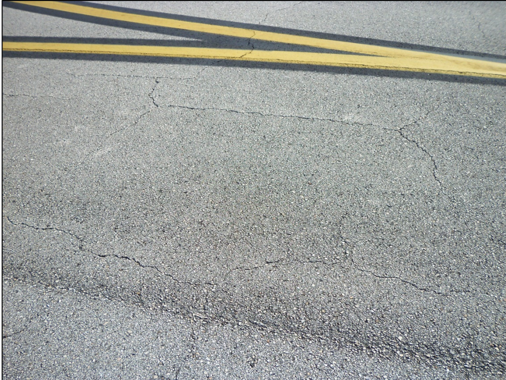
Taxiway Alpha, Section 110, Sample Unit 130 – Low severity (43) Block Cracking, (48) Longitudinal and Transverse Cracking, (52) Raveling and Weathering
