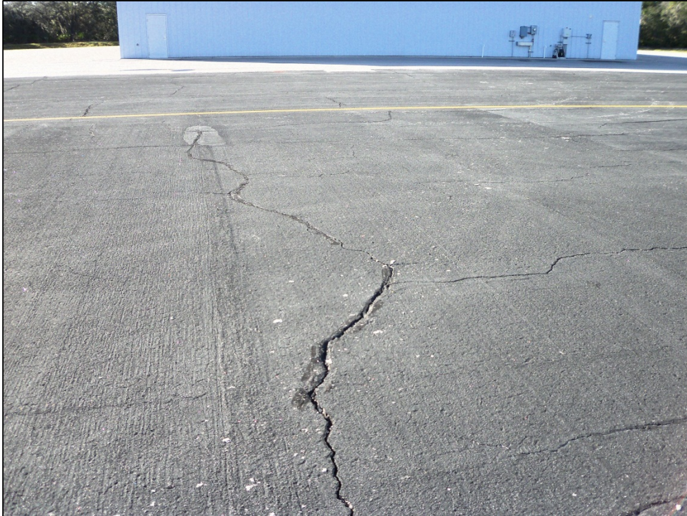
Apron, Section 4105, Sample Unit 300 – Low severity (43) Block Cracking, (52) Raveling and Weathering
