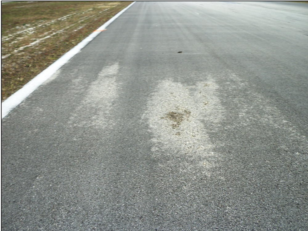
Runway 10-28, Section 6115, Sample Unit 316 – Low severity (52) Raveling and Weathering
