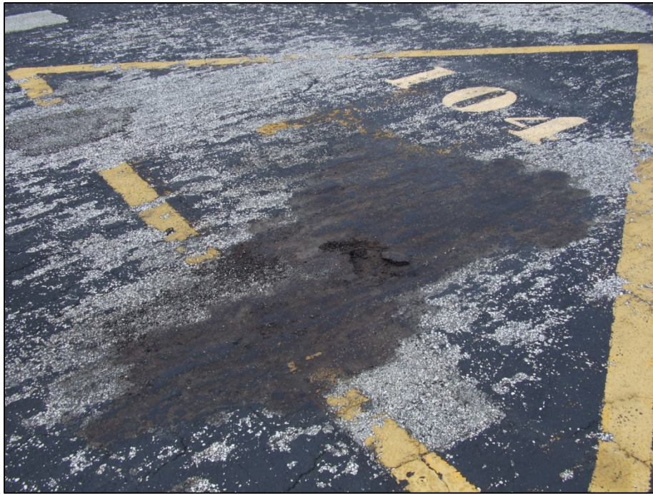
South Apron, Section 4115, Sample Unit 716 – Low severity (48) Longitudinal / Transverse Cracking, (49) Oil Spillage, and low to medium severity (52) Weathering and Raveling.
