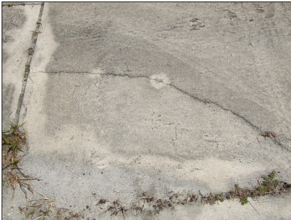
South Apron, Section 4130, Sample Unit 306 – High severity (65) Joint Seal Damage and medium severity (62) Corner Break.
