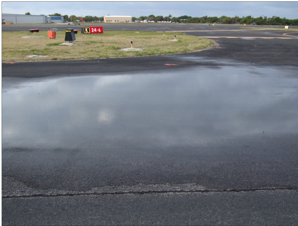
Runway 10-28, Section 6110, Sample Unit 110 – Low to medium severity (45) Depression and low severity (48) Longitudinal / Transverse Cracking.
