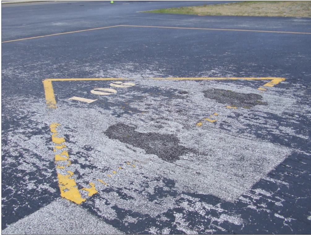
South Apron, Section 4120, Sample Unit 717 – Low to medium severity (50) Patching and low to medium severity (52) Weathering and Raveling.
