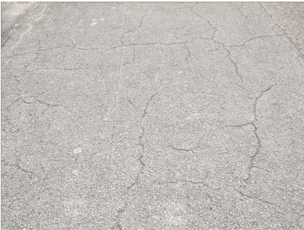
Hangar Apron, Section 4315, Sample Unit 602 –Low severity (48) Block Cracking and low severity (52) Weathering and Raveling.
