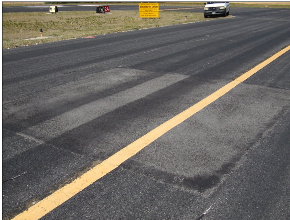
Taxiway Charlie, Section 320, Sample Unit 202 – Low severity (50) Patching and low severity (52) Weathering and Raveling.
