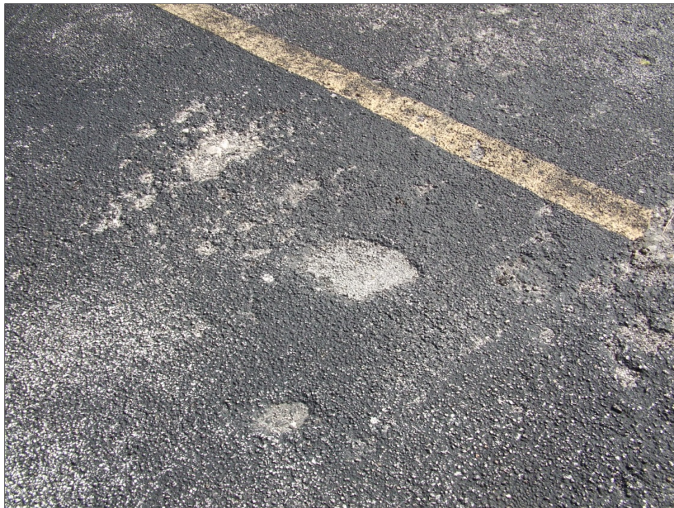
South Apron, Section 4125, Sample Unit 403 – Low to high severity (52) Weathering and Raveling.
