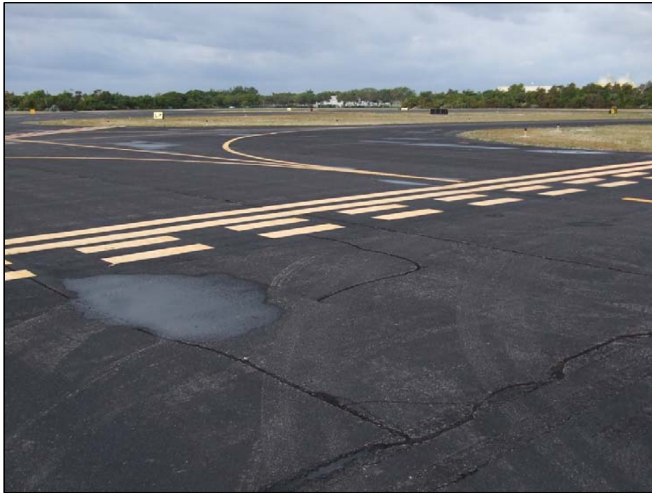
Taxiway Bravo, Section 720, Sample Unit 701 – Low severity (48) Longitudinal / Transverse Cracking and low severity (52) Weathering and Raveling
