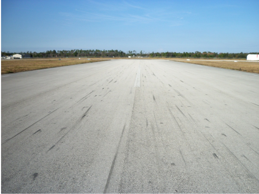
Runway 8-26, Section 6305, Sample Unit 504 – Low severity (48) Longitudinal and Transverse Cracking, low severity (52) Weathering and Raveling
