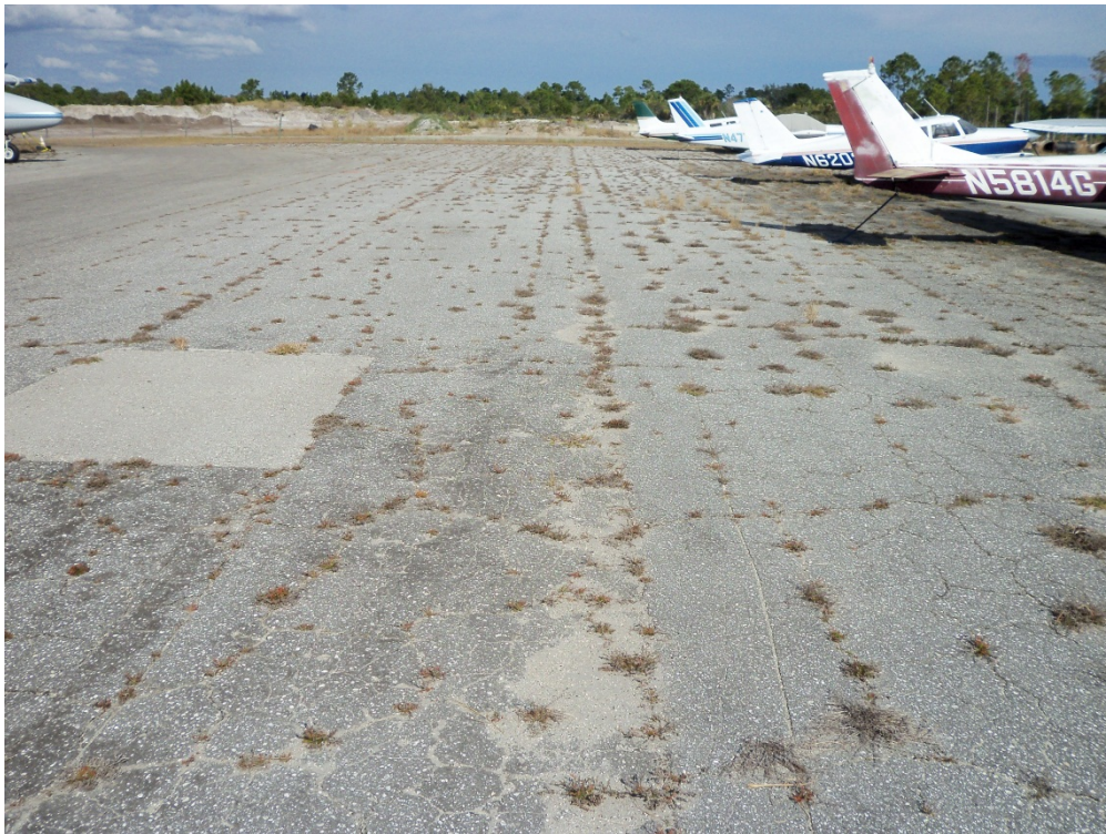
West Apron, Section 410, Sample Unit 435 – Medium severity (43) Block Cracking, low severity (52) Weathering and Raveling, low severity (50) patching
