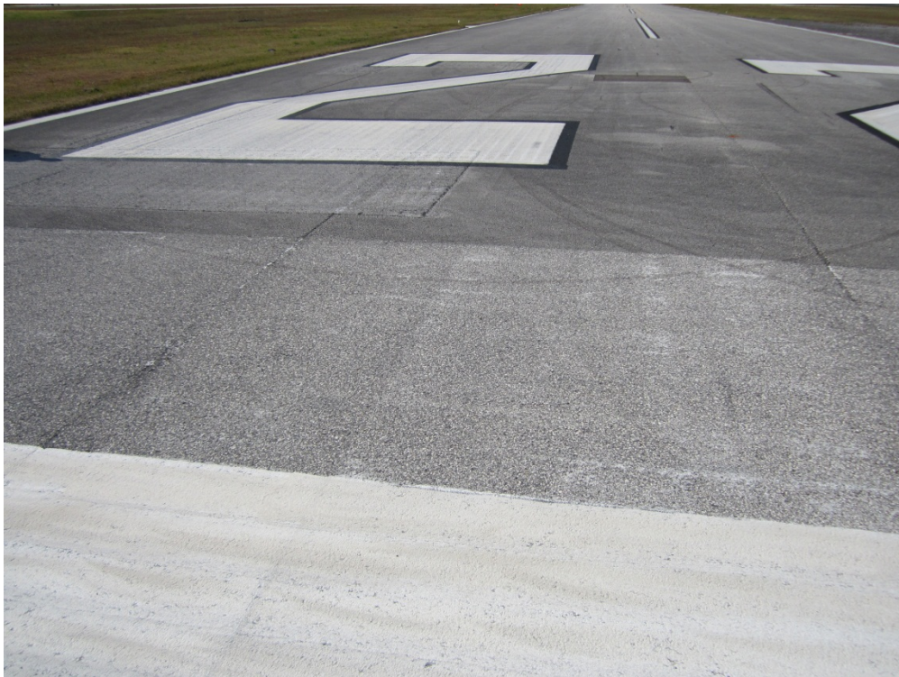
Runway 4-22, Section 6205, Sample Unit 379 – Low and medium severity (52) Weathering and Raveling, low severity (50) patching, low severity (48) Longitudinal and Transverse Cracking
