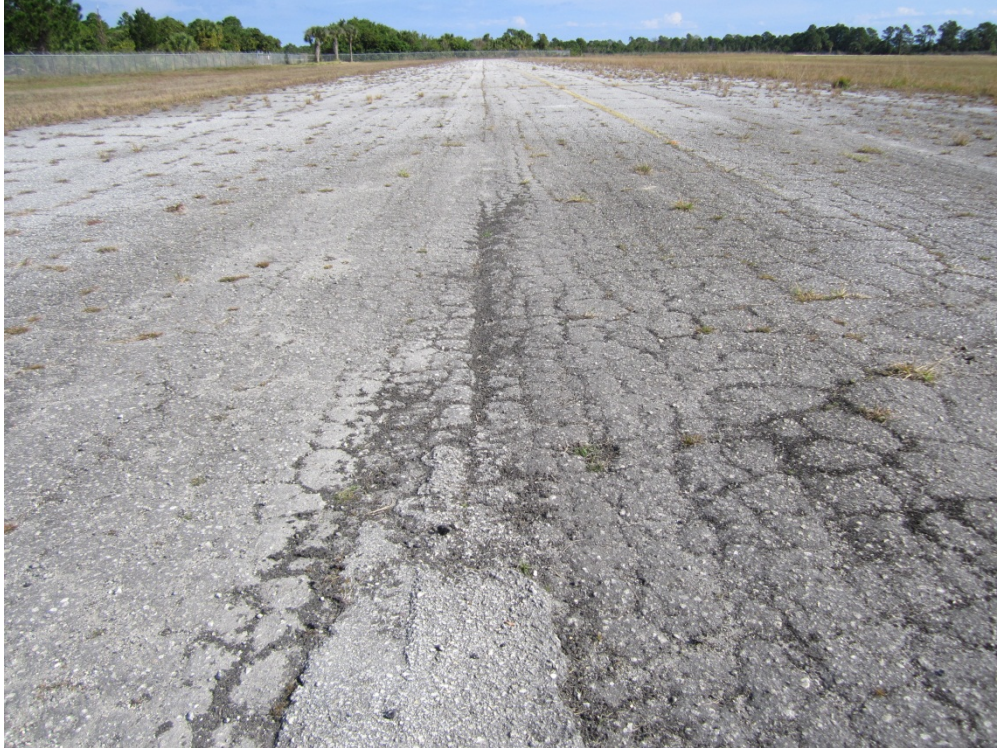
Taxiway C, Section 305, Sample Unit 300 – Medium severity (52) Weathering and Raveling, medium severity (41) Alligator Cracking, medium severity (43) Block Cracking
