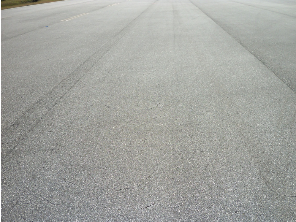
West Apron, Section 5105, Sample Unit 431 – Low severity (48) Longitudinal and Transverse Cracking
