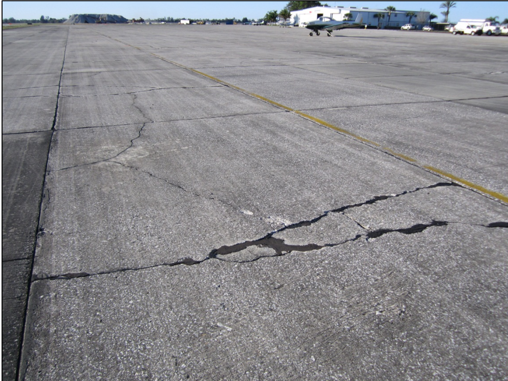
West Apron, Section 4105, Sample Unit 114 – Low severity (65) Joint Seal Damage; high severity (72) Shattered Slab
