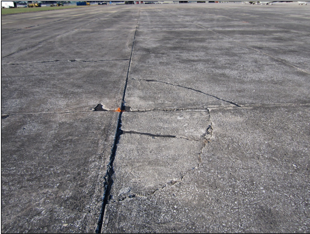
West Apron, Section 4105, Sample Unit 206 – Low severity (65) Joint Seal Damage; high severity (63) Longitudinal, Transverse, and Diagonal Cracking; medium and high severity (62) Corner Break; low severity (74) Joint Spalling
