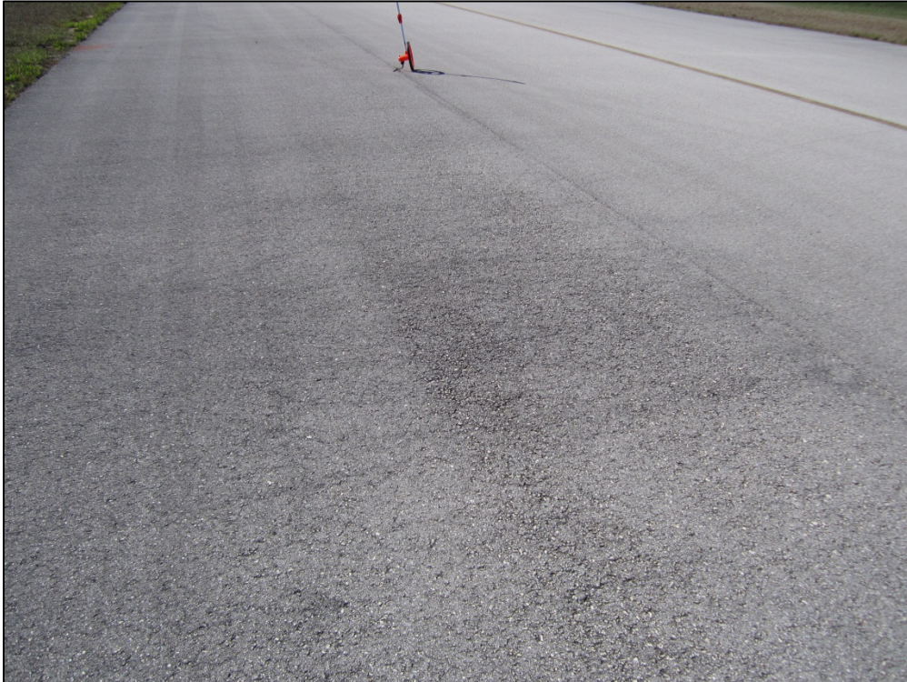
Taxiway Alpha, Section 420, Sample Unit 250 – Low severity (52) Weathering and Raveling
