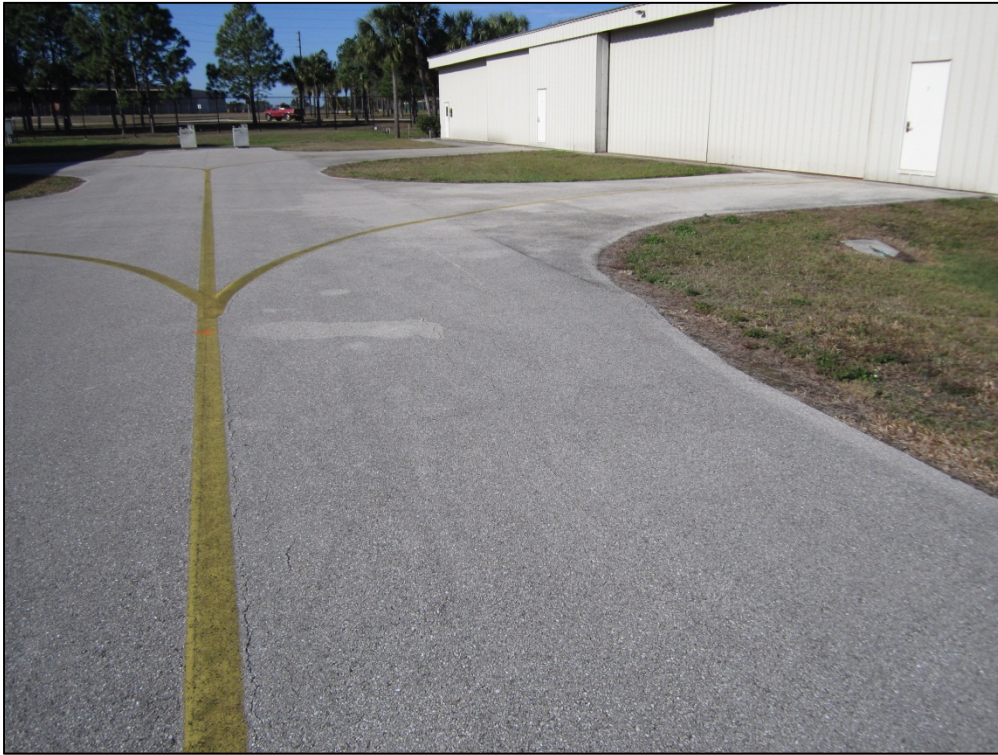
T-Hangars Taxiway, Section 505, Sample Unit 302 – Low severity (48) Longitudinal and Transverse Cracking, low severity (52) Weathering and Raveling, low severity (56) Swelling
