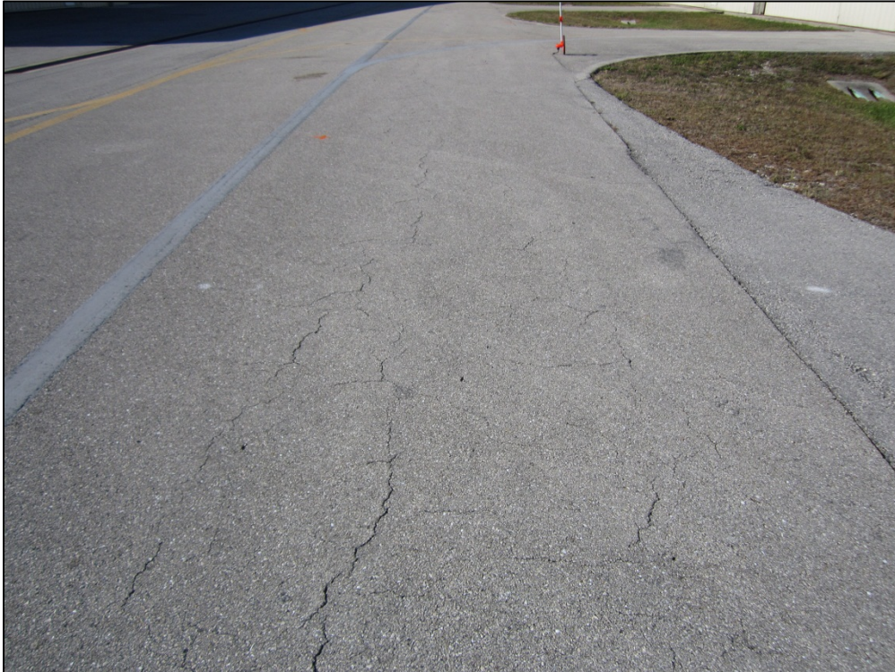
T-Hangars Taxiway, Section 505, Sample Unit 100 – Low severity (48) Longitudinal and Transverse Cracking, low severity (43) Block Cracking, low severity (56) Swelling
