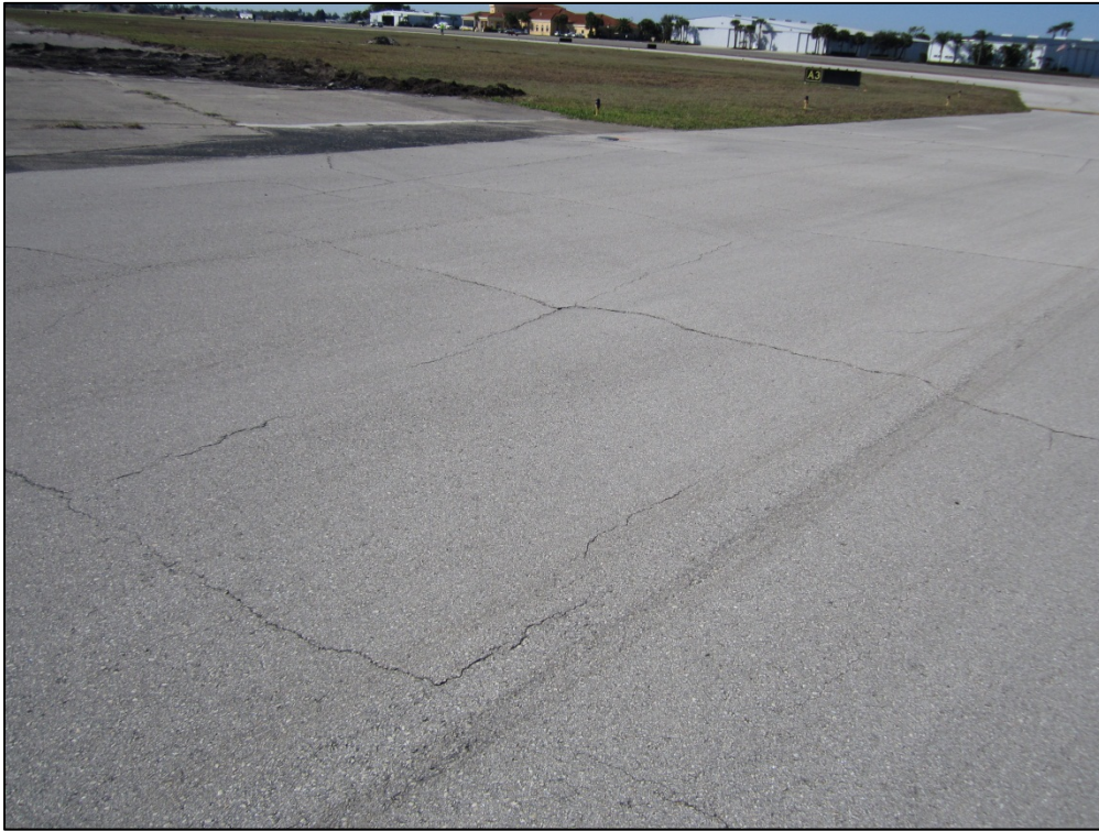
Taxiway A-3, Section 205, Sample Unit 101 – Low severity (48) Longitudinal and Transverse Cracking, low severity (52) Weathering and Raveling
