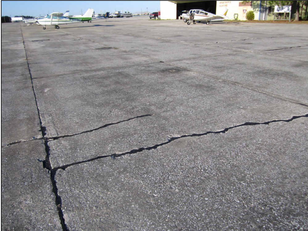
West Apron, Section 4105, Sample Unit 505 – Low severity (65) Joint Seal Damage; high severity (63) Longitudinal, Transverse, and Diagonal Cracking; (73) Shrinkage Cracking
