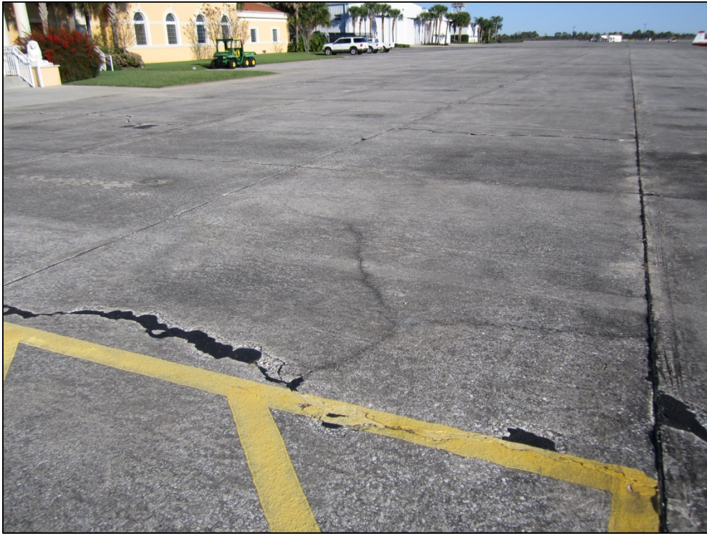
West Apron, Section 4105, Sample Unit 414 – Low severity (65) Joint Seal Damage; high severity (63) Longitudinal, Transverse, and Diagonal Cracking; low severity (75) Corner Spalling
