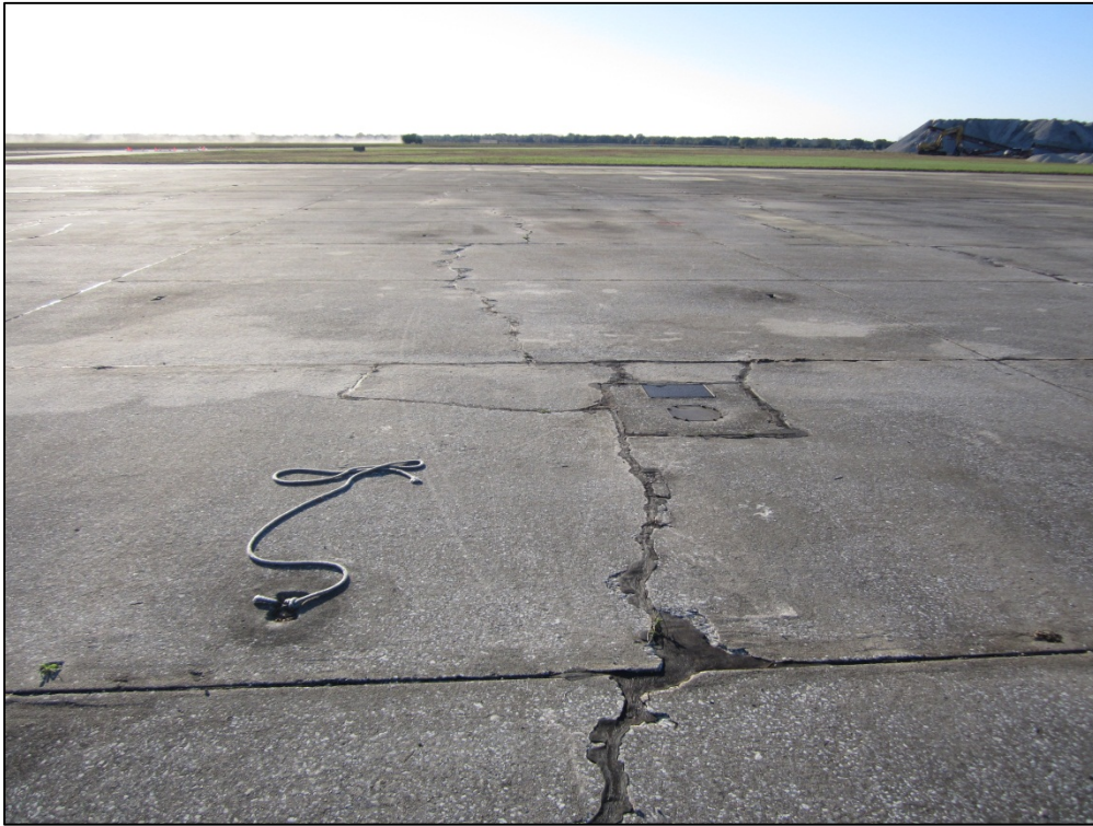
West Apron, Section 4105, Sample Unit 505 – Low severity (65) Joint Seal Damage; high severity (63) Longitudinal, Transverse, and Diagonal Cracking
