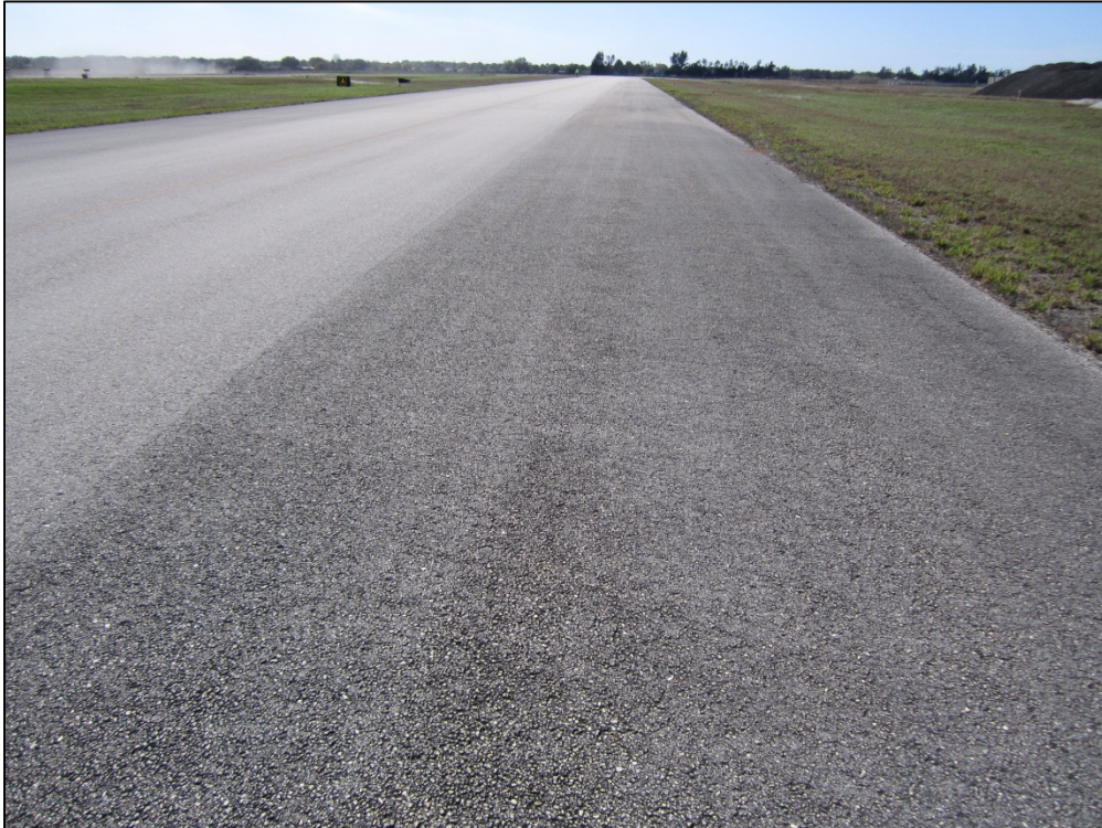
Taxiway Alpha, Section 405, Sample Unit 214 – Low severity (52) Weathering and Raveling
