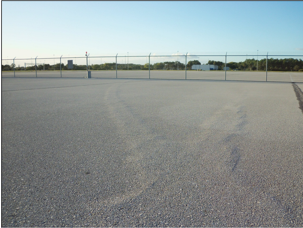
North Apron, Section 4310, Sample Unit 707 – Low severity (52) Weathering and Raveling, low severity (56) Swelling
