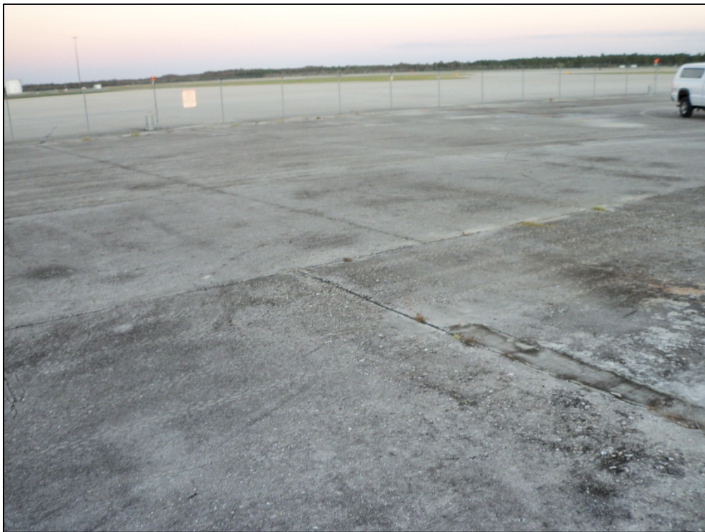
North Apron, Section 4320, Sample Unit 404 – Low severity (66) Patching, low severity (74) Joint Spalling
