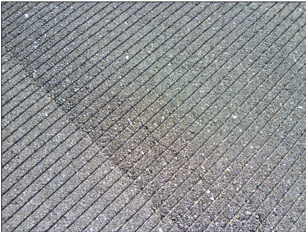
Runway 6-24, Section 6105, Sample Unit 627 – Low Severity (48) Longitudinal and Transverse Cracking
