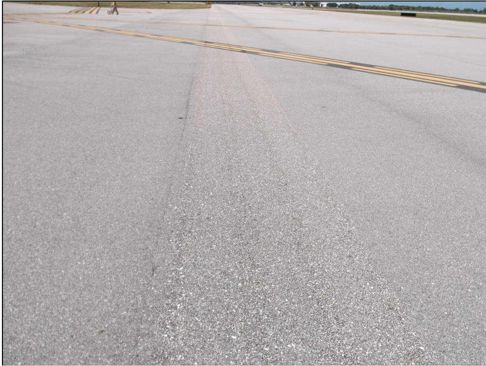
Taxiway A-8, Section 815, Sample Unit 806 – Low Severity (52) Weathering and Raveling
