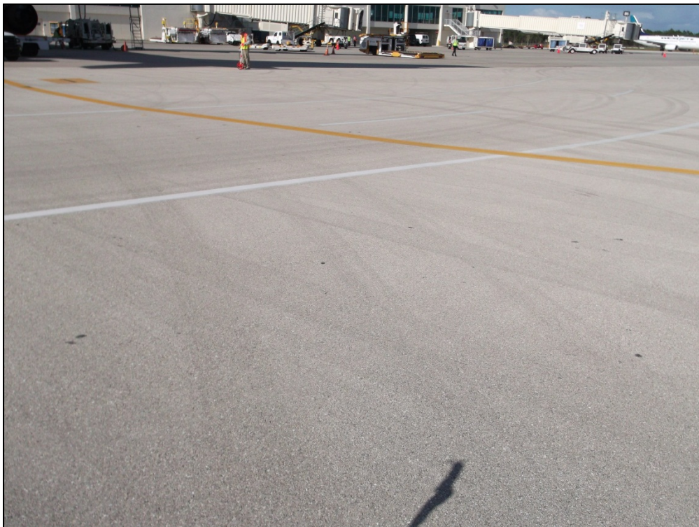
South Apron, Section 4425, Sample Unit 203 – No distresses
