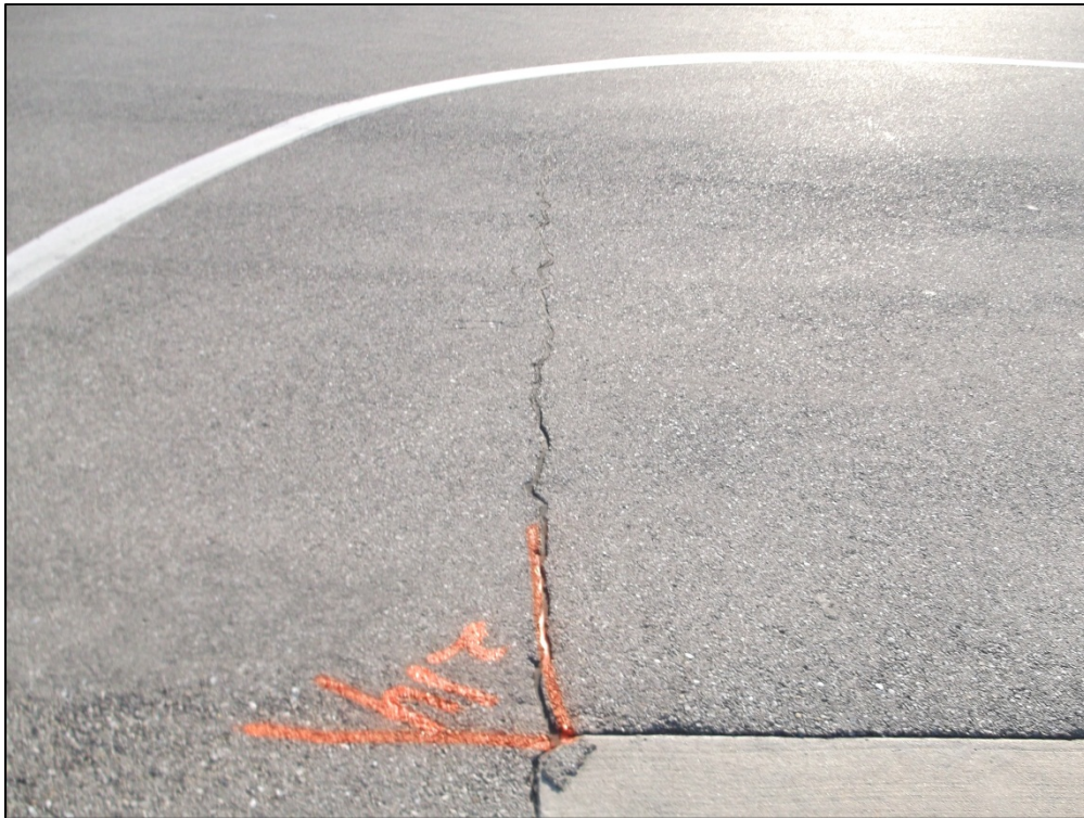
South Apron, Section 4415, Sample Unit 214 – Low Severity (48) Longitudinal and Transverse Cracking
