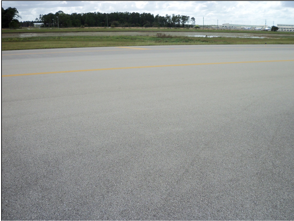
Taxiway Foxtrot, Section 260, Sample Unit 246 – No distresses
