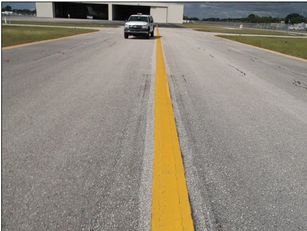
Taxiway A-5, Section 555, Sample Unit 504 – Low Severity (48) Longitudinal and Transverse Cracking and low severity (52) Weathering and Raveling
