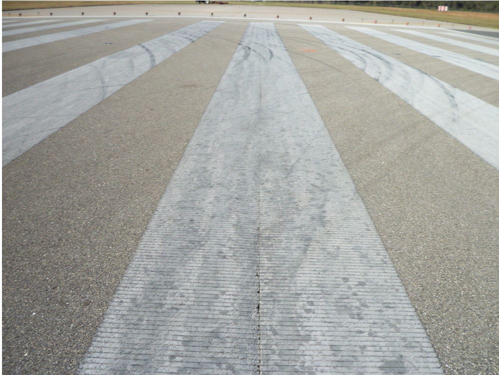
Runway 6-24, Section 6104, Sample Unit 481 – Low severity (48) Longitudinal and Transverse Cracking
