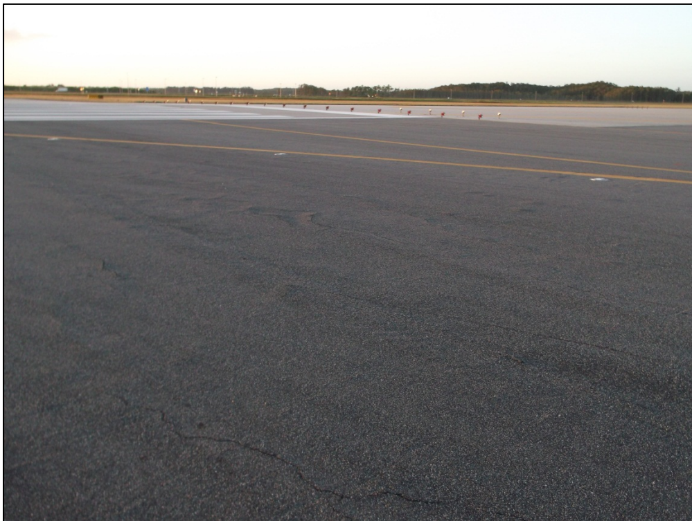
Taxiway Connector A-1, Section 103, Sample Unit 101 – Low Severity (48) Longitudinal and Transverse Cracking and low severity (56) Swelling
