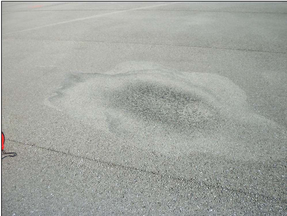
North Apron, Section 4330, Sample Unit 202 – Low Severity (46) Jet Blast Erosion
