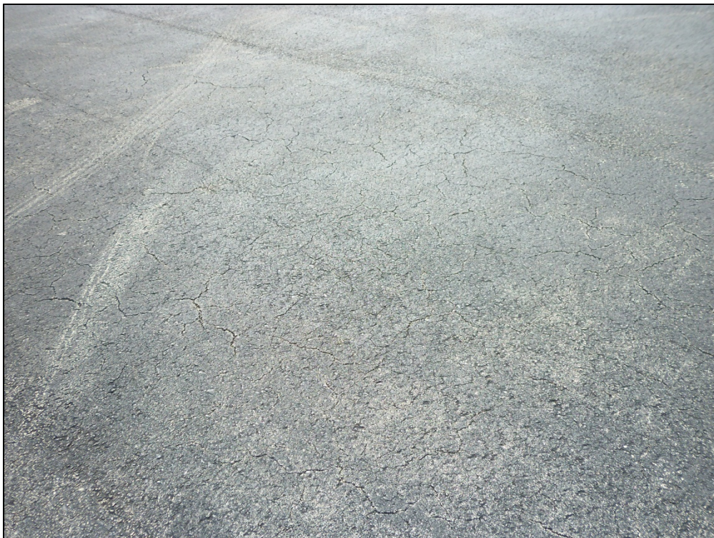
FBO Apron, Section 4205, Sample Unit 551 – Low Severity (43) Block Cracking
