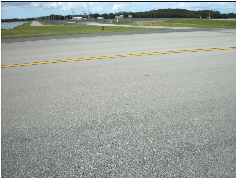
Taxiway A-3, Section 305, Sample Unit 309 – Low severity (48) Longitudinal and Transverse Cracking
