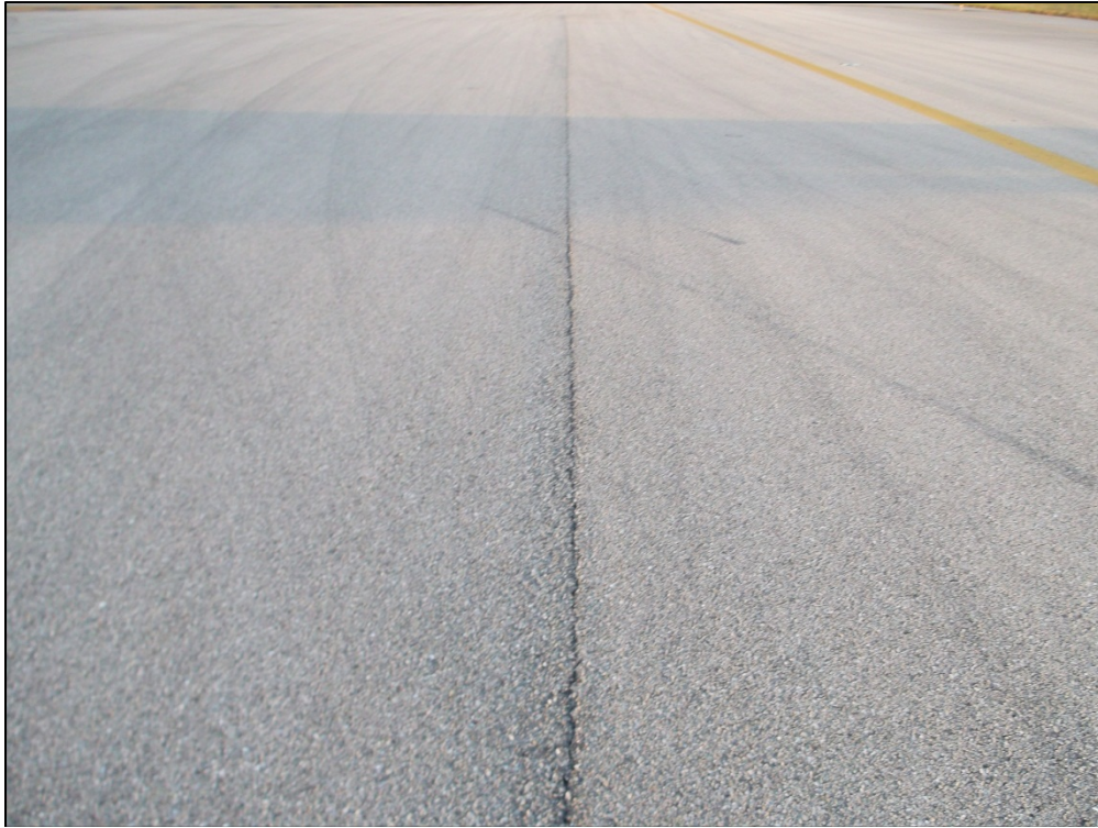
Taxiway Connector F-3, Section 520, Sample Unit 503 – Low Severity (48) Longitudinal and Transverse Cracking
