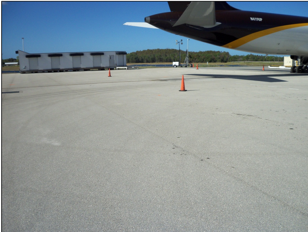
Cargo Apron, Section 4105, Sample Unit 301 – (49) Oil Spillage and Low Severity (52) Weathering and Raveling
