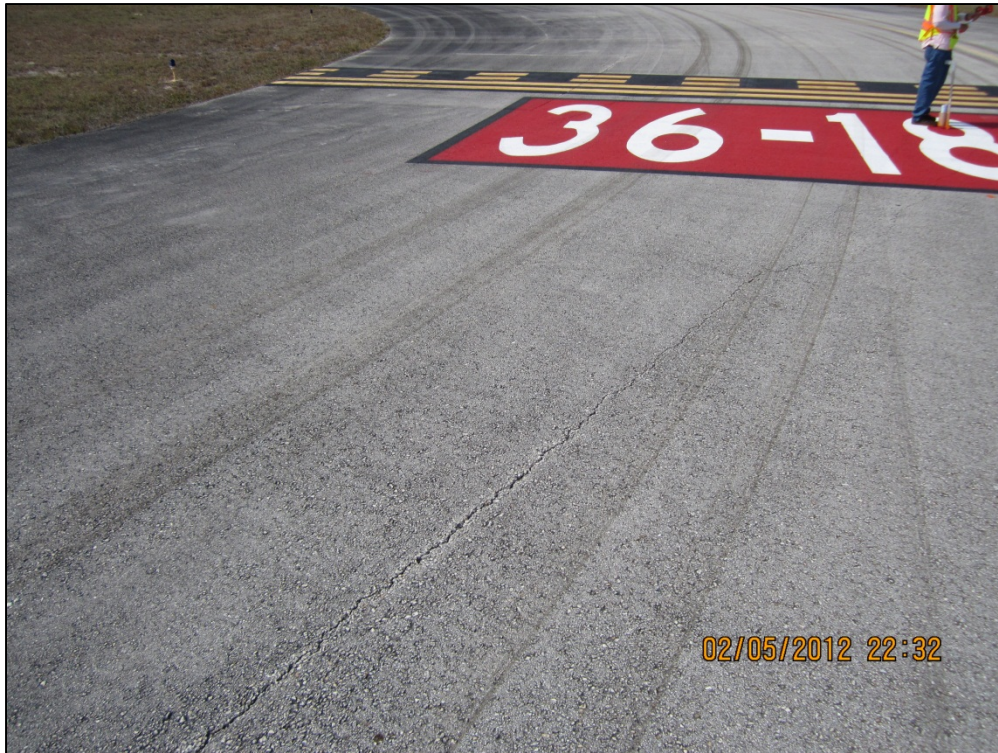
Taxiway Alpha, Section 120, Sample Unit 162 – Low severity (52) Weathering and Raveling, low severity (48) Longitudinal and Transverse Cracking
