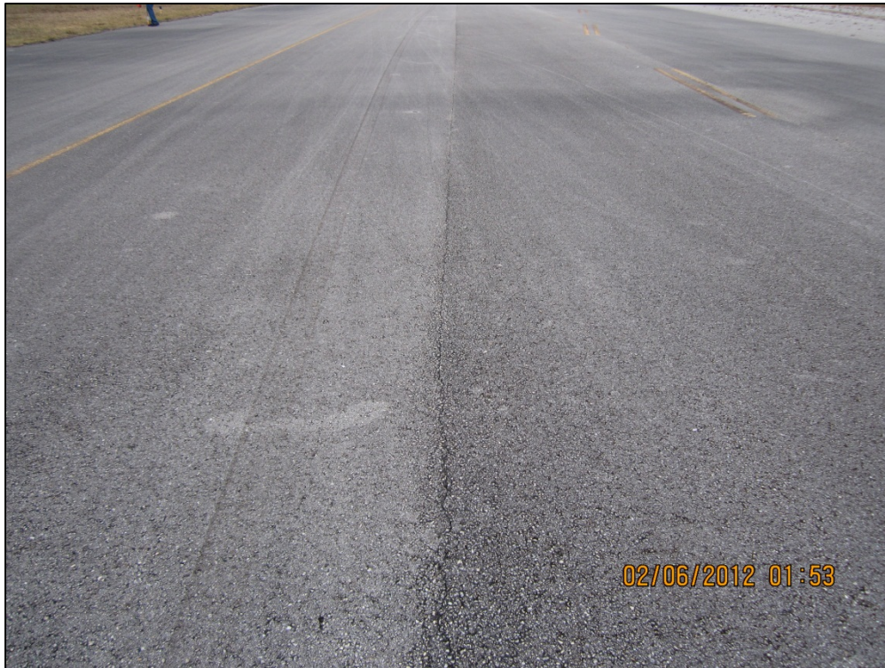
Taxiway Delta, Section 404, Sample Unit 402 – Low severity (48) Longitudinal and Transverse Cracking
