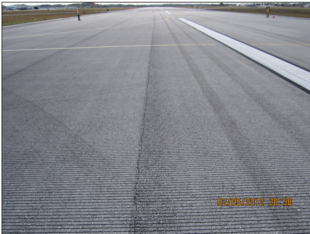
Runway 18-36, Section 6125, Sample Unit 368 – Low severity (48) Longitudinal and Transverse Cracking, low severity (52) Weathering and Raveling
