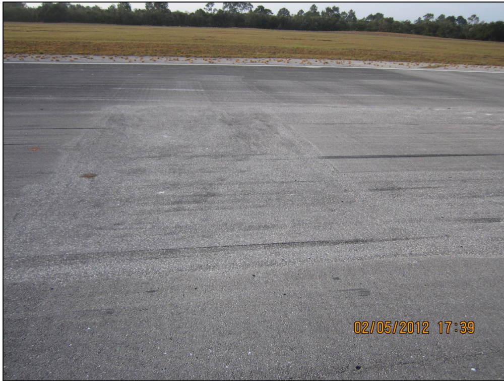
Runway 9-27, Section 6210, Sample Unit 190 – Low severity (52) Weathering and Raveling, low severity (48) Longitudinal and Transverse Cracking
