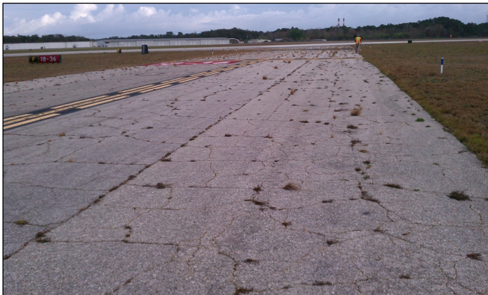
Taxiway Foxtrot, Section 605, Sample Unit 304 – Medium severity (43) Block Cracking, low severity (52) Weathering and Raveling
