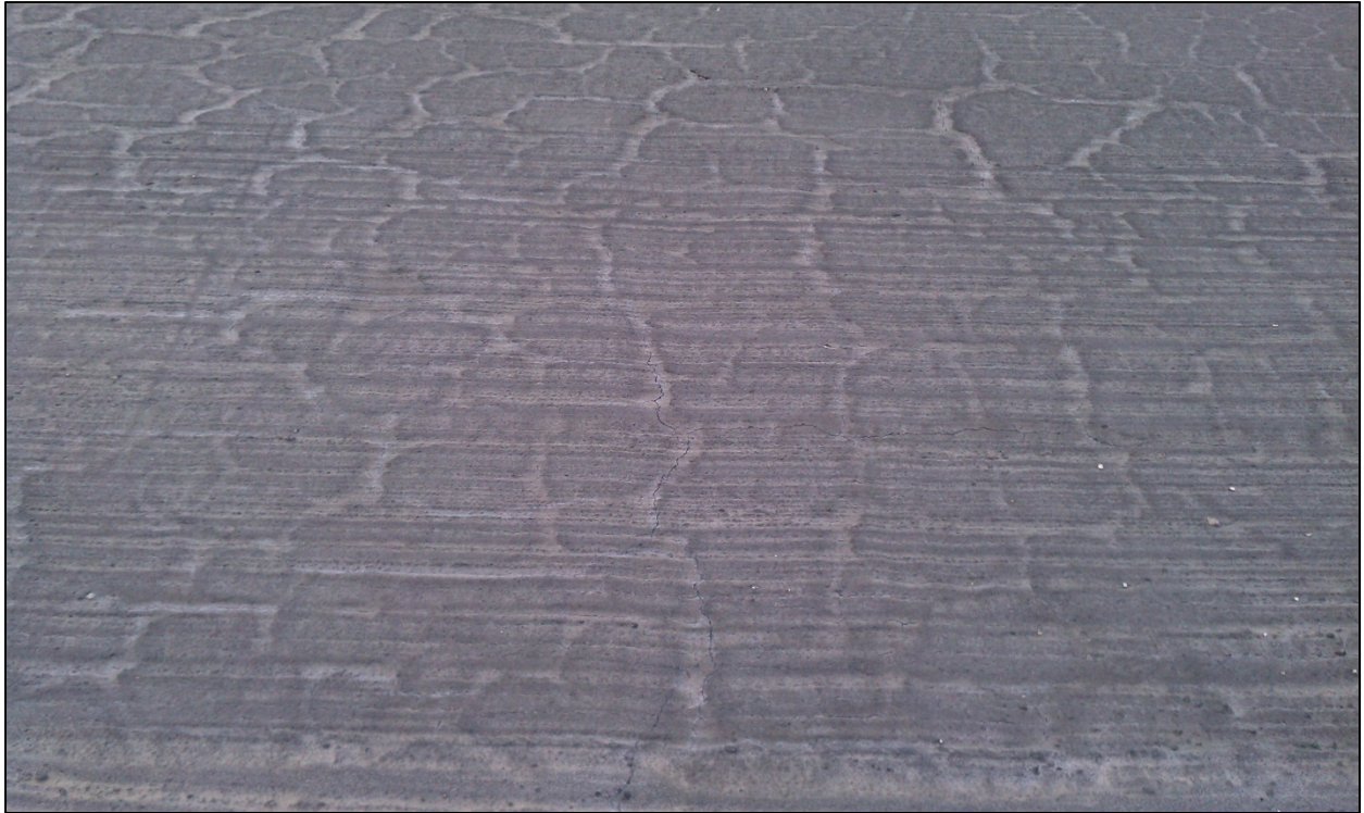
South Apron, Section 4215, Sample Unit 663 – Low severity (48) Longitudinal and Transverse Cracking
