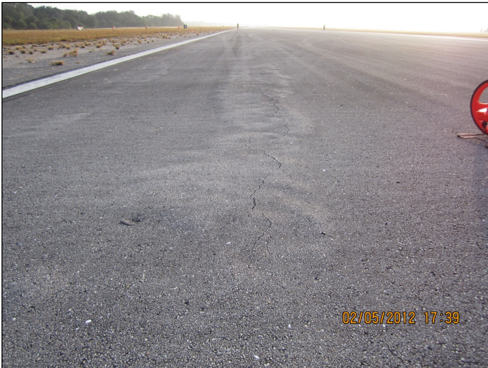
Runway 9-27, Section 6210, Sample Unit 190 – Low severity (48) Longitudinal and Transverse Cracking, low severity (52) Weathering and Raveling, low severity (56) Swelling
