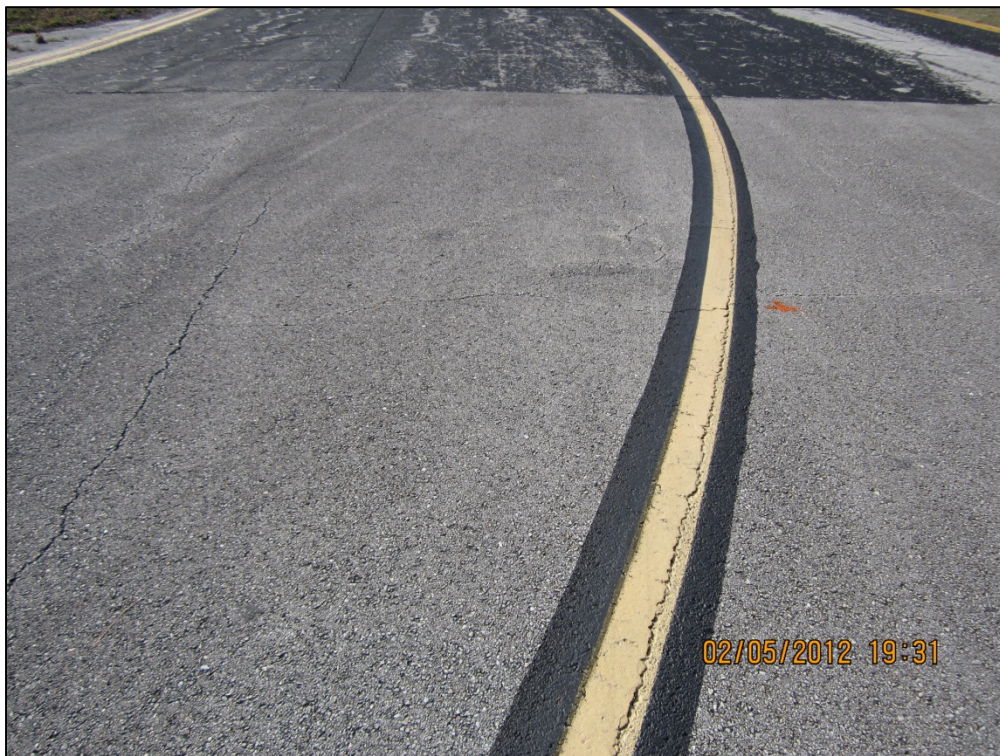
Taxiway Bravo, Section 220, Sample Unit 500 – Low severity (48) Longitudinal and Transverse Cracking, low severity (52) Weathering and Raveling, low severity (56) Swelling
