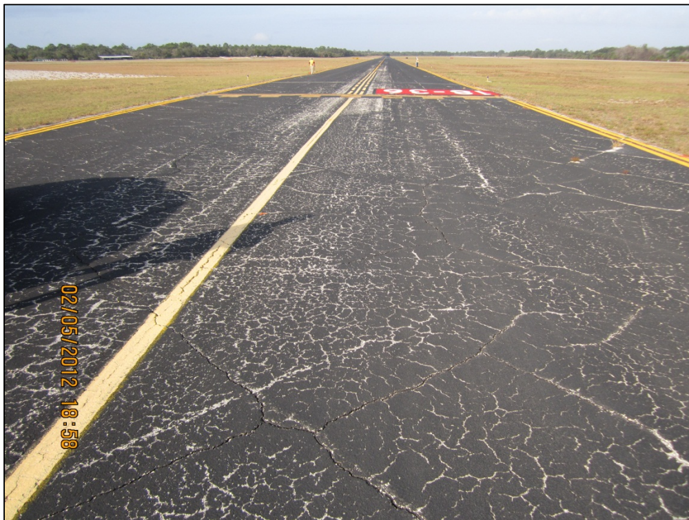
Taxiway Bravo, Section 210, Sample Unit 545 – Medium severity (43) Block Cracking, medium severity (52) Weathering and Raveling
