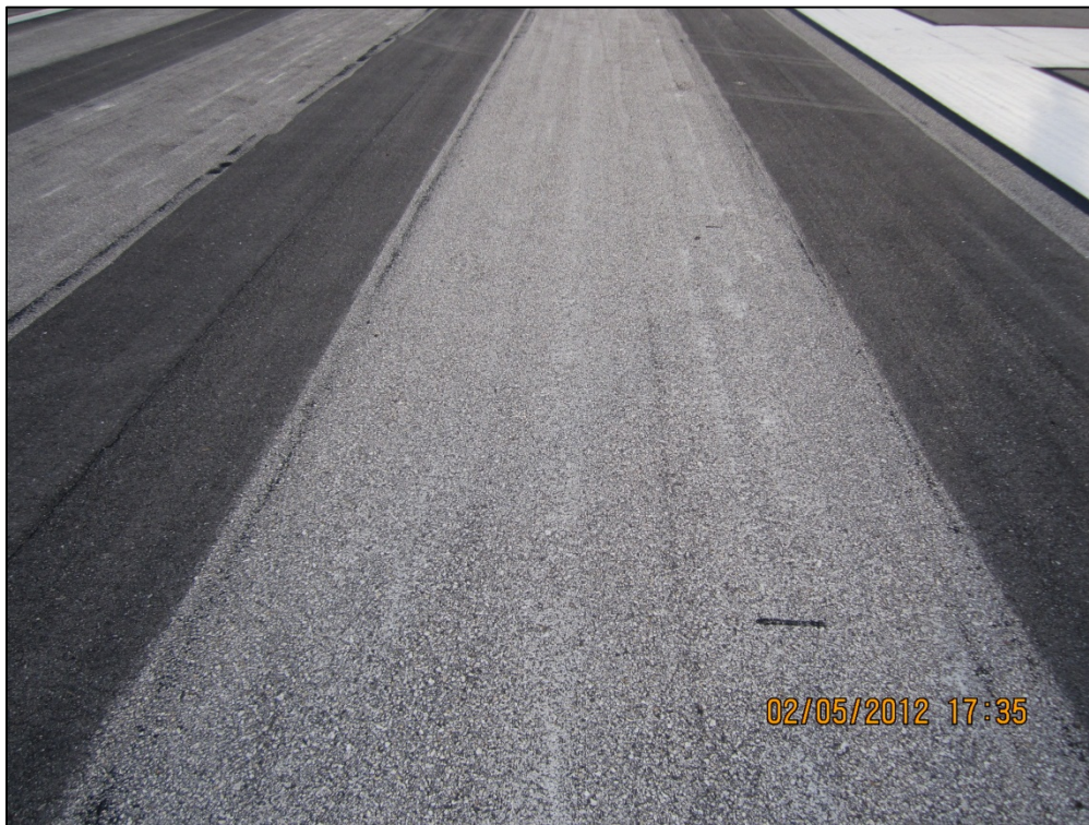
Runway 9-27, Section 6210, Sample Unit 194 – Low severity (48) Longitudinal and Transverse Cracking, low severity (52) Weathering and Raveling
