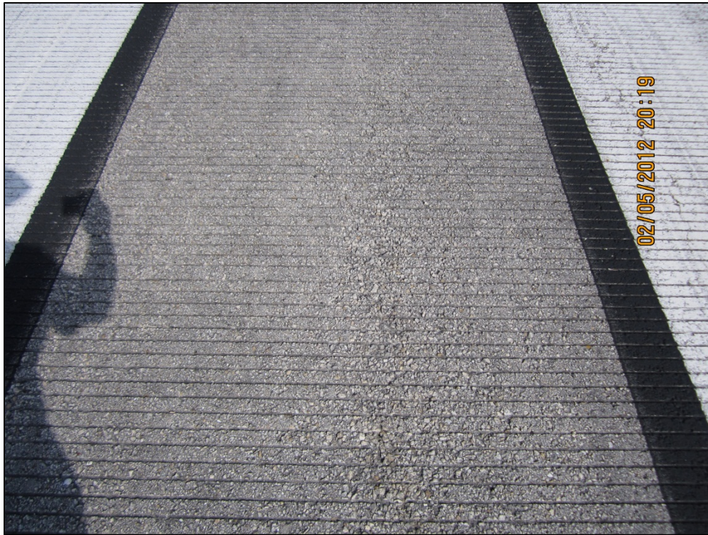
Runway 18-36, Section 6145, Sample Unit 437 – Low severity (52) Weathering and Raveling
