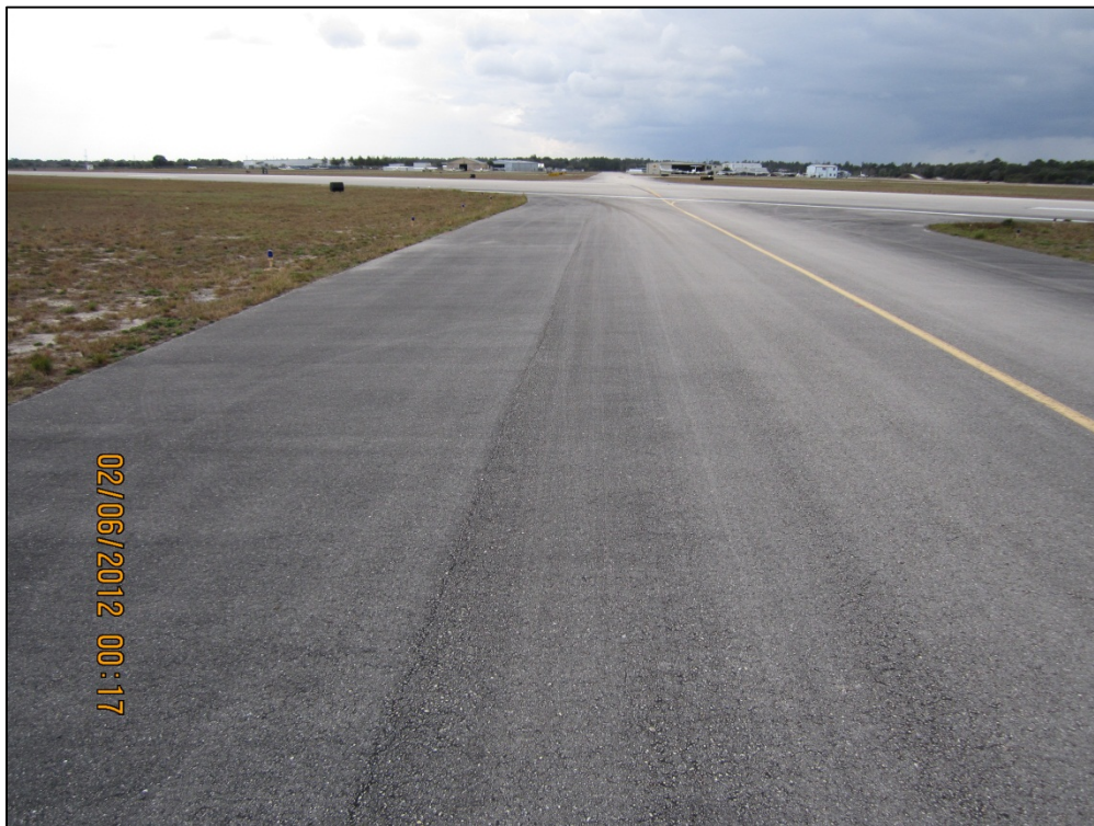
Taxiway Echo, Section 505, Sample Unit 601 – Low severity (48) Longitudinal and Transverse Cracking
