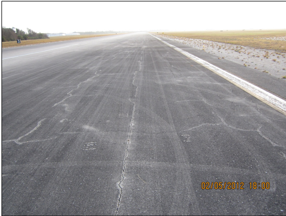
Runway 9-27, Section 6210, Sample Unit 165 – Low severity (43) Block Cracking, low severity (48) Longitudinal and Transverse Cracking, low severity (52) Weathering and Raveling
