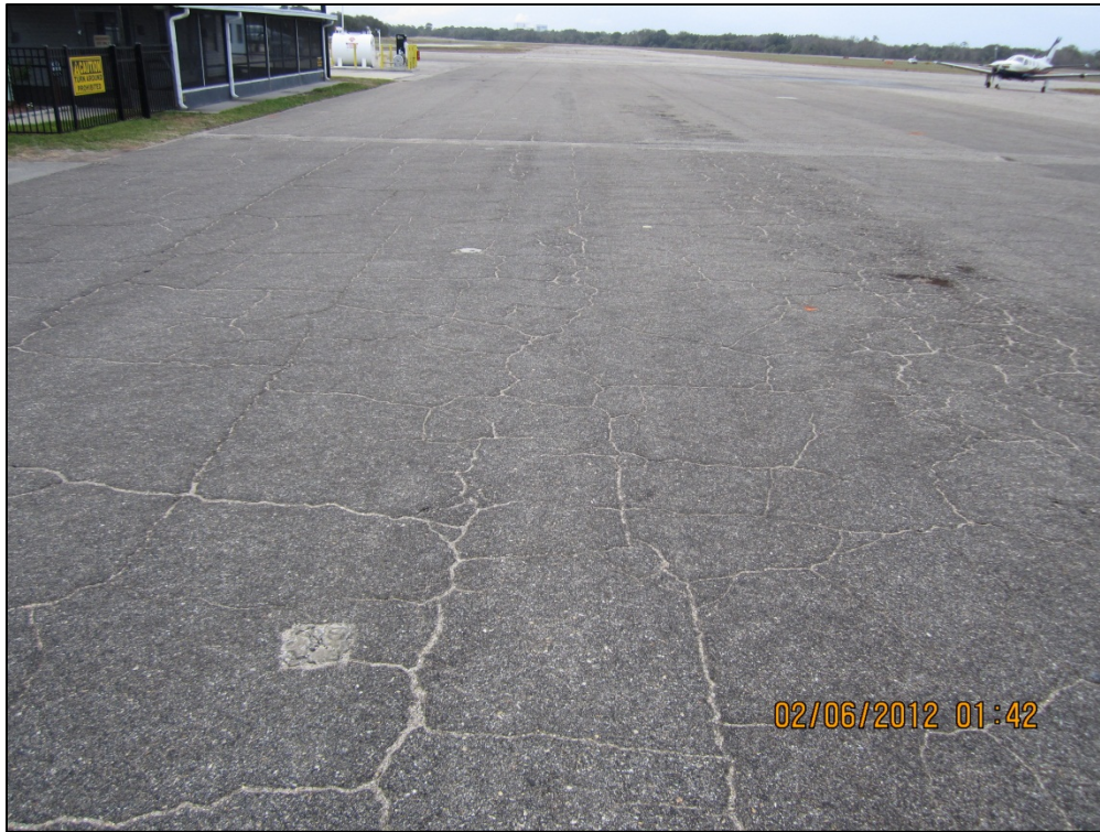
Taxiway Foxtrot, Section 610, Sample Unit 101 – Medium severity (50) Patching, medium severity (52) Weathering and Raveling, medium severity (43) Block Cracking
