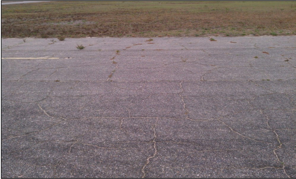
Taxiway Foxtrot, Section 620, Sample Unit 304 – Medium severity (43) Block Cracking, low severity (52) Weathering and Raveling
