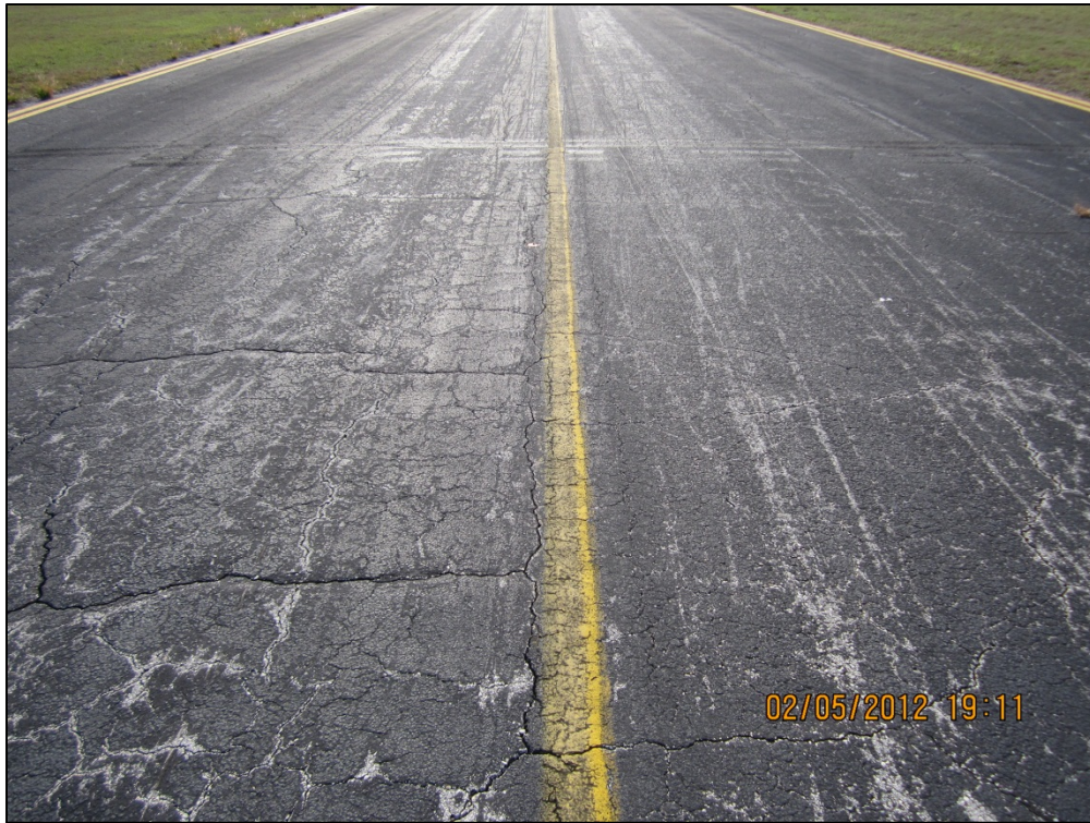
Taxiway Charlie, Section 315, Sample Unit 701 – Low severity (43) Block Cracking, medium severity (52) Weathering and Raveling
