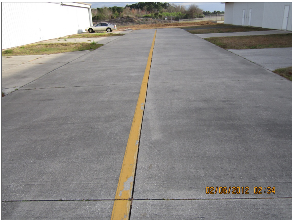
T-Hangar Taxiway, Section 4225, Sample Unit 201 – Low severity (65) Joint Seal Damage
