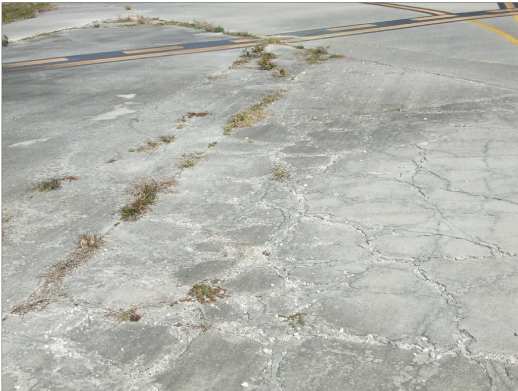
Center Apron, Section 4112, Sample Unit 400 – High severity (65) Joint Seal Damage and high severity (72) Shattered Slab.
