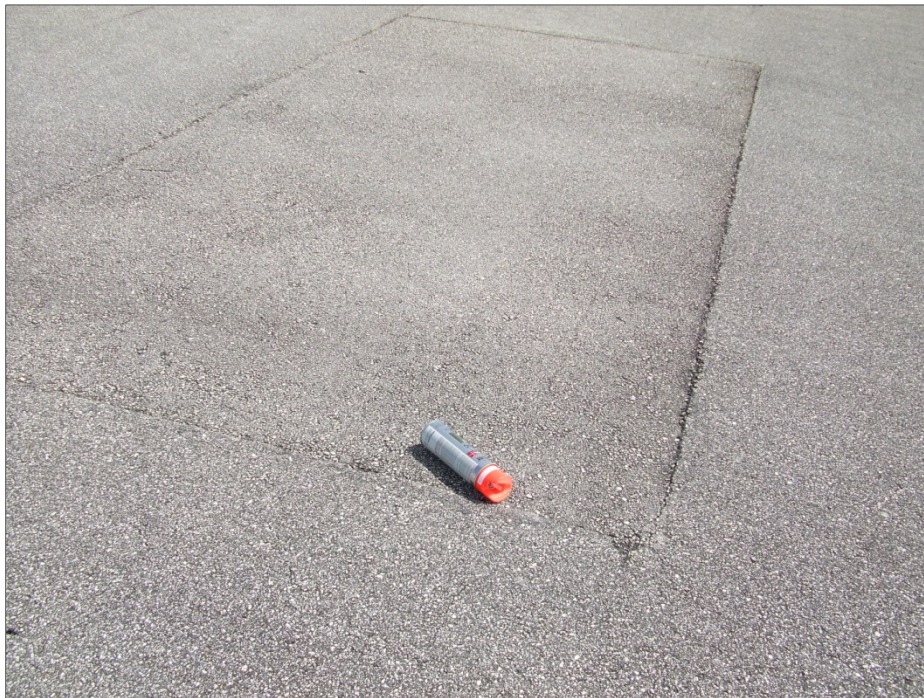
Runway 14-32, Section 6205, Sample Unit 177 – Low severity (50) Patching.
