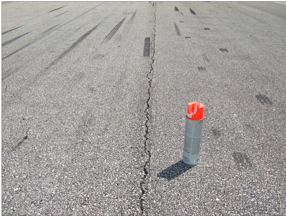
Runway 14-32, Section 6205, Sample Unit 114 – Low severity (48) Longitudinal and Transverse Cracking and low severity (52) Weathering and Raveling.
