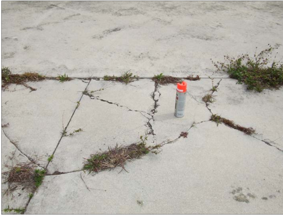
Southeast Apron, Section 4305, Sample Unit 603 – High severity (62) Corner Break and high severity (65) Joint Seal Damage.
