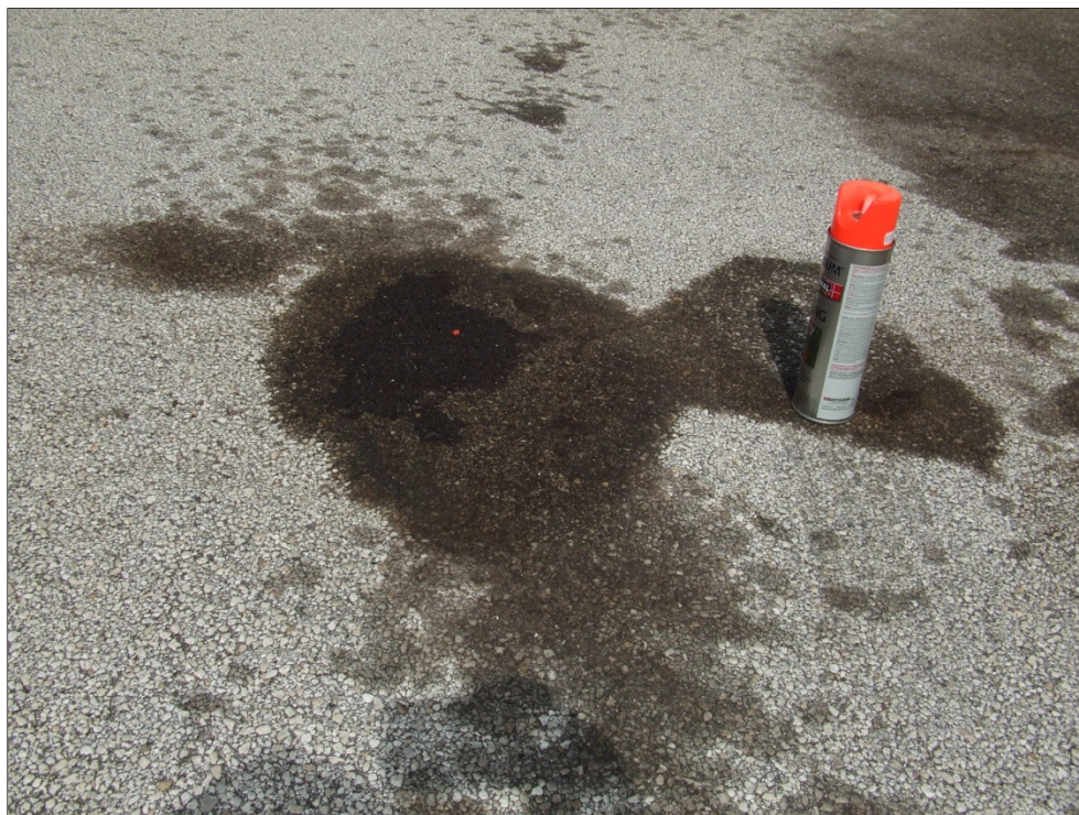
East Apron, Section 4405, Sample Unit 104 – (49) Oil Spillage and low severity (52) Weathering and Raveling.
