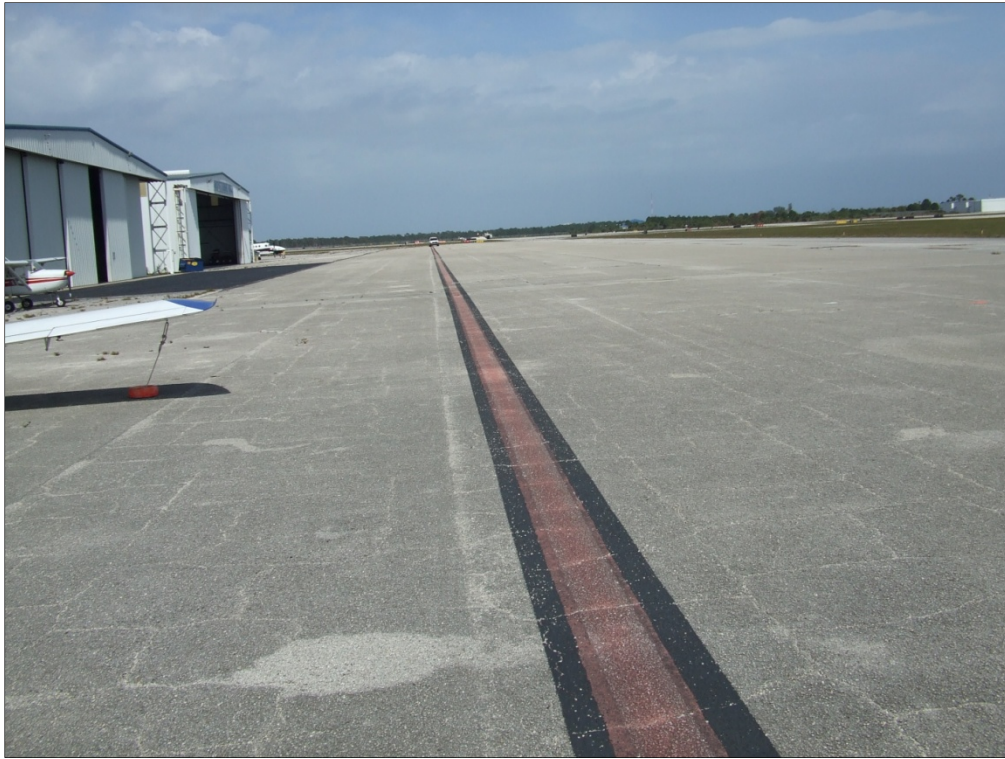
Center Apron, Section 4125, Sample Unit 199 – Low severity (43) Block Cracking and low severity (52) Weathering and Raveling.
