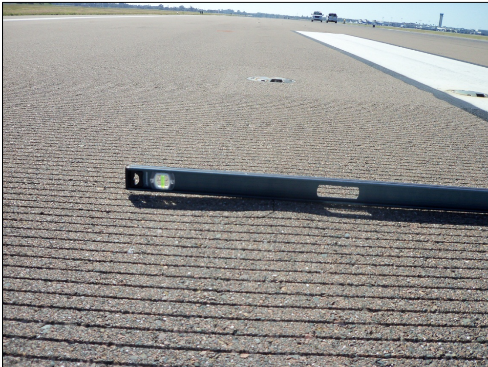
Runway 18L-36R, Section 6185, Sample Unit 419 – Low Severity (56) Swelling
