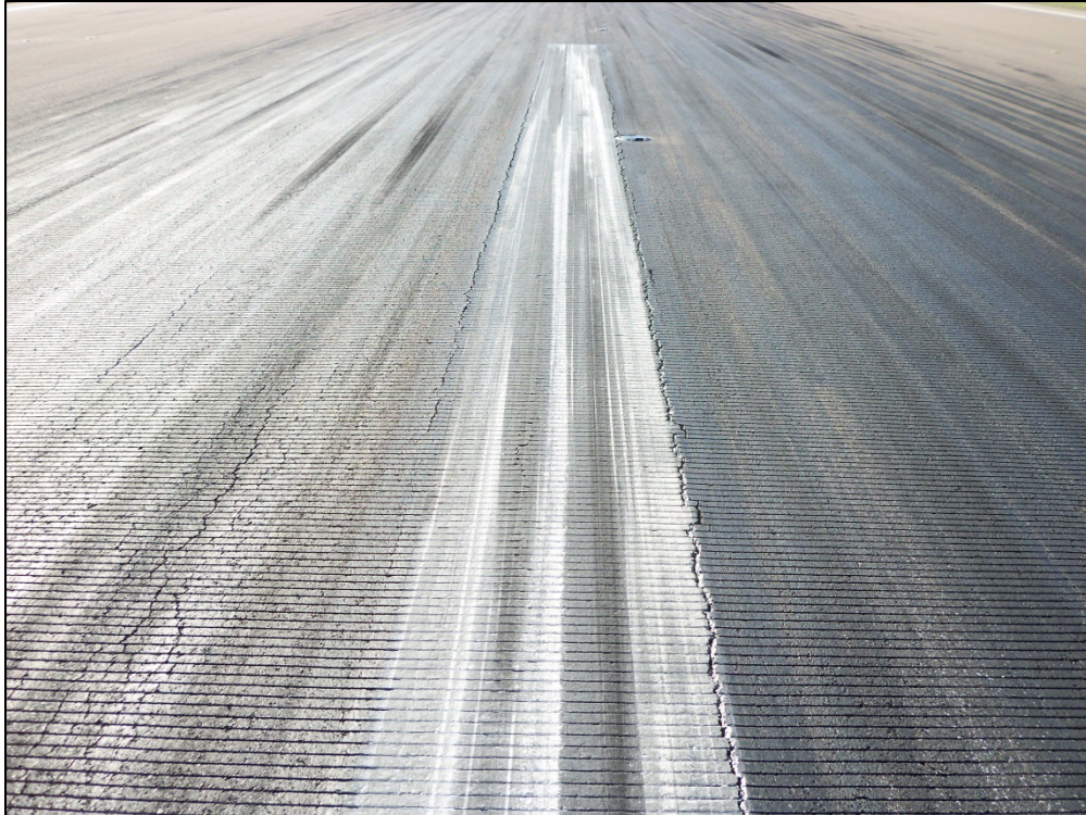
Runway 18L-36R, Section 6185, Sample Unit 437 – Low and Medium Severity (48) Longitudinal and Transverse Cracking
