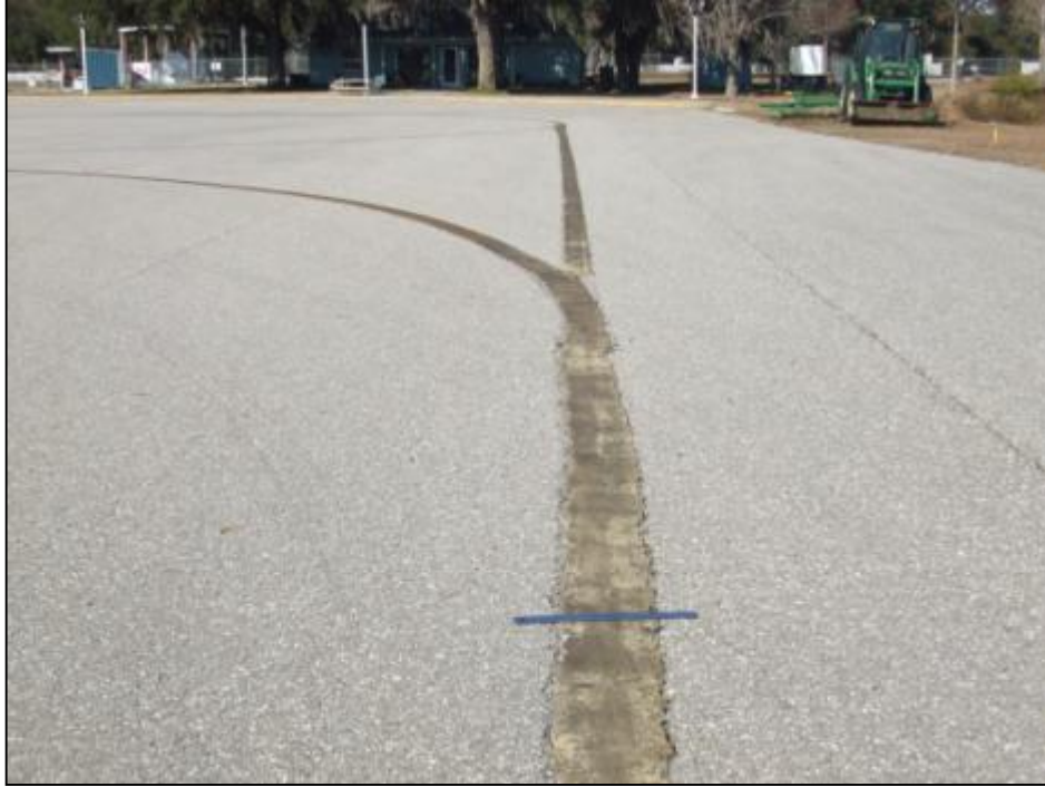
Taxiway, Section 120, Sample Unit 100 - Low and medium severity (48) Longitudinal and Transverse Cracking, low and medium severity (52) Weathering and Raveling.
