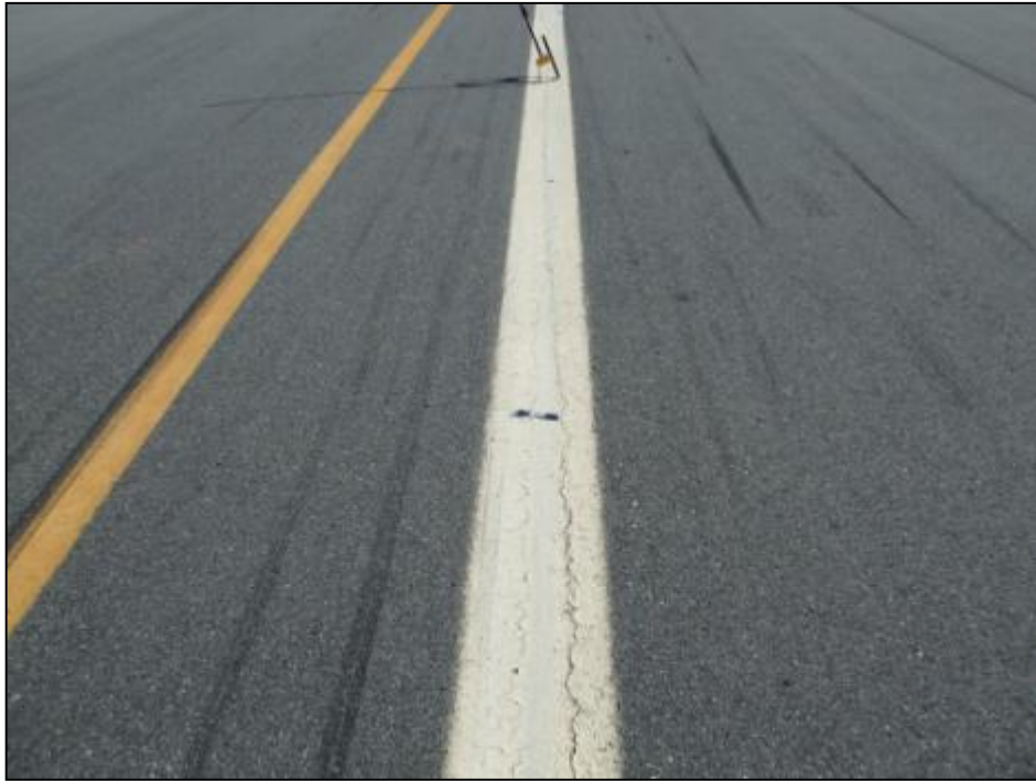
Runway 7-25, Section 6105, Sample Unit 115 – Low severity (48) Longitudinal and Transverse Cracking, low and high severity (52) Weathering and Raveling.
