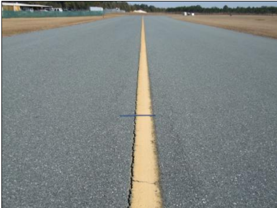
Taxiway, Section 105, Sample Unit 104 – Low and medium severity (48) Longitudinal and Transverse Cracking, low severity (56) Swelling.
