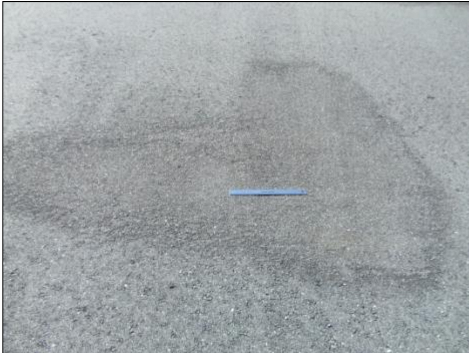
Runway 7-25, Section 6105, Sample Unit 103 – Low severity (48) Longitudinal and Transverse Cracking, low and medium severity (52) Weathering and Raveling.
