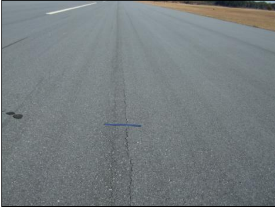
Runway 7-25, Section 6110, Sample Unit 146 - Low severity (48) Longitudinal and Transverse Cracking, low severity (52) Weathering and Raveling.
