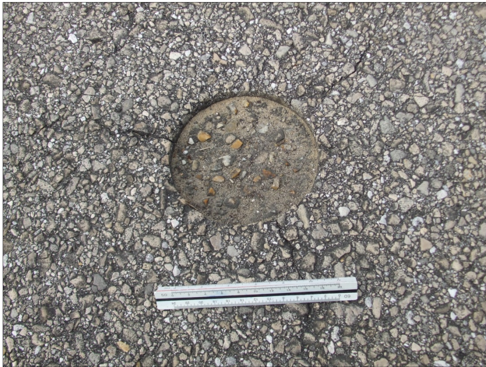
Taxiway Mike, Section 1330, Sample Unit 100 – Medium severity (50) Patching, low severity (52) Weathering and Raveling, low severity (48) Longitudinal / Transverse Cracking.
