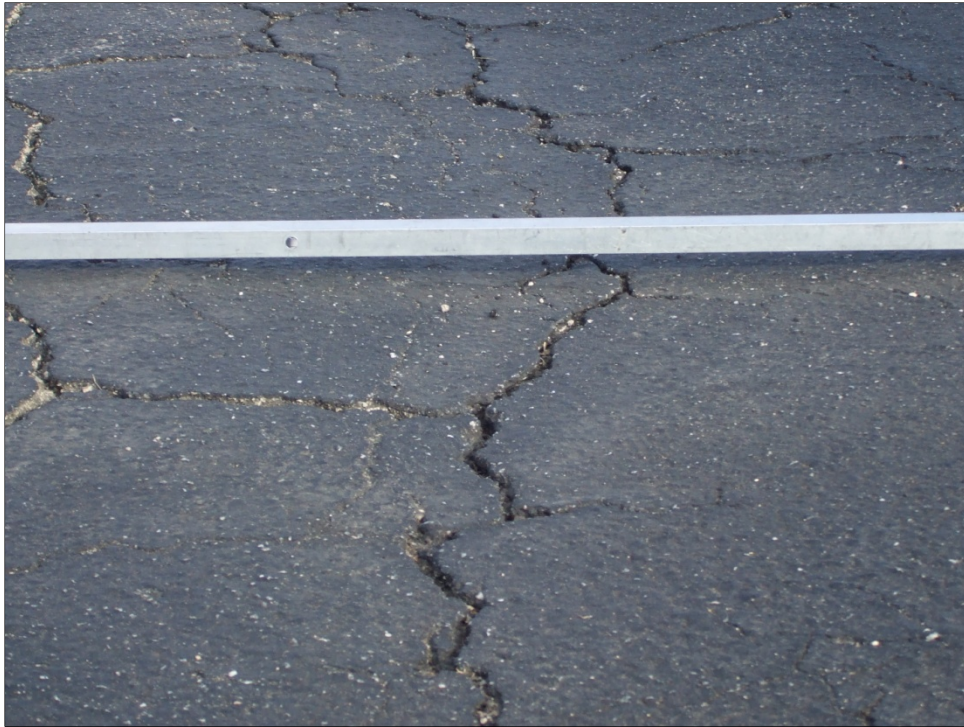
GA Apron, Section 4332, Sample Unit 359 – Low severity (45) Depression, medium severity (43) Block Cracking.
