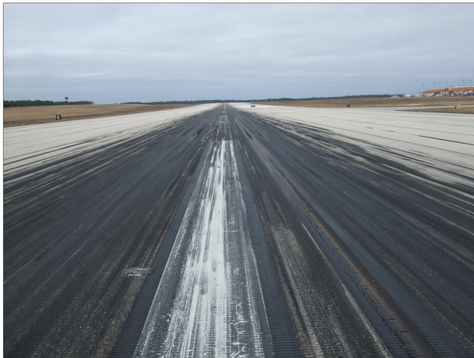
Runway 9-27, Section 6205, Sample Unit 428 – Low to medium severity (52) Weathering and Raveling.
