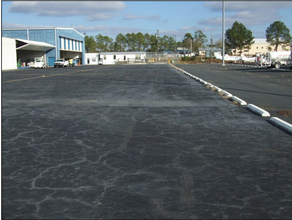
GA Apron, Section 4330, Sample Unit 611 – Low severity (43) Block Cracking, and medium severity (52) Weathering and Raveling.
