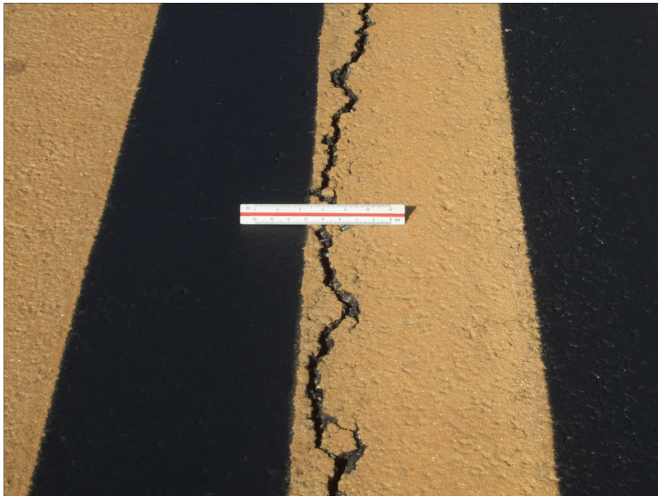
Taxiway Kilo, Section 1105, Sample Unit 106 – Medium severity (48) Longitudinal / Transverse Cracking.
