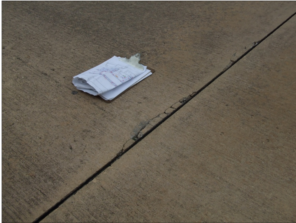
Terminal Apron, Section 4105, Sample Unit 456 – Low severity (74) Joint Spall
