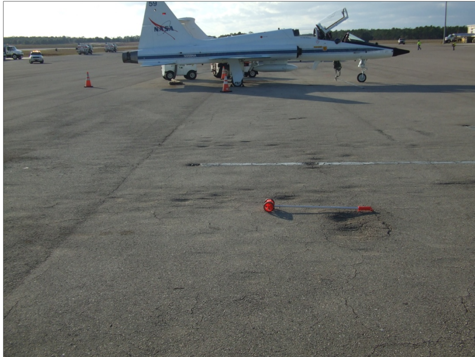
GA Apron, Section 4310, Sample Unit 306 – Medium severity (45) Depression; medium severity (56) swelling; low to medium severity (48) Longitudinal / Transverse Cracking; low to medium severity (52) Weathering and Raveling.
