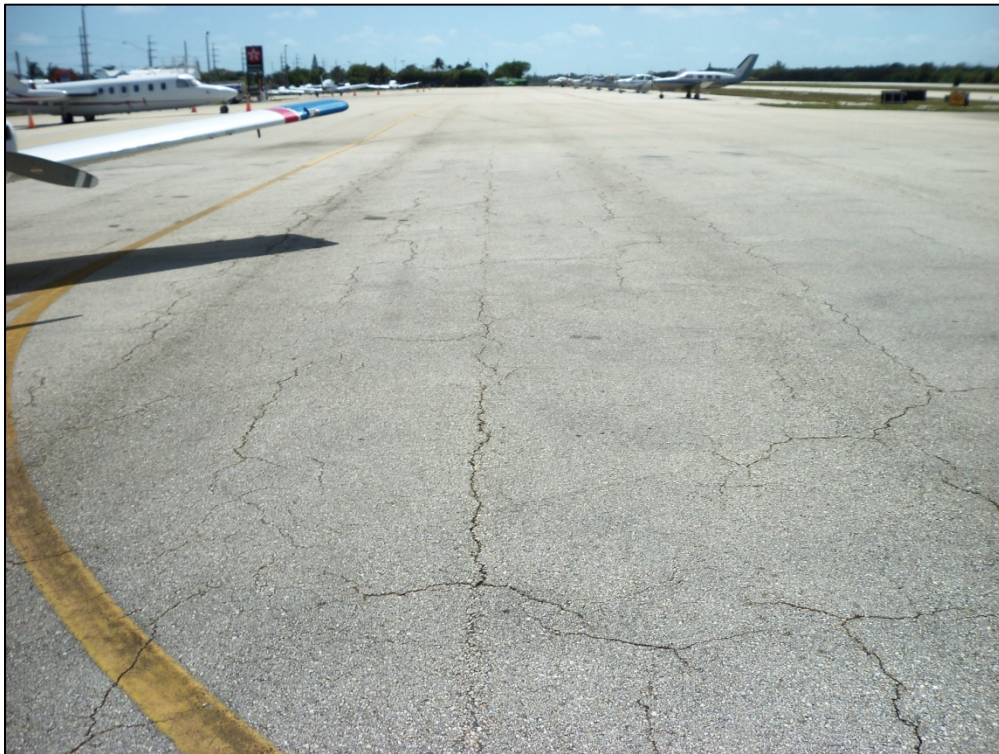
Apron, Section 4105, Sample Unit 409 – Low severity (43) Block Cracking, low severity (52) Raveling and Weathering
