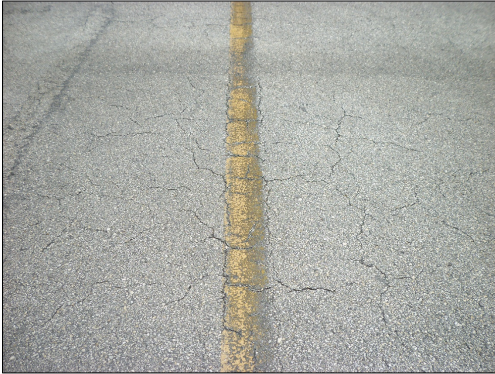
Apron, Section 4305, Sample Unit 151 – Low severity (43) Block Cracking, low severity (48) Longitudinal and Transverse Cracking, low and medium severity (50) Patch, low severity (52) Raveling and Weathering
