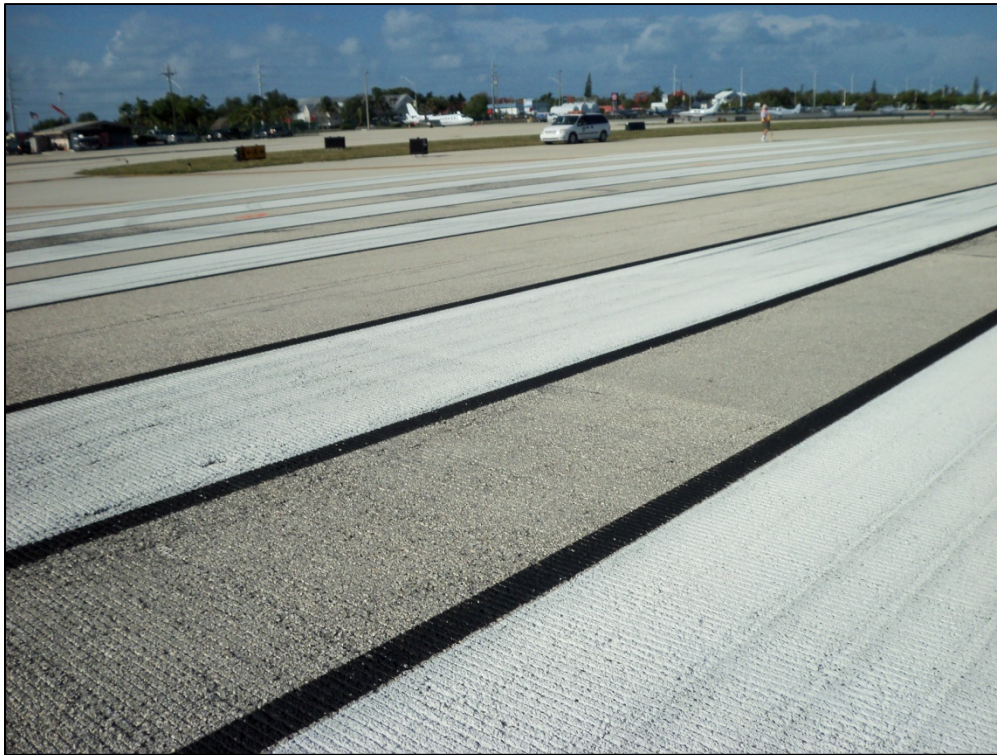
Runway 7-25, Section 6105, Sample Unit 199 – Low and medium severity (48) Longitudinal and Transverse Cracking, low, medium and high severity (52) Raveling and Weathering
