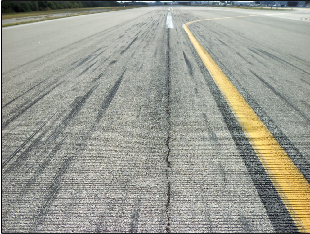
Runway 7-25, Section 6105, Sample Unit 182 – Low and high severity (48) Longitudinal and Transverse Cracking, low and medium severity (52) Raveling and Weathering
