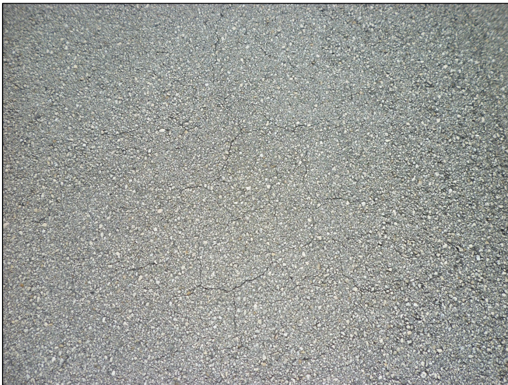
Taxiway Alpha, Section 105, Sample Unit 111 – Low severity (43) Block Cracking, low severity (48) Longitudinal and Transverse Cracking, (49) Oil Spillage, low severity (52) Raveling and Weathering
