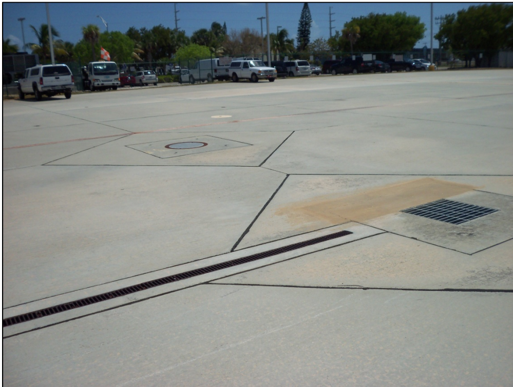
Apron, Section 4220, Sample Unit 305 – Low severity (63) Longitudinal, Transverse and Diagonal Cracking, low severity (67) Patch, low severity (70) Map Cracking, (73) Shrinkage Cracking, low severity (74) Joint Spalling, low severity (74) Corner Spalling
