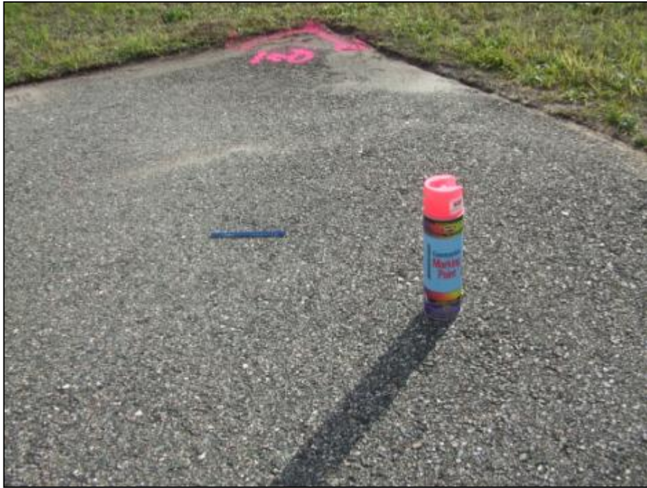
Runup Apron, Section 5105, Sample Unit 100 - Low severity (48) Longitudinal and Transverse Cracking, low severity (52) Weathering and Raveling.
