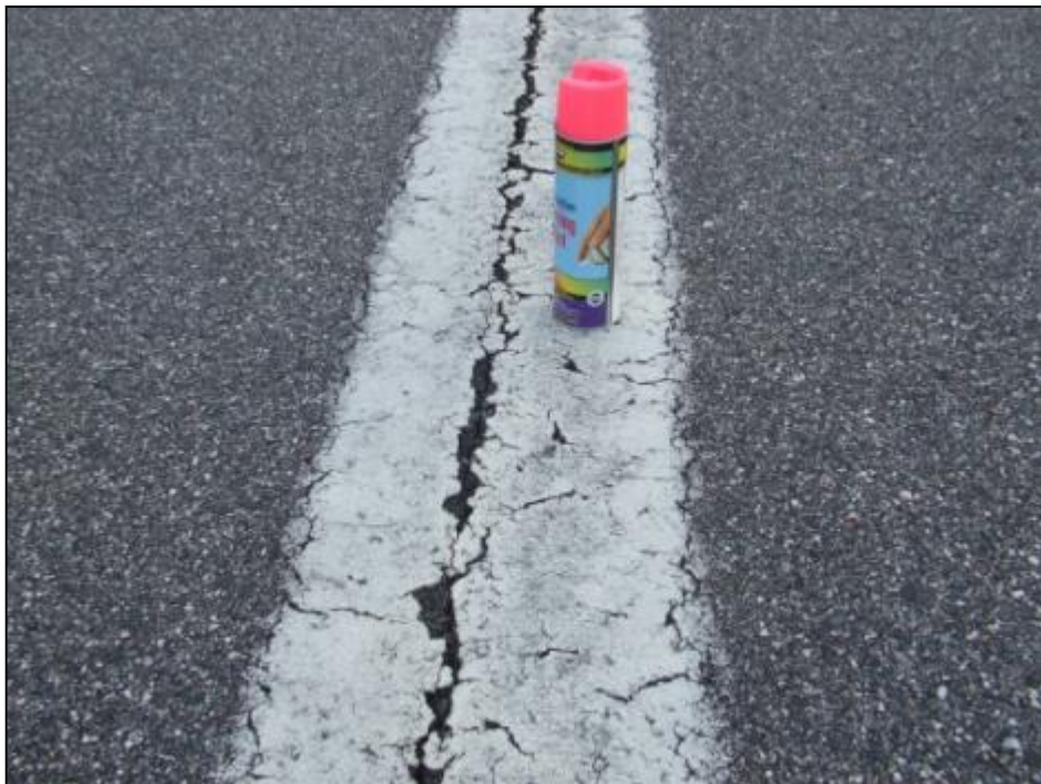
Runway 18-36, Section 6105, Sample Unit 222 - Low severity (48) Longitudinal and Transverse Cracking, low severity (52) Weathering and Raveling.
