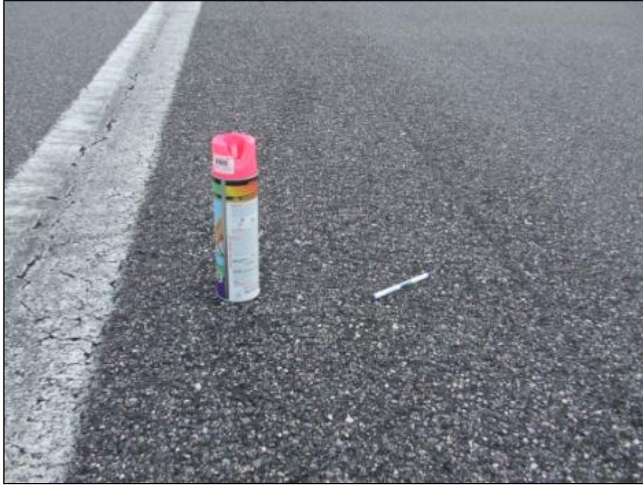
Runway 18-36, Section 6105, Sample Unit 207 – Low severity (48) Longitudinal and Transverse Cracking, low severity (52) Weathering and Raveling.
