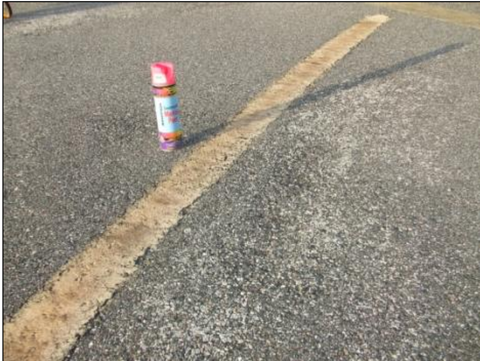
Terminal Apron, Section 4105, Sample Unit 100 – Low severity (48) Longitudinal and Transverse Cracking, low severity (50) Patching, low and medium severity (52) Weathering and Raveling.
