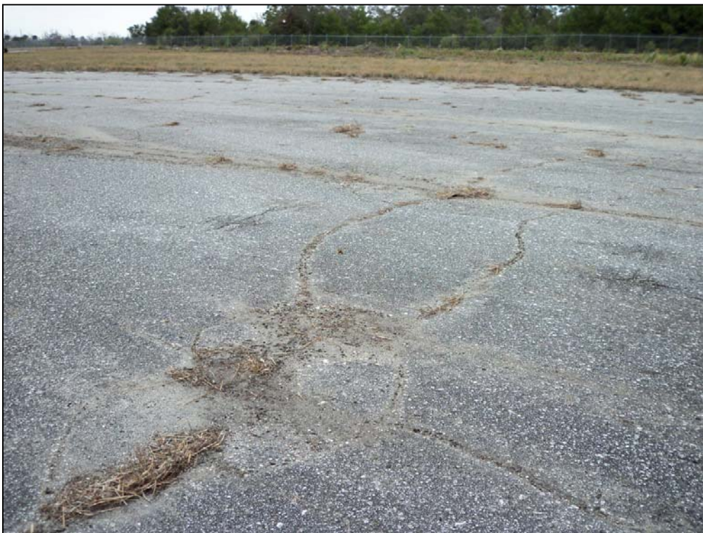
Shoulder pavement of Runway 14-32, located north of runway. High Severity Block Cracking and High Severity Weathering and Raveling.
