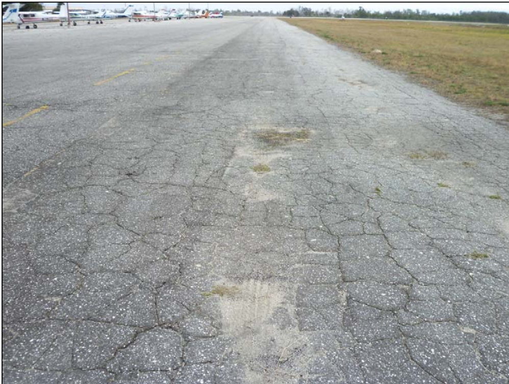
Apron, Section 4105, Sample Unit 306 – Medium/High Severity (43) Block Cracking, medium severity (52) Weathering and Raveling, and medium severity (45) Depression
