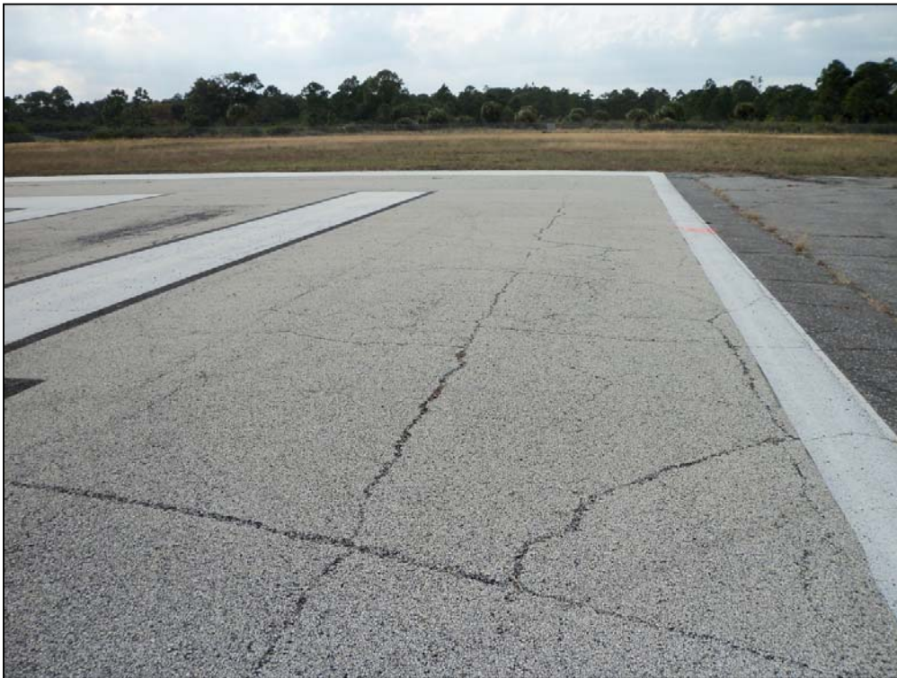
Runway 10-28, Section 6205, Sample Unit 101 – High Severity (52) Weathering and Raveling, Medium Severity (43) Block Cracking
