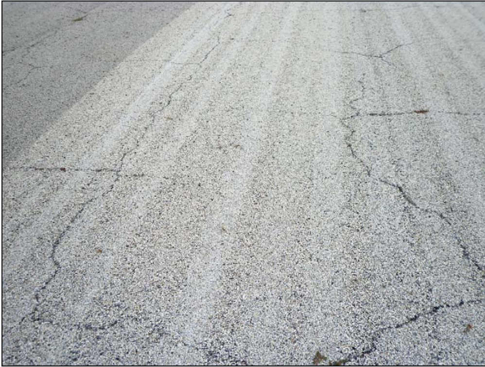
Runway 10-28, Section 6205, Sample Unit 125 – High Severity (52) Weathering and Raveling, Medium Severity (43) Block Cracking
