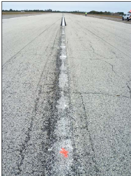
Runway 10-28, Section 6205, Sample Unit 125 – High Severity (52) Weathering and Raveling, Medium Severity (43) Block Cracking
