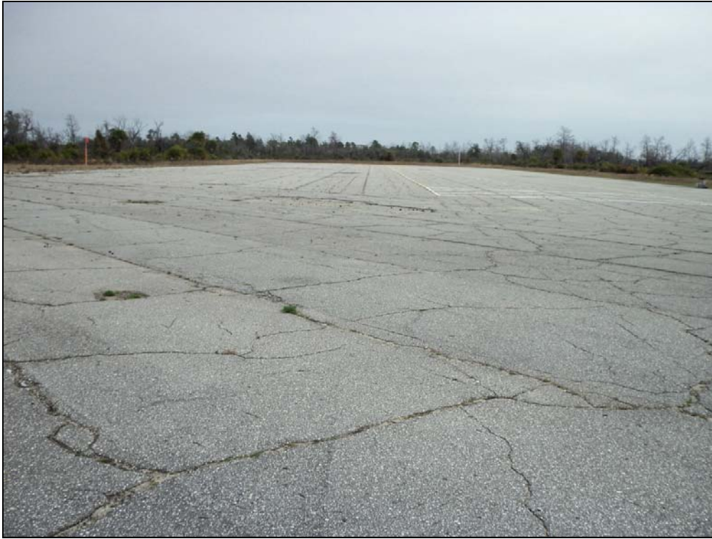
Former Runway 18-36, extension of Taxiway Bravo north of Runway 14-32. High Severity Block Cracking and High Severity Weathering and Raveling.
