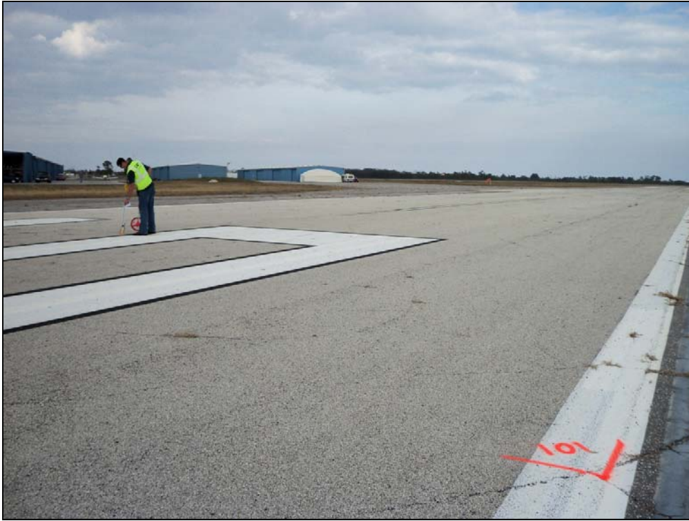
Runway 10-28, Section 6205, Sample Unit 101 – High Severity (52) Weathering and Raveling
