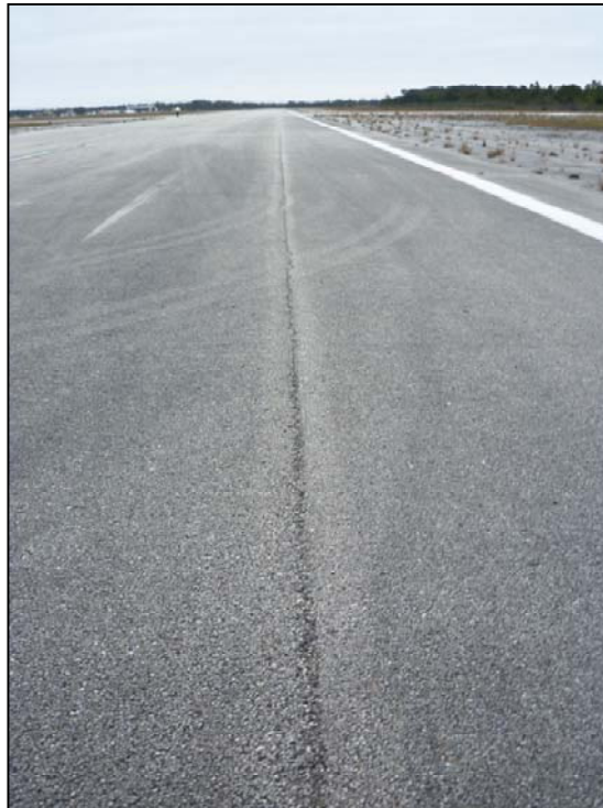
Runway 14-32, Section 6105, Sample Unit 103 – Low Severity (48) Longitudinal/Transverse Cracking and low severity (52) Weathering and Raveling
