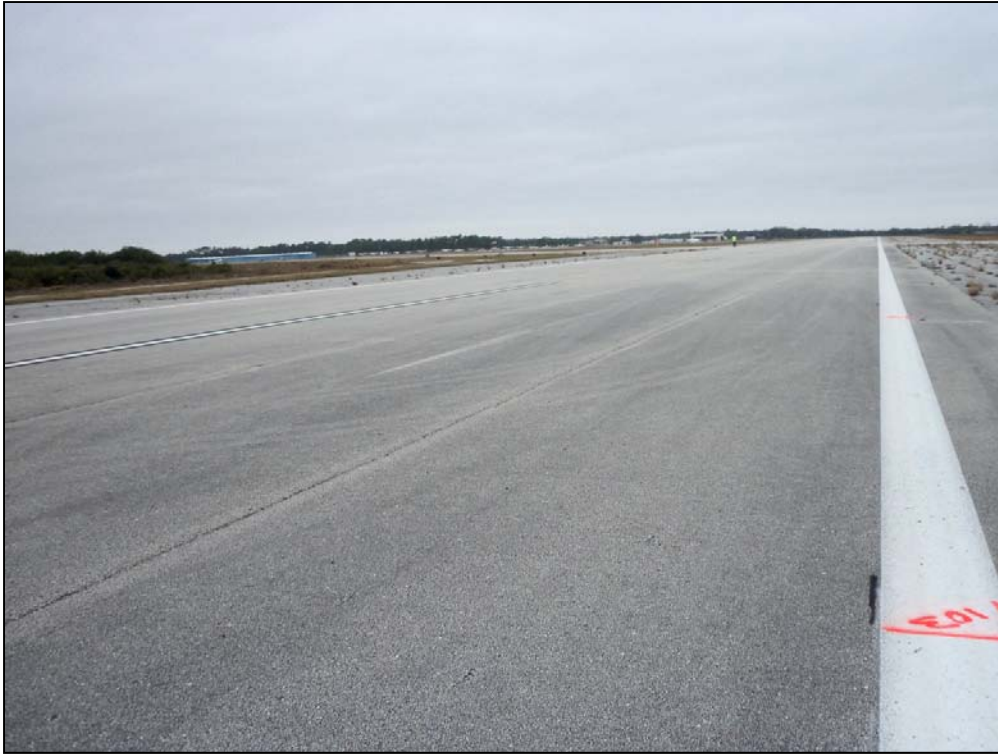
Runway 14-32, Section 6105, Sample Unit 103 – Low Severity (48) Longitudinal/Transverse Cracking and low severity (52) Weathering and Raveling
