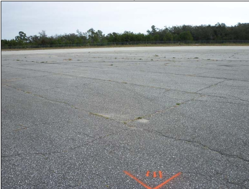
Taxiway Bravo, Section 105, Sample Unit 111 – Medium Severity (43) Block Cracking and low severity (52) Weathering and Raveling
