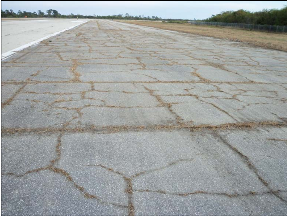
Shoulder pavement of Runway 10-28, located between runway and golf course. High Severity Block Cracking and High Severity Weathering and Raveling.
