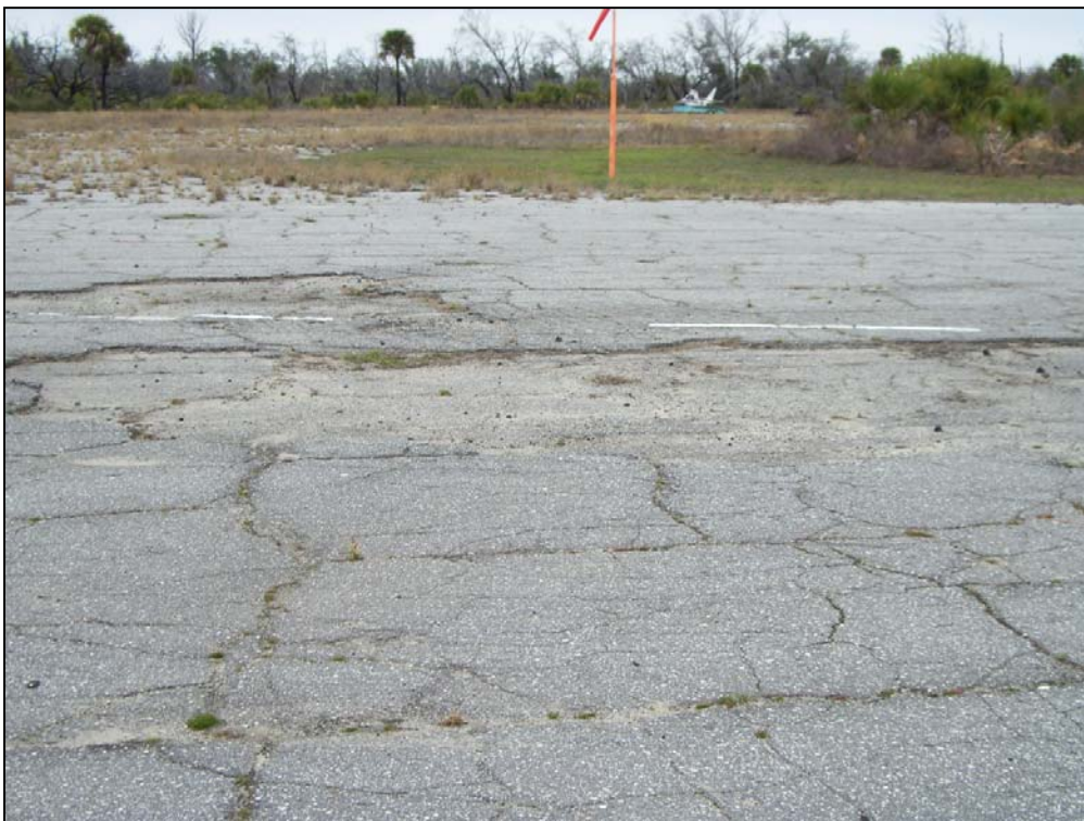
Former Runway 4-22, apron extension beyond Runway 14-32. High Severity Block Cracking and High Severity Weathering and Raveling.
