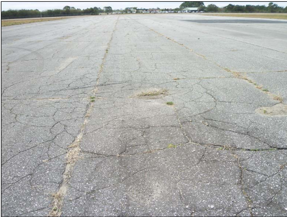
Taxiway Bravo, Section 105, Sample Unit 105 – Medium Severity (43) Block Cracking, high severity (45) Depression, and low severity (52) Weathering and Raveling
