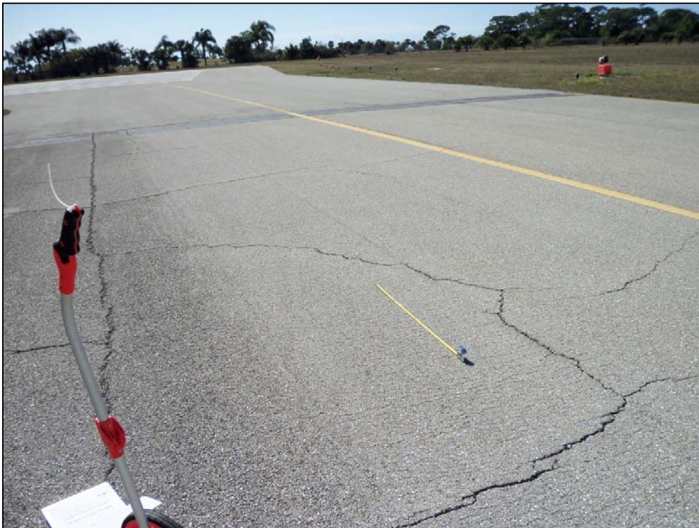
Taxiway Alpha, Section 115, Sample Unit 142 – Low and medium severity (43) Block Cracking, low severity (52) Weathering and Raveling
