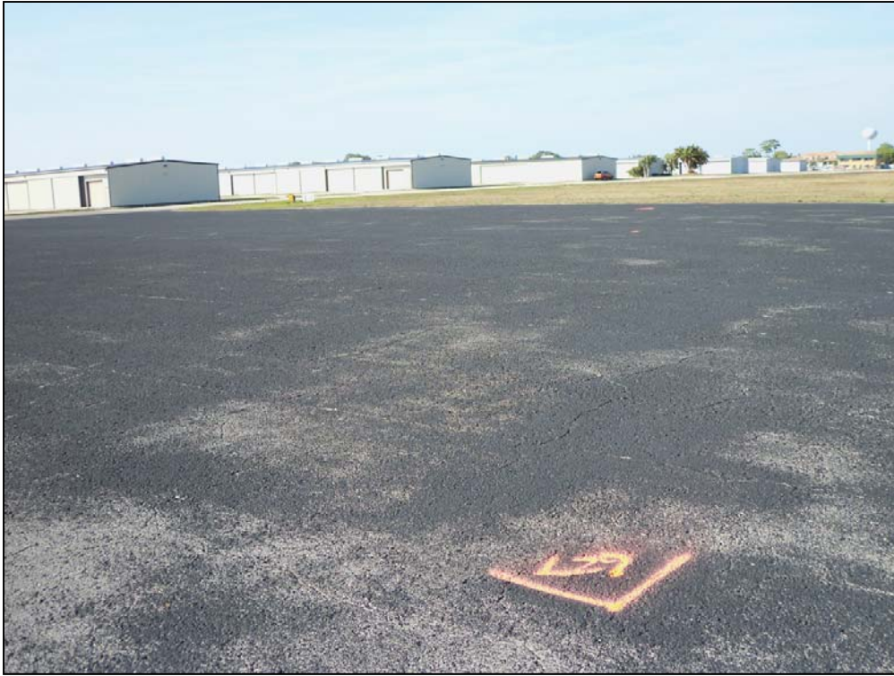
Former Runway 9-27, Section 6415, Sample Unit 627 – Medium severity (43) Block Cracking, medium severity (52) Weathering and Raveling
