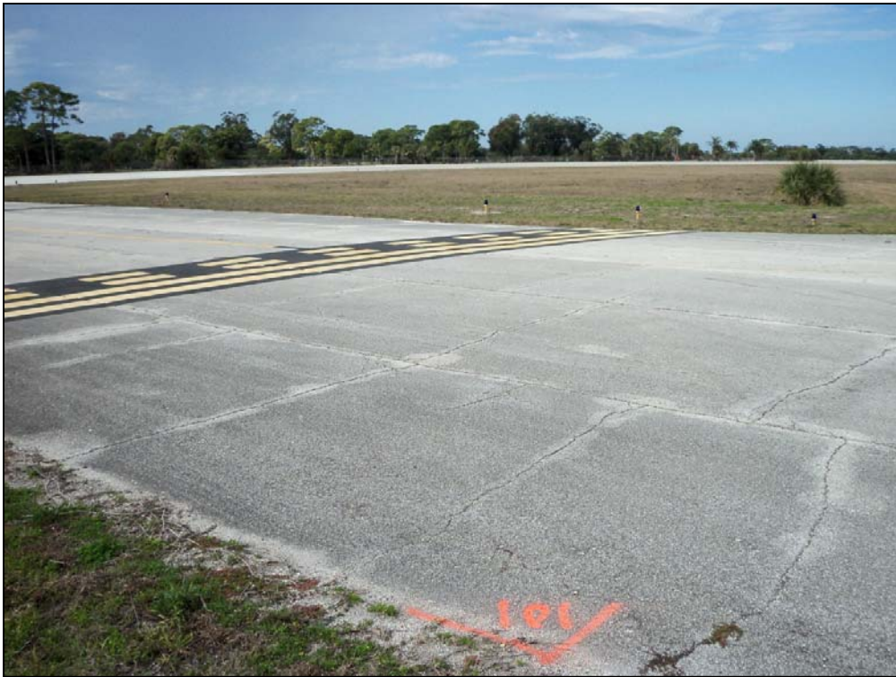
Taxiway Delta, Section 350, Sample Unit 101 – Medium and high severity (43) Block Cracking, medium severity (52) Weathering and Raveling
