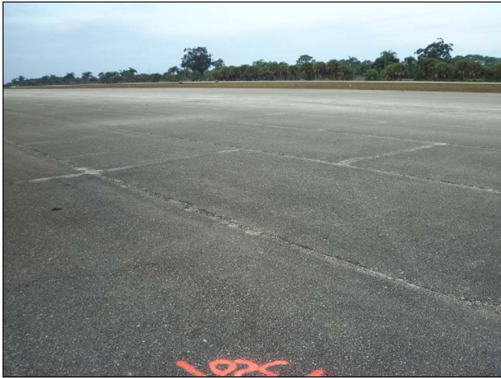
Runway 4-22, Section 6205, Sample Unit 320 – Medium severity (43) Block Cracking, medium severity (48) Longitudinal and Transverse Cracking, medium and high severity (52) Weathering and Raveling
