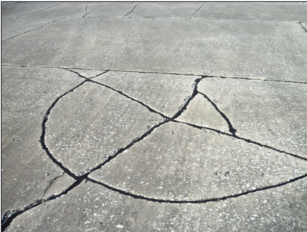
Apron, Section 4120, Sample Unit 351 – Low and medium severity (62) Corner Break, low, medium and high severity (63) LTD Cracking, medium severity (65) Joint Seal Damage, low severity (70) Scaling/Map Cracking, medium severity (72) Shattered Slab, low, medium and high severity (74) Joint Spalling, low severity (75) Corner Spalling
