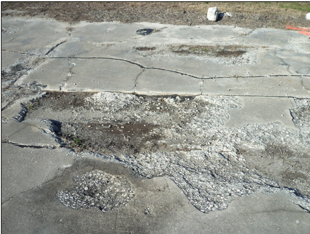
Apron, Section 4120, Sample Unit 450 – Low and high severity (63) LTD Cracking, medium severity (65) Joint Seal Damage, high severity (66) Small Patch, (63) Popouts, low and medium severity (70) Scaling/Map Cracking, medium and high severity (72) Shattered Slab, medium severity (74) Joint Spalling
