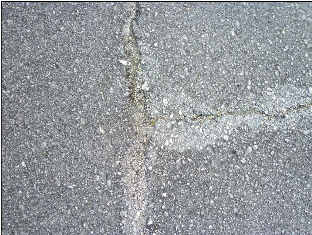
Runway 4-22 Shoulder, Section 6210, Sample Unit 520 – Medium severity (43) Block Cracking, medium severity (52) Weathering and Raveling
