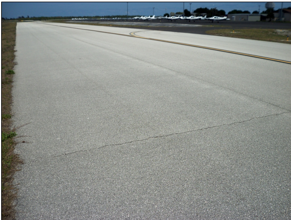
Taxiway Alpha, Section 105, Sample Unit 107 – Low severity (48) Longitudinal and Transverse Cracking, low severity (52) Weathering and Raveling
