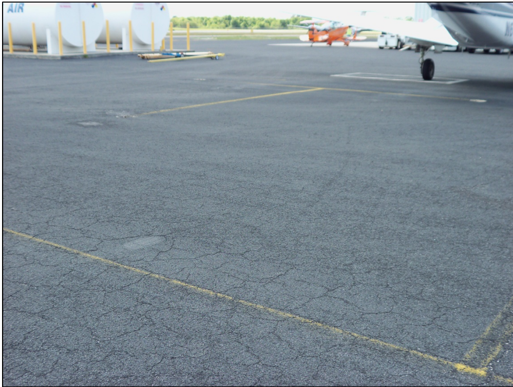
Apron, Section 4310, Sample Unit 303 – Low severity (52) Weathering and Raveling
