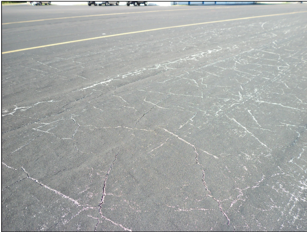
NE Apron, Section 5405, Sample Unit 212 – Low severity (43) Block Cracking, low severity (52) Weathering and Raveling
