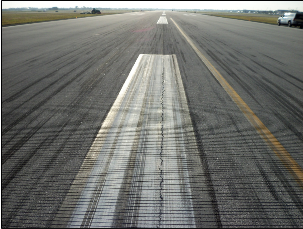
Runway 11R-29L, Section 6110, Sample Unit 134 – Low severity (48) Longitudinal Cracking and low severity (52) Weathering and Raveling
