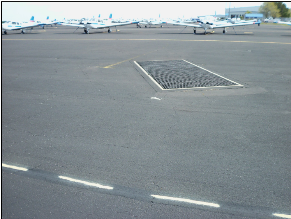
Apron, Section 4205, Sample Unit 351 – Low severity (43) Block Cracking, low severity (50) Patch, low severity (52) Weathering and Raveling
