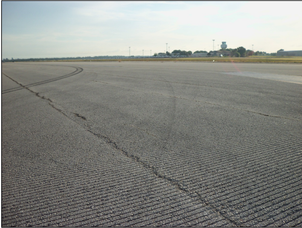
Runway 4-22, Section 6305, Sample Unit 101 – Low severity (43) Block Cracking, low and medium severity (48) Longitudinal and Transverse Cracking, low and medium severity (52) Weathering and Raveling
