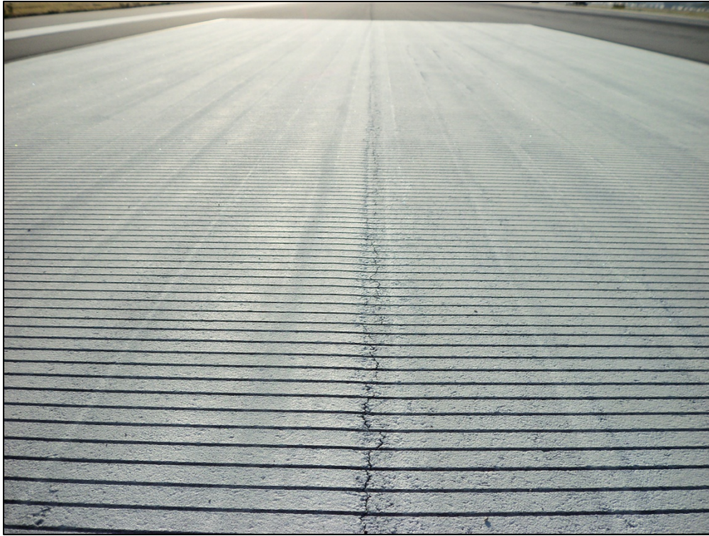
Runway 11R-29L, Section 6105, Sample Unit 122 – Low severity (48) Longitudinal Cracking and low severity (52) Weathering and Raveling
