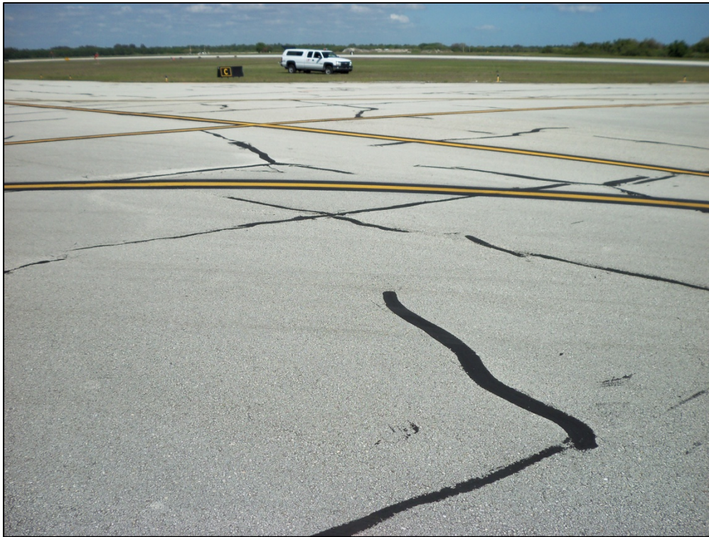
Taxiway C-1, Section 330, Sample Unit 308 – Low severity (43) Block Cracking, low severity (52) Weathering and Raveling
