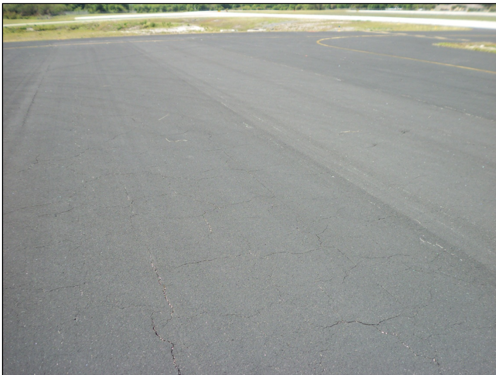
Apron, Section 4105, Sample Unit 100 – Low severity (43) Block Cracking, (52) Weathering and Raveling
