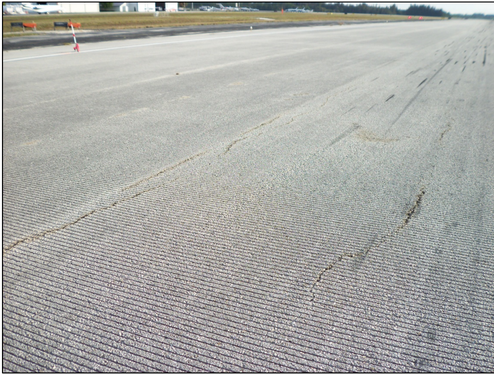
Runway 4-22, Section 6305, Sample Unit 108 – Low and medium severity (48) Longitudinal and Transverse Cracking, low and medium severity (52) Weathering and Raveling
