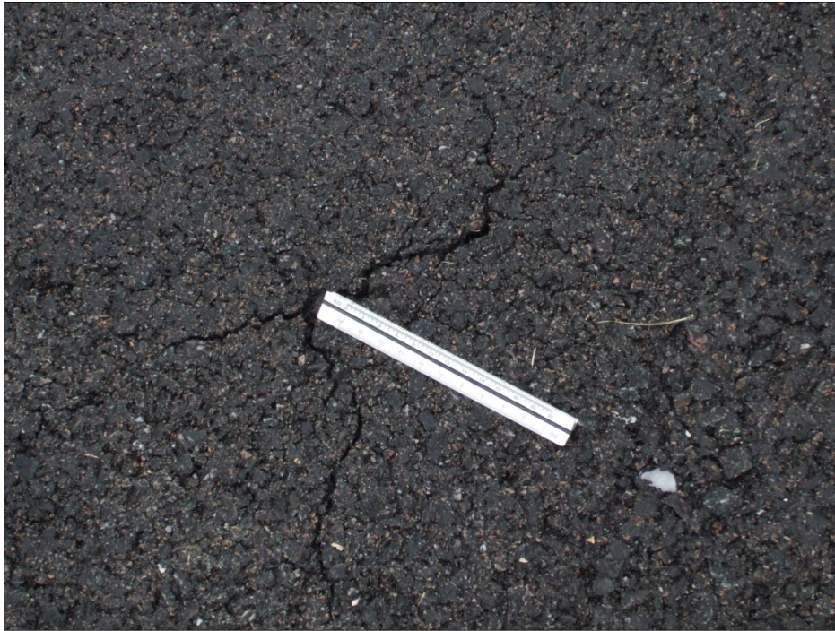
Apron, Section 4105, Sample Unit 102 – Low severity (48) Longitudinal / Transverse Cracking.
