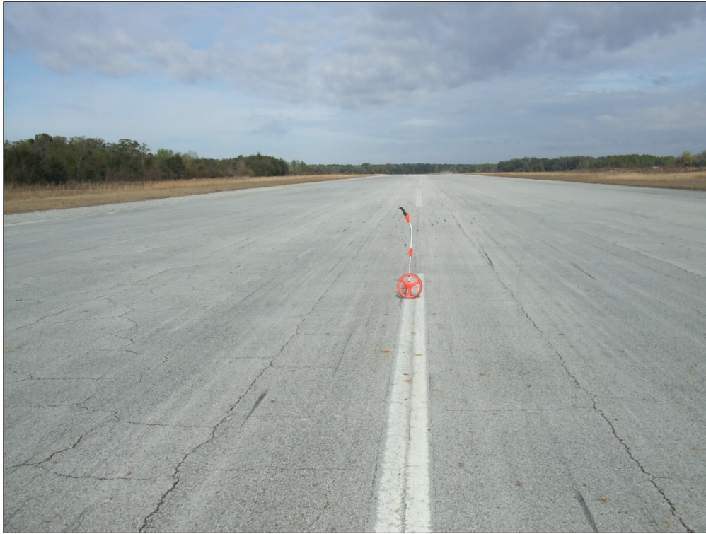
Runway 14-32, Section 6215, Sample Unit 326 – Low and moderate severity (43) Block Cracking; low severity (48) Longitudinal / Transverse Cracking, and low severity (52) Weathering and Raveling.
