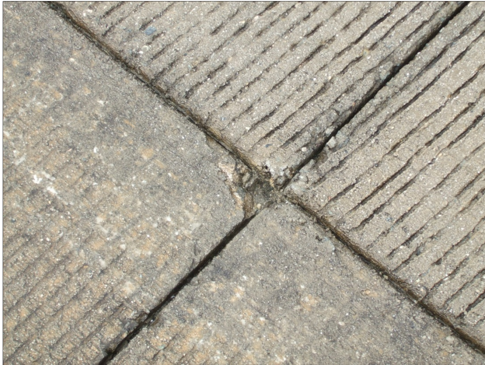
Runway 5-23, Section 6115, Sample Unit 349 – Corner spall observed in whitetopping.
