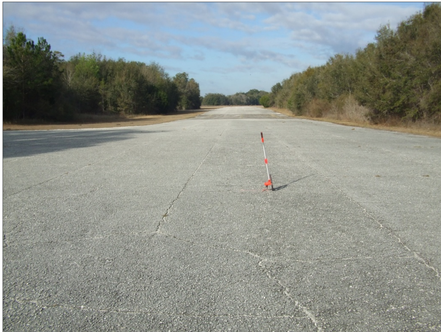
Taxiway Fox Trot, Section 550, Sample Unit 135 – Medium to high severity (43) Block Cracking; low to medium severity (48) Longitudinal / Transverse Cracking; and medium to high severity (52) Weathering and Raveling.
