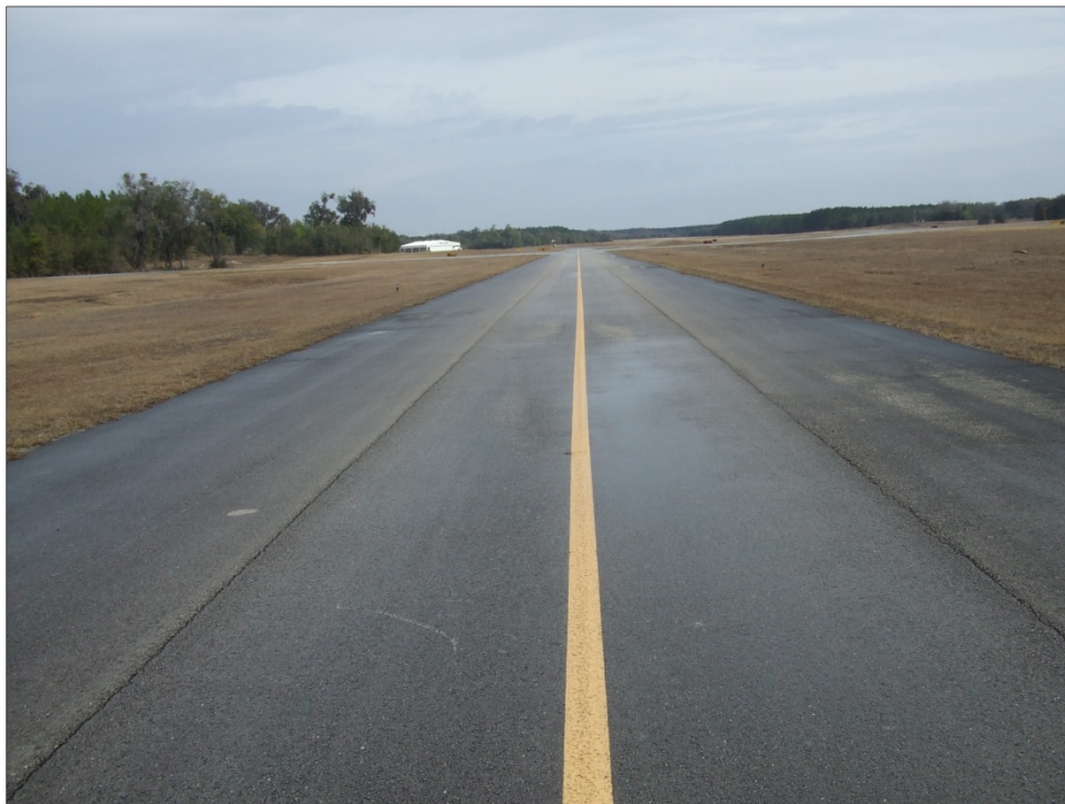
Taxiway Alpha, Section 205, Sample Unit 108 – Low severity (48) Longitudinal / Transverse Cracking; and low to medium severity (52) Weathering and Raveling.
