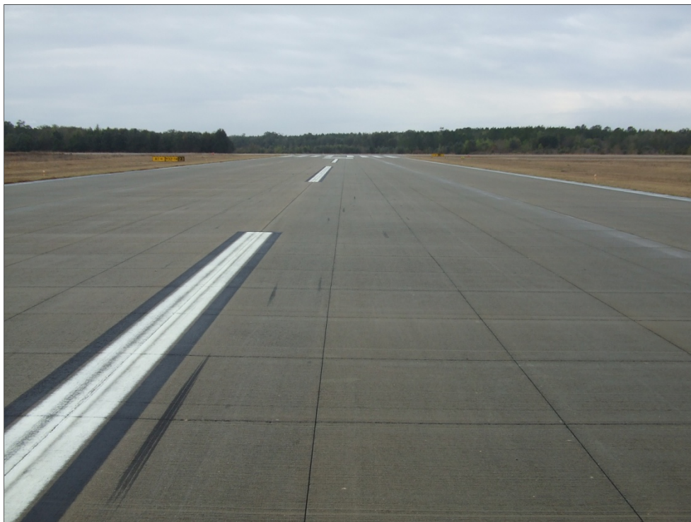
Runway 5-23, Section 6115, Sample Unit 315 – Overview of sample unit. Joint spalls observed on sample unit.
