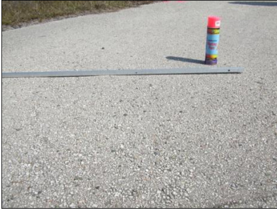
Taxiway Bravo, Section 220, Sample Unit 100 – Low severity (45) Depression, low severity (48) Longitudinal and Transverse Cracking, low severity (52) Weathering and Raveling, low severity (56) Swelling.
