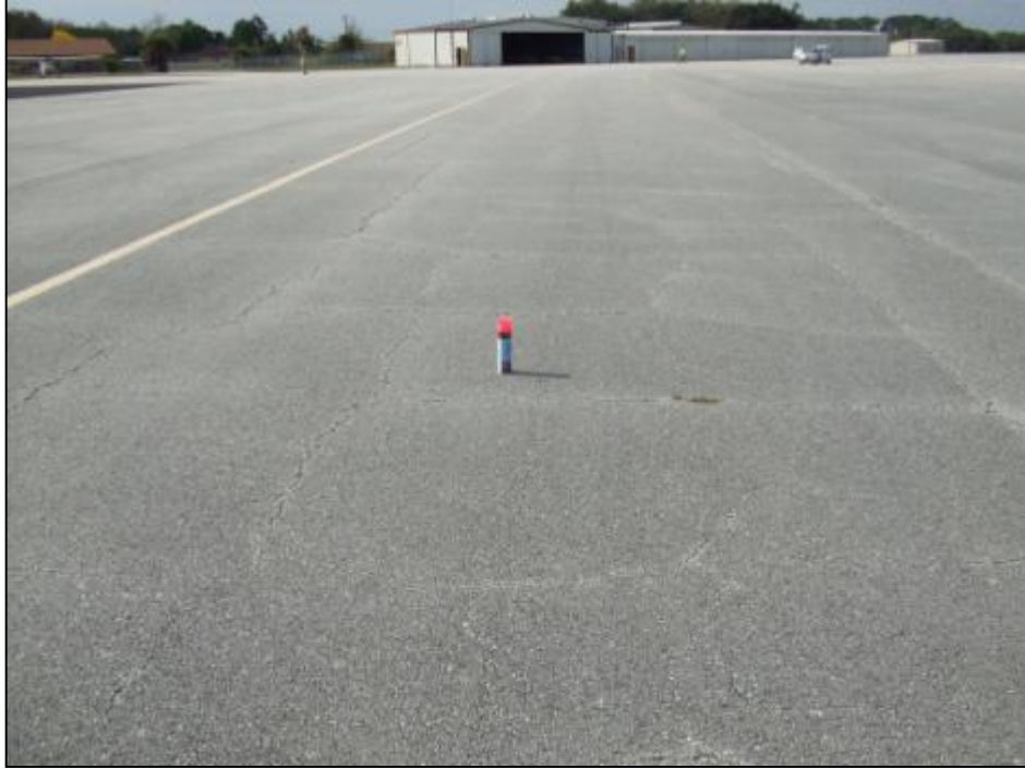
Apron Area, Section 410, Sample Unit 353 – Low and medium severity (43) Block Cracking, low severity (48) Longitudinal and Transverse Cracking, low and medium severity (52) Weathering and Raveling.
