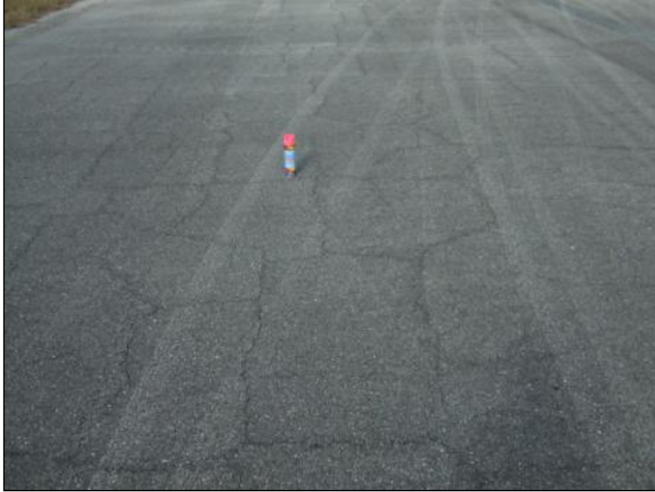
Runway 11-29, Section 5105, Sample Unit 183 – Low severity (43) Block Cracking, low severity (48) Longitudinal and Transverse Cracking, low severity (52) Weathering and Raveling, low severity (56) Swelling.
