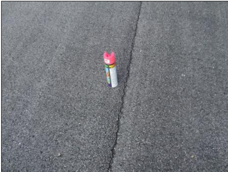
Runway 11-29, Section 6205, Sample Unit 103 – Low severity (48) Longitudinal and Transverse Cracking, low severity (50) Patching, low severity (52) Weathering and Raveling.
