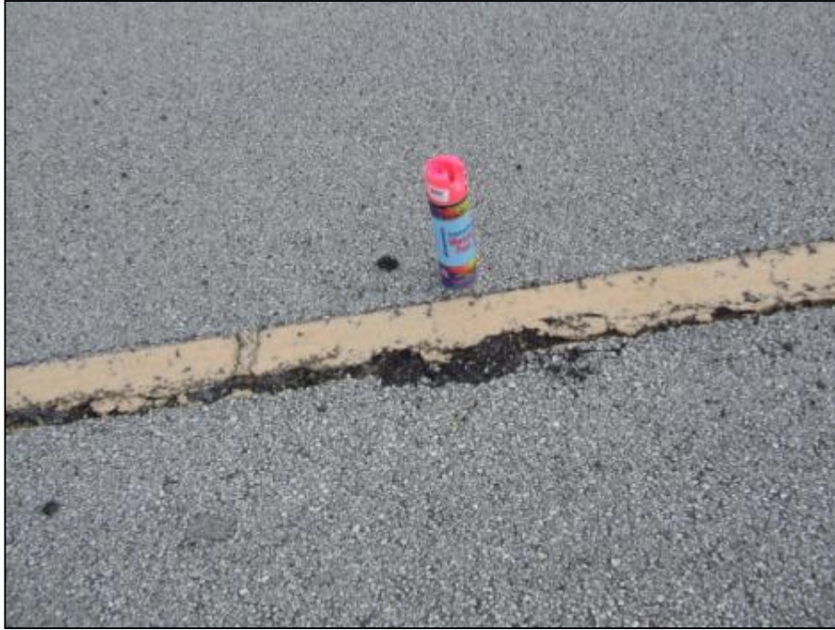
Taxiway Alpha, Section 110, Sample Unit 406 – Low and medium severity (48) Longitudinal and Transverse Cracking, low and medium severity (52) Weathering and Raveling.
