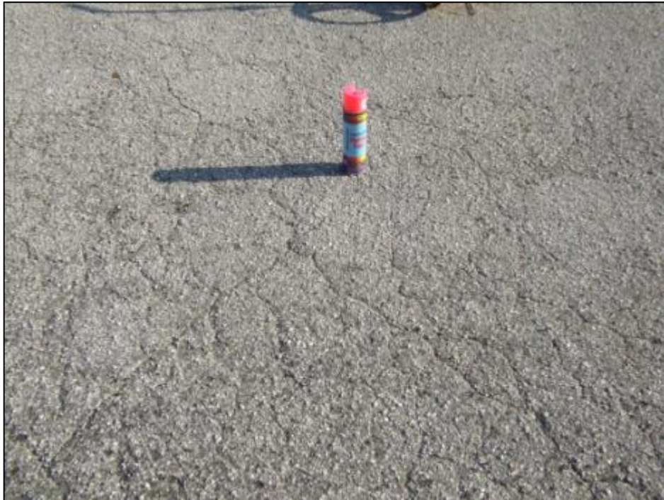
Apron Area, Section 4125, Sample Unit 101 – Medium severity (41) Alligator Cracking, low severity (45) Depression, low severity (48) Longitudinal and Transverse Cracking, low severity (52) Weathering and Raveling, low severity (56) Swelling.
