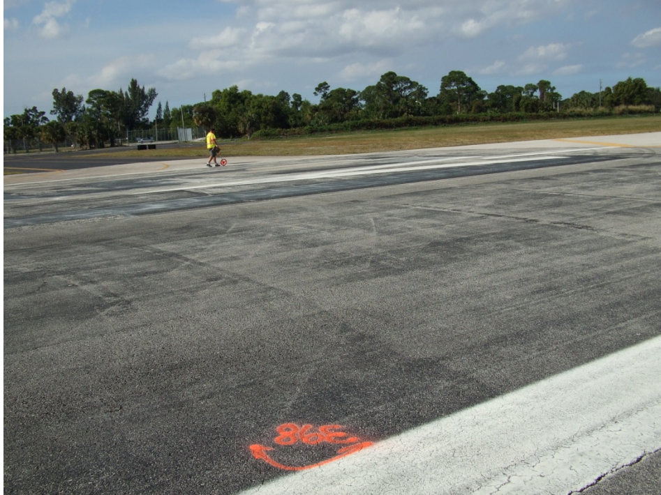
Runway 16-34, Section 6305, Sample Unit 398 – Low severity (48) Longitudinal and Transverse Cracking, Medium severity (52) Weathering and Raveling.
