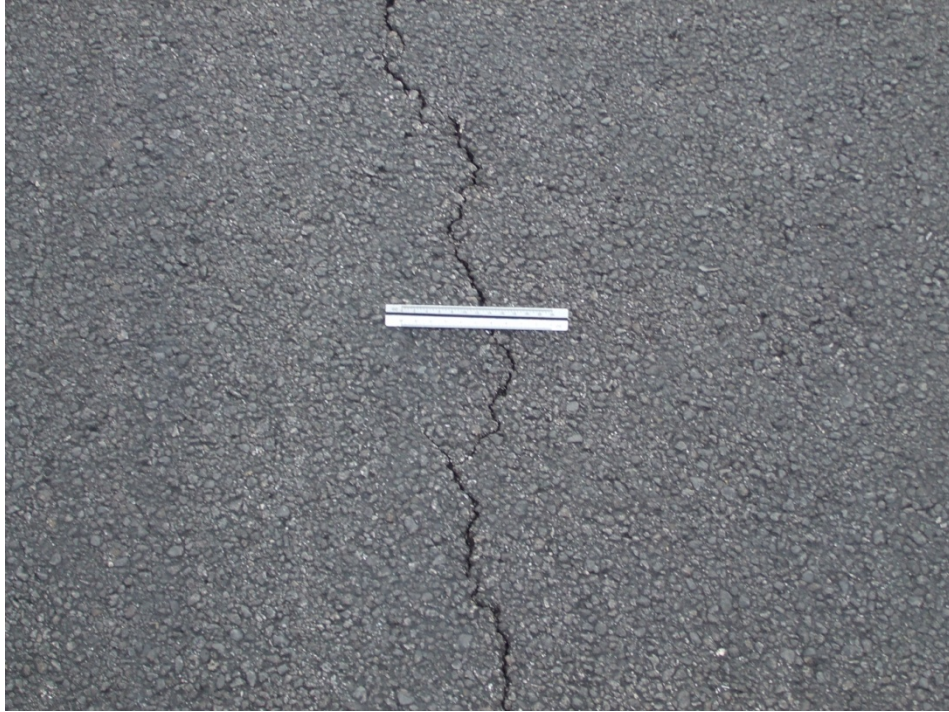
Taxiway Alpha, Section 136, Sample Unit 100 – Low severity (48) Longitudinal and Transverse Cracking, low severity (52) Weathering and Raveling.
