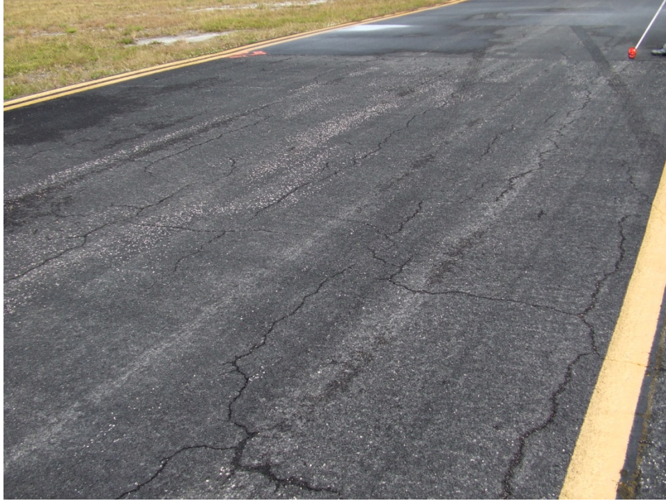
Taxiway Bravo, Section 206, Sample Unit 201 – Medium severity (43) Block Cracking, medium severity (52) Weathering and Raveling.
