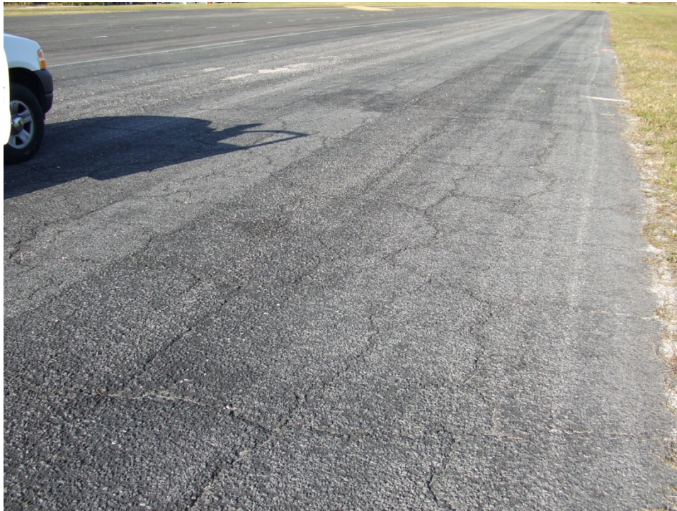
North Apron, Section 4405, Sample Unit 312 – High severity (52) Weathering and Raveling, Medium severity (43) Block Cracking.
