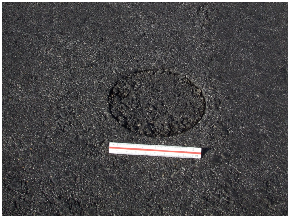
Taxiway Delta, Section 405, Sample Unit 320 – Low severity (50) Patching.
