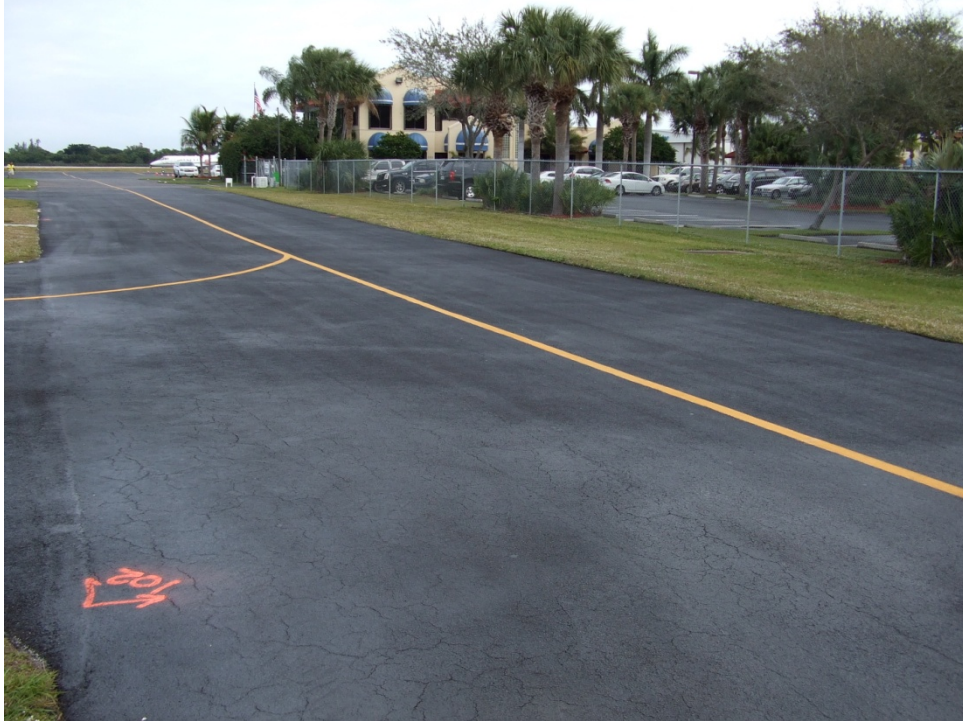
East Apron, Section 4215, Sample Unit 102 – Low severity (48) Longitudinal and Transverse Cracking, low severity (52) Weathering and Raveling, low severity (43) Block Cracking.
