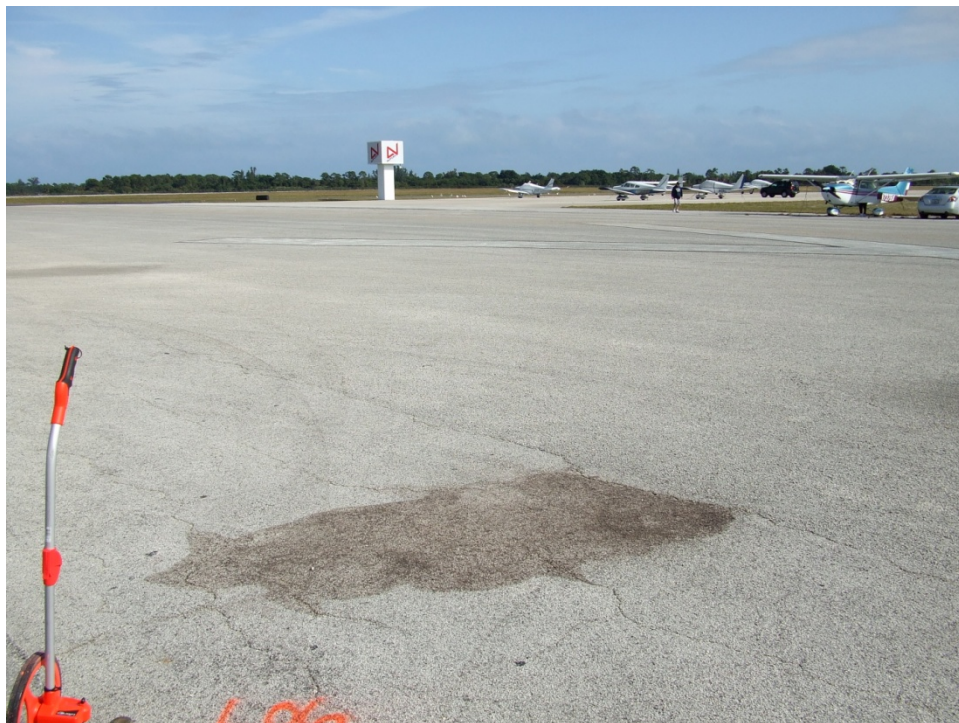
Taxiway Charlie, Section 330, Sample Unit 907 – Medium severity (45) Depression, Medium severity (52) Weathering and Raveling.
