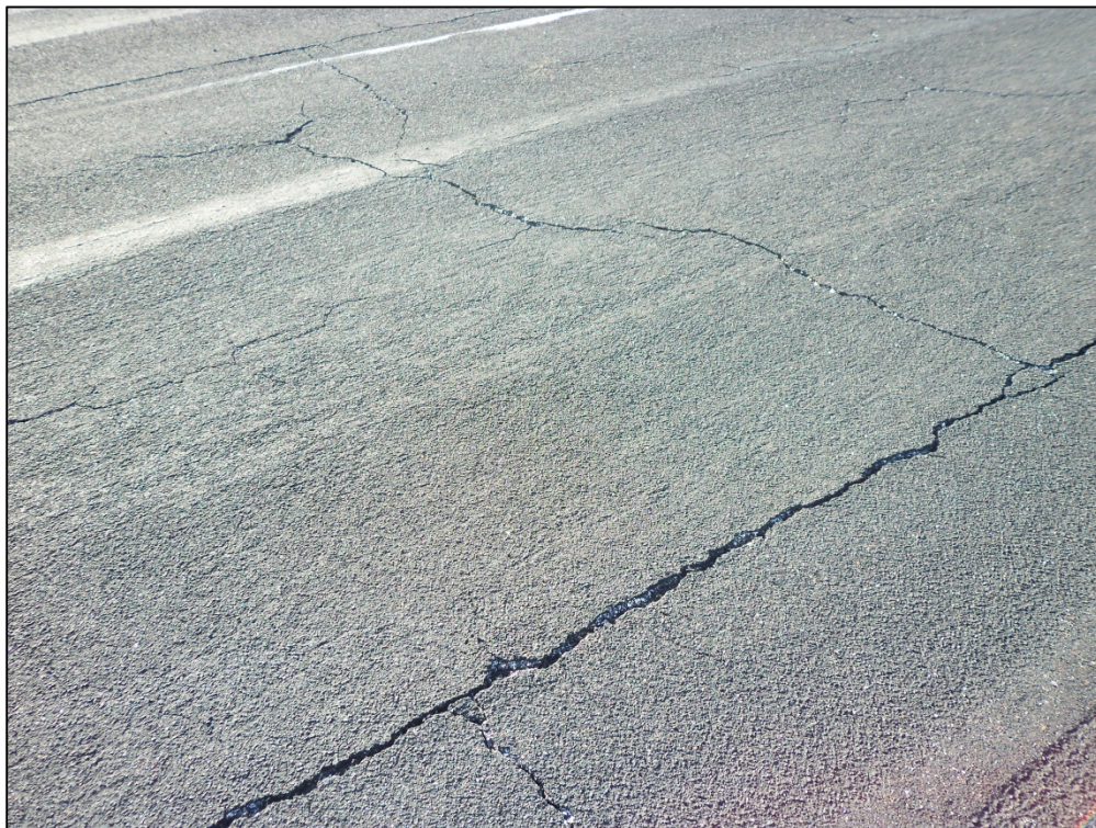
Runway 4-22, Section 6105, Sample Unit 134 –Medium severity (48) Longitudinal and Transverse Cracking, Low severity (52) Raveling and Weathering
