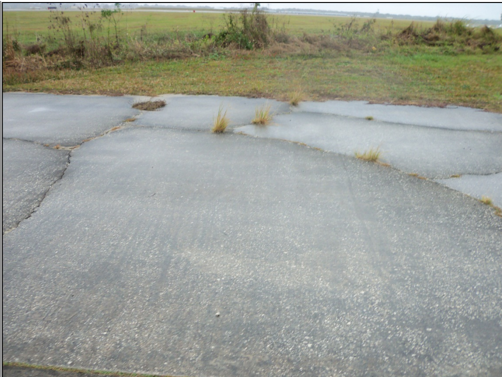
Apron East, Section 5405, Sample Unit 202 – Medium severity (65) Joint Seal Damage, High severity (72) Shattered Slab
