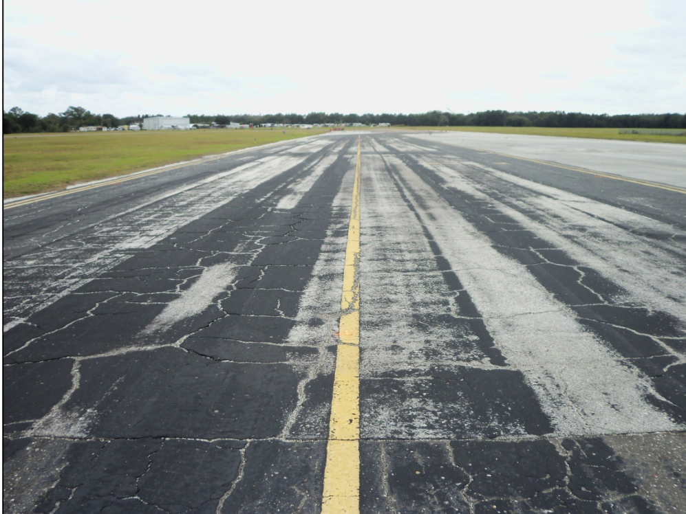
Taxiway Bravo, Section 220, Sample Unit 219 – High severity (43) Block cracking, High severity (52) Raveling and Weathering
