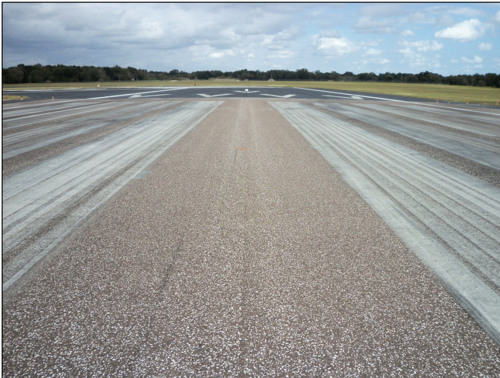
Runway 18-36, Section 6205, Sample Unit 390 –Low severity (52) Raveling and Weathering
