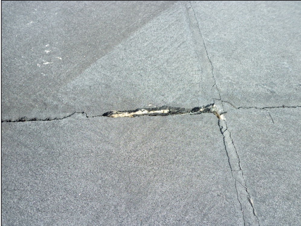
Runway 18-36, Section 6213, Sample Unit 301 –Medium severity (47) Joint Reflection Cracking, Low severity (48) Longitudinal and Transverse Cracking
