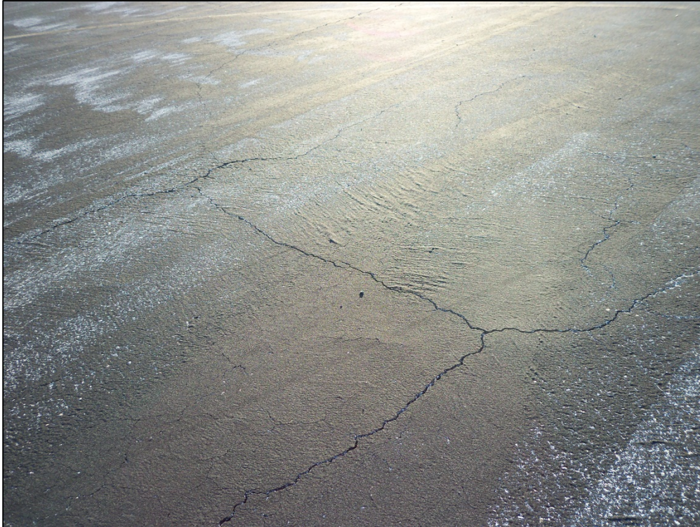
Taxiway Connector A-2, Section 310, Sample Unit 103 – Low severity (48) Longitudinal and Transverse Cracking, (52) Raveling and Weathering
