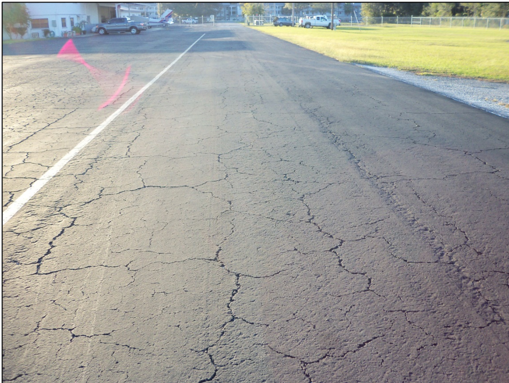
Apron Taxiway Delta, Section 5205, Sample Unit 201 – Low severity (43) Block Cracking
