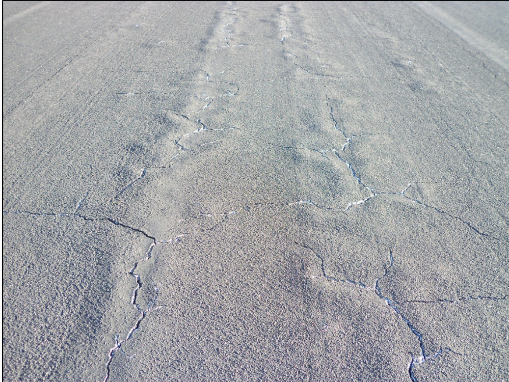
Runway 4-22, Section 6105, Sample Unit 103 – Low severity (43) Block cracking, High severity (48) Longitudinal and Transverse Cracking, Low severity (56) Swell
