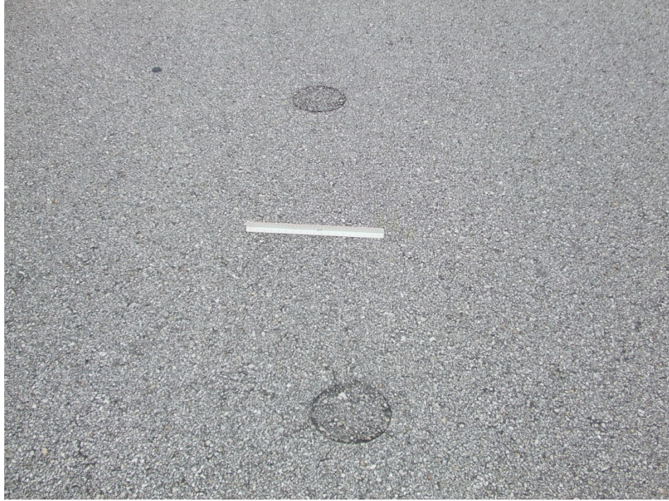
Apron at T-Hangars, Section 4210, Sample Unit 402 – Low severity (50) Patching, low severity (52) Weathering and Raveling.
