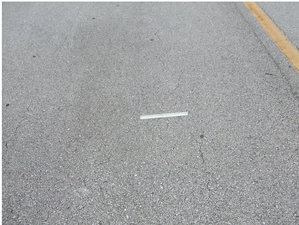
Apron at T-Hangars, Section 4210, Sample Unit 202 – Low severity (48) Longitudinal and Transverse Cracking, low severity (52) Weathering and Raveling.
