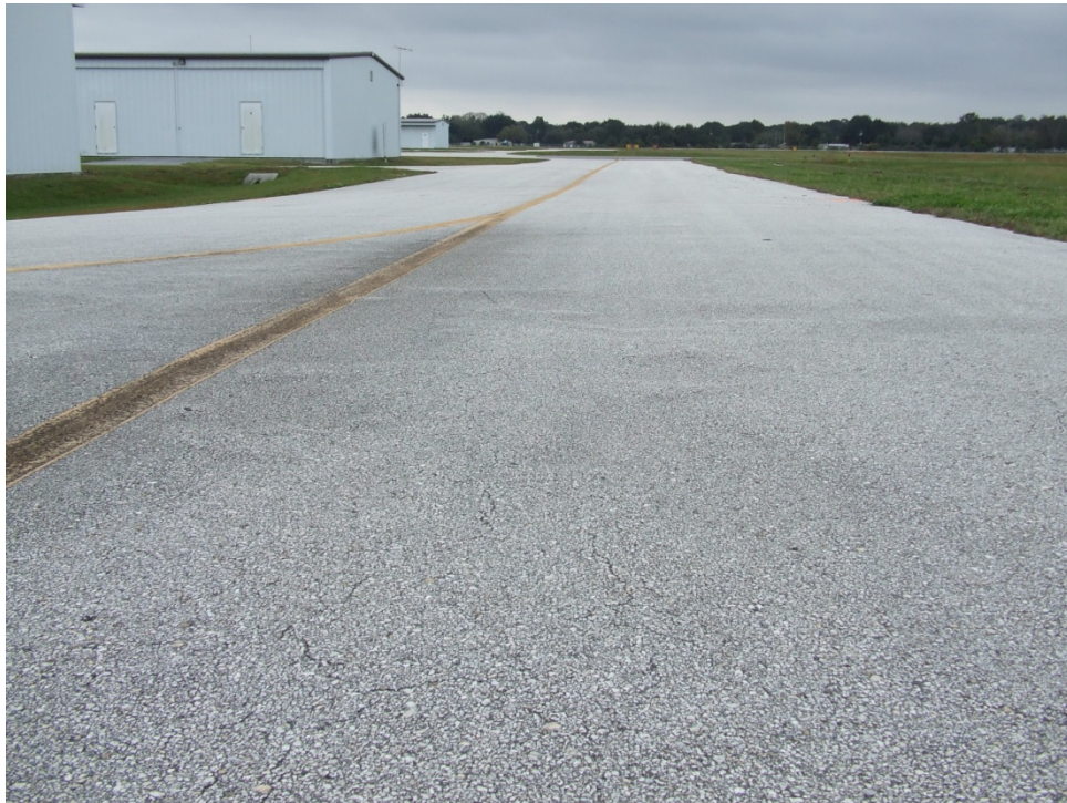
Apron at T-Hangars, Section 4205, Sample Unit 302 – Low severity (45) Depression, low severity (52) Weathering and Raveling, low severity (56) Swelling.
