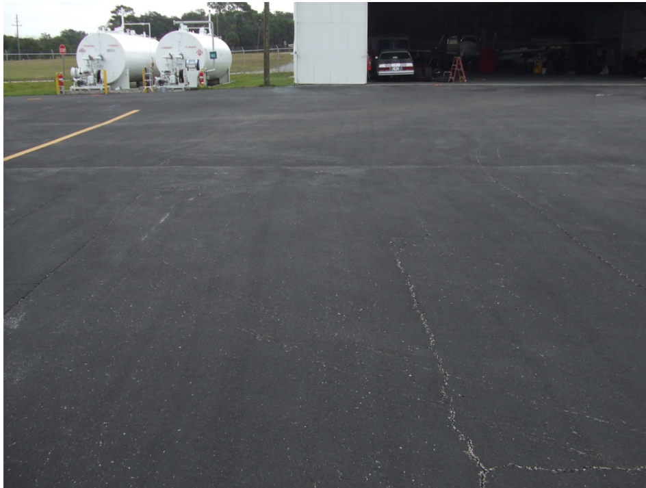
Apron, Section 4107, Sample Unit 203 – Low severity (48) Longitudinal and Transverse Cracking, low severity (52) Weathering and Raveling.
