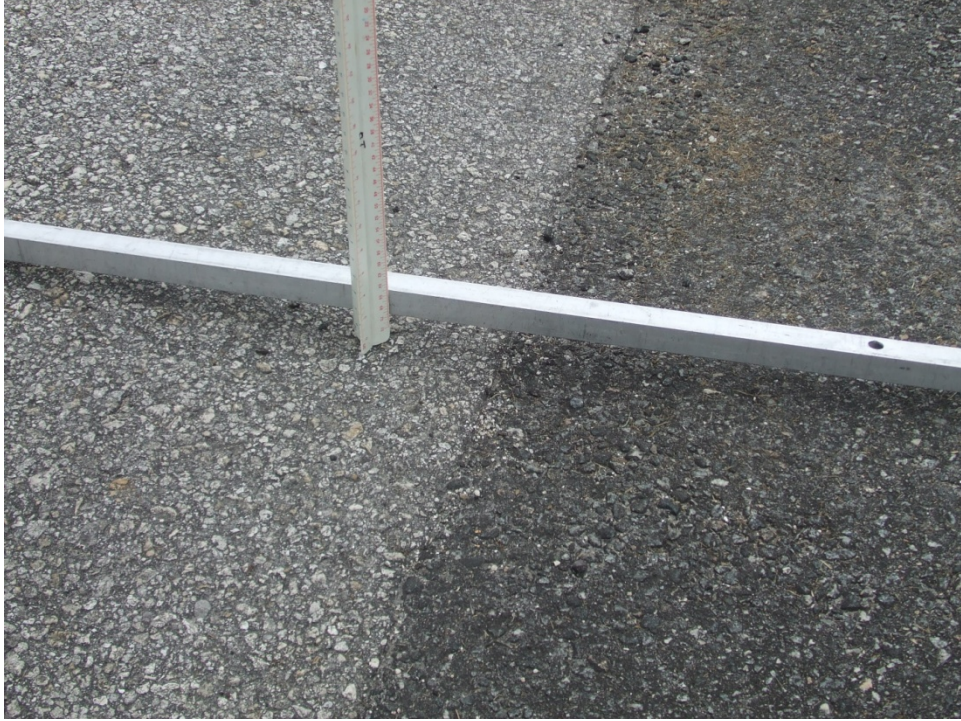
Taxiway Charlie, Section 320, Sample Unit 105 – Low severity (45) Depression, low severity (52) Weathering and Raveling.
