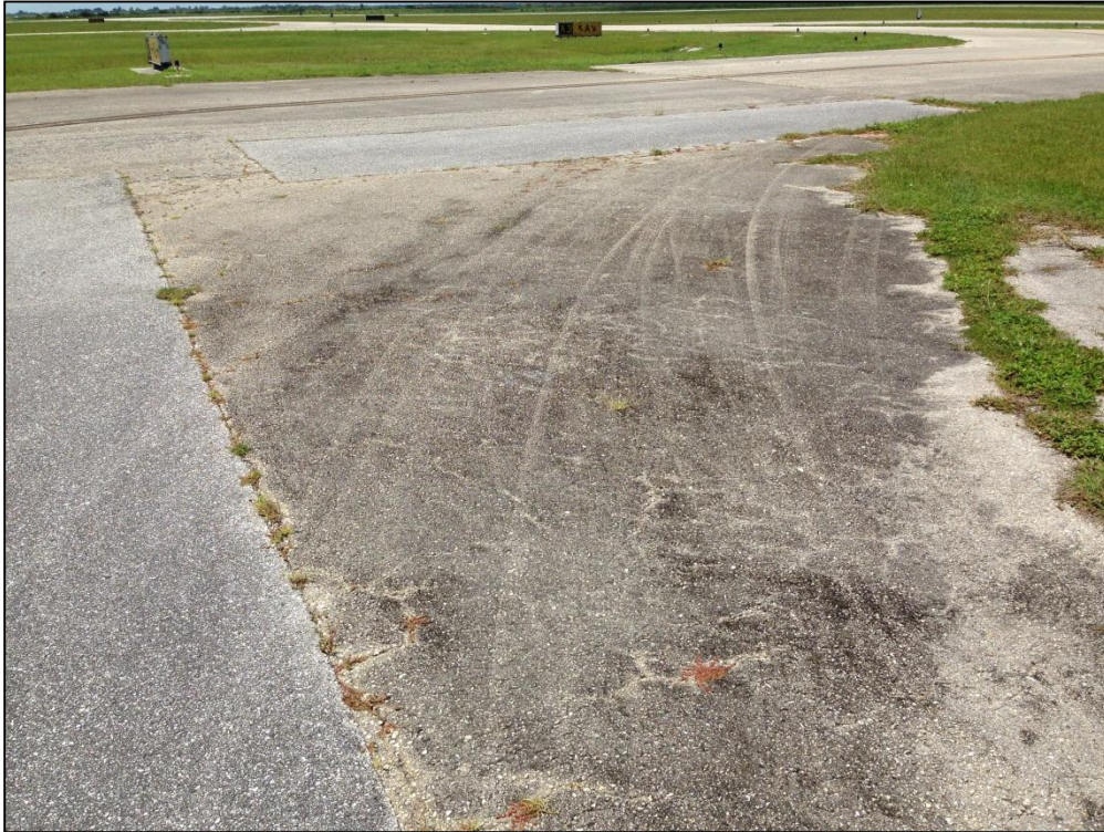
Taxiway South Apron, Section 505, Sample Unit 100 – Low Severity (48) Longitudinal and Transverse Cracking, Medium Severity (52) Raveling, Low Severity (43) Block Cracking
