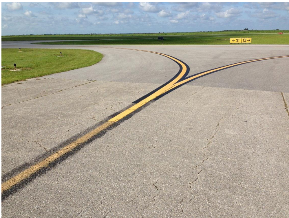
Taxiway Hangar, Section 407, Sample Unit 100 – Medium Severity (52) Raveling, Low Severity (43) Block Cracking
