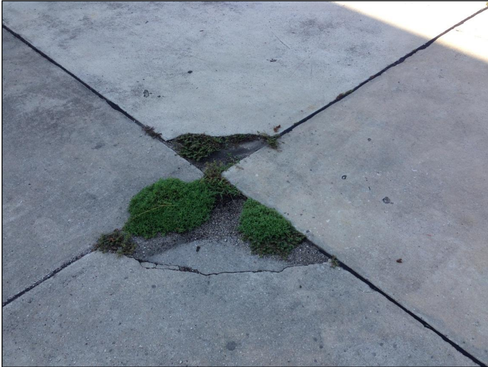
Apron Hangar, Section 4205, Sample Unit 100 – Low Severity (65) Joint Seal Damage, Medium Severity (62) Corner Break
