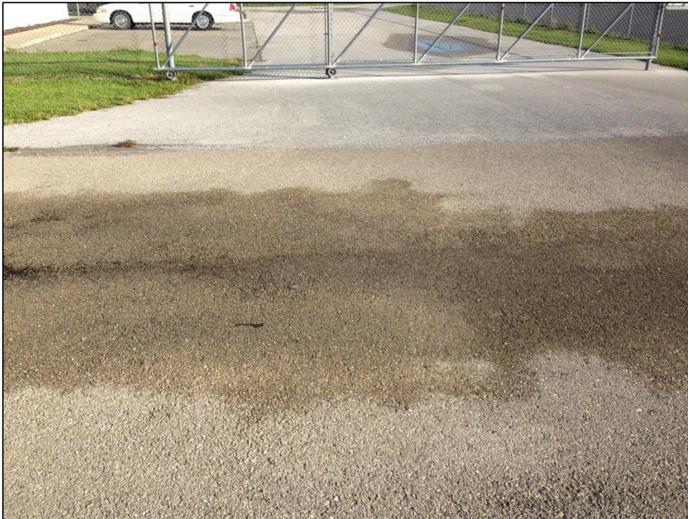
Apron South, Section 4305, Sample Unit 203 – Low Severity (48) Longitudinal and Transverse Cracking, Low and Medium Severity (52) Raveling, Low Severity (45) Depression
