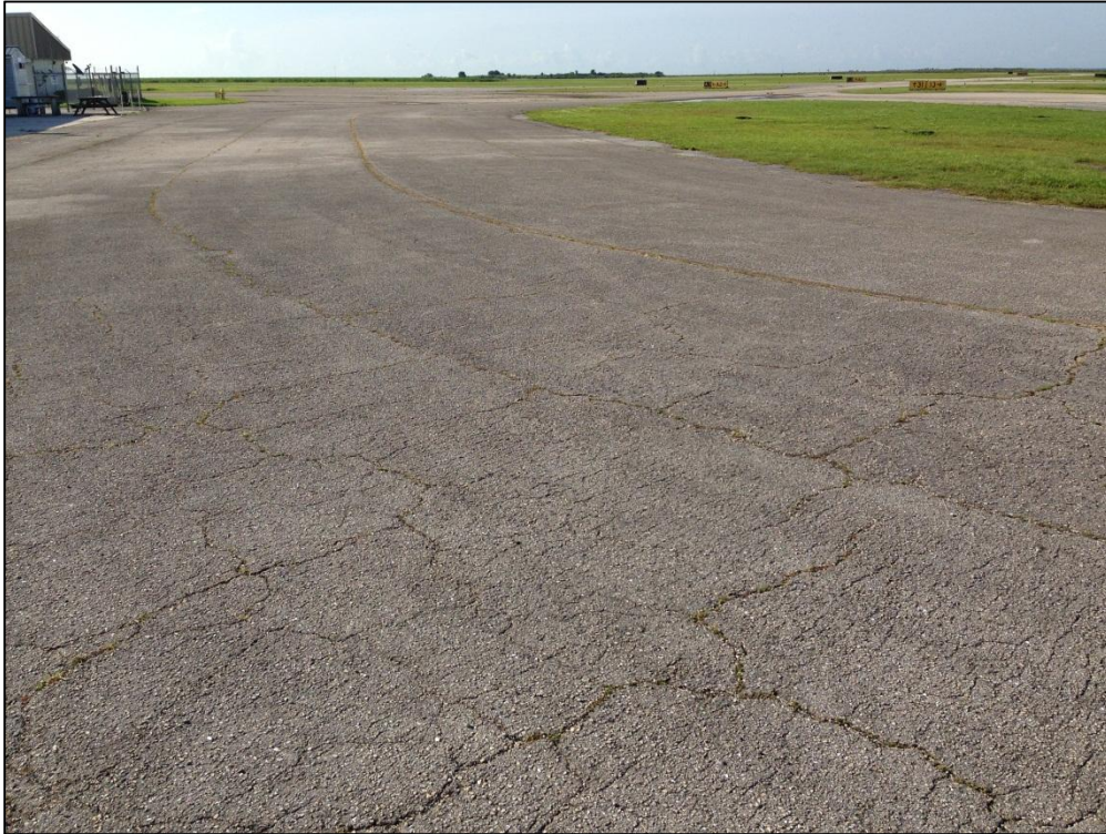
Taxiway Hangar, Section 405, Sample Unit 103 – Medium Severity (52) Raveling, Low and Medium Severity (43) Block Cracking
