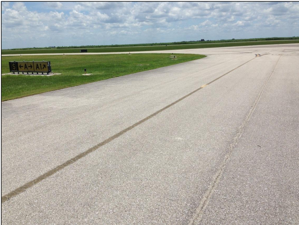
Taxiway South, Section 605, Sample Unit 101 – Low Severity (48) Longitudinal and Transverse Cracking, Low Severity (57) Weathering
