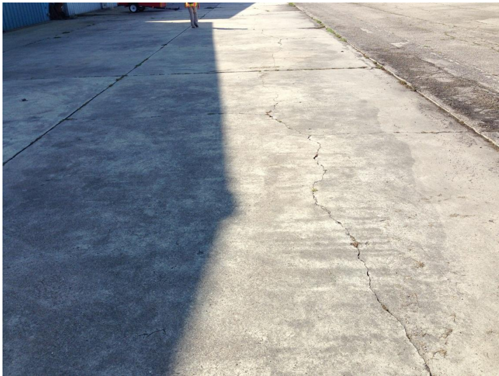
Apron Hangar, Section 4205, Sample Unit 100 – Low Severity (65) Joint Seal Damage, Low Severity (72) Shattered Slab
