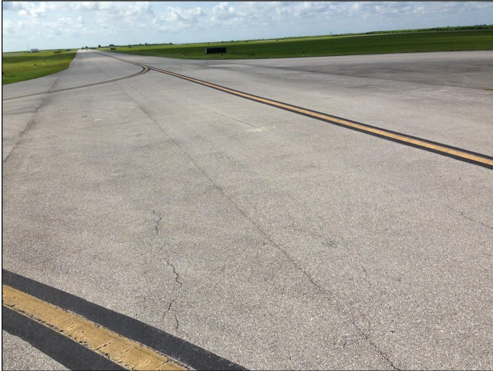
Taxiway Alpha, Section 103, Sample Unit 121 – Low Severity (48) Longitudinal and Transverse Cracking, Low Severity (57) Weathering, Low Severity (56) Swelling
