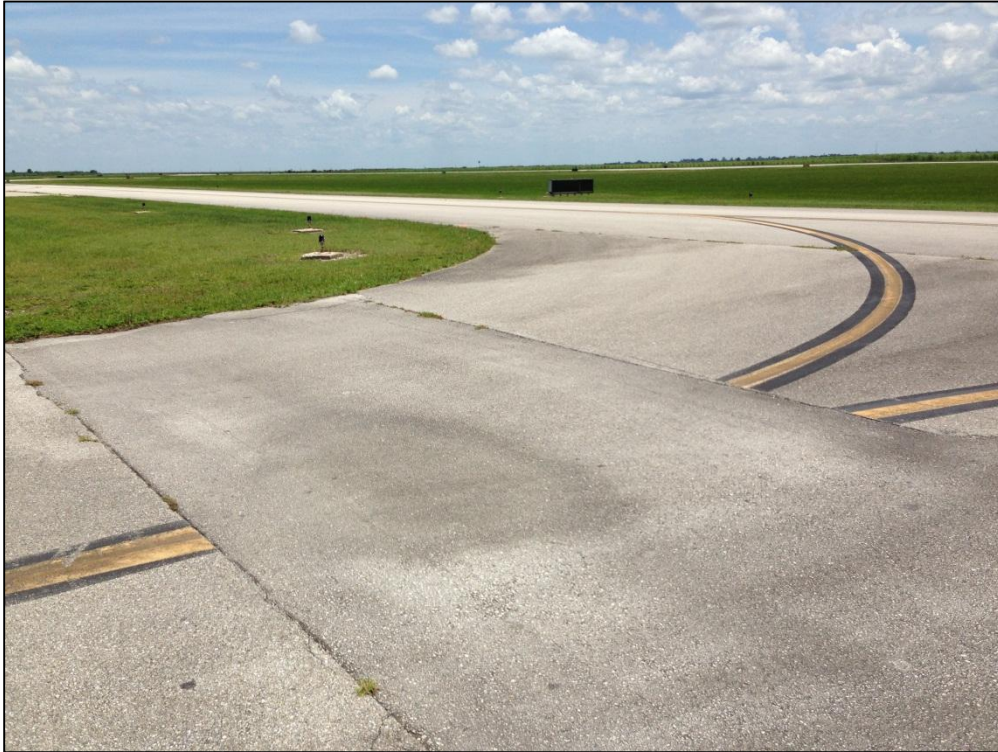
Taxiway West Apron, Section 305, Sample Unit 100 – Medium Severity (48) Longitudinal and Transverse Cracking, Medium Severity (50) Patching, Low and Medium Severity (52) Raveling
