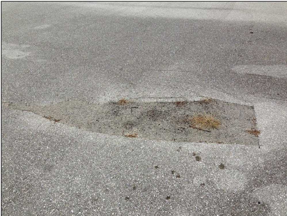
Apron West, Section 4115, Sample Unit 102 – Low Severity (48) Longitudinal and Transverse Cracking, Low Severity (57) Weathering, Low Severity (52) Raveling, High Severity (50) Patching
