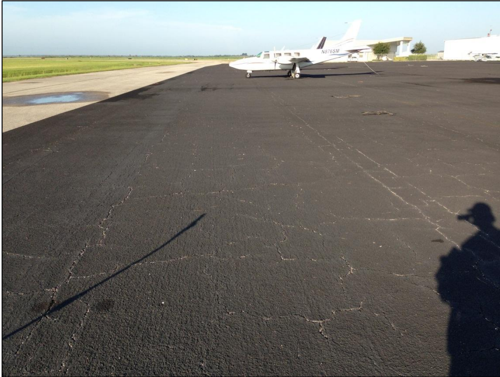
Apron East, Section 4505, Sample Unit 503 – Low Severity (52) Raveling, Low and Medium Severity (43) Block Cracking
