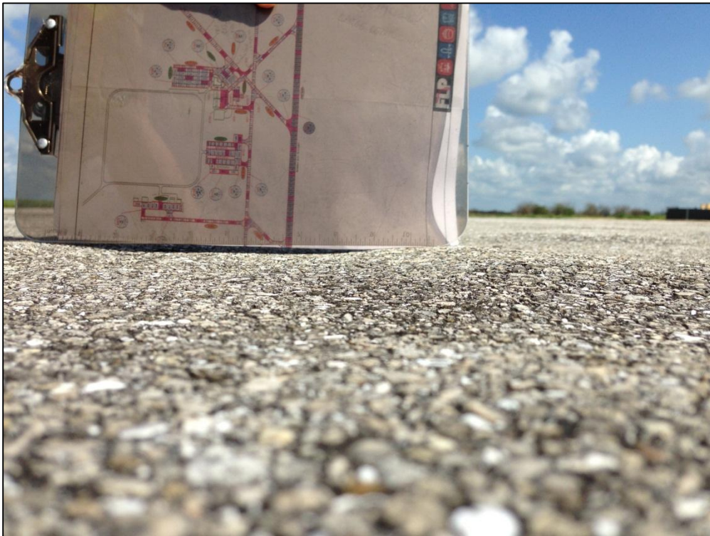
Taxiway Alpha, Section 103, Sample Unit 121 – Low Severity (57) Weathering, Low Severity (56) Swelling
