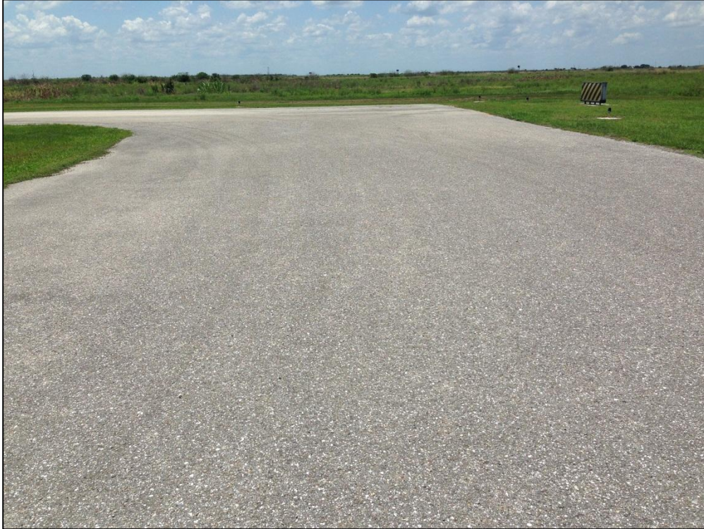
Apron North West, Section 4405, Sample Unit 201 – Medium Severity (52) Raveling
