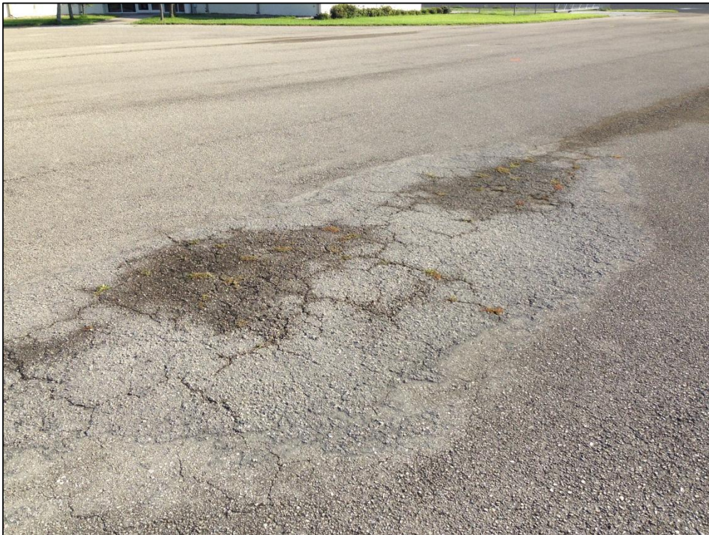
Apron South, Section 4305, Sample Unit 201 – Low and Medium Severity (48) Longitudinal and Transverse Cracking, Low and Medium Severity (52) Raveling, High Severity (50) Patching
