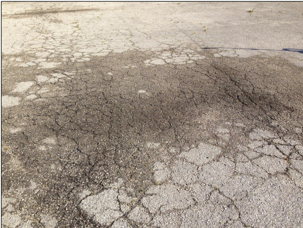
Taxiway Hangar, Section 405, Sample Unit 103 – Medium Severity (52) Raveling, Medium Severity (41) Alligator Cracking, Low and Medium Severity (43) Block Cracking, Low Severity (45) Depression
