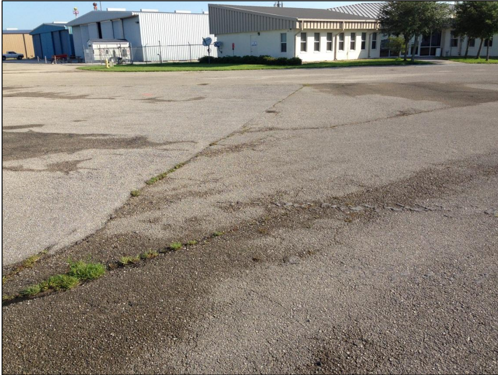
Apron South, Section 4305, Sample Unit 201 – Low and Medium Severity (48) Longitudinal and Transverse Cracking, Low and Medium Severity (52) Raveling, Low Severity (45) Depression
