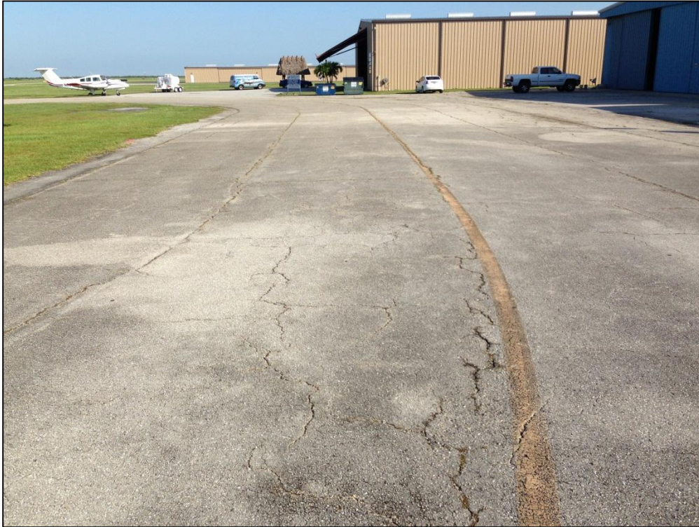
Taxiway Hangar, Section 405, Sample Unit 104 – Low Severity (48) Longitudinal and Transverse Cracking, Medium Severity (52) Raveling, Low and Medium Severity (43) Block Cracking
