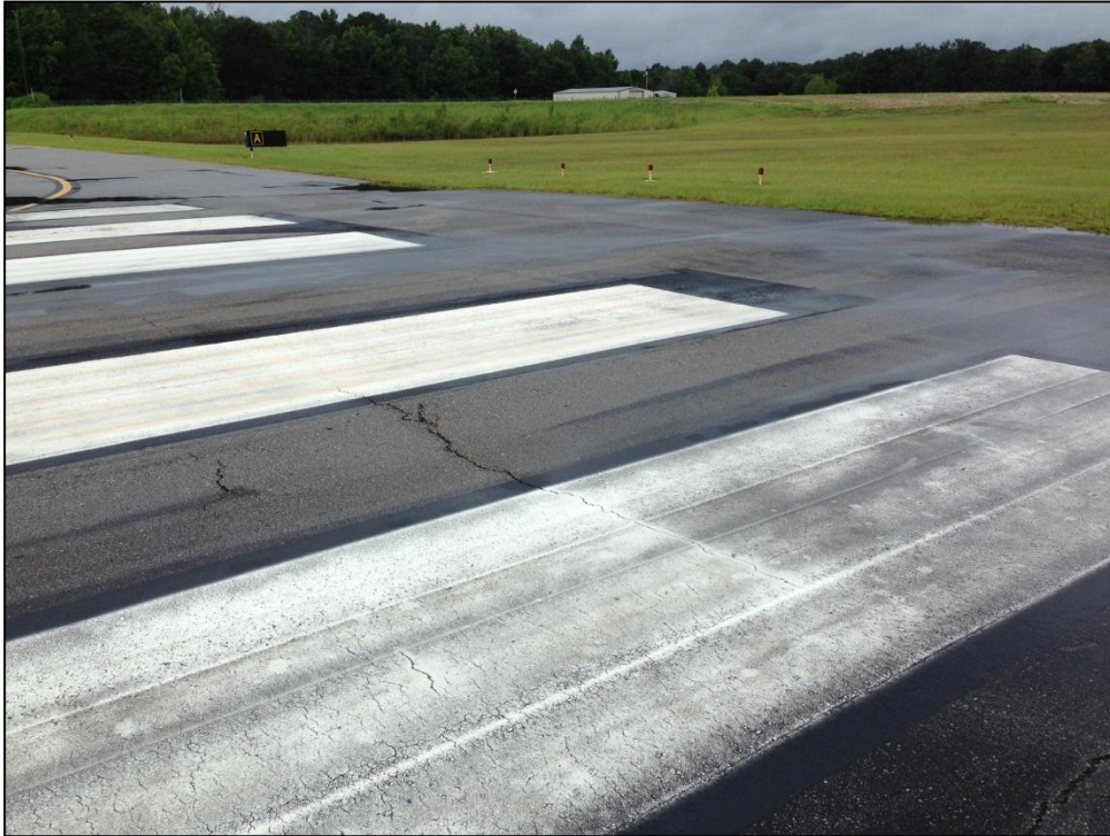
Runway 1-19, Section 6105, Sample Unit 179 – Low Severity (48) Longitudinal and Transverse Cracking, Low Severity (57) Weathering, Low Severity (52) Raveling
