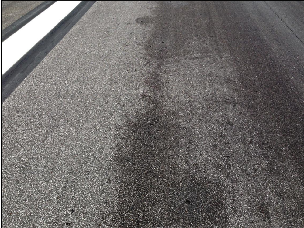
Runway 1-19, Section 6105, Sample Unit 143 – Low Severity (48) Longitudinal and Transverse Cracking, Low Severity (57) Weathering, Low Severity (52) Raveling, Low Severity (56) Swelling
