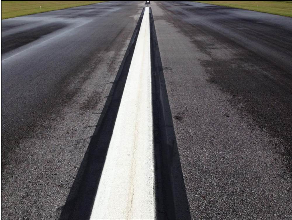
Runway 1-19, Section 6105, Sample Unit 143 – Low Severity (48) Longitudinal and Transverse Cracking, Low Severity (57) Weathering, Low Severity (52) Raveling
