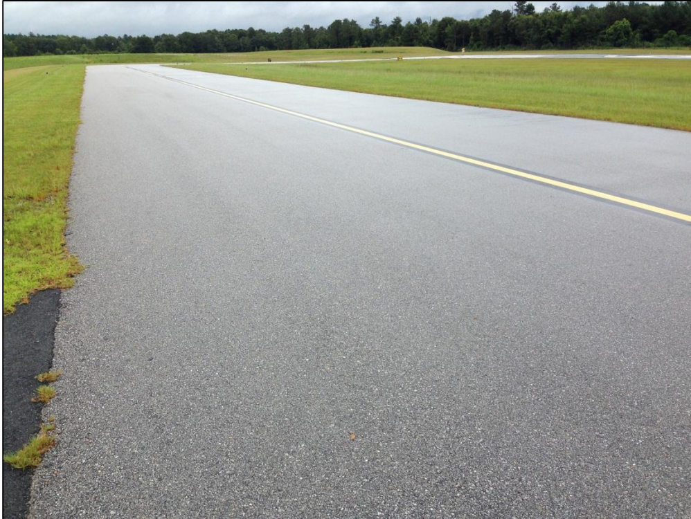
Taxiway A, Section 110, Sample Unit 101 – Low Severity (57) Weathering, Low Severity (48) Longitudinal and Transverse Cracking
