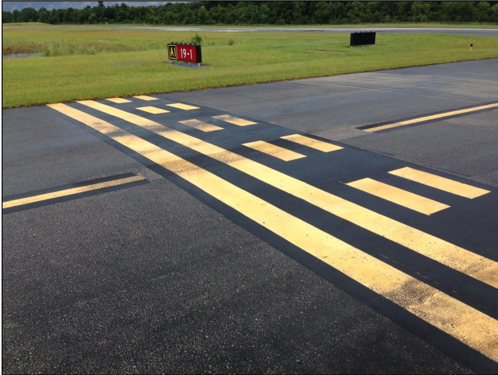
Taxiway A1, Section 105, Sample Unit 101 – Low Severity (48) Longitudinal and Transverse Cracking, Low Severity (57) Weathering, Low Severity (52) Raveling
