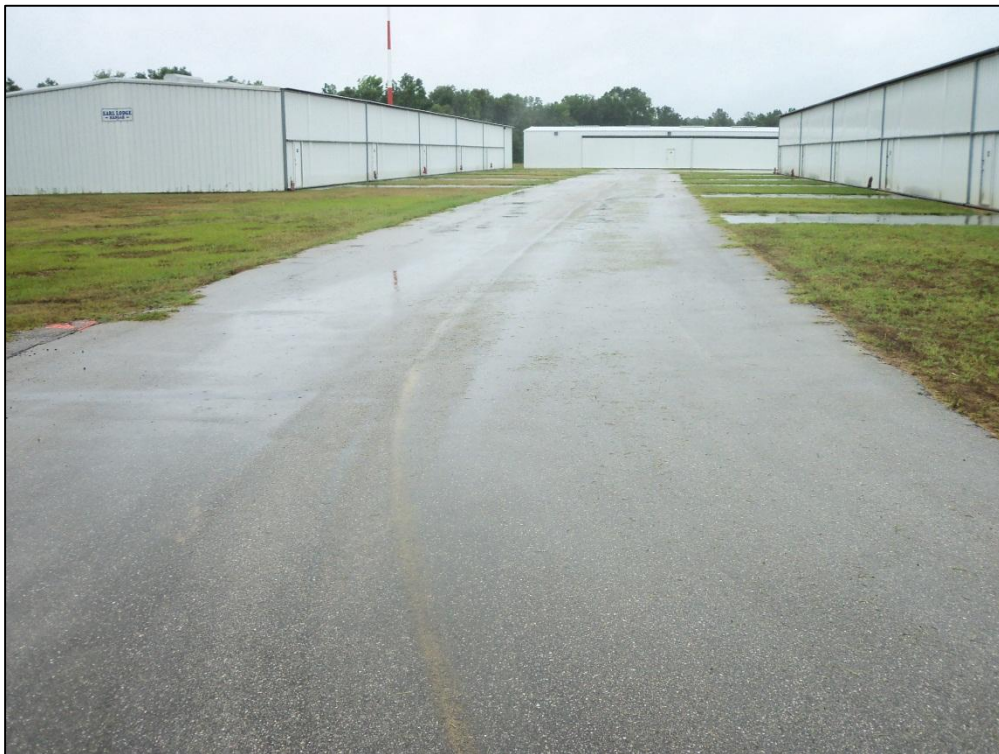
Taxiway Hangar, Section 125, Sample Unit 202 –Low Severity (57) Weathering, Low Severity (52) Raveling
