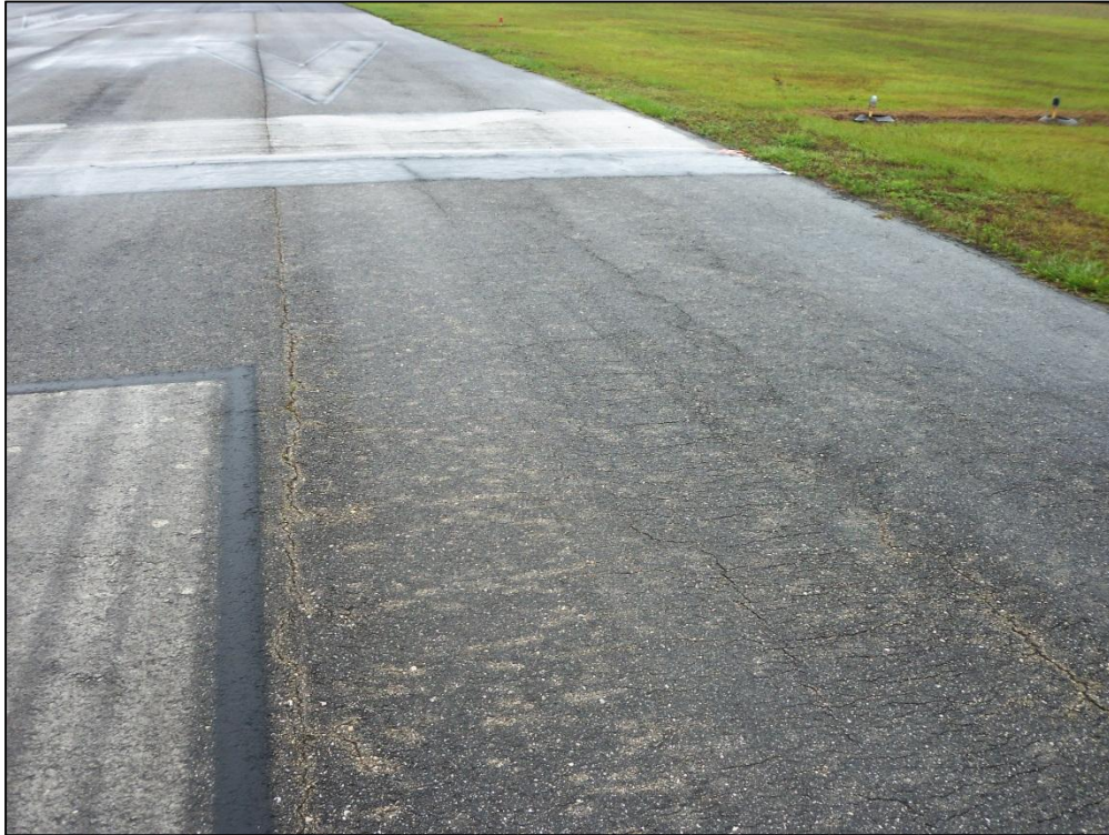
Runway 14-32, Section 6110, Sample Unit 105 – Low Severity (48) Longitudinal and Transverse Cracking, Low Severity (57) Weathering, Low Severity (52) Raveling
