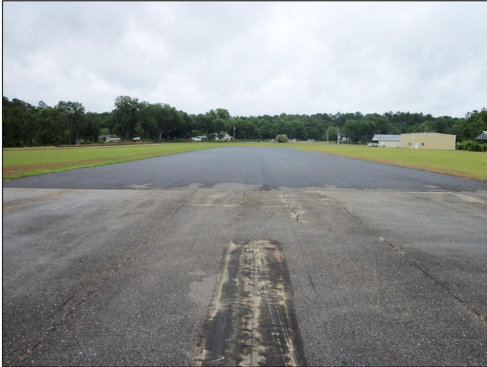
Runway 14-32, Section 6105, Sample Unit 109 – Low and Medium Severity (48) Longitudinal and Transverse Cracking, Low Severity (57) Weathering, Low Severity (52) Raveling
