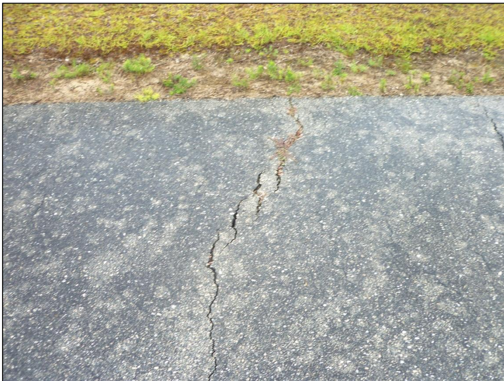
Taxiway Hangar, Section 110, Sample Unit 100 – Low and Medium Severity (48) Longitudinal and Transverse Cracking, Low Severity (57) Weathering
