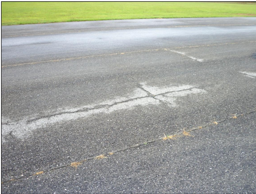
Runway 14-32, Section 6105, Sample Unit 154 – Low and Medium Severity (48) Longitudinal and Transverse Cracking, Low Severity (57) Weathering, Low Severity (52) Raveling
