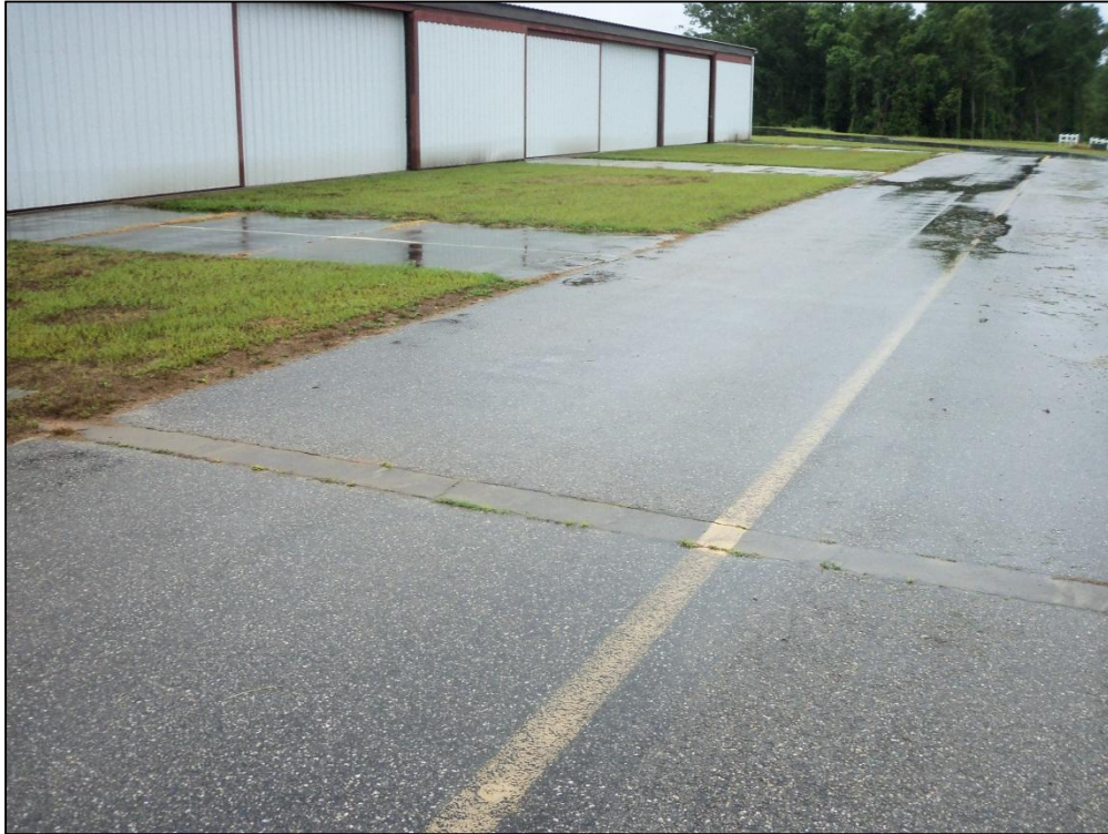
Taxiway Hangar, Section 120, Sample Unit 101 –Low Severity (57) Weathering, Low Severity (52) Raveling, Low Severity (50) Patching
