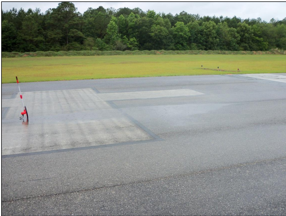
Runway 14-32, Section 6110, Sample Unit 105 – Low Severity (48) Longitudinal and Transverse Cracking, Low Severity (57) Weathering, Low Severity (52) Raveling, Low Severity (45) Depression
