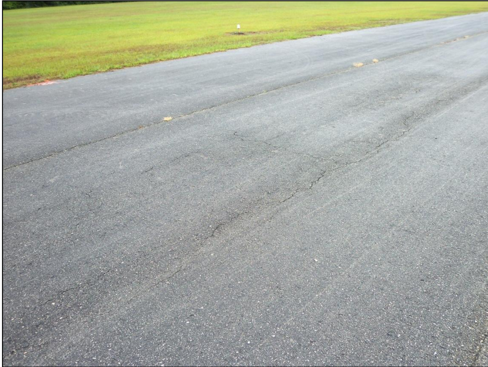
Runway 14-32, Section 6105, Sample Unit 124 – Low and Medium Severity (48) Longitudinal and Transverse Cracking, Low Severity (57) Weathering, Low Severity (52) Raveling
