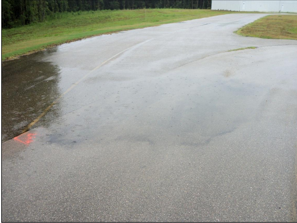
Taxiway Hangar, Section 125, Sample Unit 202 –Low Severity (57) Weathering, Low Severity (52) Raveling, Medium Severity (45) Depression
