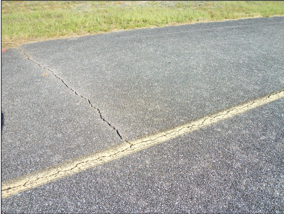
Taxiway B, Section 205, Sample Unit 117 – Low and Medium Severity (48) Longitudinal and Transverse Cracking, Medium Severity (57) Weathering
