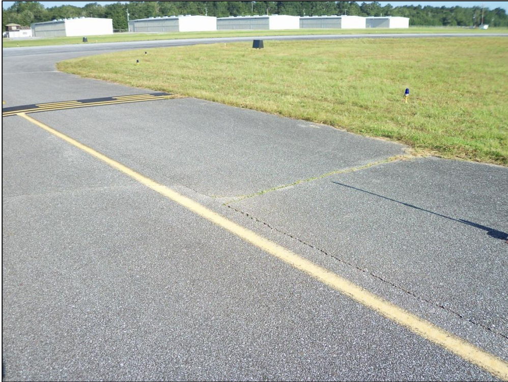
Taxiway B, Section 205, Sample Unit 120 – Low, Medium, and High Severity (48) Longitudinal and Transverse Cracking, Low Severity (57) Weathering
