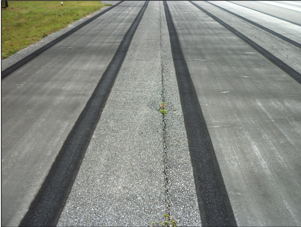
Runway 18-36, Section 6105, Sample Unit 171 – Medium Severity (48) Longitudinal and Transverse Cracking, Low Severity (57) Weathering
