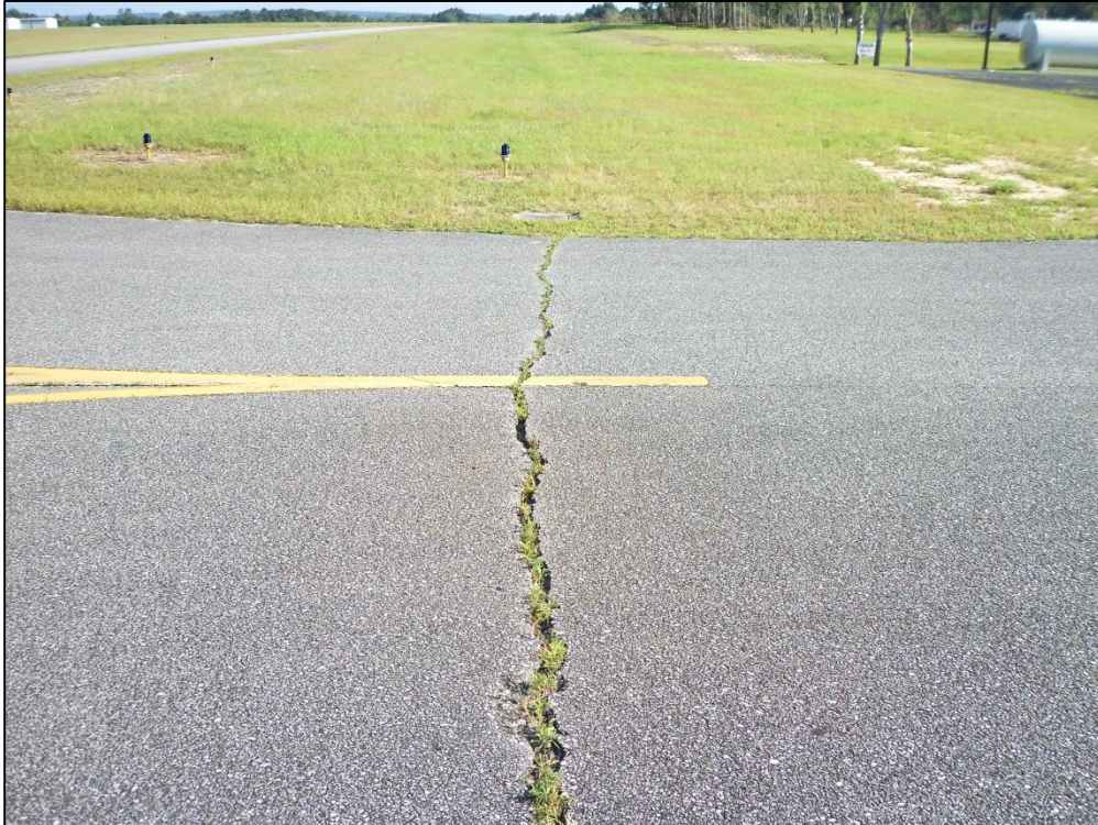
Taxiway B, Section 250, Sample Unit 200 – High Severity (48) Longitudinal and Transverse Cracking, Medium Severity (57) Weathering
