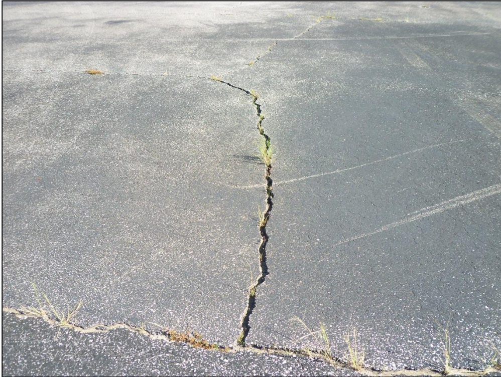
Apron, Section 4205, Sample Unit 251 – Medium and High Severity (48) Longitudinal and Transverse Cracking, Low Severity (57) Weathering
