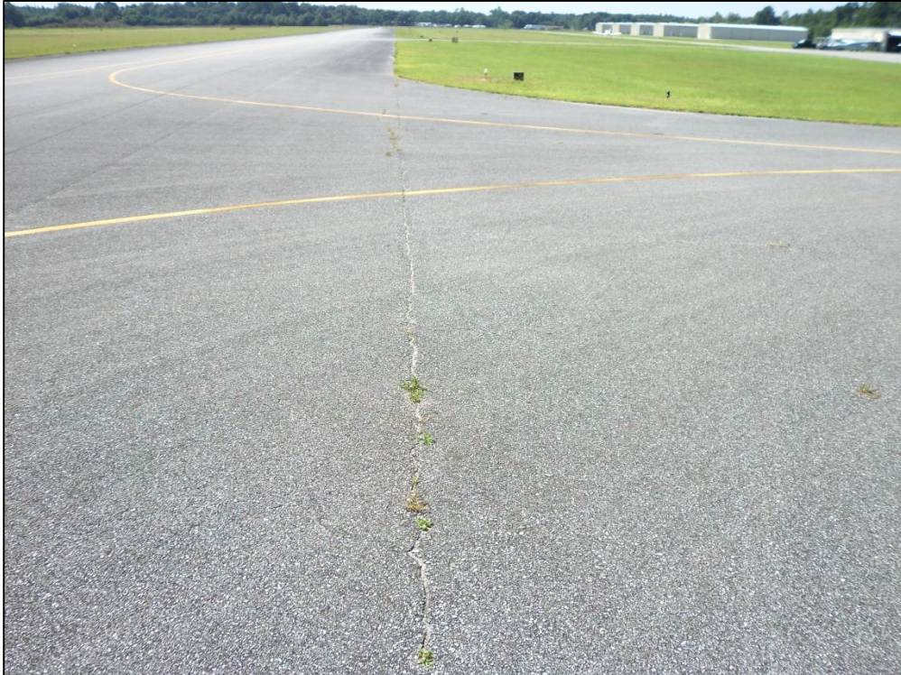
Taxiway D, Section 410, Sample Unit 400 – Medium Severity (48) Longitudinal and Transverse Cracking, Low Severity (52) Raveling, Low Severity (57) Weathering
