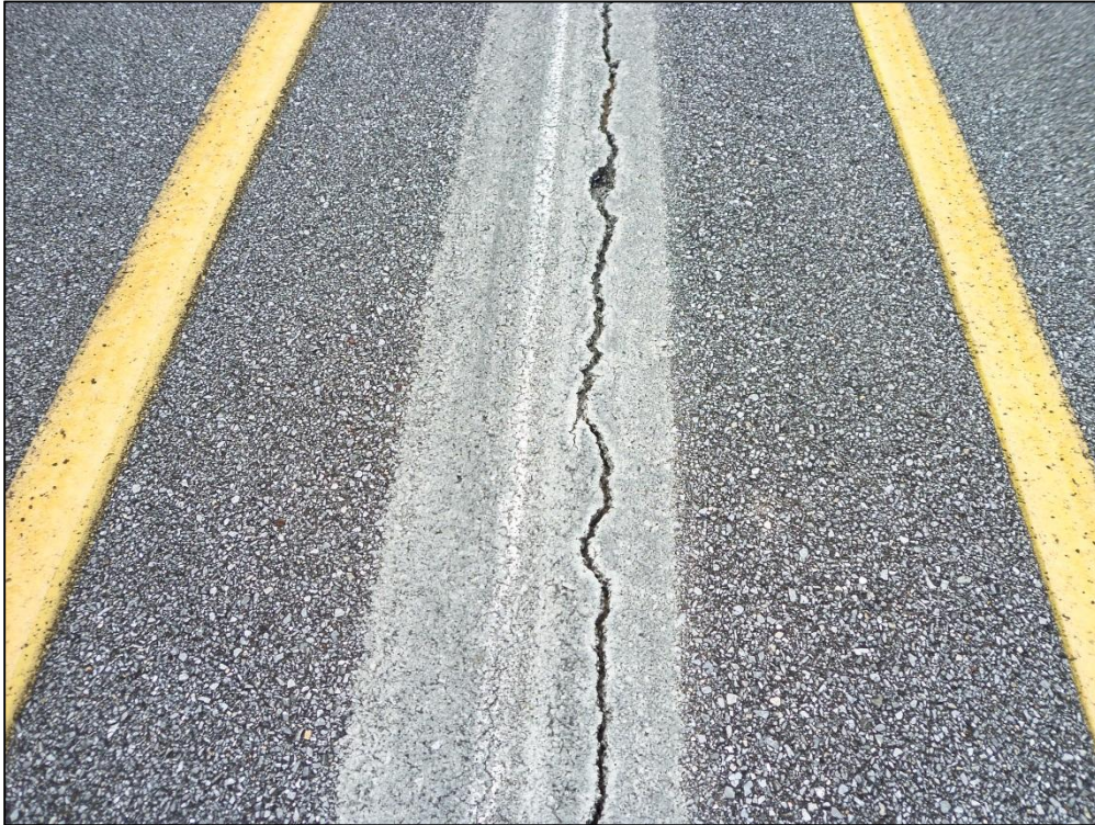
Runway 18-36, Section 6105, Sample Unit 141 – Medium Severity (48) Longitudinal and Transverse Cracking, Low Severity (52) Raveling, Low Severity (57) Weathering
