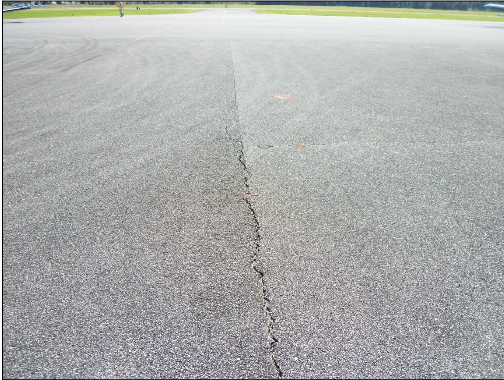
Apron, Section 4115, Sample Unit 502 – Low and Medium Severity (48) Longitudinal and Transverse Cracking, Low Severity (52) Raveling, Low Severity (57) Weathering
