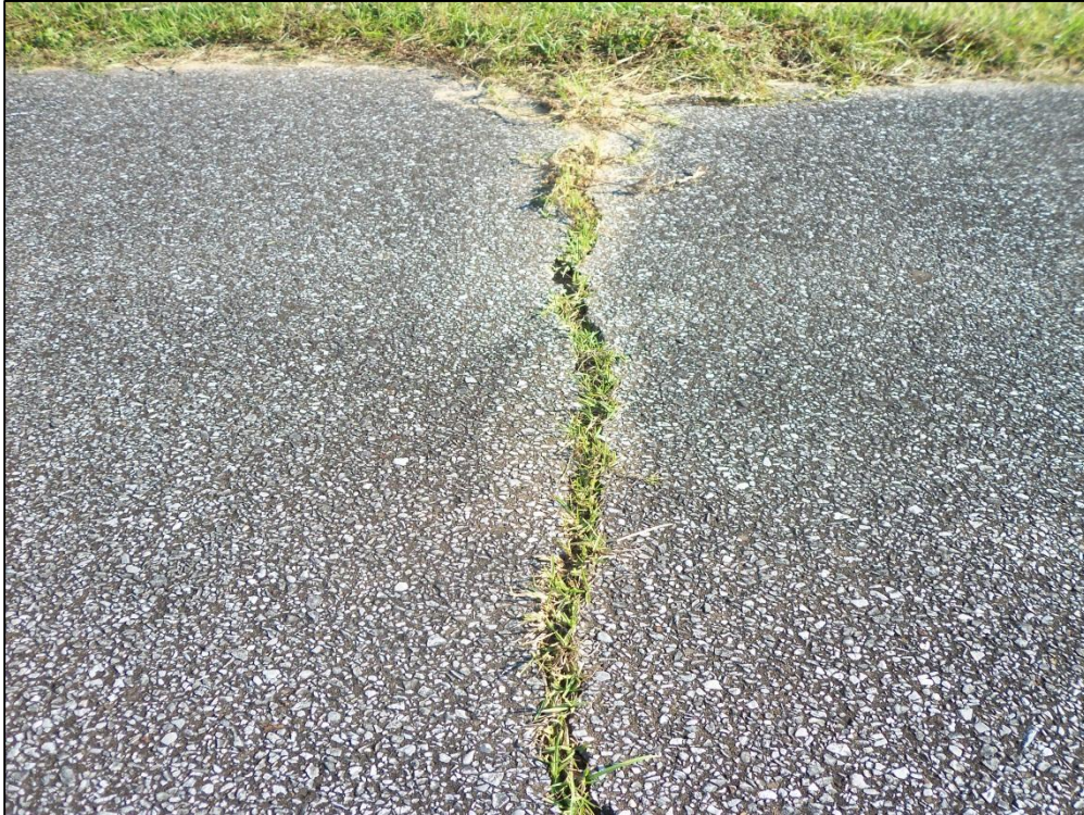
Taxiway B, Section 205, Sample Unit 120 – High Severity (48) Longitudinal and Transverse Cracking, Low Severity (57) Weathering
