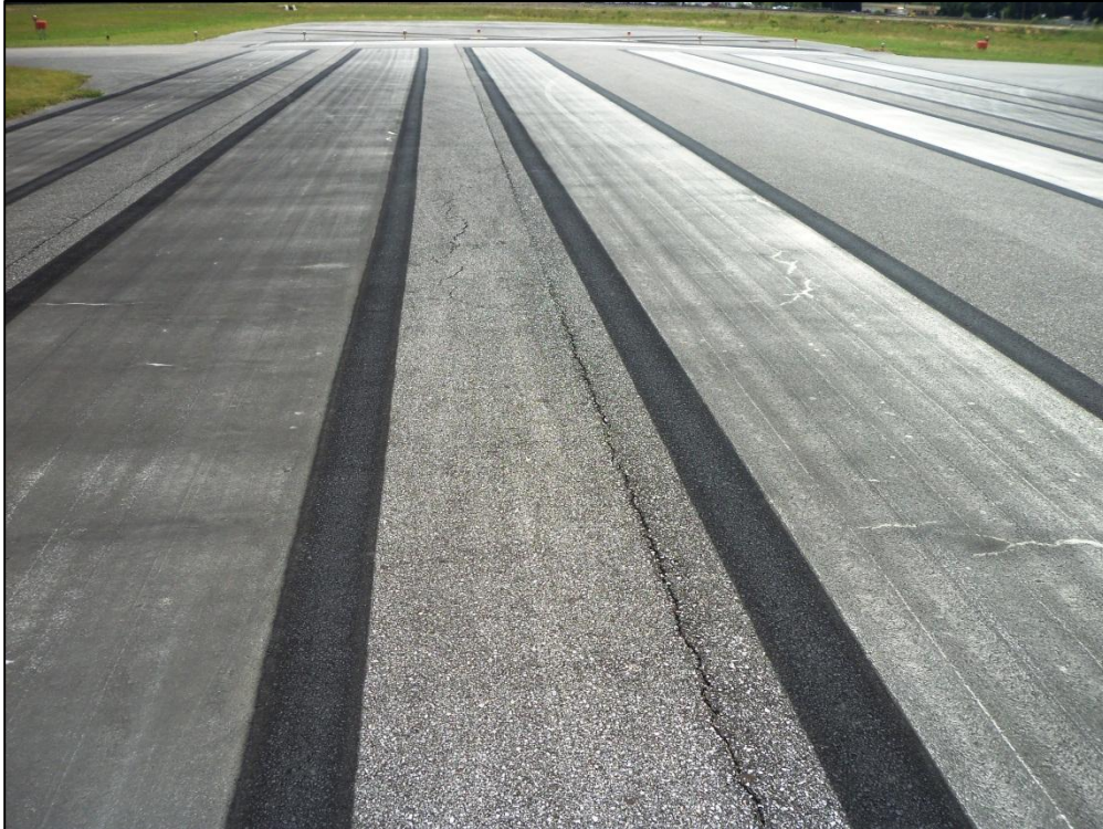
Runway 18-36, Section 6105, Sample Unit 171 – Low Severity (48) Longitudinal and Transverse Cracking, Low Severity (52) Raveling, Low Severity (57) Weathering
