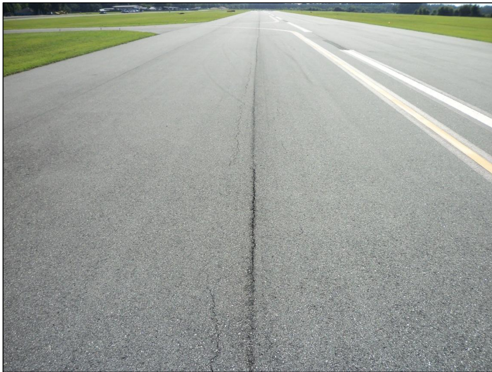
Runway 7-25, Section 6110, Sample Unit 134 – Low Severity (48) Longitudinal and Transverse Cracking
