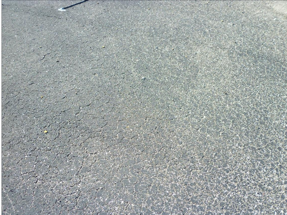
Apron, Section 4105, Sample Unit 454 – High Severity (57) Weathering
