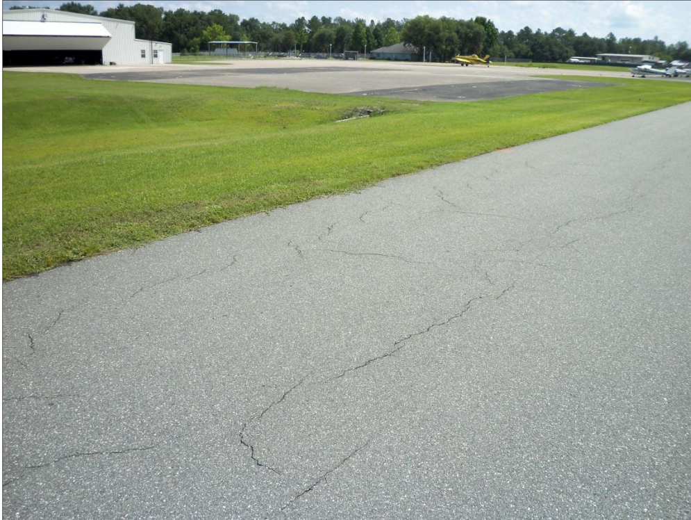
Taxiway A, Section 110, Sample Unit 117 – Low Severity (48) Longitudinal and Transverse Cracking, Low Severity (57) Weathering
