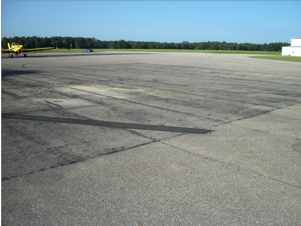
Apron, Section 4105, Sample Unit 454 – Low and Medium Severity (48) Longitudinal and Transverse Cracking, High Severity (50) Patching, Low Severity (52) Raveling, Low Severity (57) Weathering
