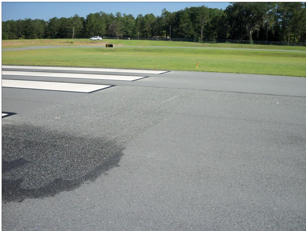
Runway 7-25, Section 6105, Sample Unit 103 – Low Severity (52) Raveling, Low Severity (57) Weathering
