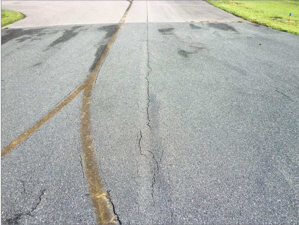
Apron Connector, Section 120, Sample Unit 100 – Low and Medium Severity (48) Longitudinal and Transverse Cracking, Low Severity (57) Weathering, Low Severity (52) Raveling, Low Severity (56) Swelling
