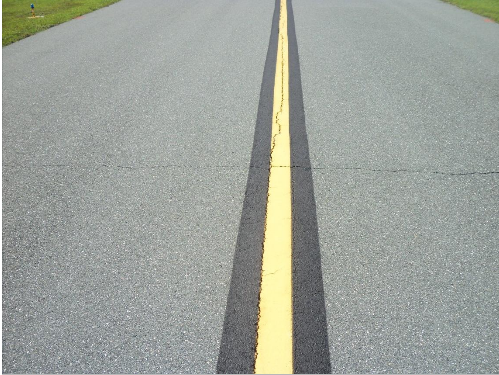
Taxiway A1, Section 115, Sample Unit 101 – Low Severity (48) Longitudinal and Transverse Cracking, Low Severity (57) Weathering
