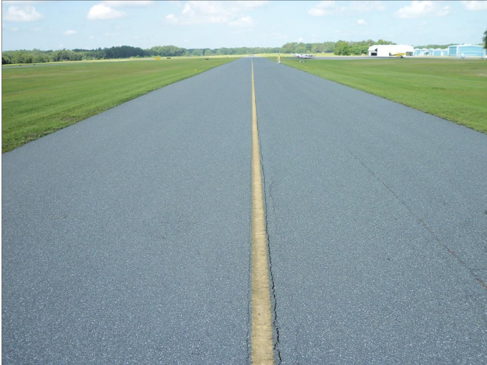
Taxiway A, Section 105, Sample Unit 104 – Low Severity (48) Longitudinal and Transverse Cracking, Low Severity (57) Weathering
