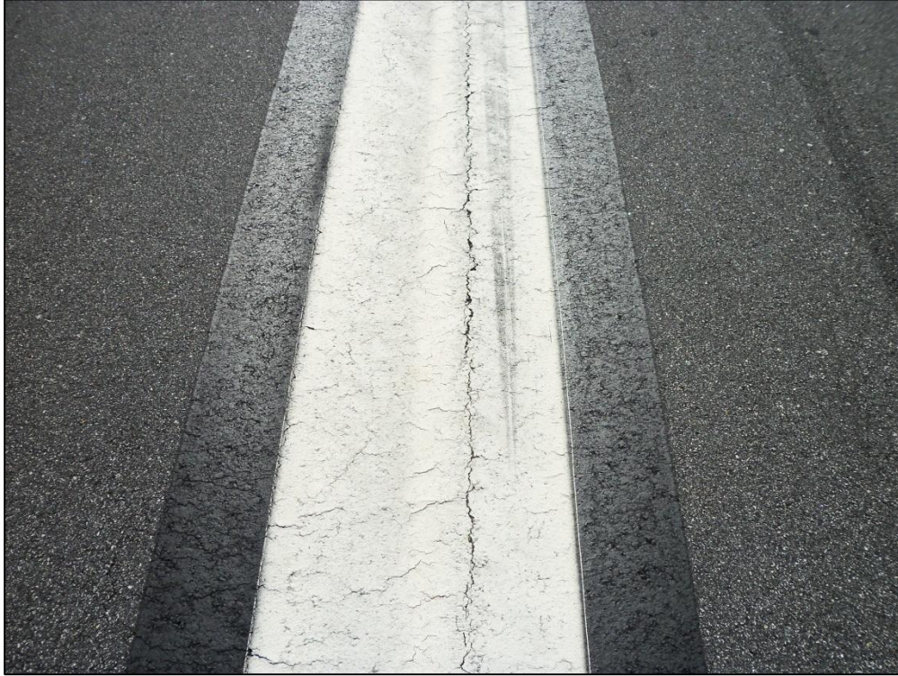
Runway 9-27, Section 6105, Sample Unit 134 – Low Severity (48) Longitudinal and Transverse Cracking
