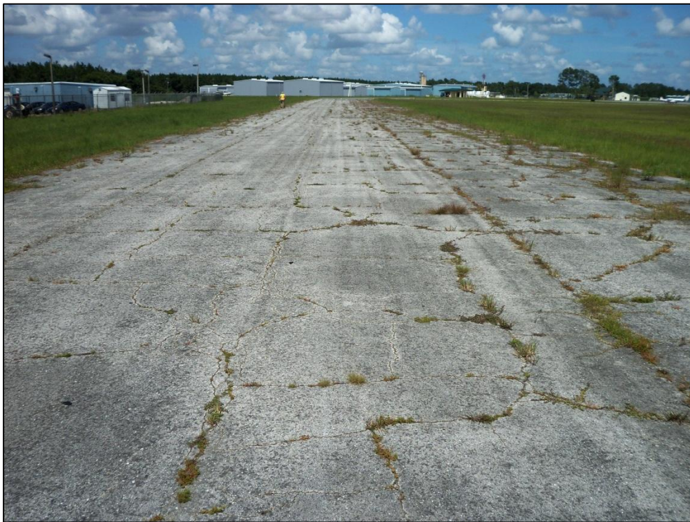
Taxiway Bravo, Section 705, Sample Unit 105 – Medium Severity (52) Raveling, Medium Severity (43) Block Cracking
