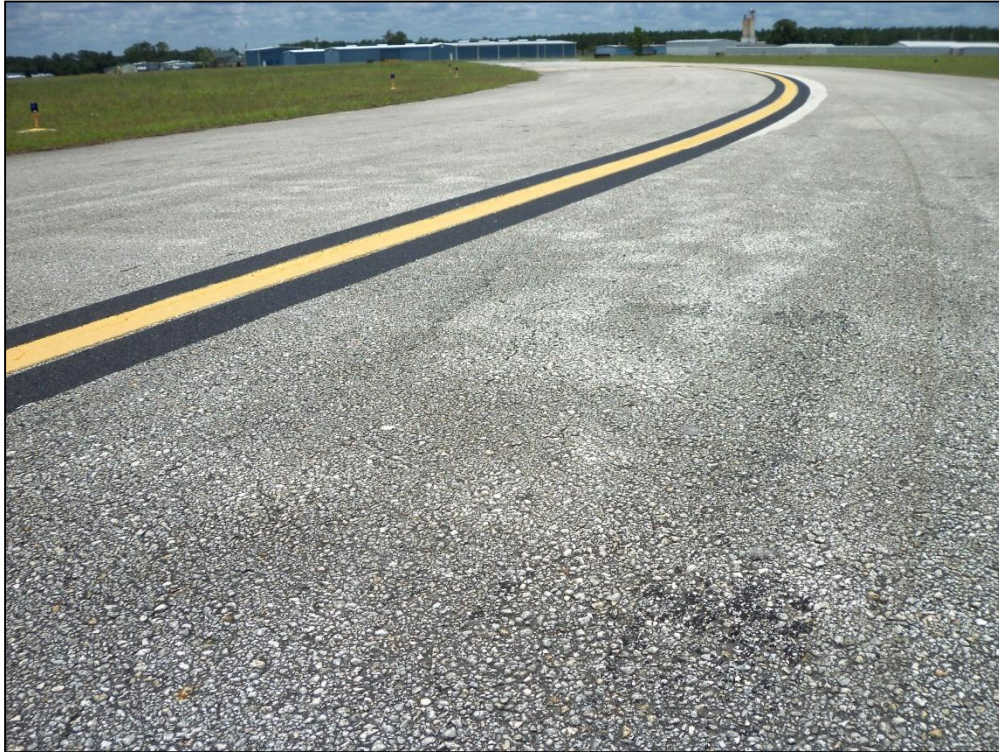
Taxiway Bravo, Section 2005, Sample Unit 101 – Low Severity (48) Longitudinal and Transverse Cracking, Low Severity (57) Weathering, Low and Medium Severity (52) Raveling, Low Severity (56) Swelling
