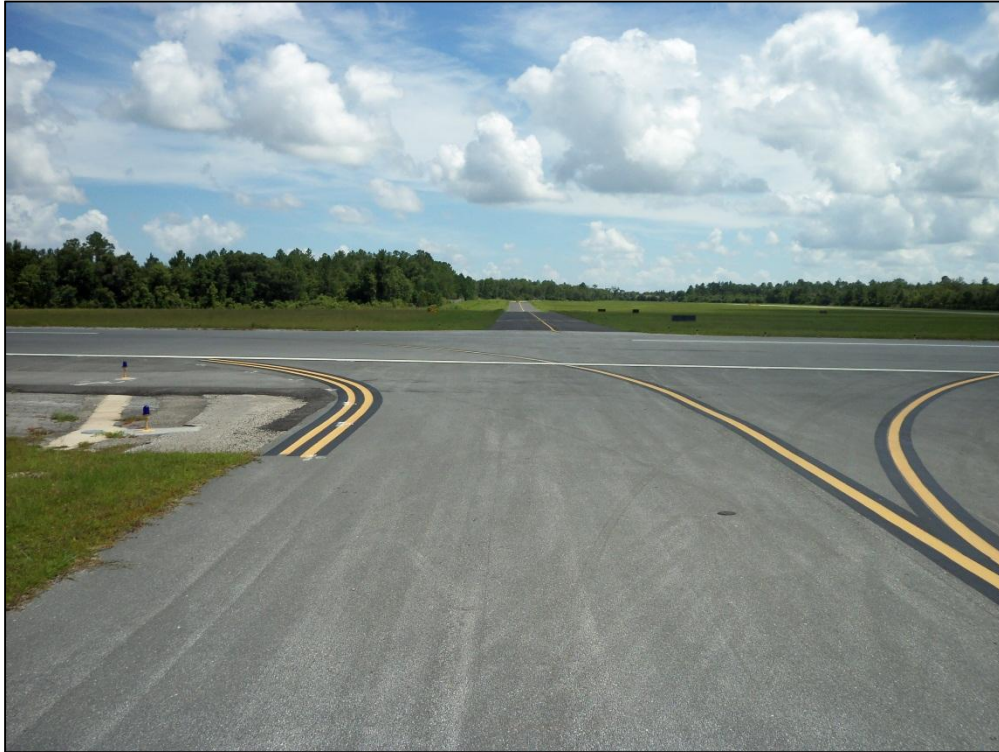
Taxiway Charlie, Section 315, Sample Unit 100 – Low Severity (57) Weathering
