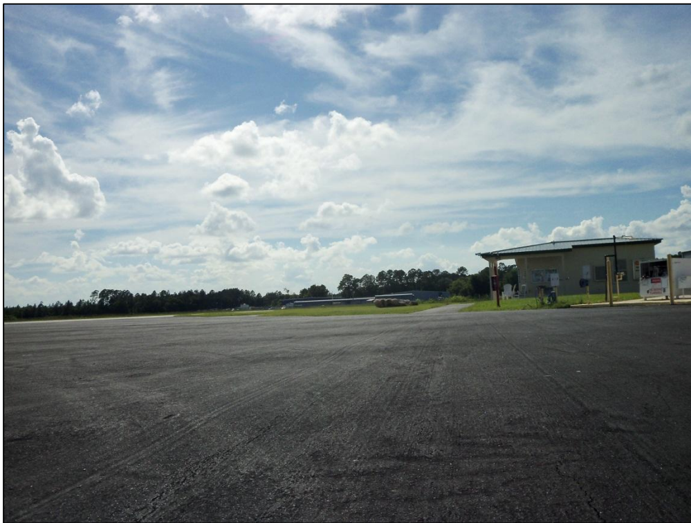
Apron North T-Hangar, Section 4215, Sample Unit 100 – Low Severity (48) Longitudinal and Transverse Cracking, Low Severity (57) Weathering, Low Severity (45) Depression
