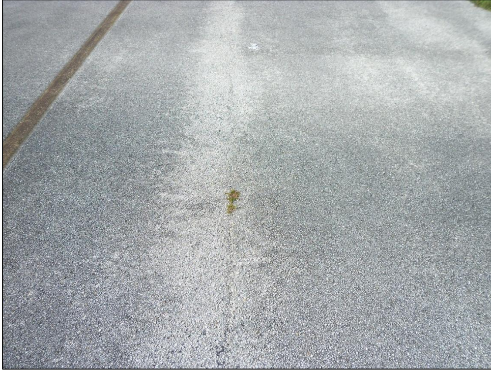
Apron North T-Hangar, Section 4205, Sample Unit 503 – Low Severity (48) Longitudinal and Transverse Cracking, Low Severity (57) Weathering, Low and Medium Severity (52) Raveling
