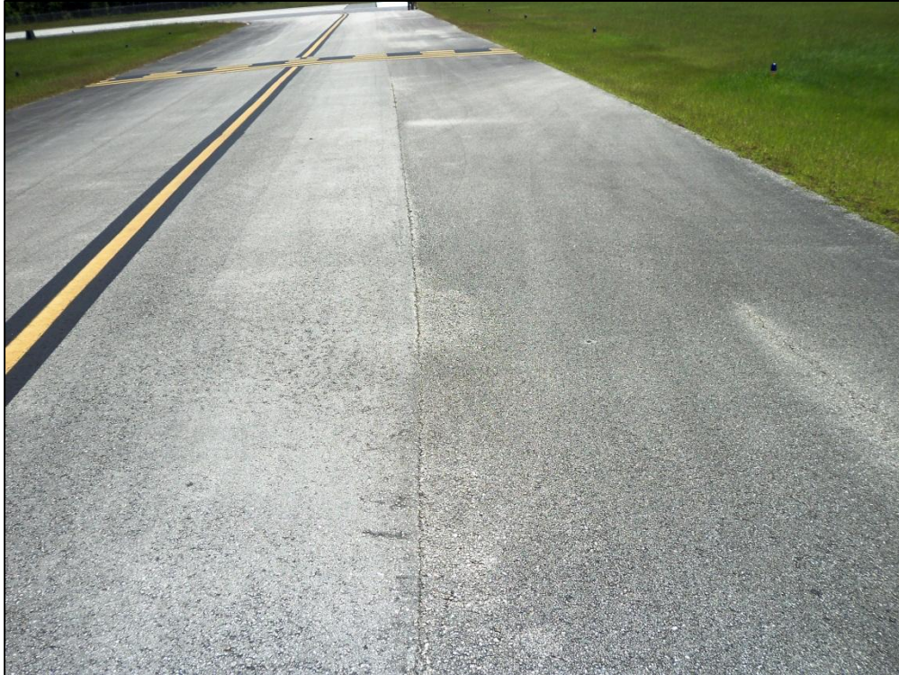
Taxiway Alpha, Section 100, Sample Unit 102 – Low Severity (48) Longitudinal and Transverse Cracking, Low Severity (57) Weathering, Low Severity (52) Raveling
