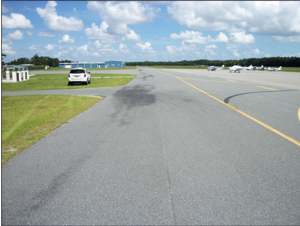
Taxiway Bravo, Section 215, Sample Unit 108 – Low Severity (57) Weathering, Bleeding (42)
