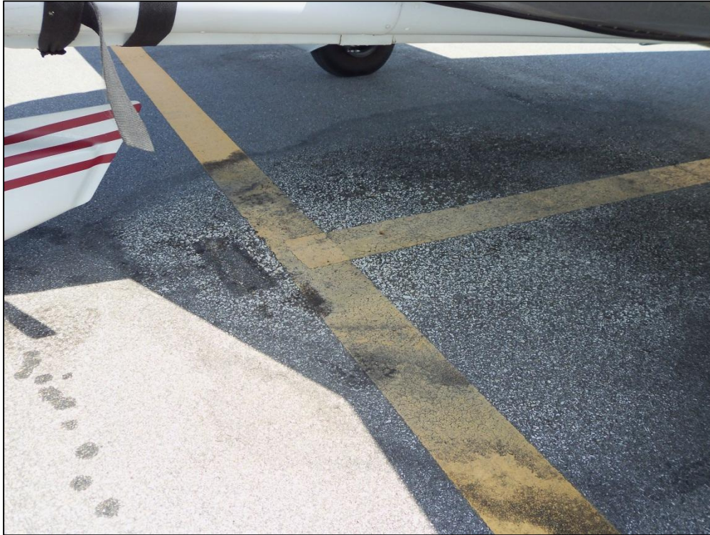
Apron, Section 4115, Sample Unit 301 – Oil Spillage (49), Low Severity (57) Weathering
