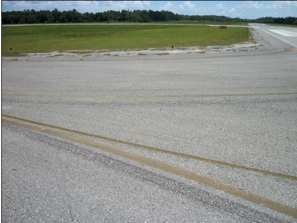
Taxiway Alpha, Section 107, Sample Unit 125 – Low Severity (48) Longitudinal and Transverse Cracking, Low Severity (57) Weathering, Low and Medium Severity (52) Raveling
