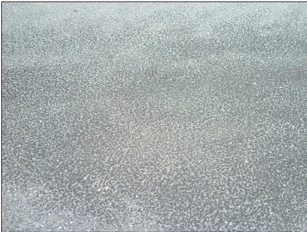
Taxiway B, Section 215, Sample Unit 108 – Bleeding (42)
