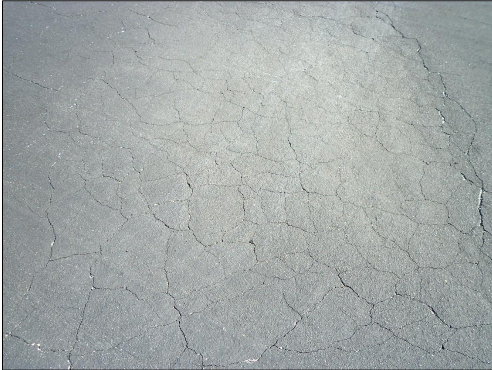
Apron North T-Hangar, Section 4215, Sample Unit 100 – Low Severity (57) Weathering, Low Severity (41) Alligator Cracking
