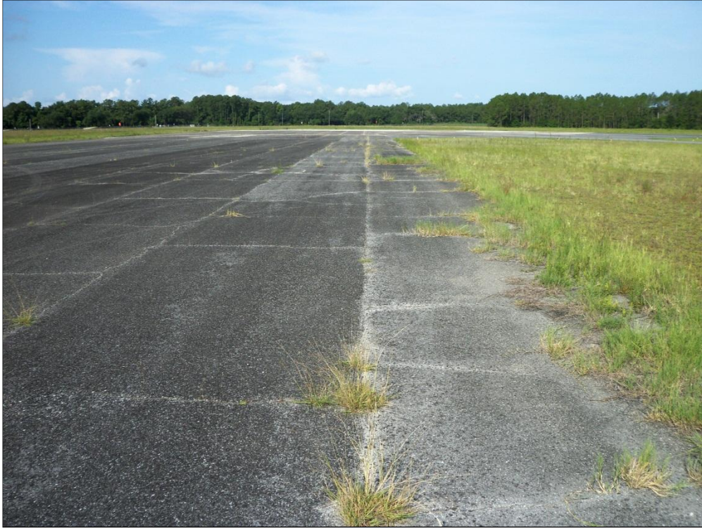
Runway 6-24, Section 6220, Sample Unit 111 – Medium Severity (52) Raveling, High and Medium Severity (43) Block Cracking
