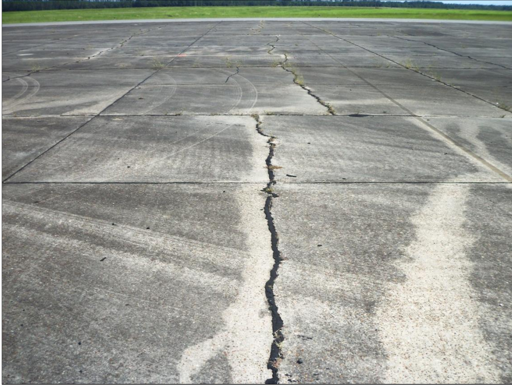
Apron, Section 4105, Sample Unit 301 - Low and Medium Severity (63) Longitudinal, Transverse and Diagonal Cracking, Medium Severity (65) Joint Seal Damage
