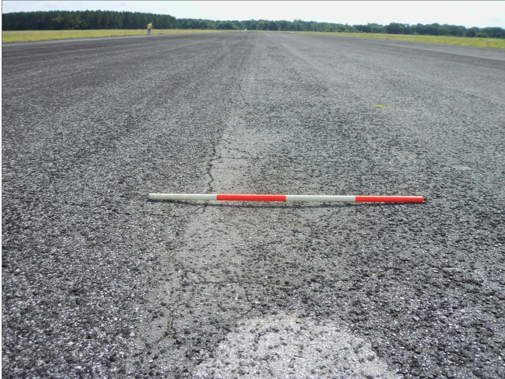
Runway 6-24, Section 6215, Sample Unit 374 – Medium Severity (52) Raveling, Low and Medium Severity (43) Block Cracking, Low Severity (45) Depression
