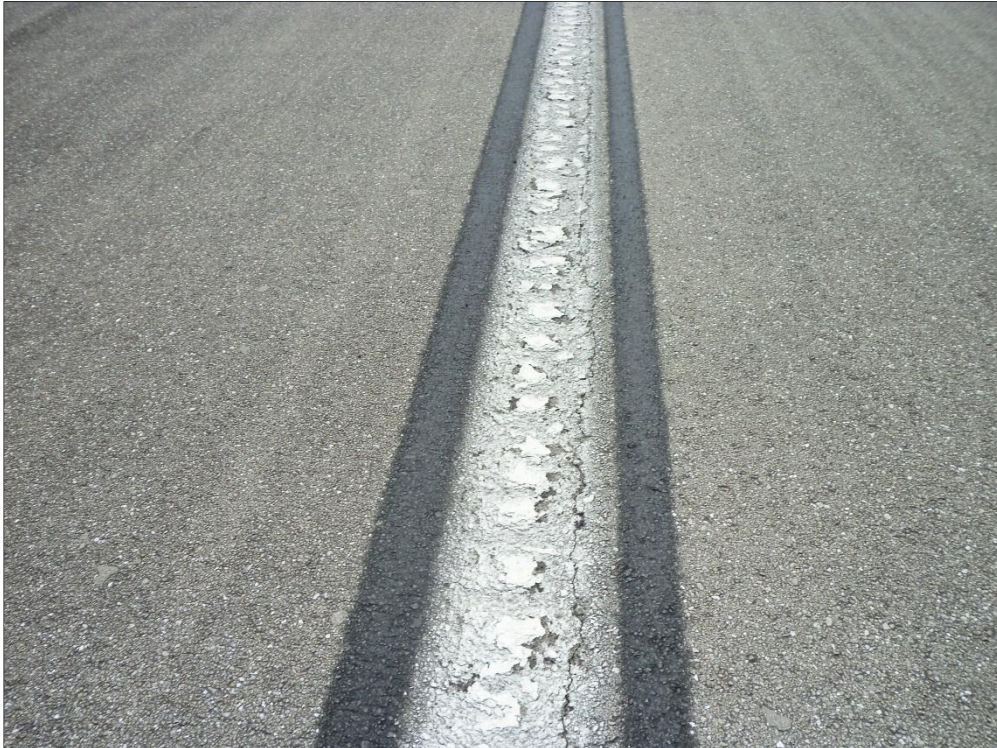
Runway 12-30, Section 6115, Sample Unit 339 – Low and Medium Severity (57) Weathering, Low Severity (48) Longitudinal and Transverse Cracking, High Severity (52) Raveling
