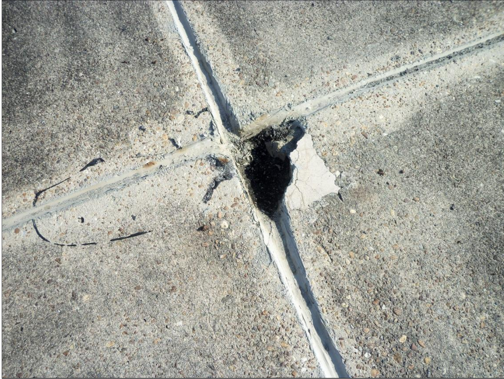
Runway 6-24, Section 6210, Sample Unit 500 – High Severity (75) Corner Spalling
