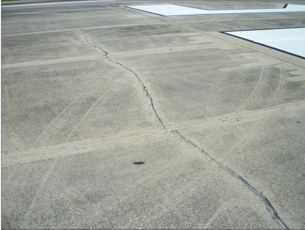
Runway 18-36, Section 6310, Sample Unit 300 – Low Severity (63) Longitudinal, Transverse, and Diagonal Cracking
