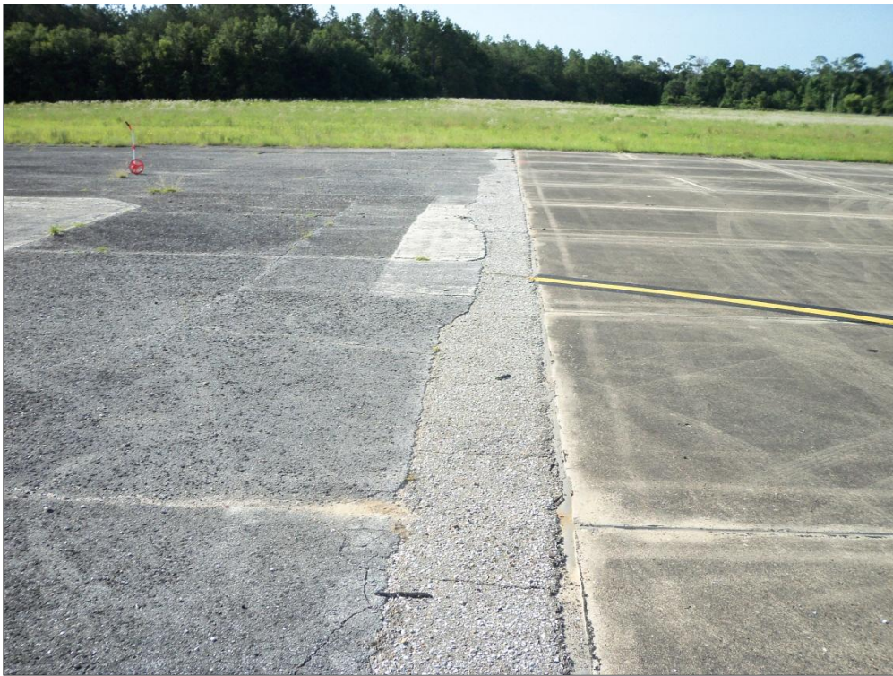
Runway 6-24, Section 6215, Sample Unit 307 – High Severity (50) Patching, Medium Severity (52) Raveling, Low and Medium Severity (43) Block Cracking
