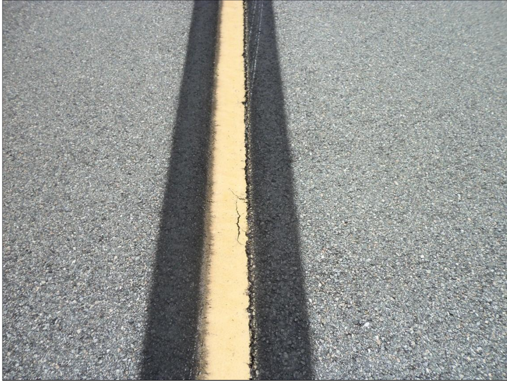
Taxiway C, Section 205, Sample Unit 119 – Low Severity (52) Raveling, Medium Severity (48) Longitudinal and Transverse Cracking, Low Severity (57) Weathering
