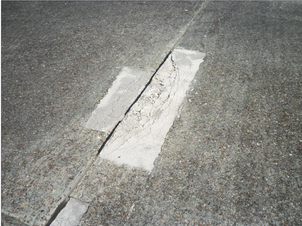
Apron, Section 4105, Sample Unit 205 - High Severity (50) Patching
