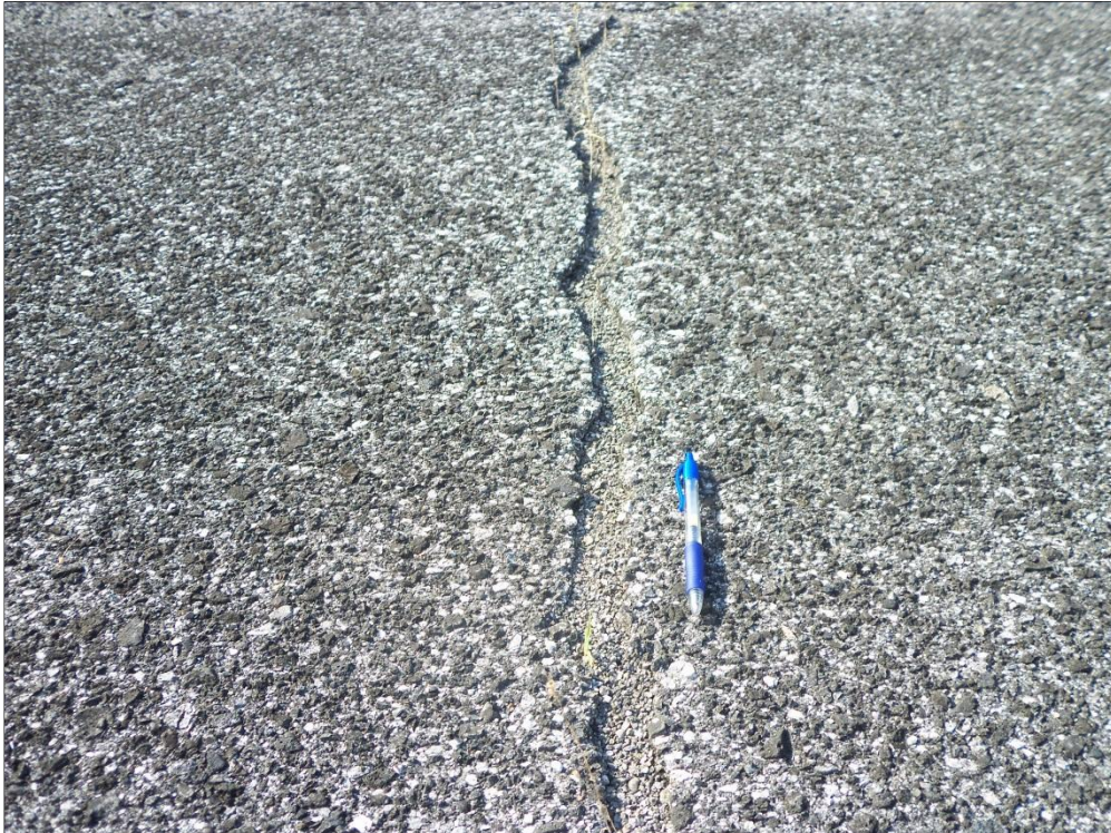
Runway 6-24, Section 6220, Sample Unit 111 – Medium Severity (52) Raveling, High Severity (43) Block Cracking
