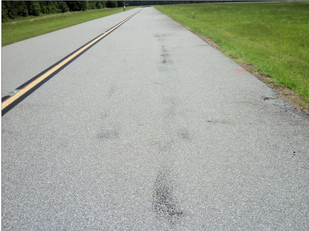
Taxiway B, Section 105, Sample Unit 120 – Low Severity (52) Raveling, (42) Bleeding, Low Severity (57) Weathering
