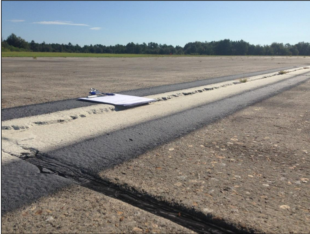
Runway 11-29, Section 6205, Sample Unit 195 – Medium Severity (65) Joint Seal Damage, Medium Severity (71) Faulting
