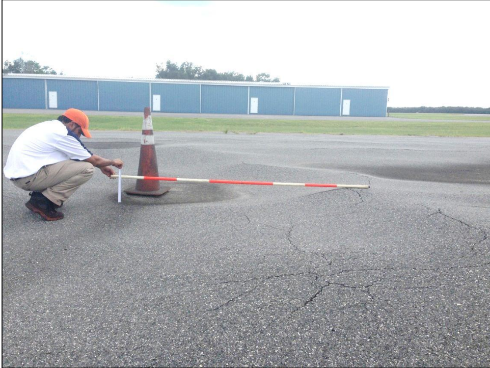
Apron T-Hang, Section 4520, Sample Unit 402 – Low Severity (48) Longitudinal and Transverse Cracking, Low Severity (57) Weathering, High Severity (56) Swelling
