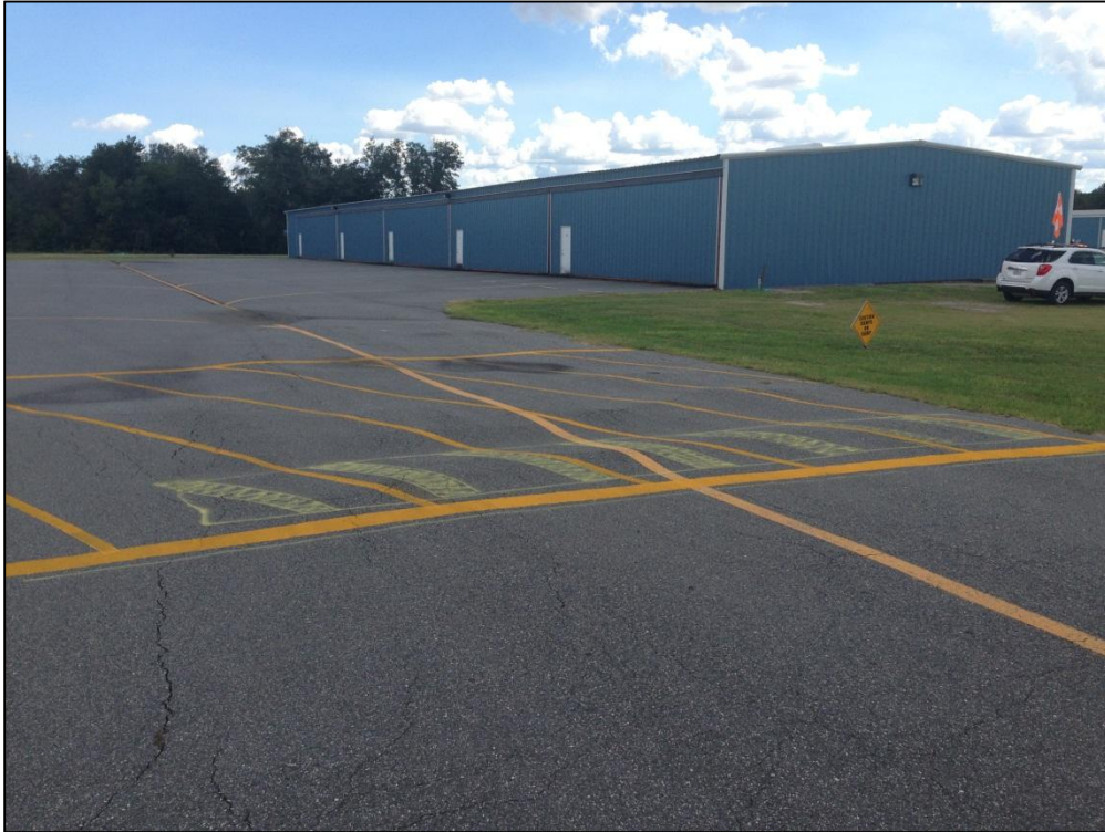
Apron T-Hang, Section 4520, Sample Unit 100 – Low Severity (48) Longitudinal and Transverse Cracking, Low Severity (57) Weathering, High Severity (56) Swelling
