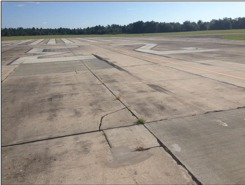
Runway 5-23, Section 6130, Sample Unit 344 – Medium Severity (65) Joint Seal Damage, Low Severity (63) Longitudinal, Transverse, and Diagonal Cracking, Low Severity (66) Small Patching, Low Severity (67) Large Patching, Low Severity (62) Corner Break, (73) Shrinkage Cracking
