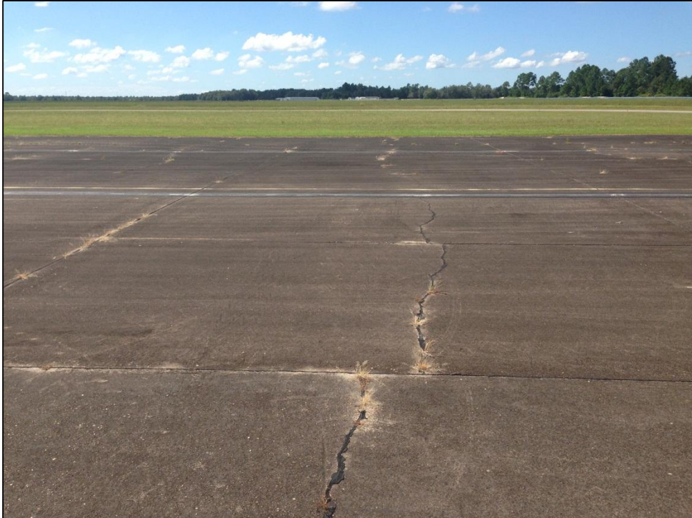
Runway 11-29, Section 6220, Sample Unit 103 – Medium Severity (65) Joint Seal Damage, Low Severity (63) Longitudinal, Transverse, and Diagonal Cracking
