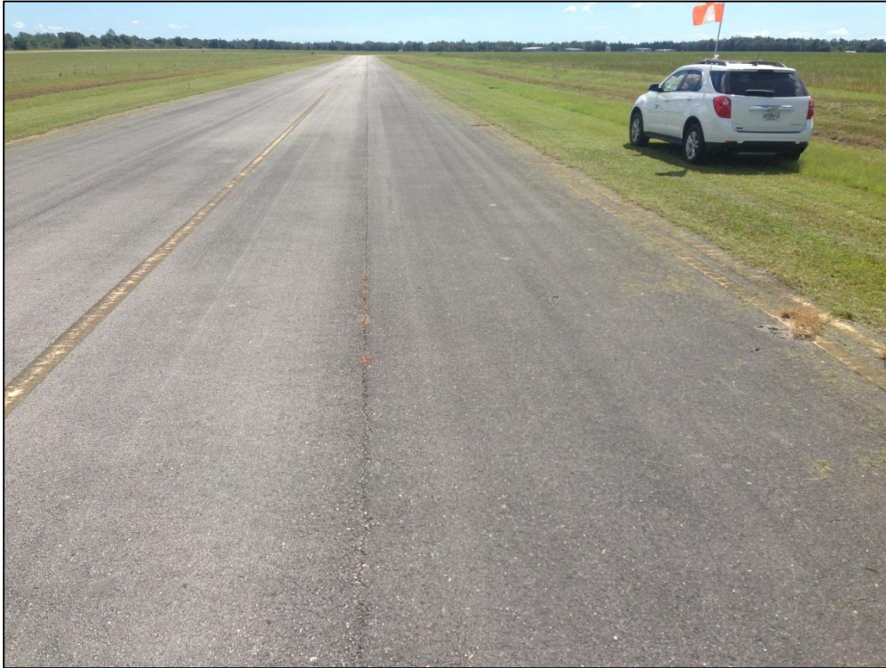
Taxiway C, Section 305, Sample Unit 132 – Low Severity (48) Longitudinal and Transverse Cracking, Low Severity (52) Raveling, Low Severity (57) Weathering
