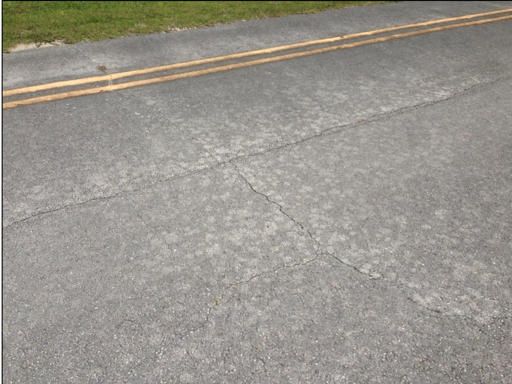
Taxiway B, Section 205, Sample Unit 101 – Low Severity (48) Longitudinal and Transverse Cracking, Low Severity (52) Raveling, Low Severity (57) Weathering
