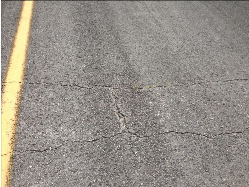
Taxiway A, Section 105, Sample Unit 153 – Low and Medium Severity (48) Longitudinal and Transverse Cracking, Low Severity (52) Raveling, Low Severity (57) Weathering
