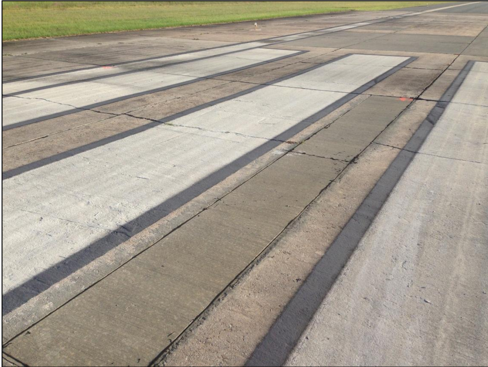
Runway 5-23, Section 6110, Sample Unit 96 – Medium Severity (65) Joint Seal Damage, Low Severity (63) Longitudinal, Transverse, and Diagonal Cracking, Low Severity (67) Large Patching
