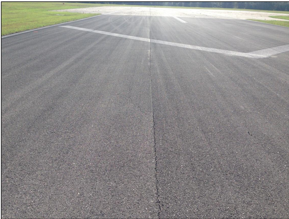
Runway 11-29, Section 6215, Sample Unit 192 – Low Severity (48) Longitudinal and Transverse Cracking, Low Severity (52) Raveling, Low Severity (57) Weathering
