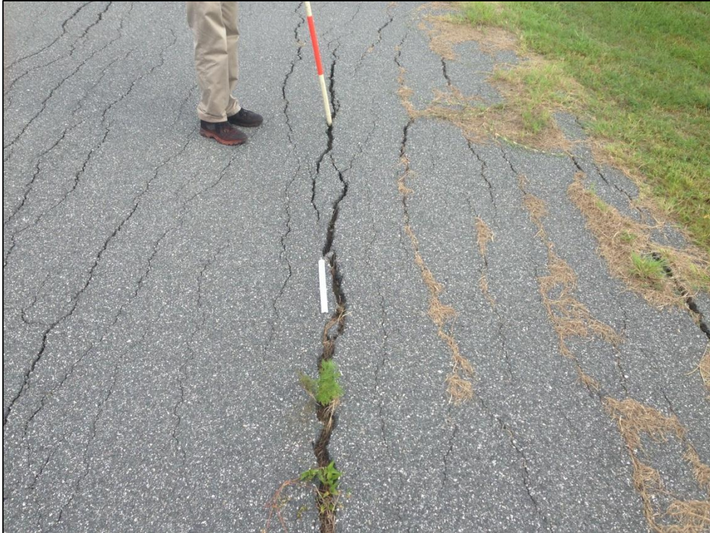
Apron T-Hang, Section 4520, Sample Unit 402 – Low and High Severity (48) Longitudinal and Transverse Cracking, Low Severity (57) Weathering, High Severity (56) Swelling
