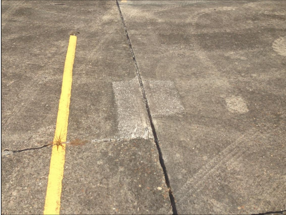
Apron, Section 4105, Sample Unit 500 – Medium Severity (65) Joint Seal Damage, Low Severity (63) Longitudinal, Transverse, and Diagonal Cracking, Low and Medium Severity (66) Small Patching
