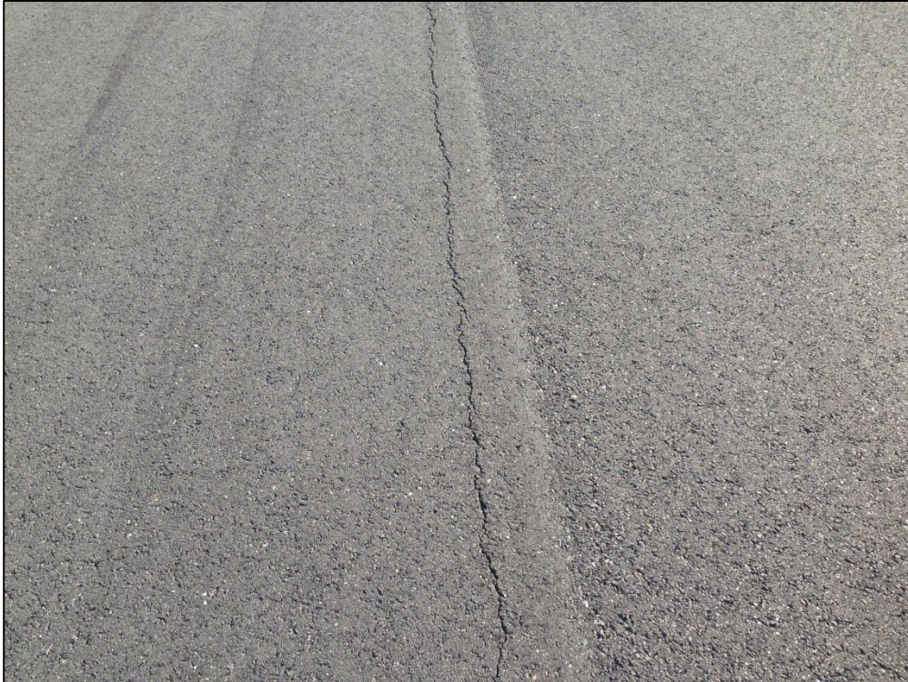
Runway 5-23, Section 6115, Sample Unit 307 – Low Severity (48) Longitudinal and Transverse Cracking
