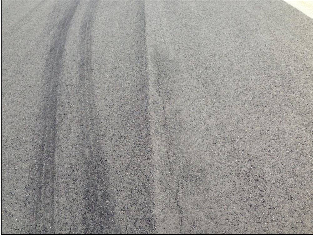
Runway 5-23, Section 6120, Sample Unit 504 – Low Severity (48) Longitudinal and Transverse Cracking
