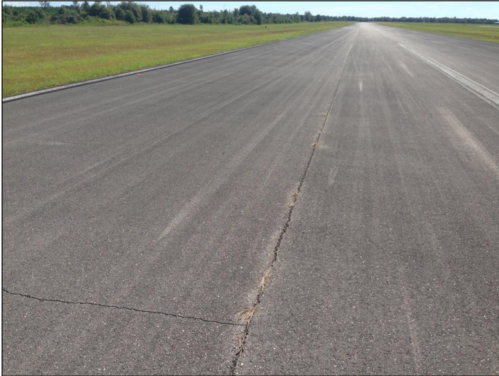
Runway 11-29, Section 6215, Sample Unit 111 – Low and Medium Severity (48) Longitudinal and Transverse Cracking, Low Severity (52) Raveling, Low Severity (57) Weathering
